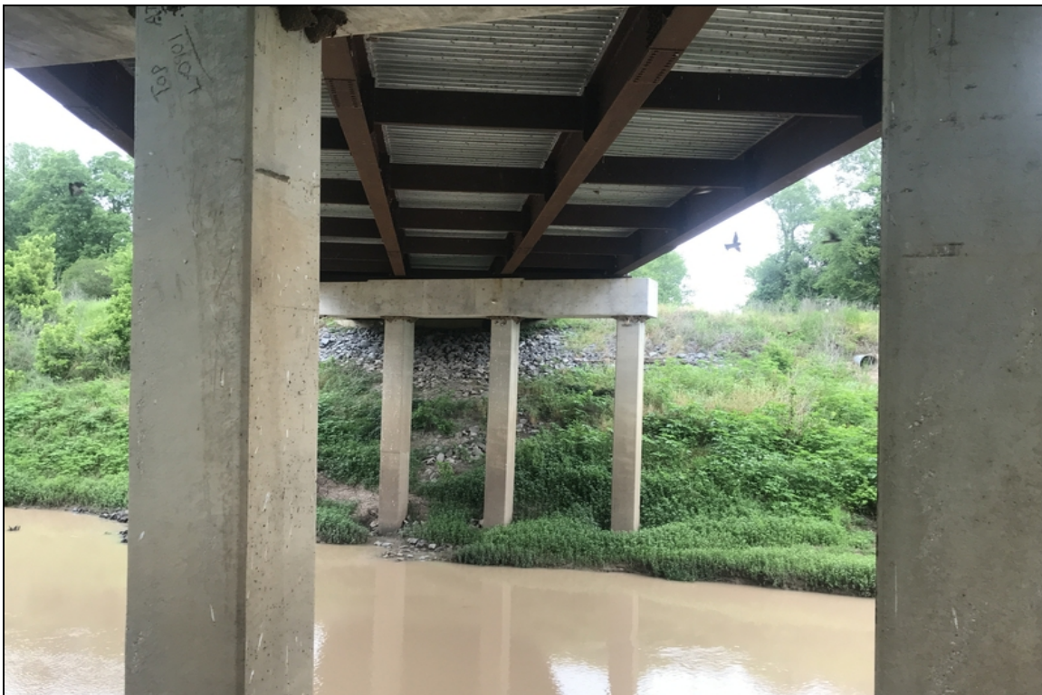
Overview of soffit and girders.
