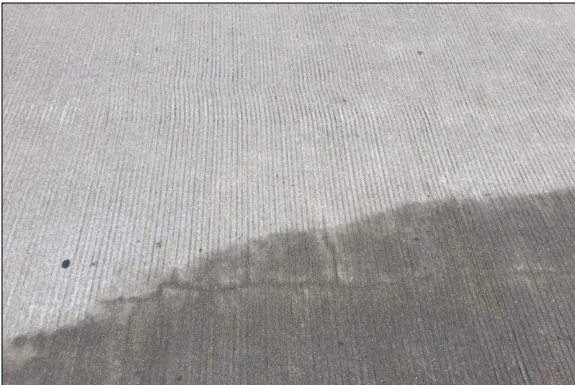
Deck cracking.
