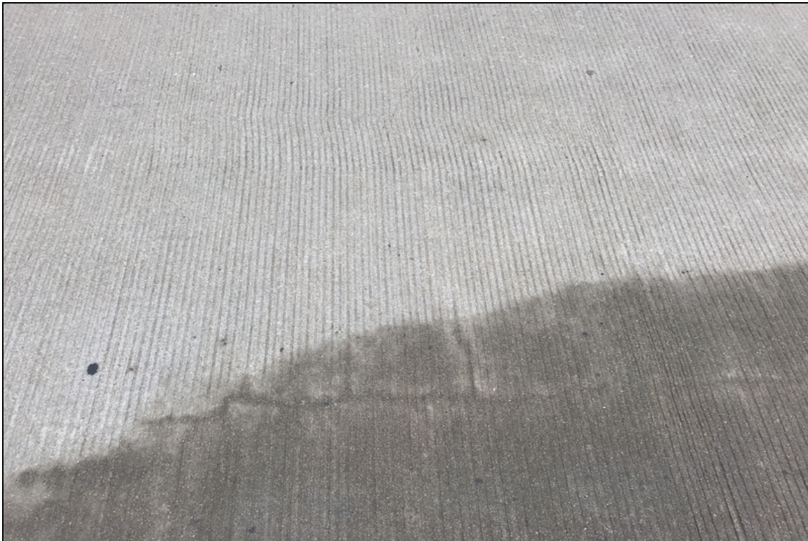
Deck cracking.
