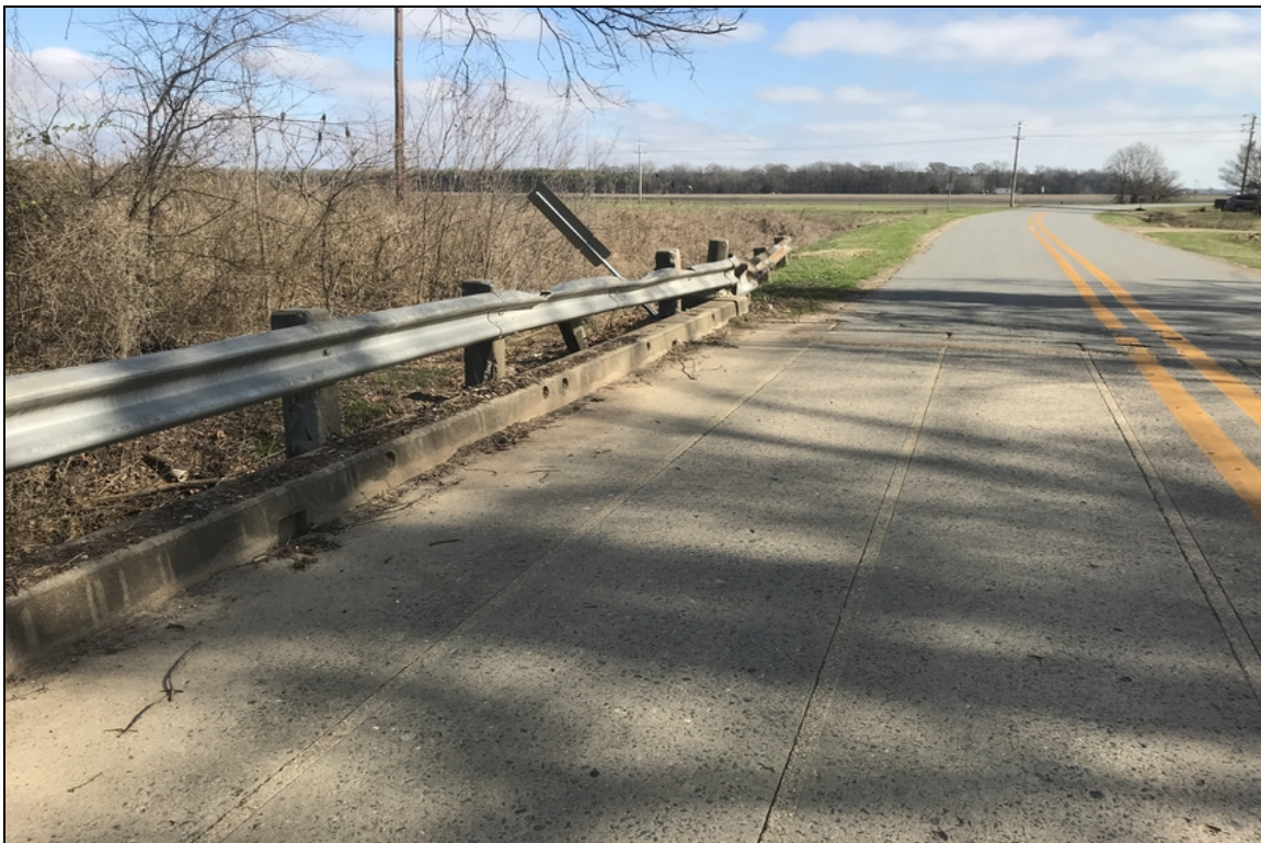
Gaurdrailing and concrete post damage at bent 9 left side ..
