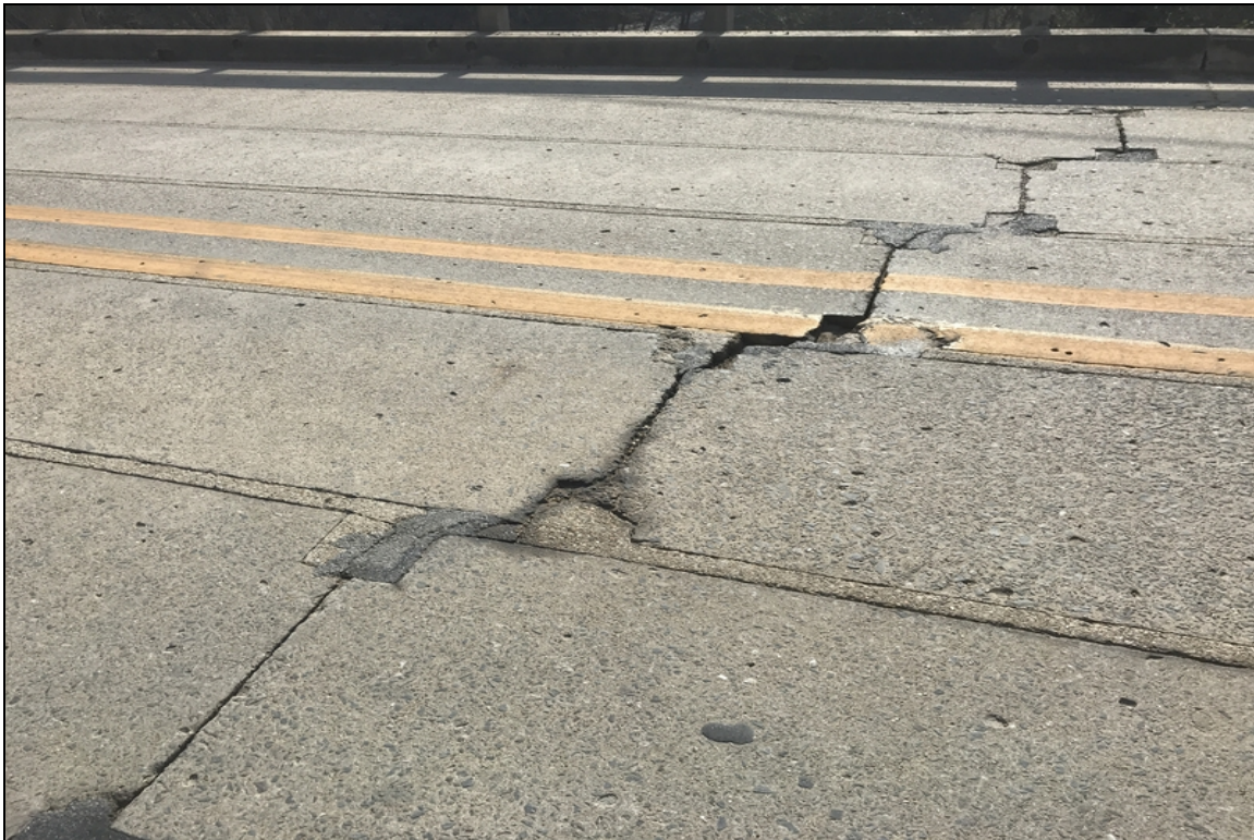
Spalls at ends of top flange deck slabs.
