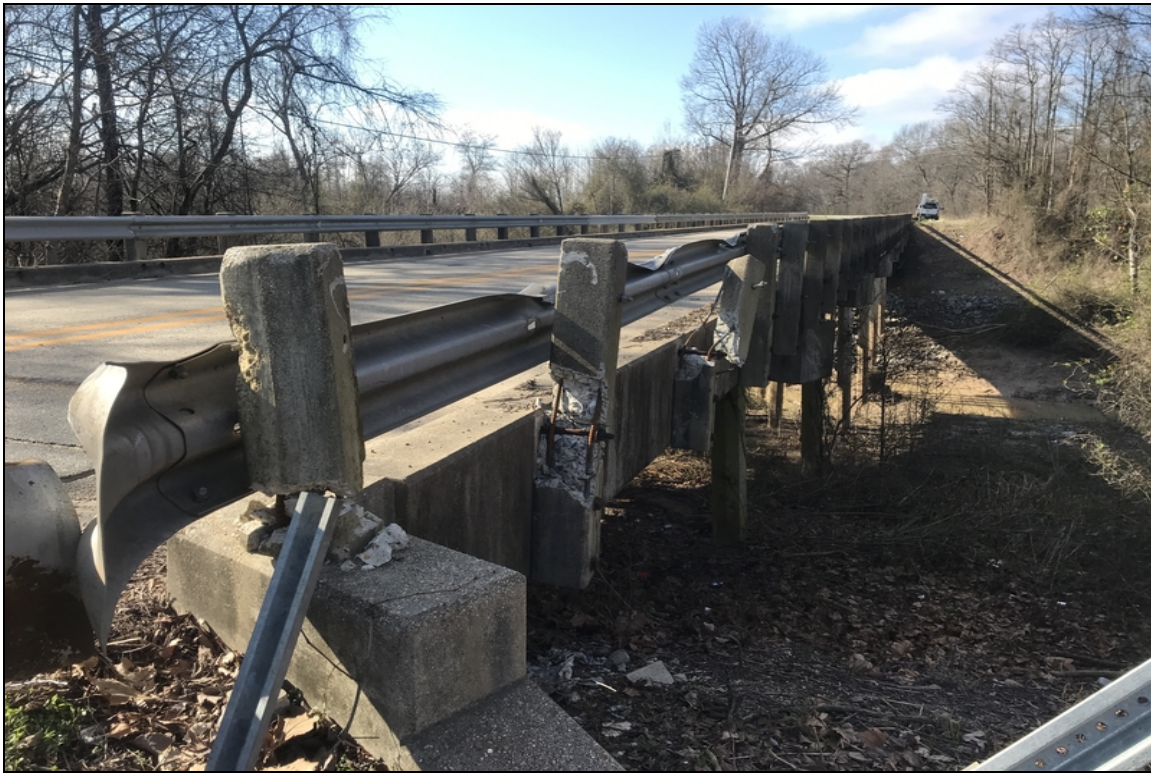
Concrete railing post damage at span 8 near bent 9.
