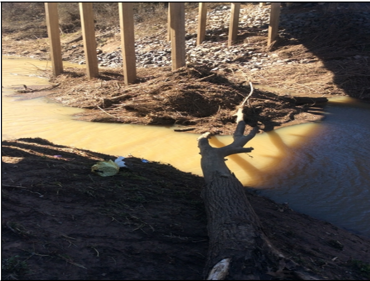
Channel - Bent 4: Debris
