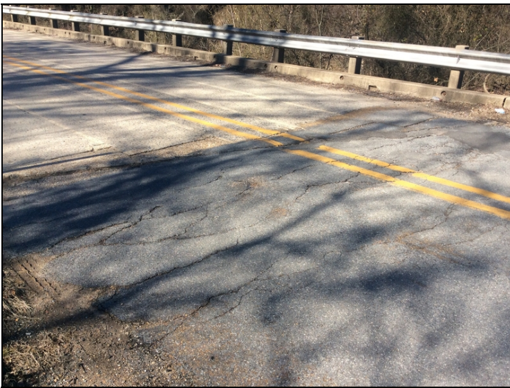
Approach roadway - Bent 8: Drop off
