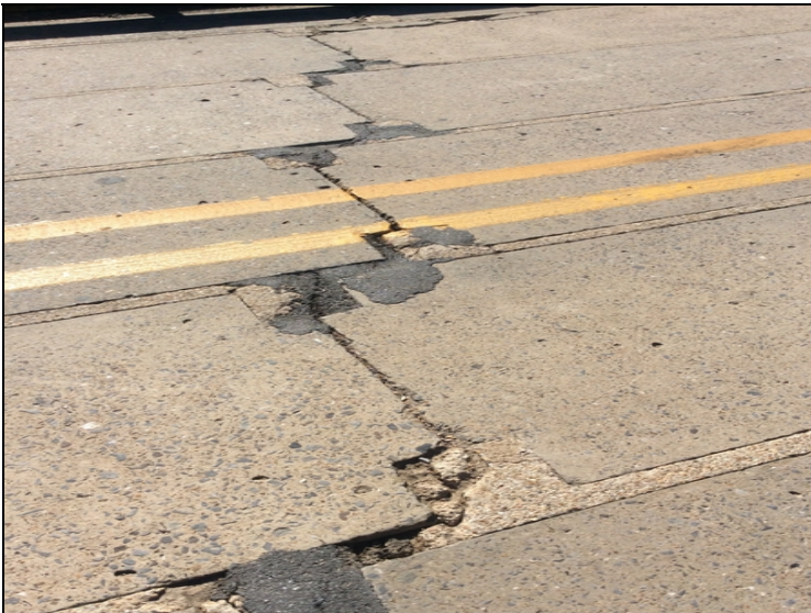
Deck - Bent 3: Spalls
