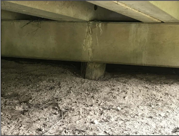
Bent 4 pile 4 has heavy decay.
