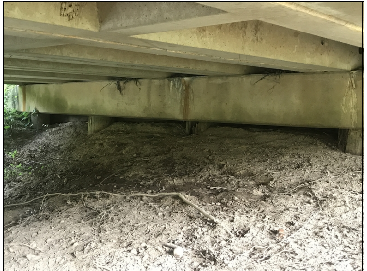
Bent 4 pile 2 and 3 have decay. Pile 3 has no bearing capacity.
