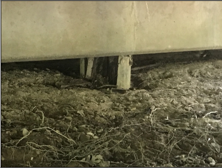
Bent 4 pile 4 hollow with heavy decay.
