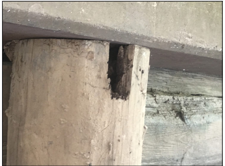
Bent 1 pile 3 hollow and decayed at cap.
