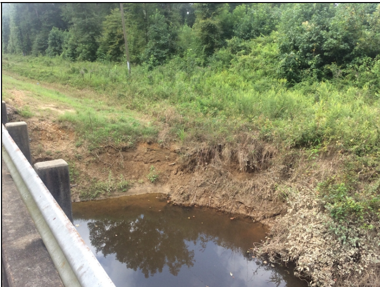
Channel - Spans 1 & 2 left: Erosion
