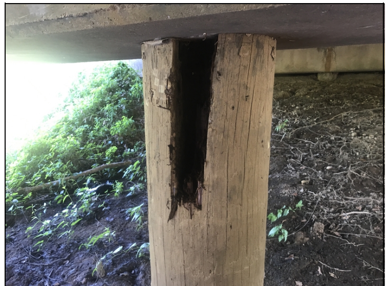
Bent 3 pile 3 heavy decay with small core.
