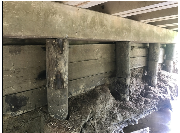
CORRECTED - Bent 1 Piles 1-4: Decay
