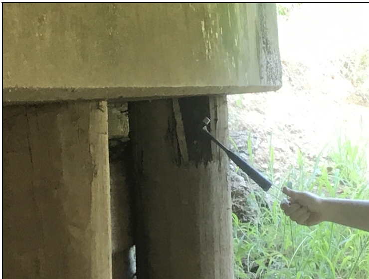
Bent 1 pile 1 hollow and decayed at cap.
