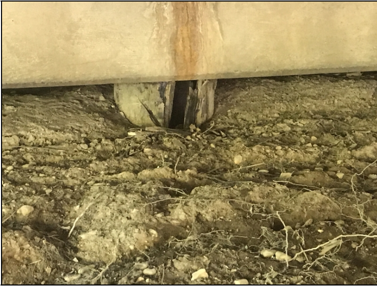
Bent 4 pile 3 hollow with heavy decay.
