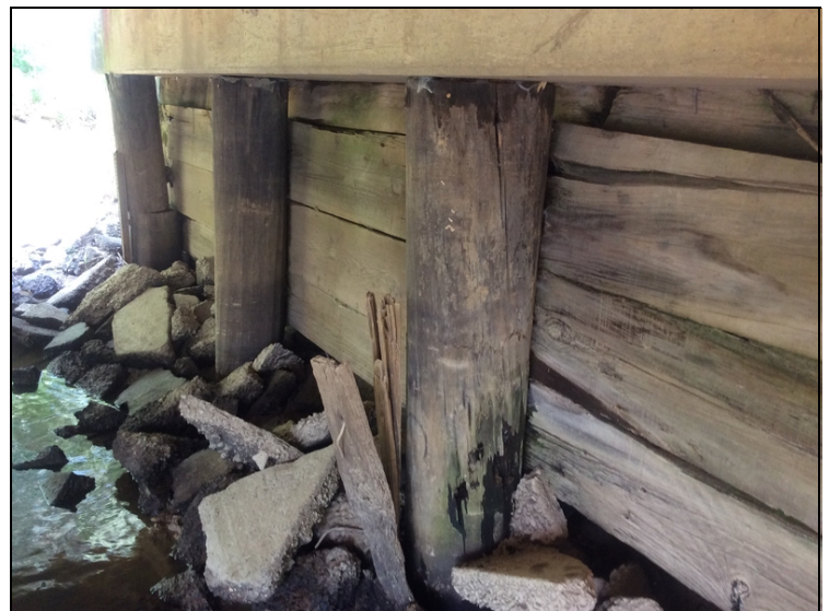
Bent 1 Piles 3-4 (decay)
