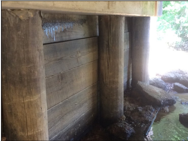
Bent 3 Pile 4 (decay)
