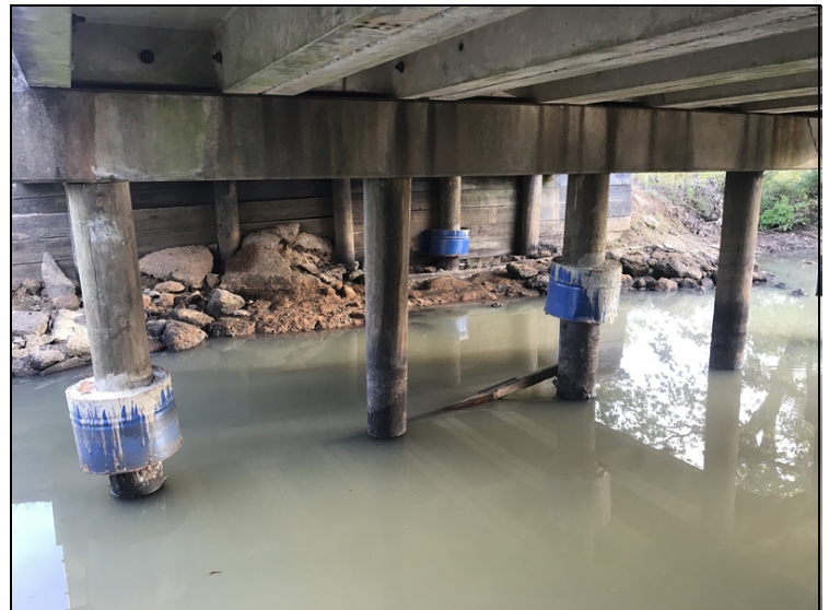
CORRECTED - Bents 2&3 pile repairs.
