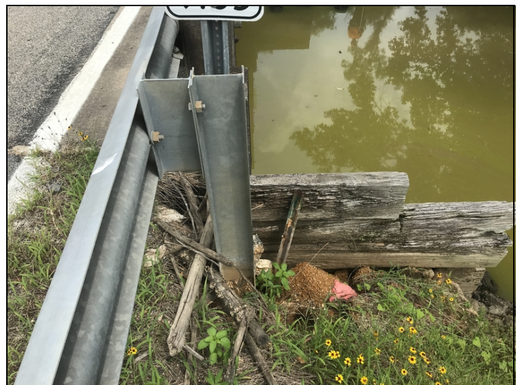
Approach roadway - Bent 1 right: Erosion
