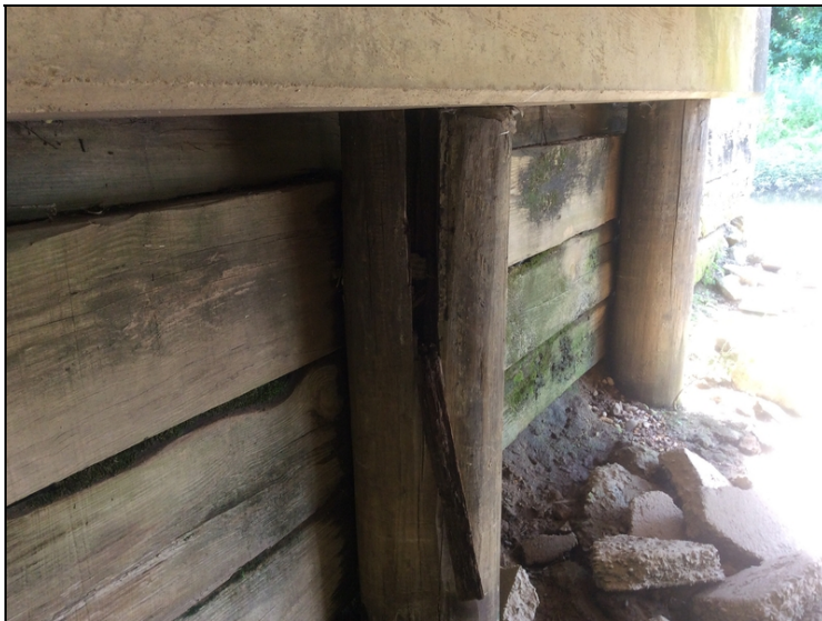
Bent 1 Piles 1-2 (decay)
