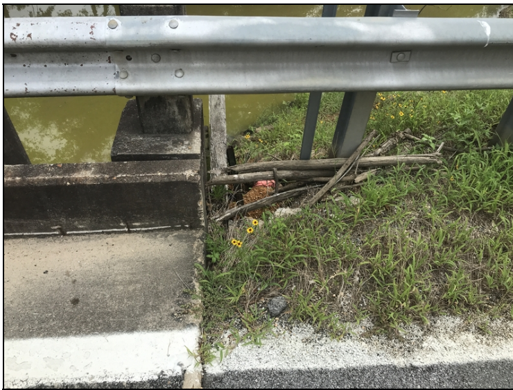
Approach roadway - Bent 1 right: Erosion
