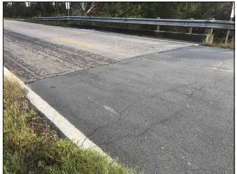
Approach roadway south end has settlement about 2-3 in drop.
