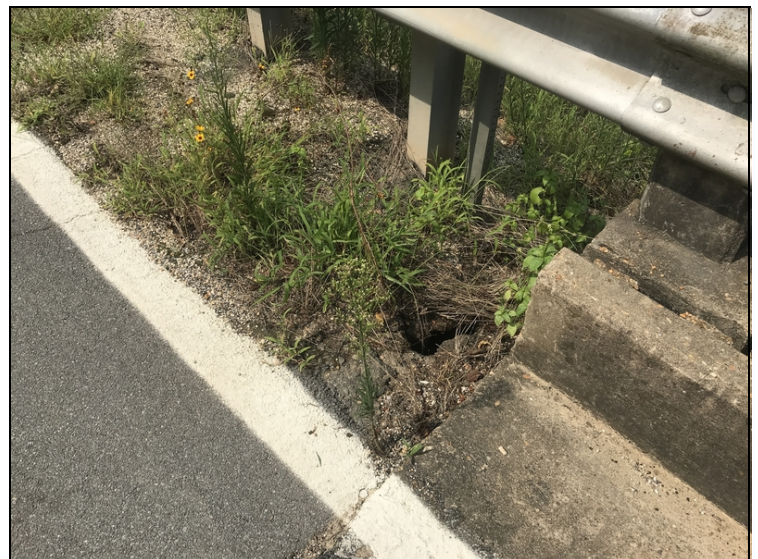
Approach roadway - Bent 1 left: Erosion
