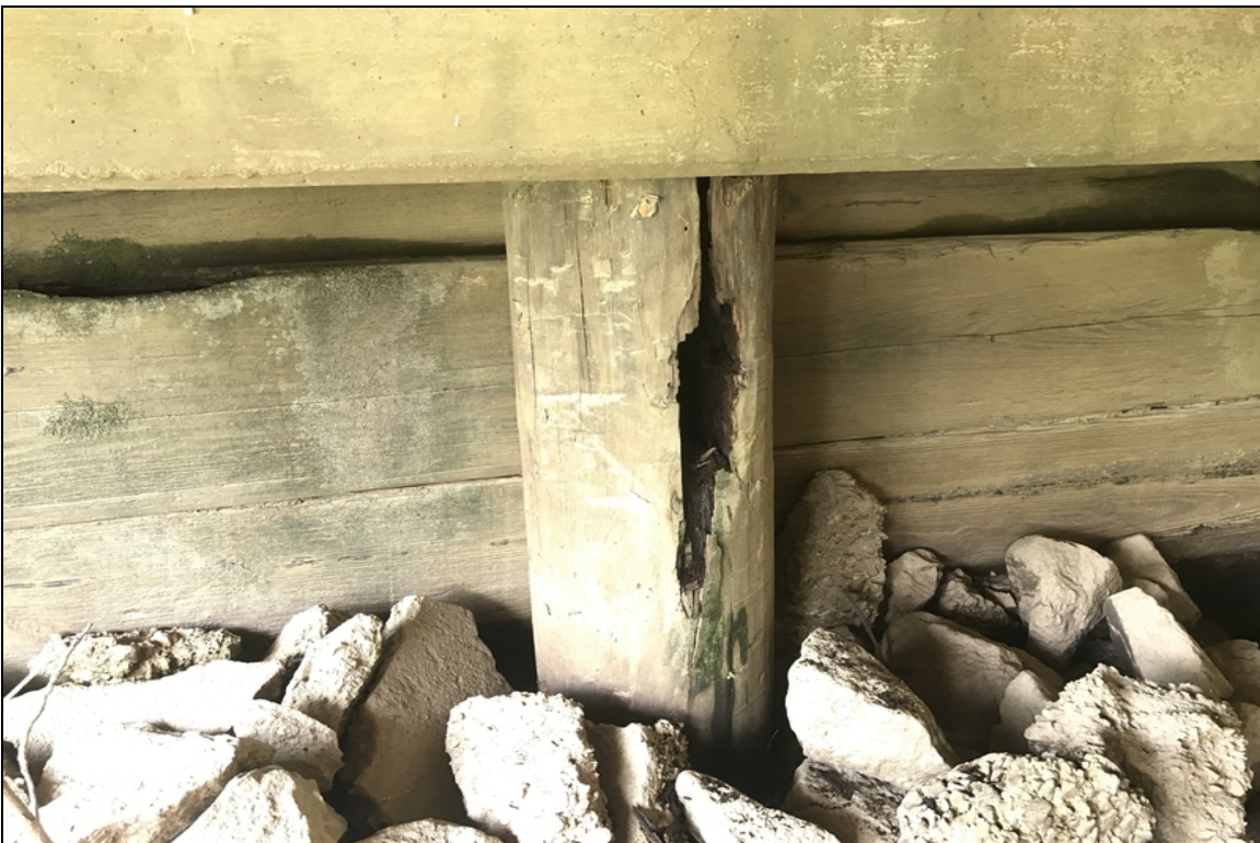
Bent 3 Pile 2: Decay
