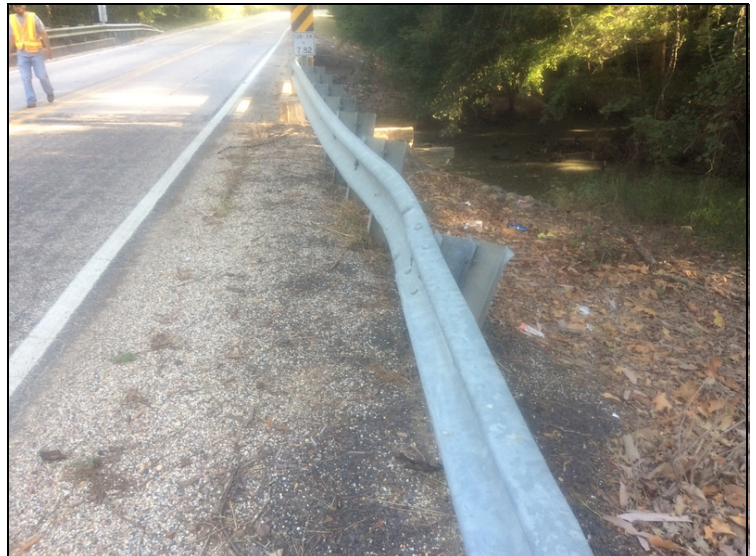
South east end of bridge, Guard rail damage
