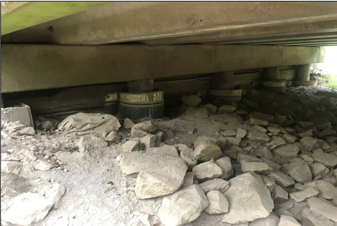
Bent 1 pile repaired.
