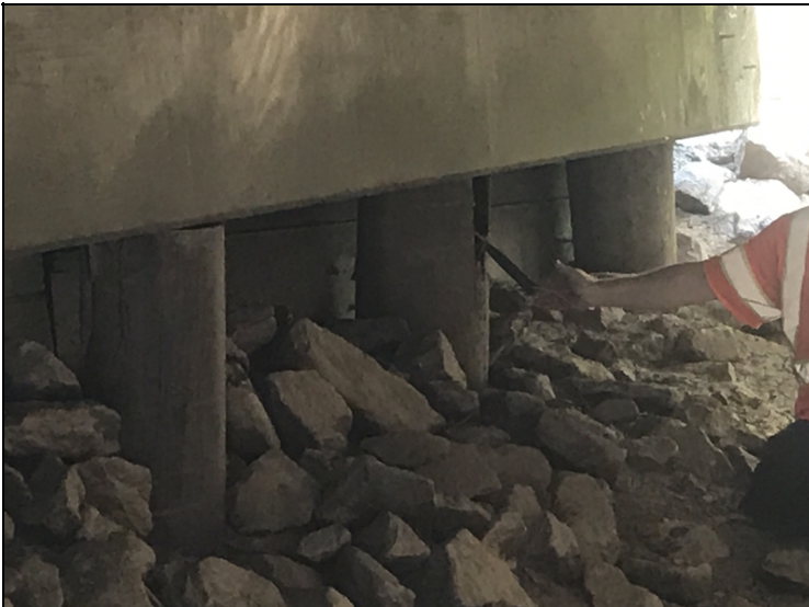
Bent 1 pile 2 hollow from cap down to ground line.
