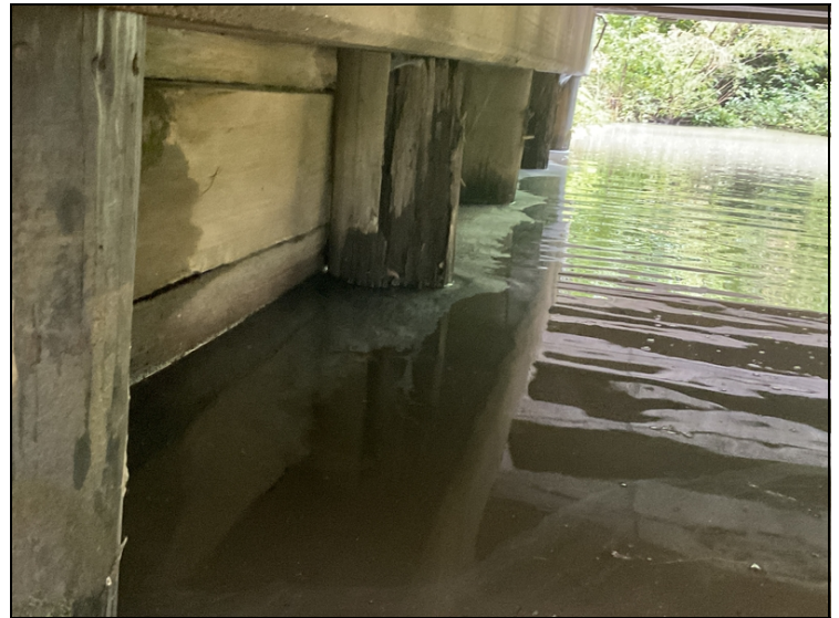
Bent 2 pile 2 has outer shell missing with heavy decay.
