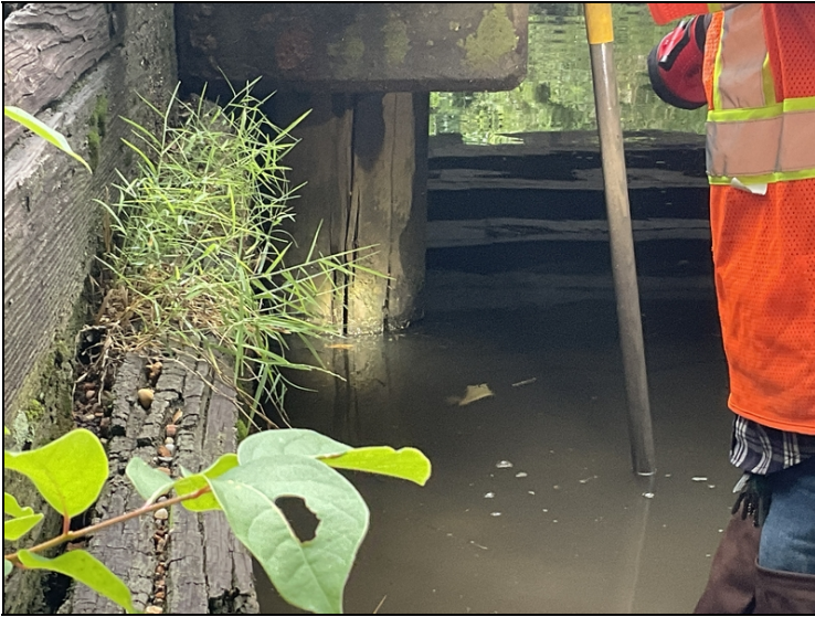
Bent 2 pile 1 has large checks.
