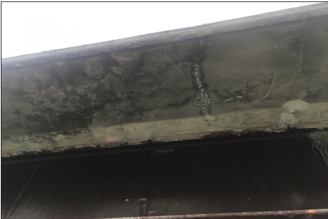
Soffit areas under walls have cracking with very light efflorescence beginning.
