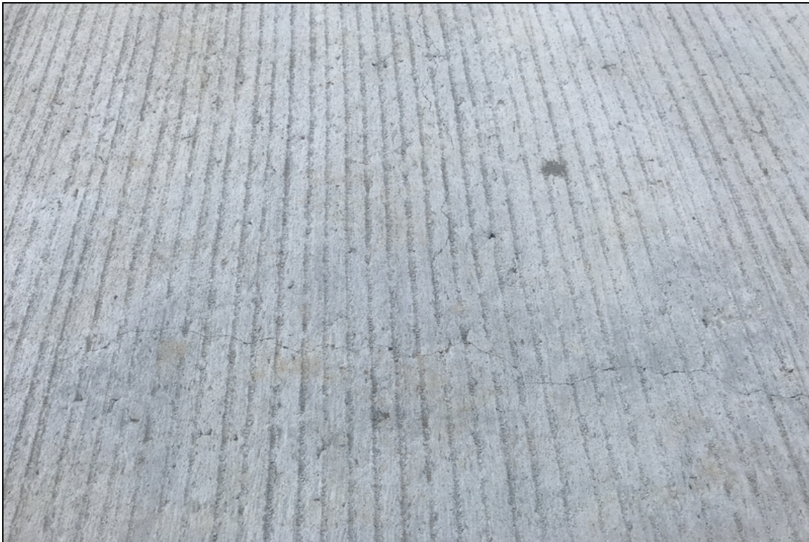
Deck. Span 2 & 3 have a couple of unsealed longitudinal and transverse cracks over girders 2 & 3.
