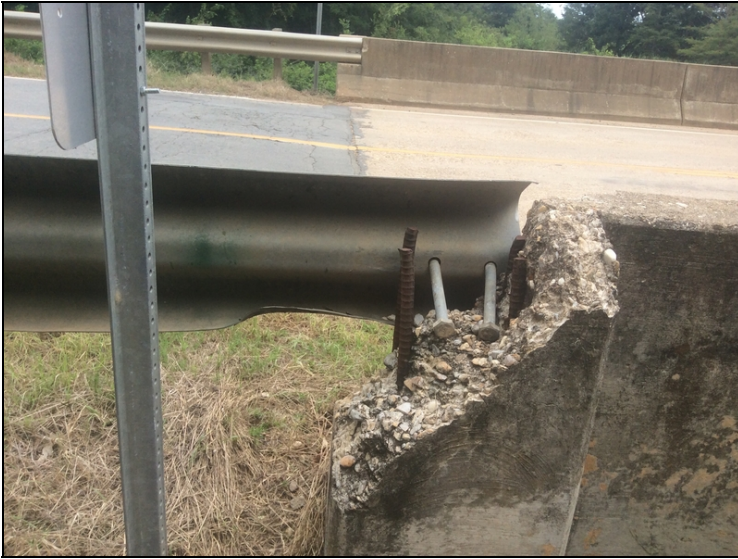
Bent 1 right side end rail has spall with exposed rebar.
