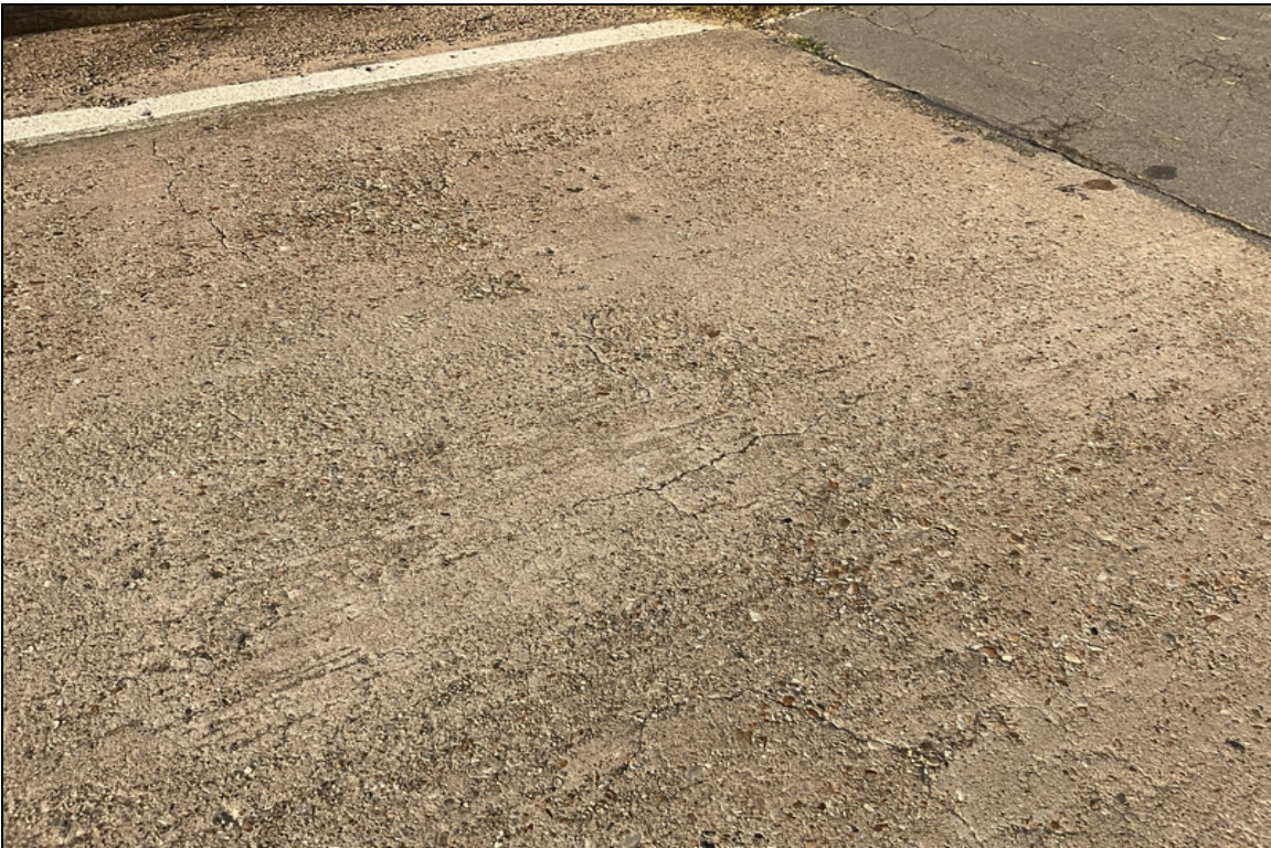
Moderate deck cracking at span 1 right lane. Common all spans.
