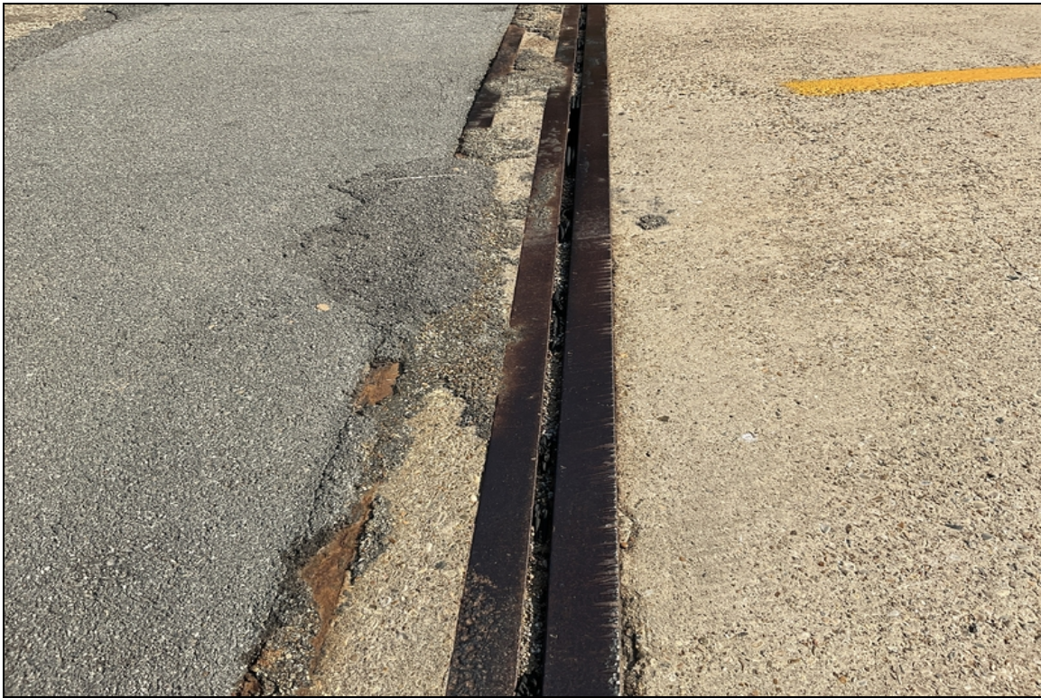
Span 1 joint seals are torn with small areas missing and have debris impactation.
