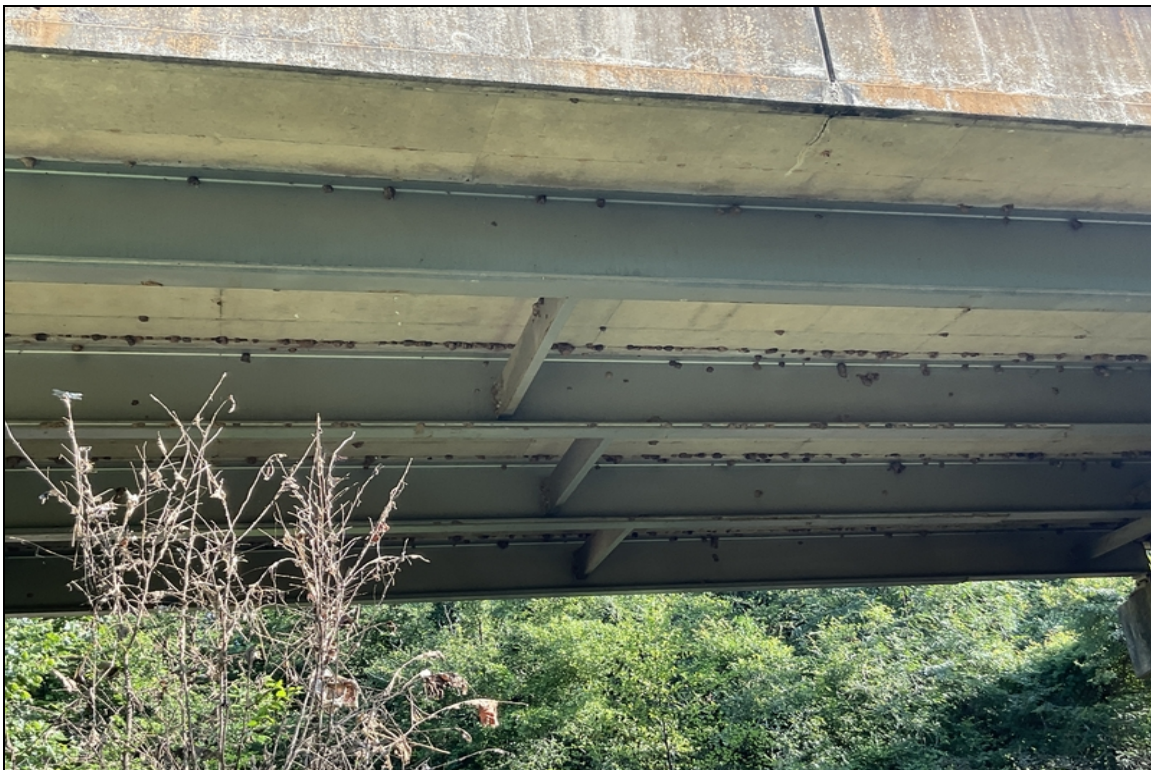
Typical paint condition.
