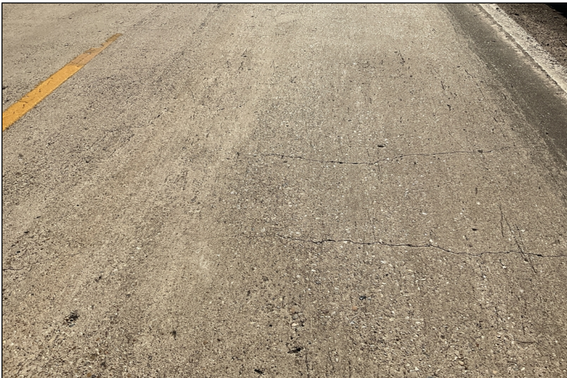
Deck span large unsealed cracks.
