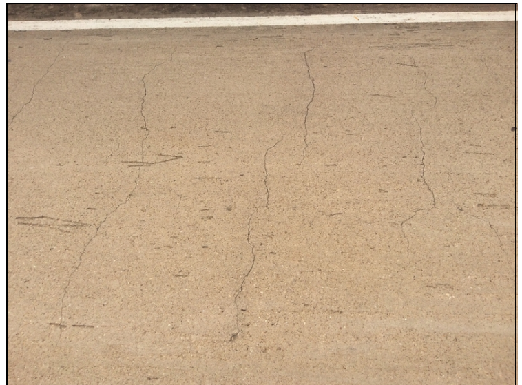
Deck span 4 has large unsealed cracks up to 0.060"
