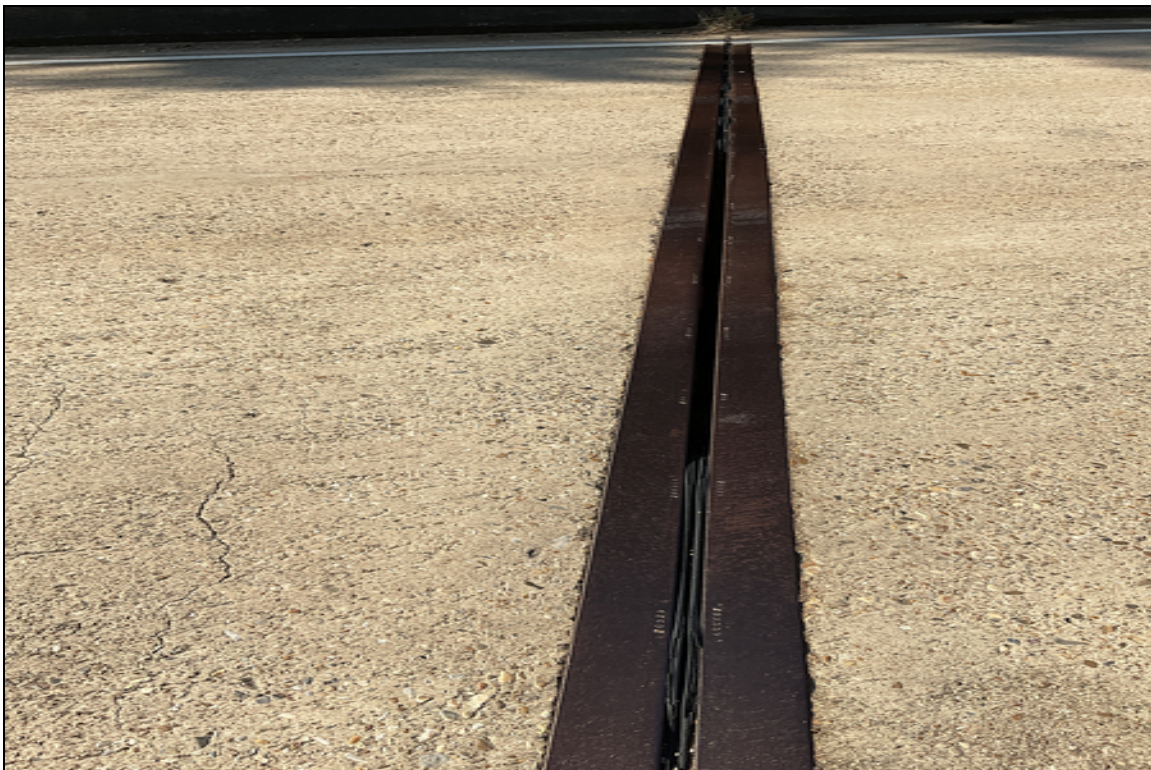
Bent 6 joint material missing.
