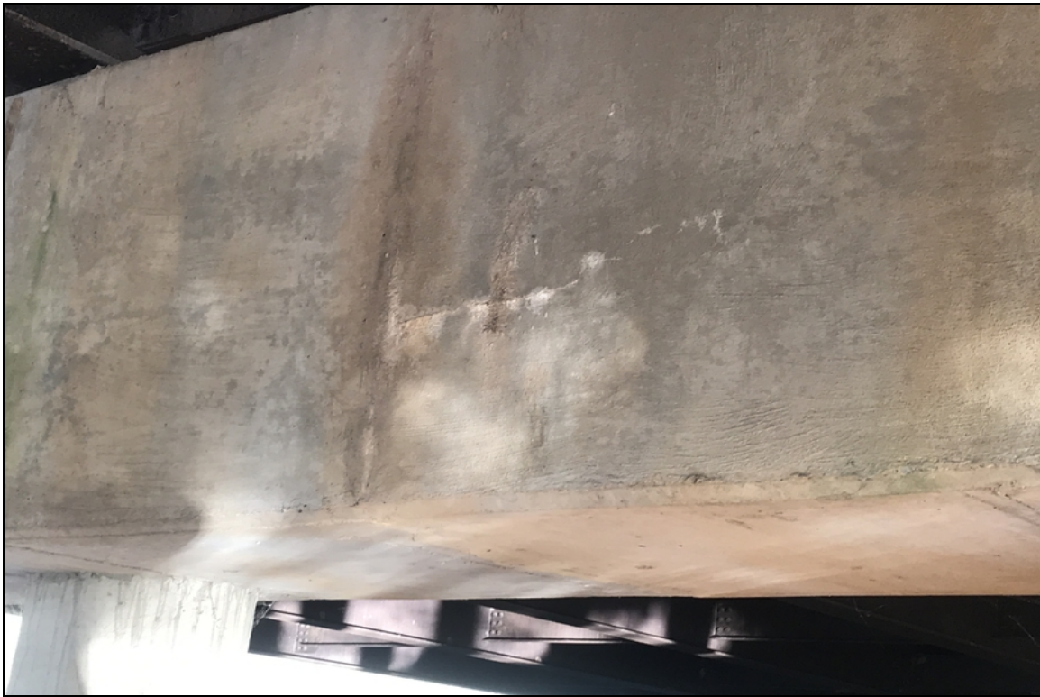
Bent 2 ahead has small horizontal crack with light efflorescence near cold joint.
