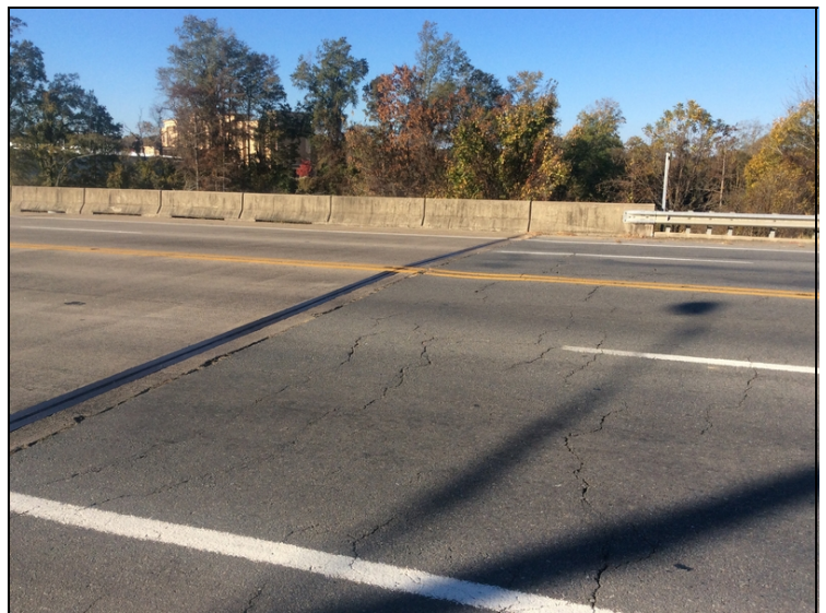
Approach roadway - Bent 1 (settlement)
