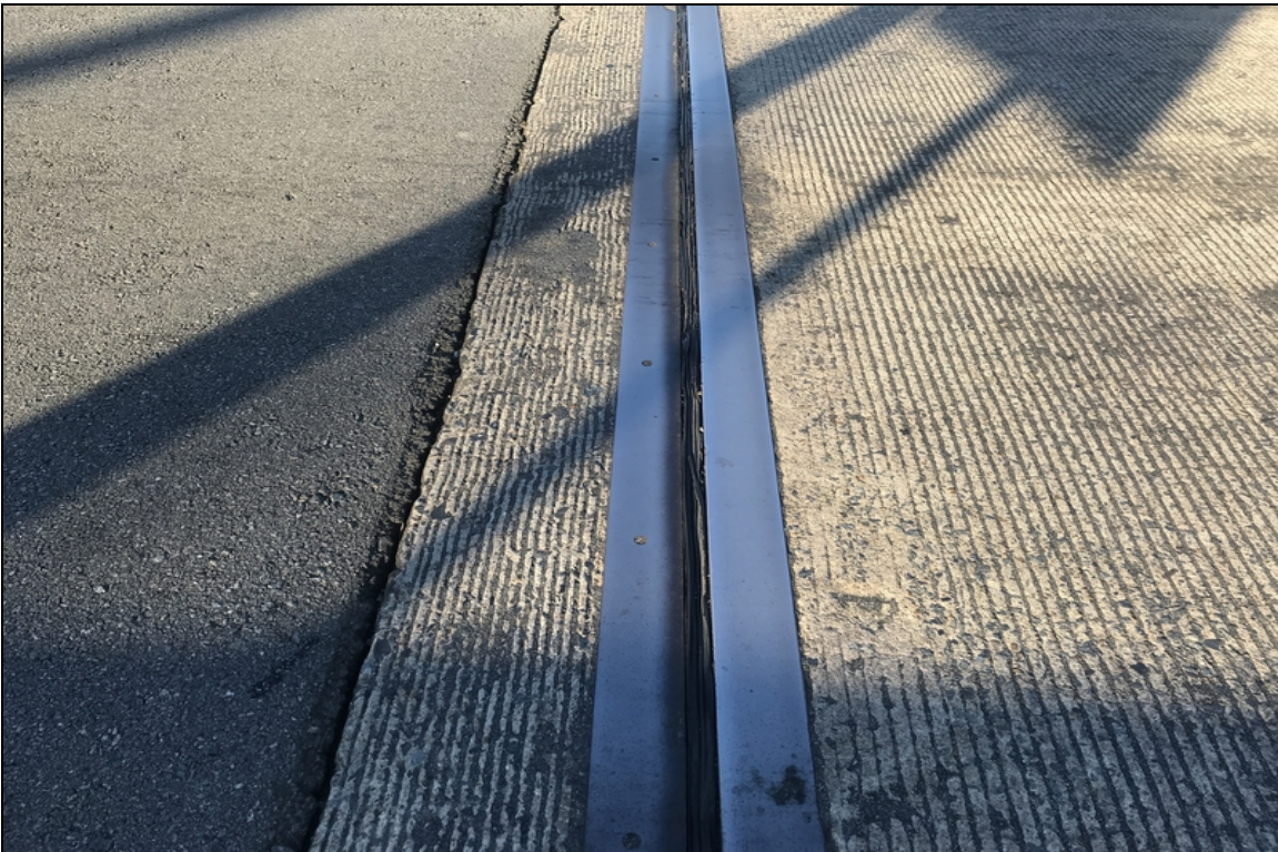
Joint seals torn and leaking.
