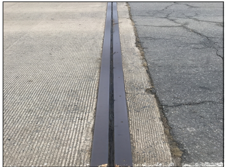
Joint - Bent 1 : Tattering
