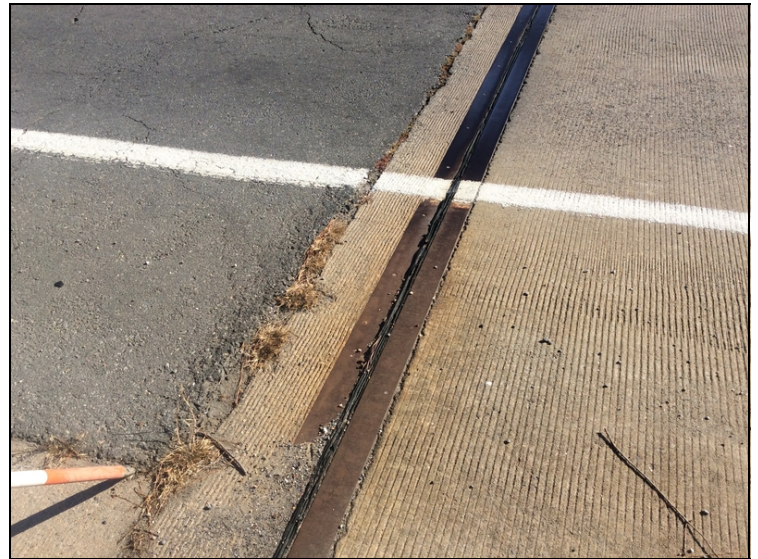
Joint - Bent 1 right (damage)
