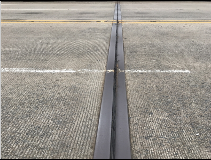
Joint - Bent 2 : Damaged
