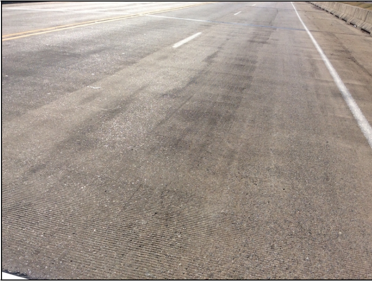
Deck - Span 1 (longitudinal cracking)
