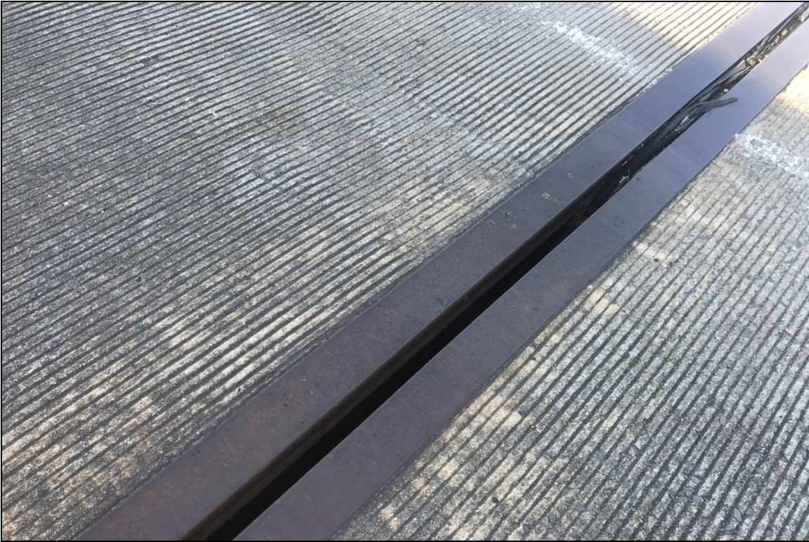
Bent 4 left seal missing in shoulder area.
