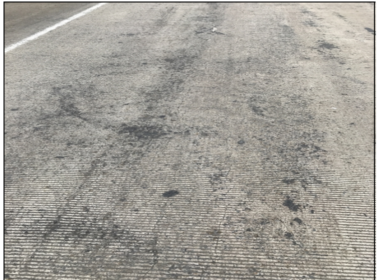
Deck - Span 6 left : Heavy cracking
