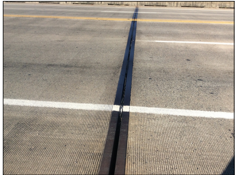
Joint - Bent 4 (damage & loss of adhesion)
