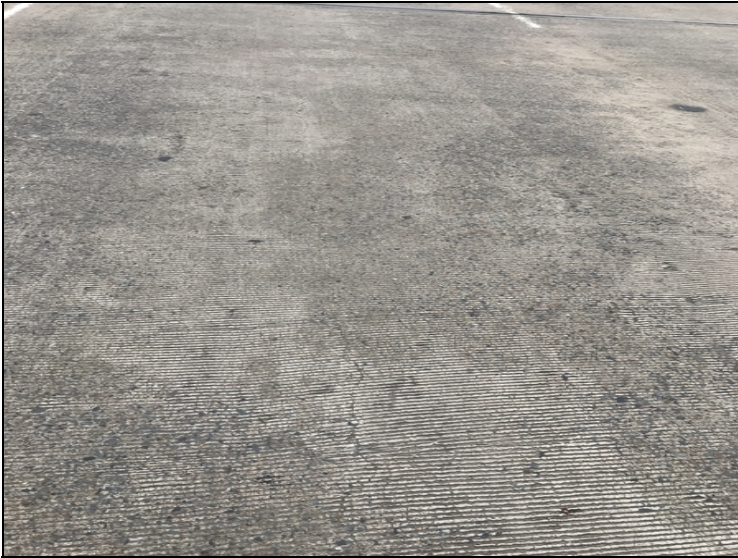
Deck - Span 2 left : Cracking
