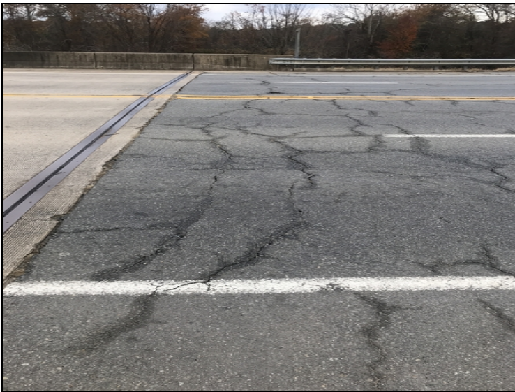
Approach roadway - Bent 1 : Pot hole and cracking
