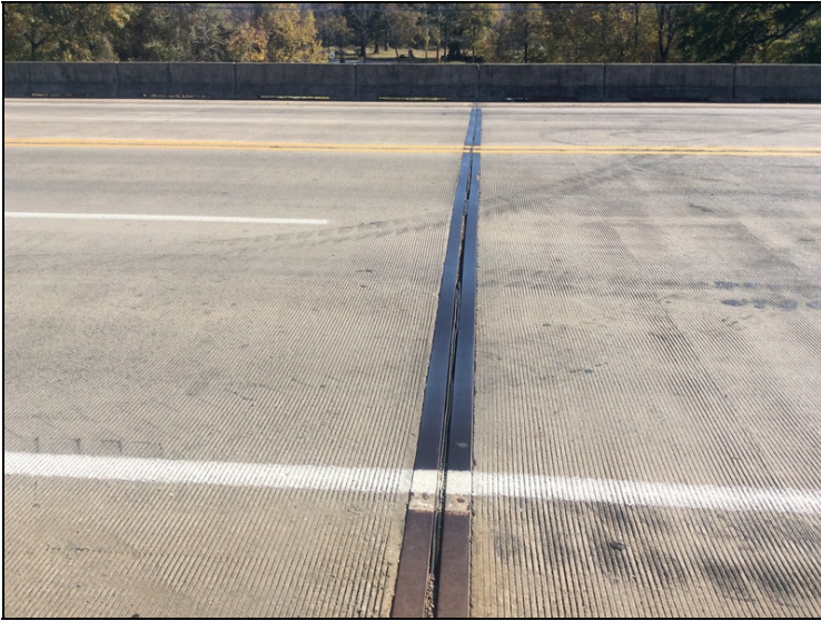
Joint - Bent 5 (loss of adhesion)
