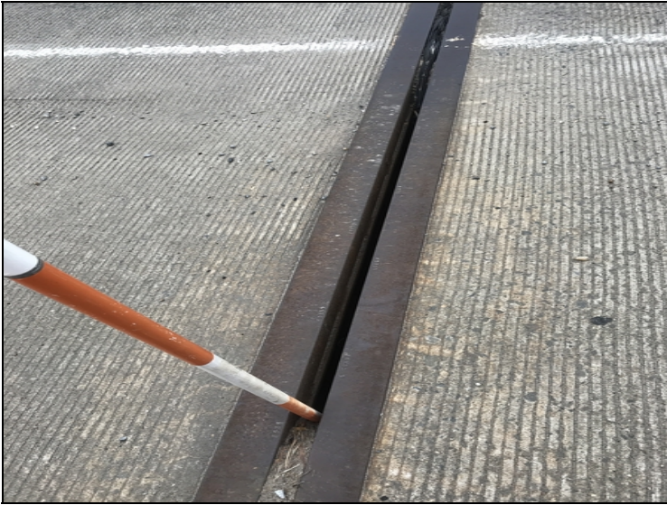
Joint - Bent 4: Loss of adhesion
