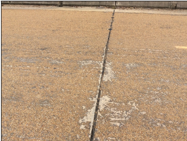
Joint - Bent 2: Loss of adhesion
