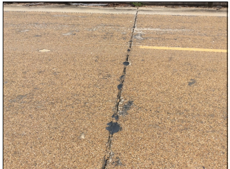
Joint - Bent 5: Loss of adhesion
