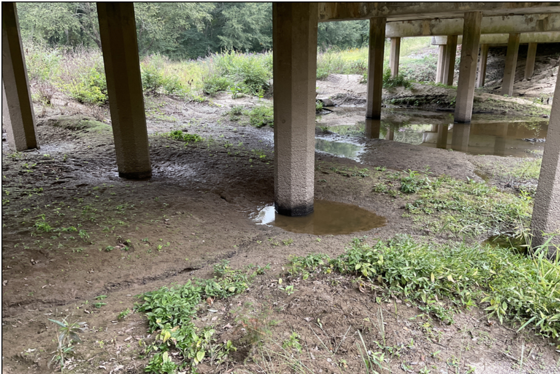
Localized scour at Bent 3. Common on most bents.
