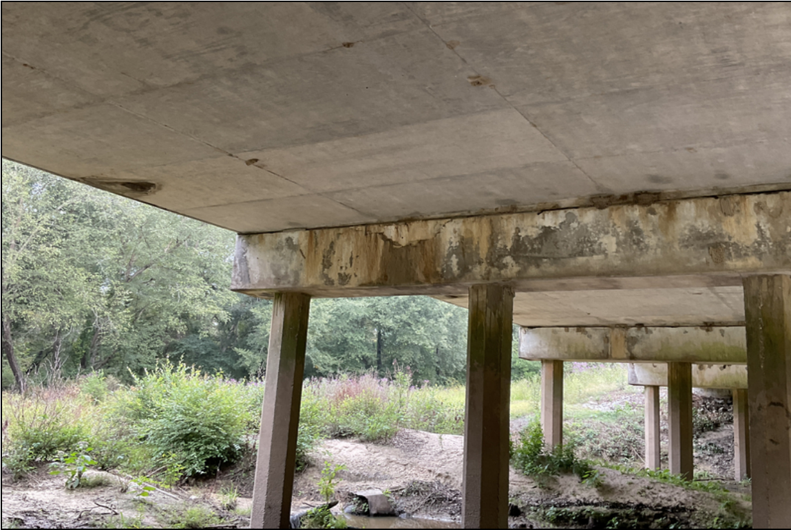
Bent 4 cap left back has delam.
