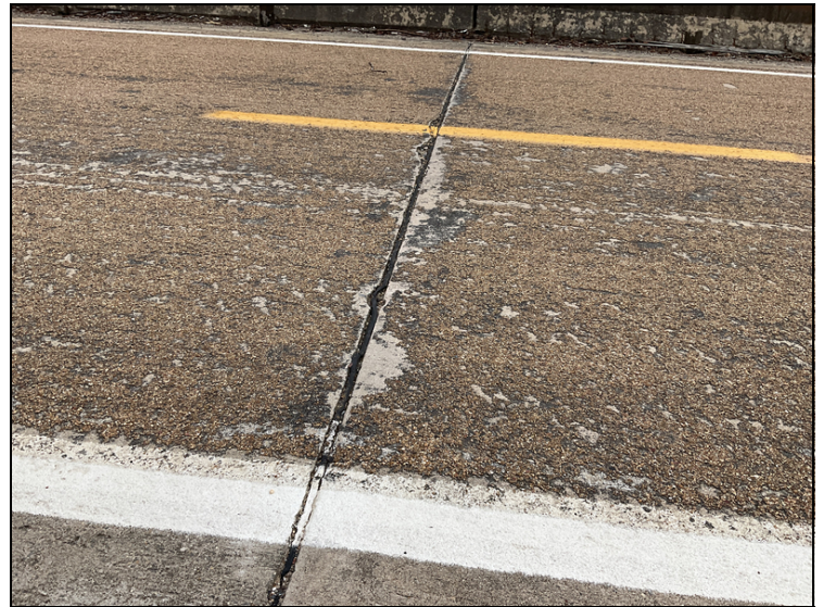
Bent 6 joint seal has loss of adhesion. Common on most joint seals.
