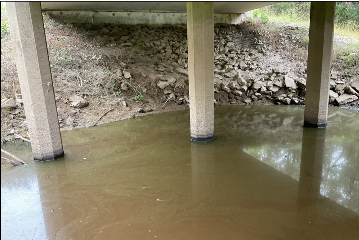
Abrasion on piles at Bent 2. Common on most piles at bents 2-5.
