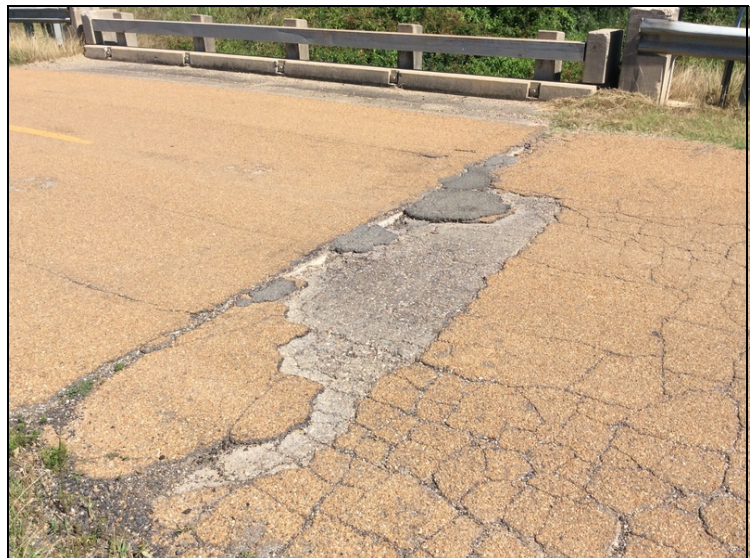
Approach roadway - Bent 2 (deterioration of wearing surface)
