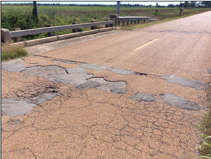
Approach roadway - Bent 1 (deterioration of wearing surface)
