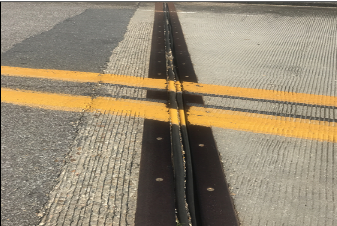
Bent 1 joint seal has small areas of loss of adhesion
