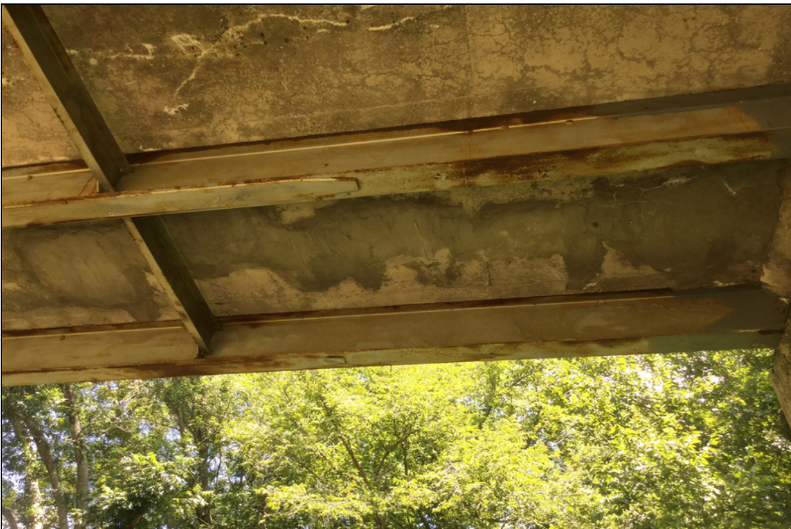
Span 6 left side patched area with grout
