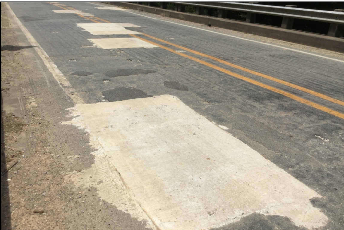
Span 6 repaired deck patches
