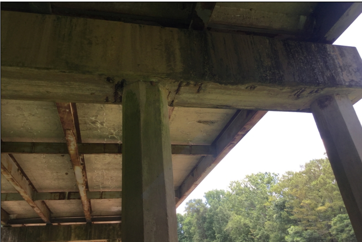
Cap 1 has cs3 rebar spalls on the under face of cap.
