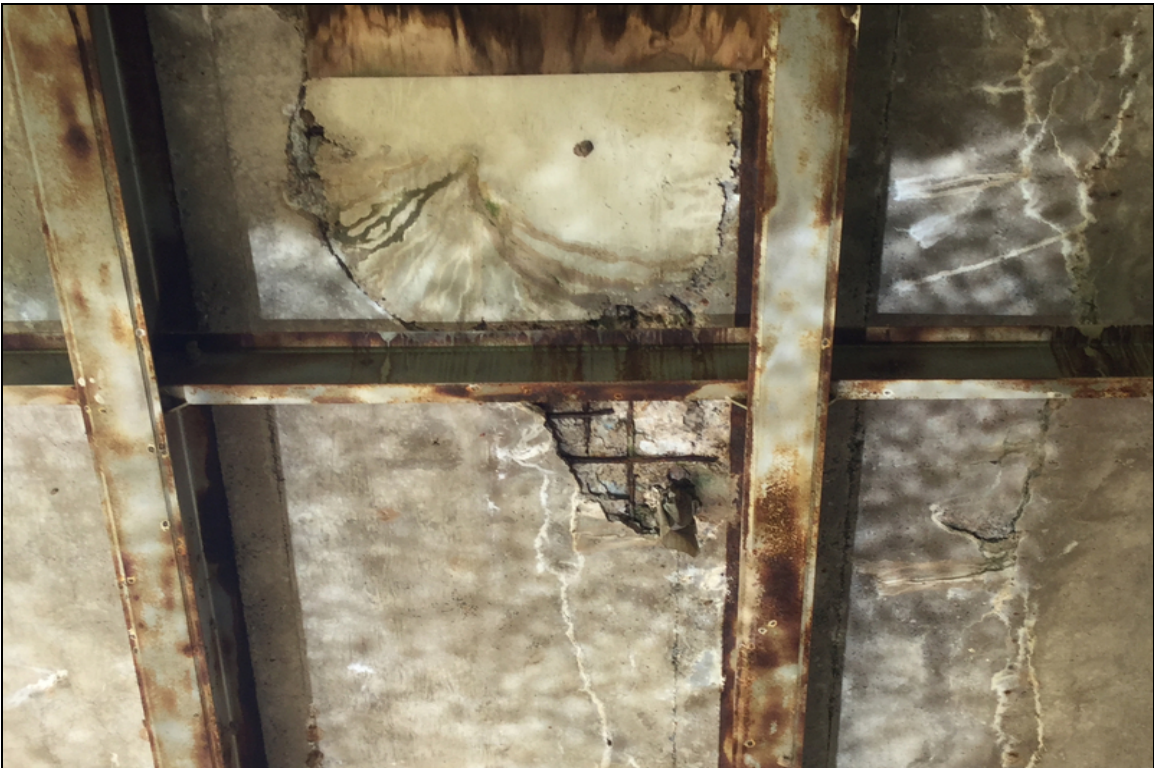
Span 5 rebar and repaired full depth failures
