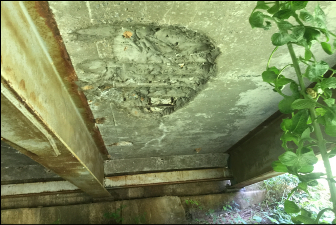
Span 7 bay 4 Cs3 rebar
