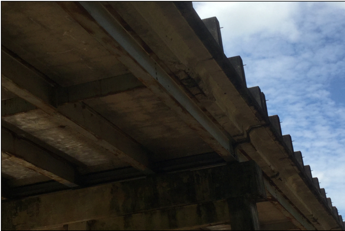
Typical Cs3 rebar on edges of soffit scattered throughout
