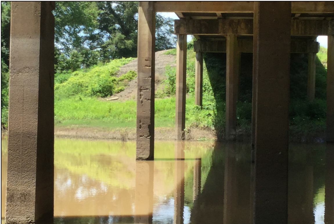
Cs3 rebar at bent 3 Column 3,2 bent 4 column 3,1; Bent 3 column 1 is CS2 rebar
