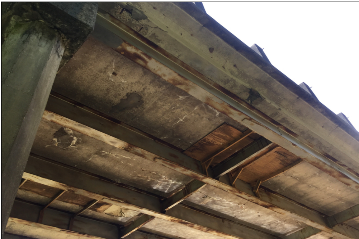
Span 5, 6 have three large repaired full depth failures
