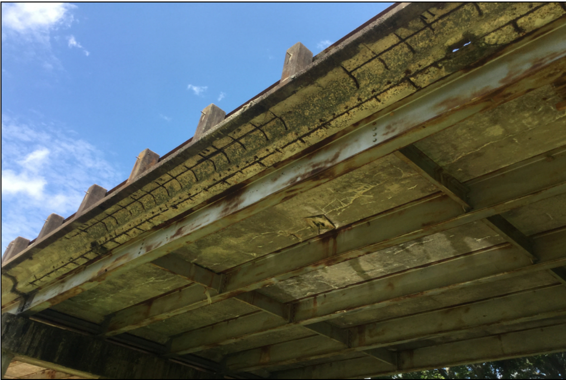
Span 6 right side soffit Cs3 rebar
