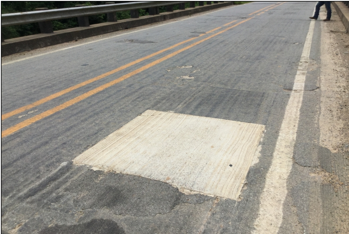
Span 2 Wearing surface has reflective cracking throughout and appears to have a lot of patched areas under asphalt. There is efflorescence cracking throughout under surface.
