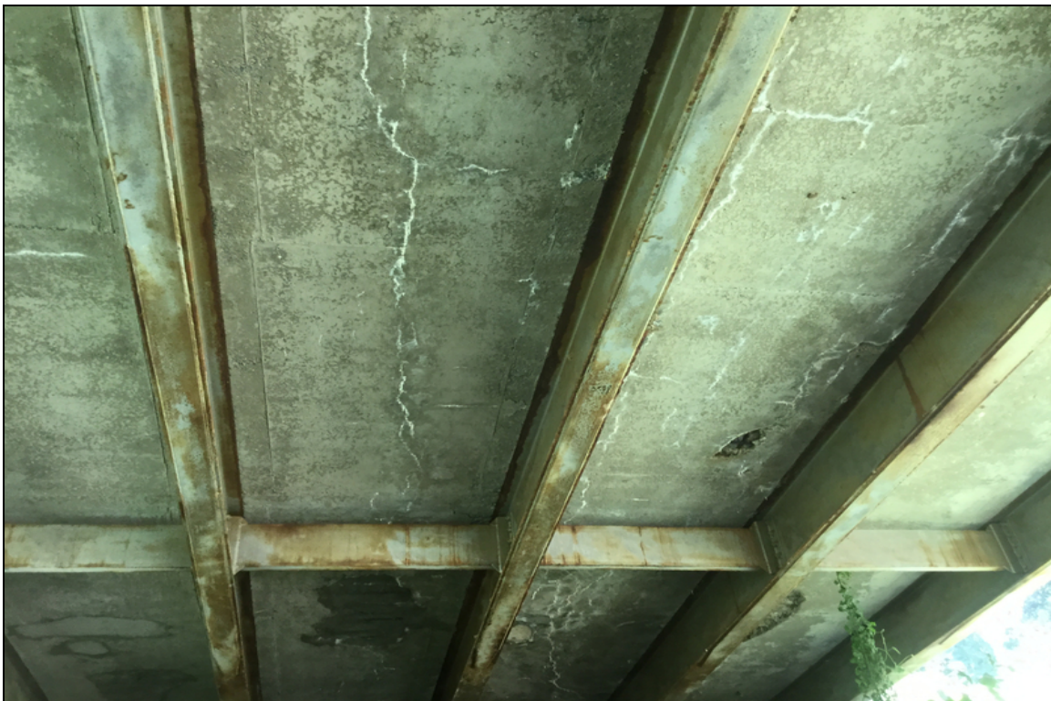
Span 7 cs3 efflorescence this is typical throughout under surface of the deck.
