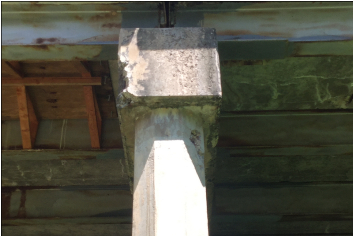
Bent 6 pile 4. Cap 6 spalling Cs3
