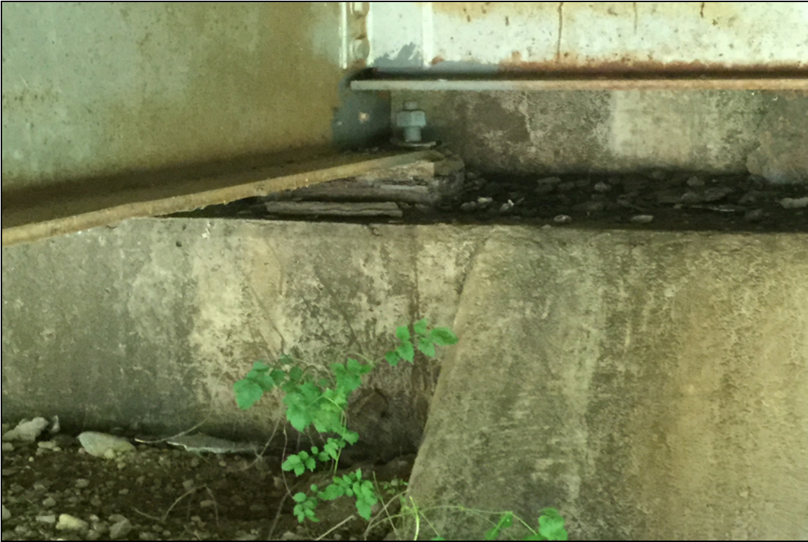
Abutment 2 bearing 4 pack rust Cs3 typical
