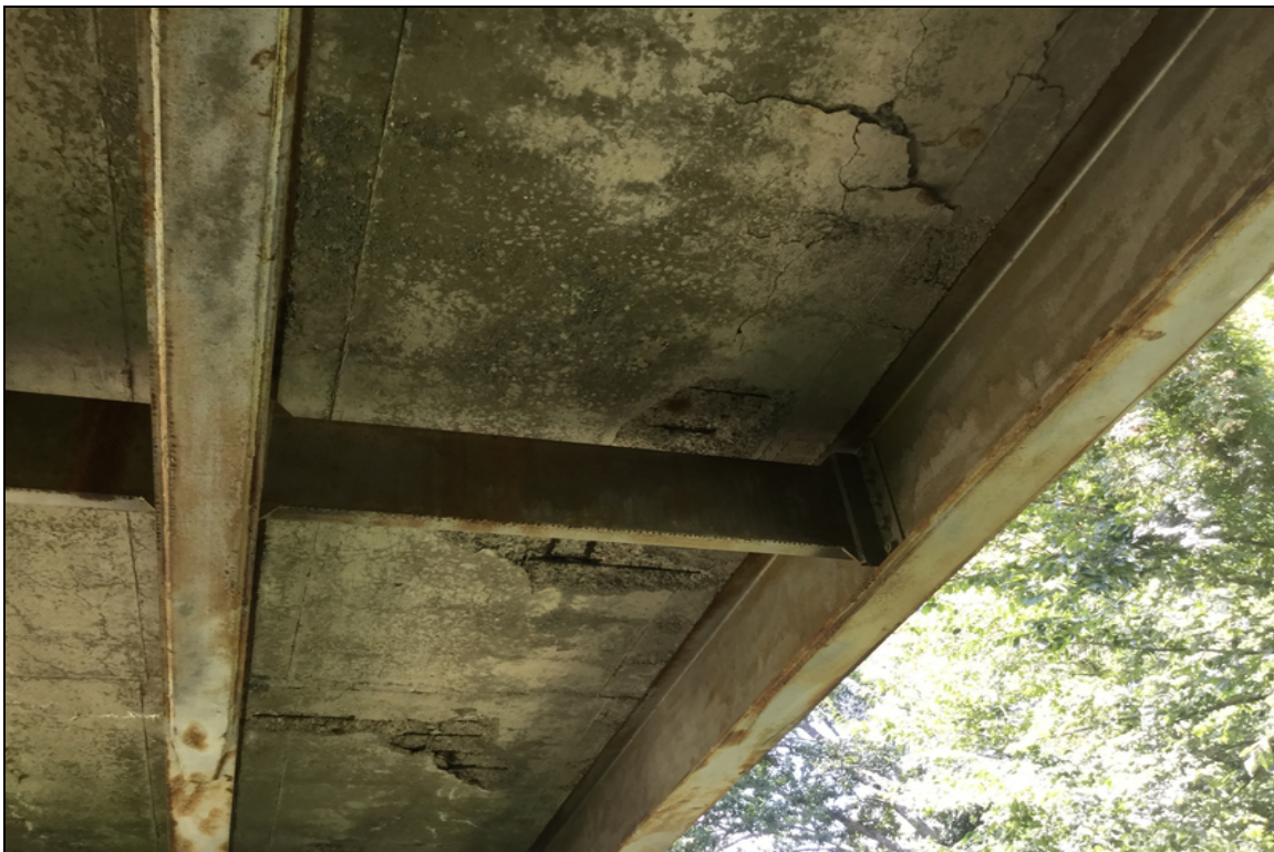
Span 7 bay 1 large Cs3 rebar areas and delam. This is typical in all spans
