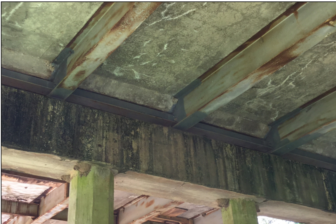
Ends of girders have had rust removed and repainted
