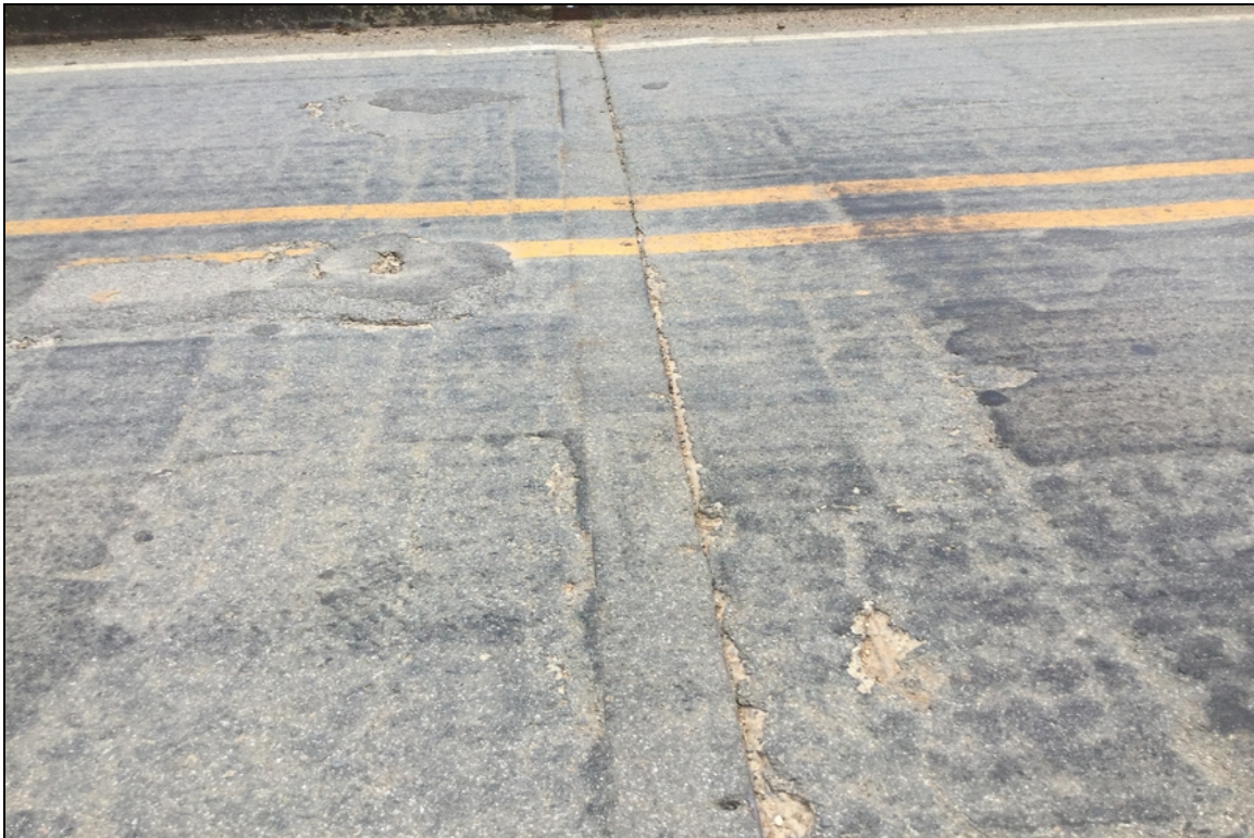
Bent 3 assembly joint typical
