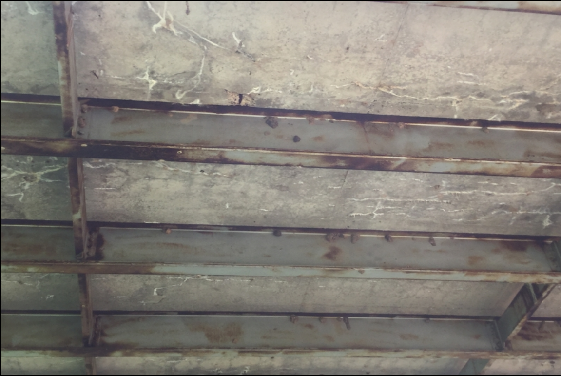
Span 2 girder 4 active Cs3 corrosion
