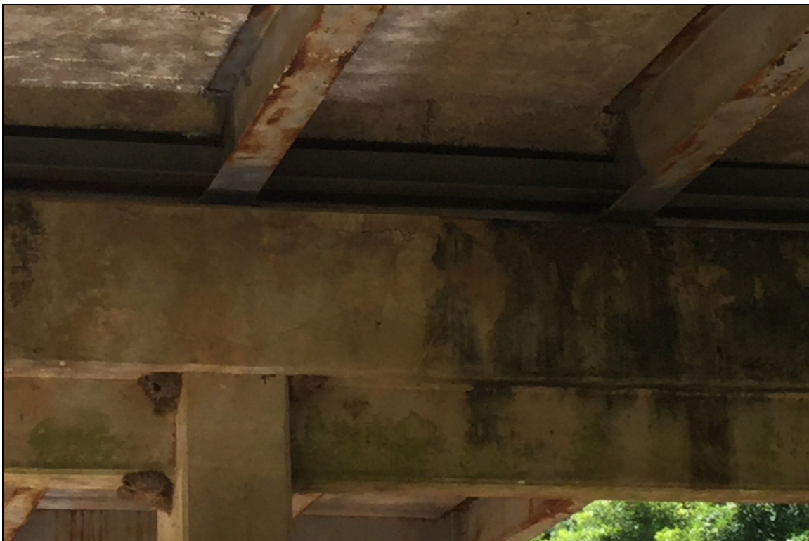
Cs3 cracking in cap 4 AHD side above column 2 this is typical at cap 3
