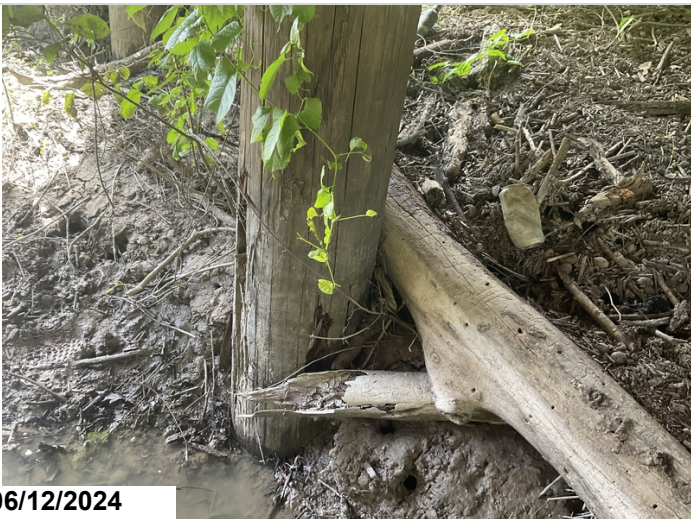
Bent 3, pile 2: outer shell decay with a small amount of section loss. 1EA CS2
