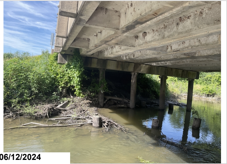
Vines and vegetation growing beside, under and onto bridge.
