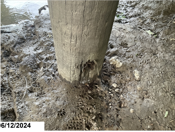
Bent 2, pile 4: minor outer shell decay at ground line. 1EA CS2
