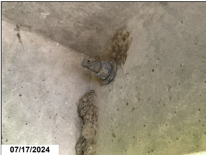
Typical loose bolt between units
