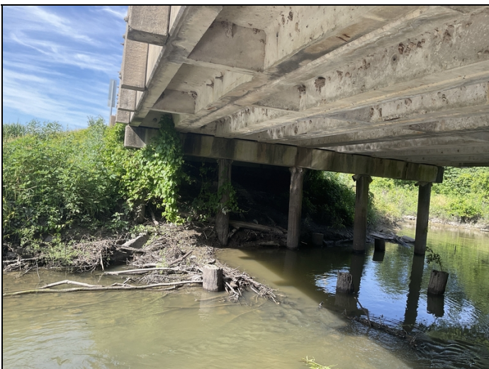
Vines and vegetation growing beside, under and onto bridge.
