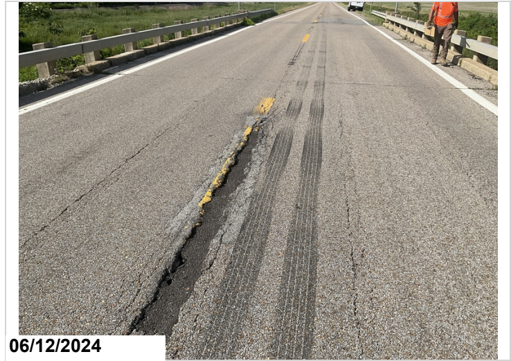
Cracking and spalling in overlay along centerline.
