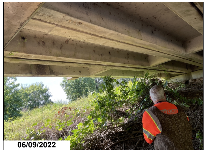
Span #3 all bolts are missing between units #1,2.
