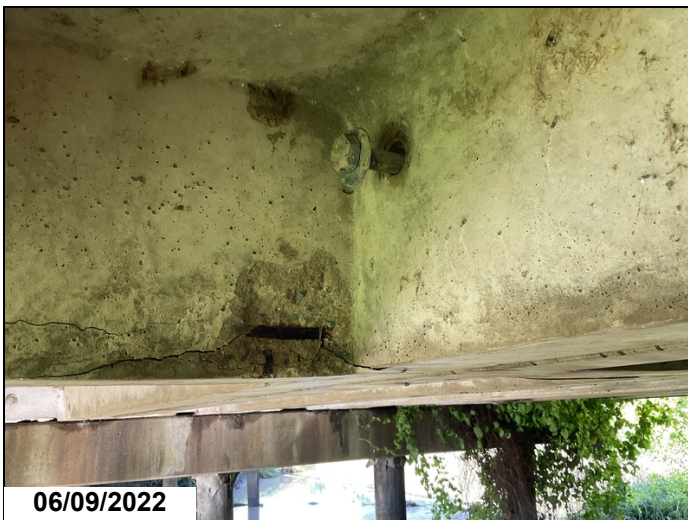
Span #1 has a loose connection bolt between unit #3,4 at mid span.
