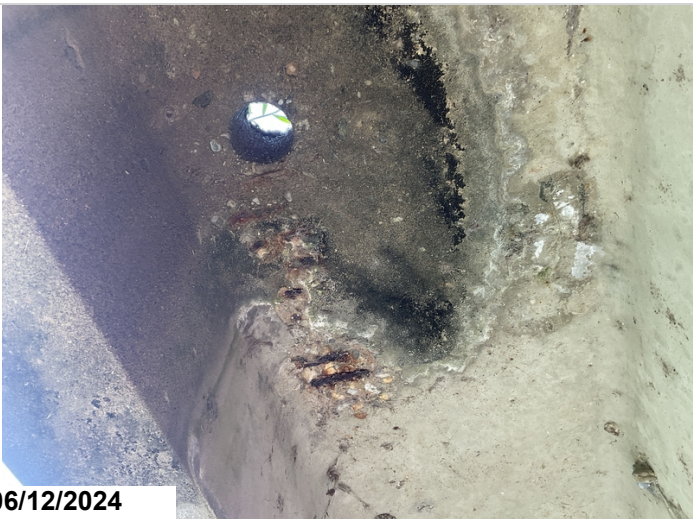
Span 1, unit 1, undersurface of deck near bent 2, at drain: 2 square feet of reinforcing steel exposed with moderate section loss near drain. 2SF CS3
