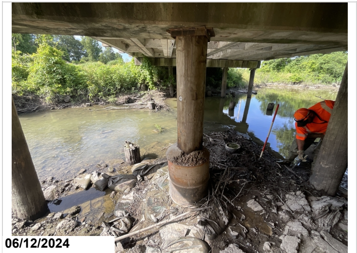
Bent 2, pile 2: spliced and encased in concrete. Structural integrity of concrete encasement unknown.
