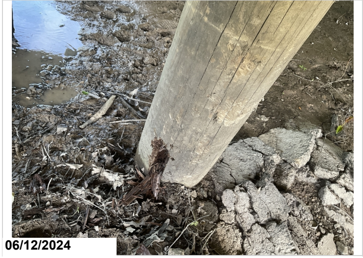
Bent 2, pile 3: minor outer shell decay at ground line. 1EA CS2
