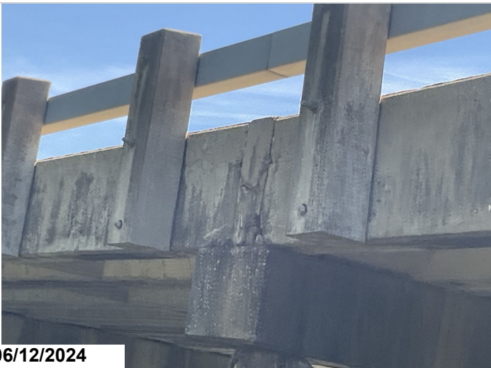
Bent 3, joint between spans 2 and 3, right side: cracked and spalled.
