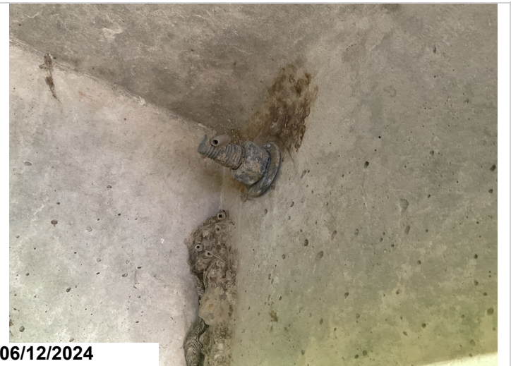
Typical loose bolt between units
