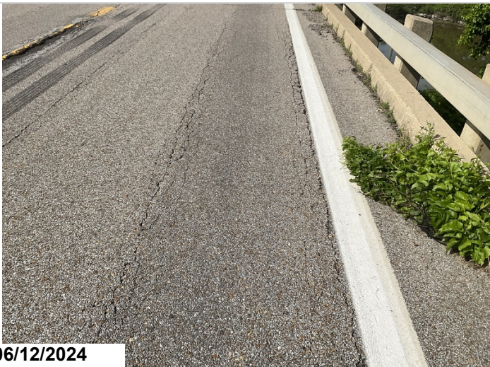
Typical longitudinal cracking in overlay along grout joints.
