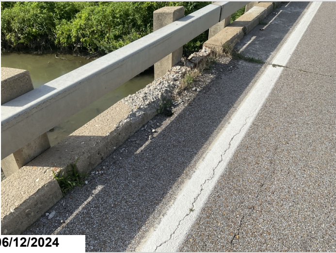
Span 1, left curb, at bent 2: spalled for 5' with 3' exposed reinforcing steel with minor section loss.
