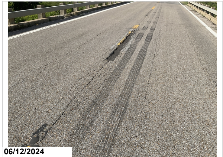
Span 1, deck, at centerline: 6" wide by 12' long patched area that is failing.
