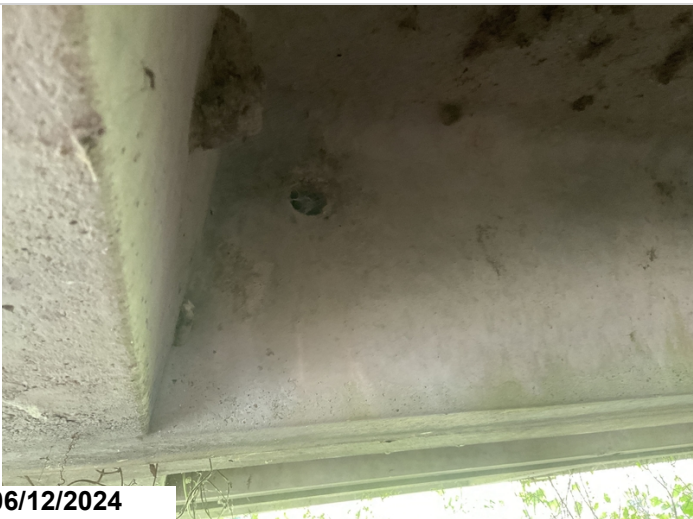
Span 3, connection bolt, between unit 2 and 3: missing bolt.
