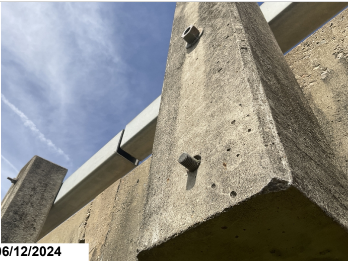
Span 2, rail post, left side, last post, bottom rail bolt: missing nut.
