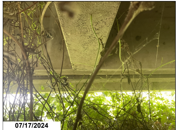
Span 3, connection bolts, between units 1 and 2: all bolts are missing.
