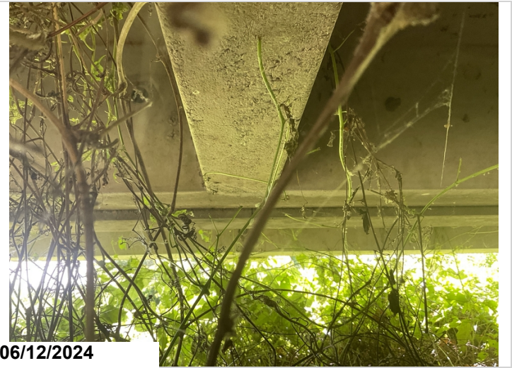
Span 3, connection bolts, between units 1 and 2: all bolts are missing.
