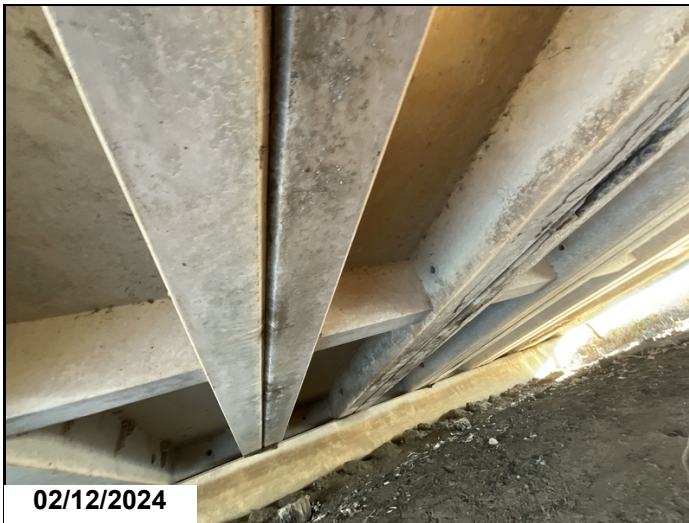
Span #1 channel beam units
