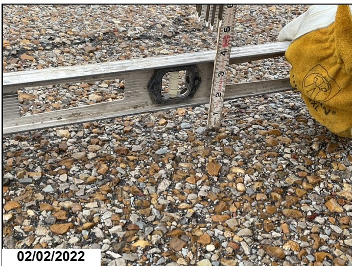
Abutment #2 approach roadway has settled up to one and a half inches
