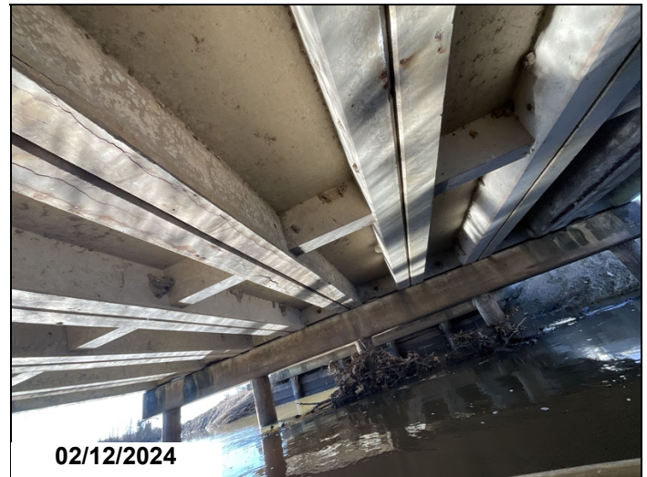
Span #2 channel beam units
