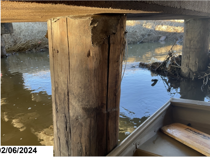
Typical pile condition
