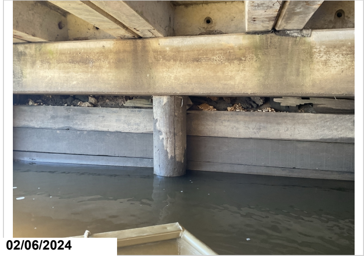
Abutment #2 timber back wall just below cap is decayed with areas of moderate to heavy section loss full length with voids to material behind cap and under roadway.
