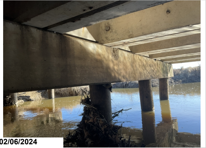
Bent #3 cap ahead face spall 8" over pile #3 no rebar exposed.
