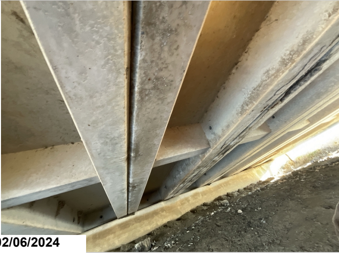
Span #1 channel beam units
