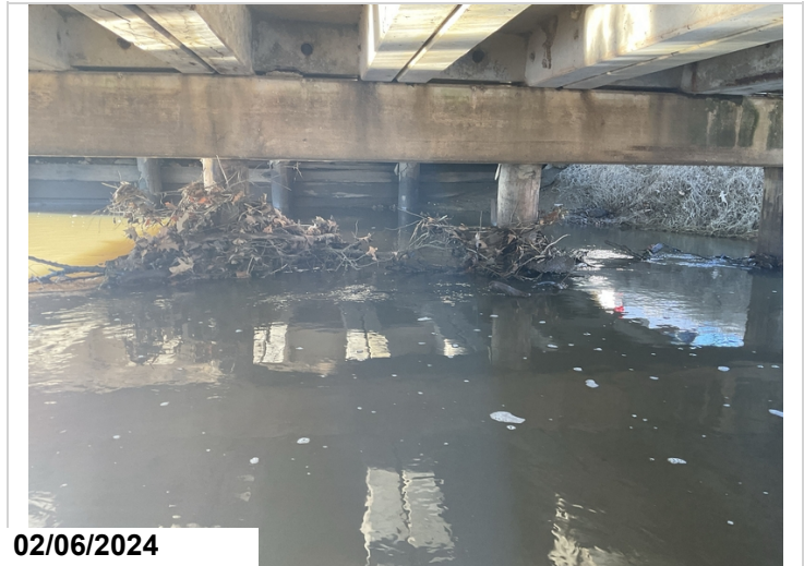
Typical drift in channel
