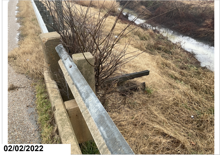
Brush growing at abutment #1 left side
