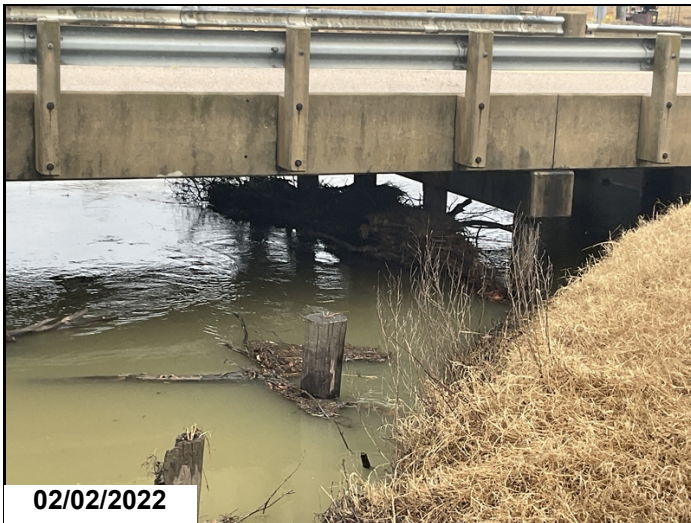
Moderate amount of drift at bent #3
