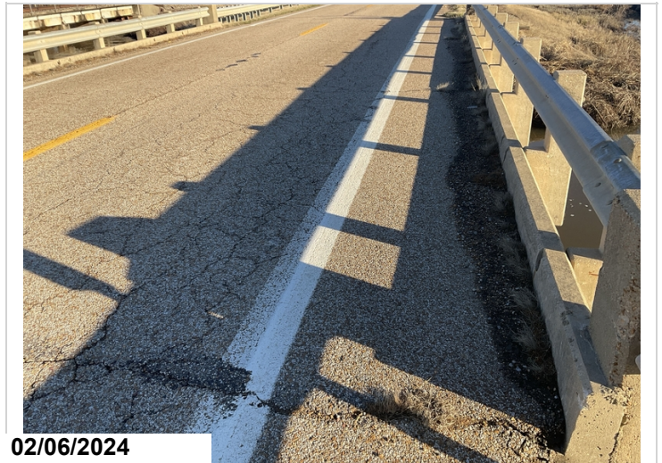
Typical debris in gutters
