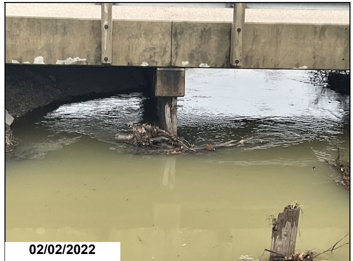
Small amount of drift at bent #2
