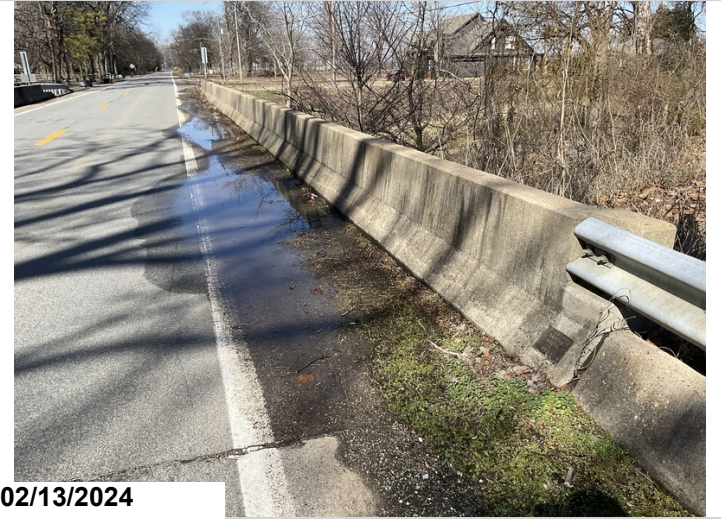
Typical debris in gutters
