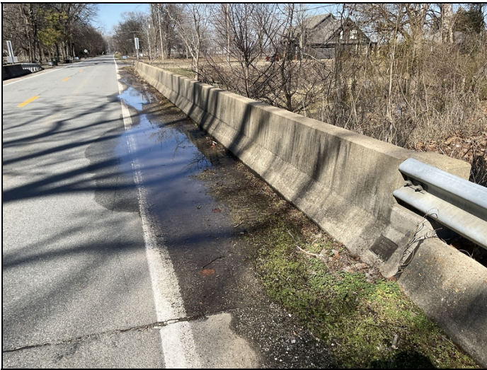
Typical debris in gutters
