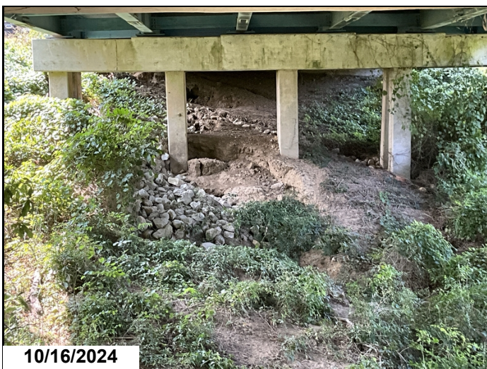
Span 1 & 2 slope erosion
