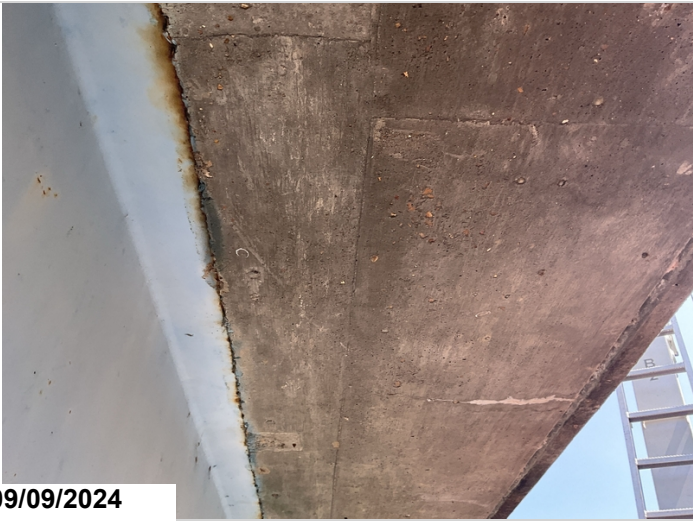
All Spans, Deck Undersurface Overhangs: Hairline transverse cracks some with light efflorescence spaced 6' apart.
