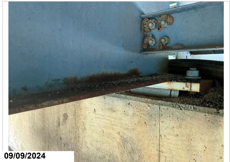
Span 4, Girders 1, 3 & 5, Bent 5: Active corrosion on bottom flange at bearing connection with minor section loss.
