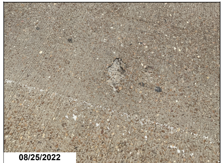
Span 8 left lane has 1' shallow spall with no exposed rebar
