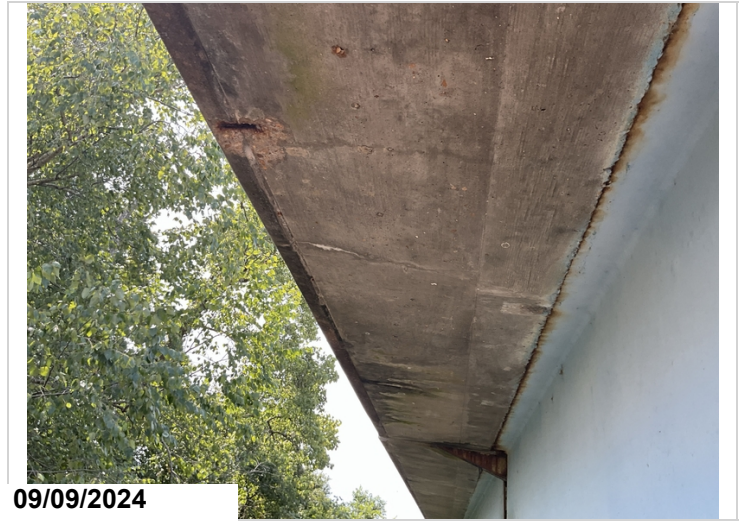
Span 5, Deck Undersurface Overhang, Right Side, 20' Ahead Of Bent 5: 6" spall exposed reinforcing steel. Reinforcing steel has minor section loss.
