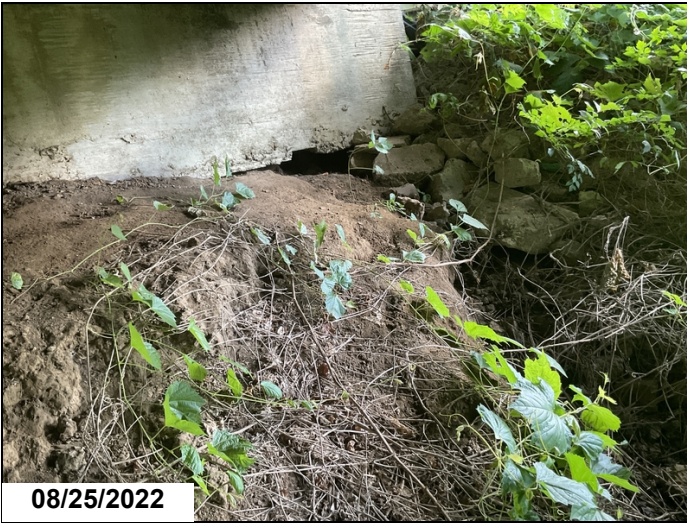
Abutment 1 cap left side undermined for 2' up to 6"
