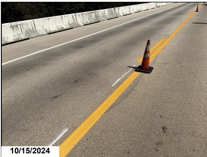
Typical deck surface repair
