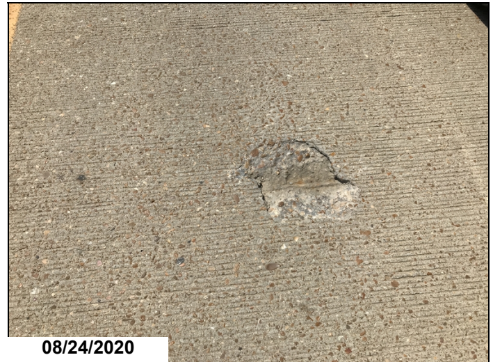
Span 2 left lane has a 1' spall with exposed rebar.
