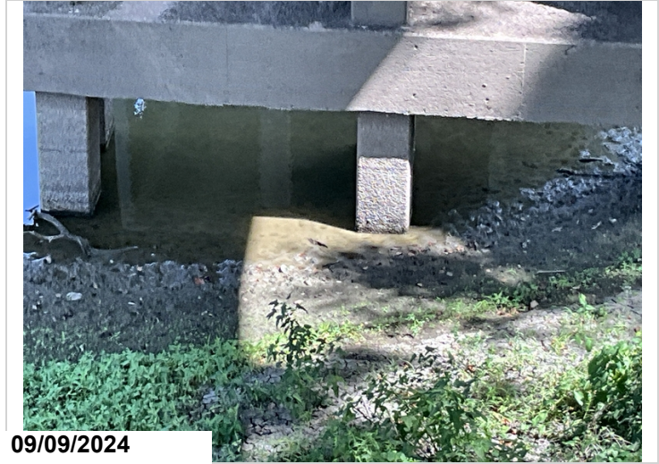
Bent 4 & 5, Piles: Light abrasion with no loose aggregate
