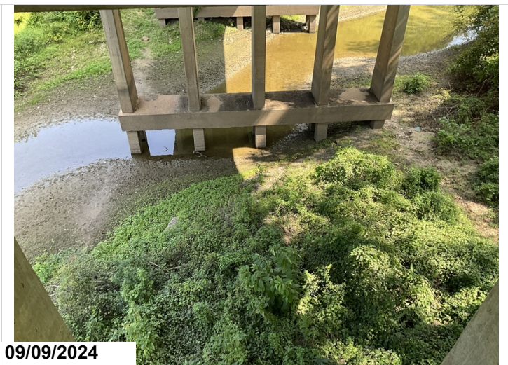
Bent 5 pile footing
