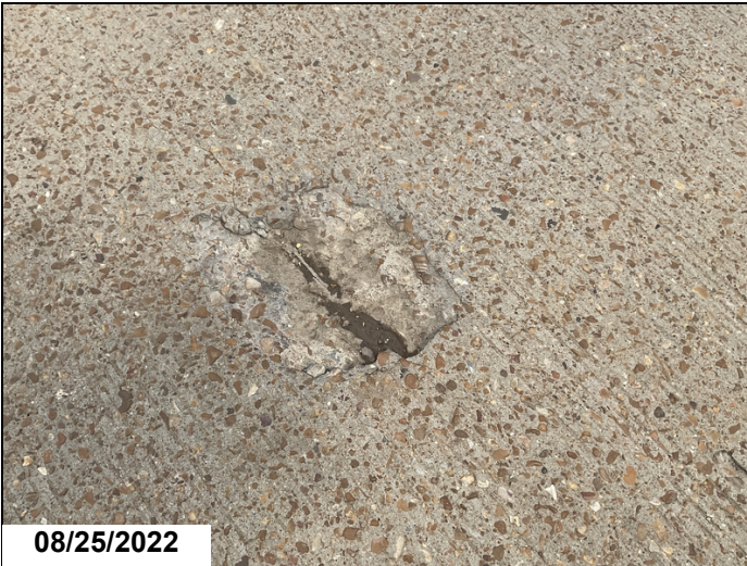
Span 4 deck right lane has 1' spall with exposed rebar with 10% section loss
