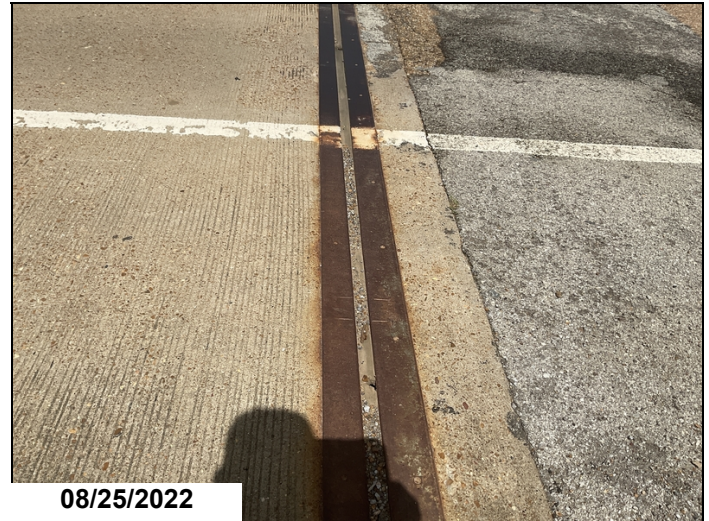
Abutment 2 seal has two 1" holes in the right lane and shoulder.
