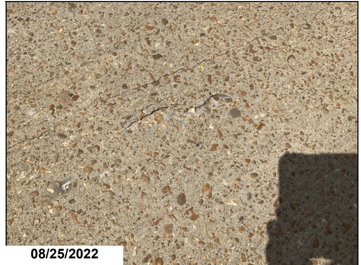
Span 2 deck right lane has 1' long by 2" wide shallow spall with no exposed rebar
