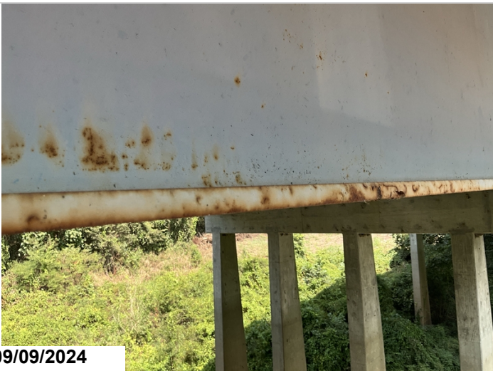
Span 5, Girder 5, 20' Ahead Of Bent 5, Right Side: Lower flange has 1" delamination.
