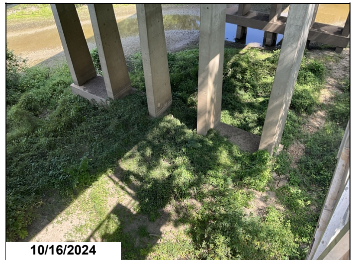
Bent 4 pile footing
