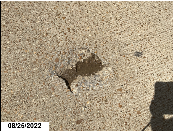
Span 2 deck left lane has 1' spall with exposed rebar
