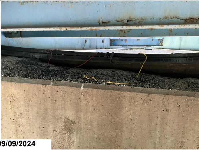
Bent 5 cap has fertilizer, dirt and debris on it.
