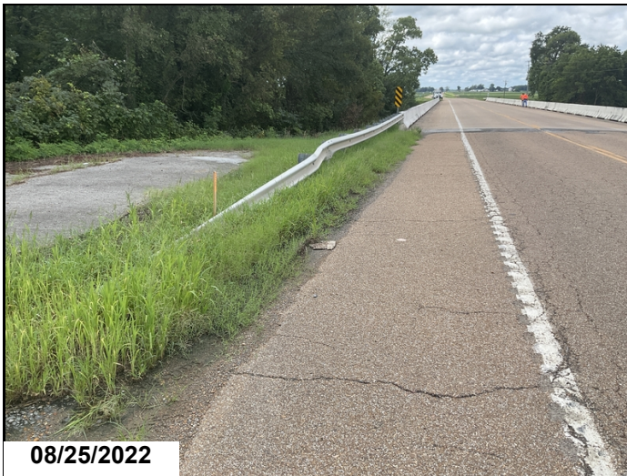
Abutment 2, Approach Rail, Right: minor collision damage.
