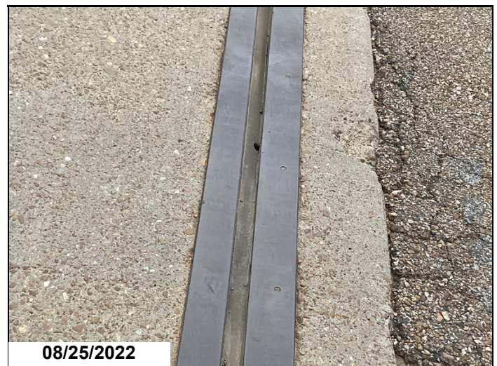
Typical hole in joint seal
