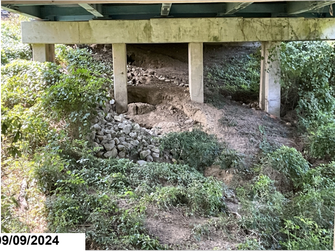
Span 1 & 2 slope erosion
