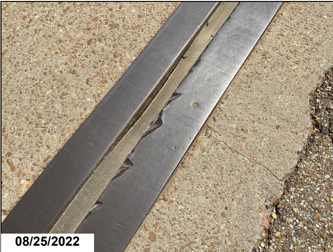
Typical joint seal lost adhesion
