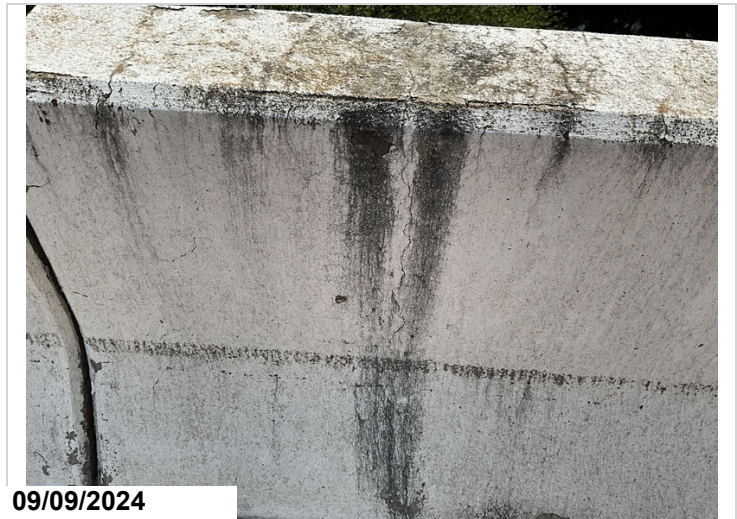
Bridge Rails, Both Sides, Full Length: Vertical cracks spaced 6' apart.
