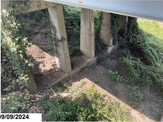
Bent 3 pile footing
