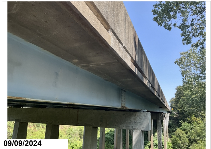
Typical deck undersurface overhang
