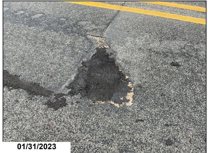
Deck span #8 unit #6 has a two foot spall at bent #8 no rebar exposed with asphalt patch.
