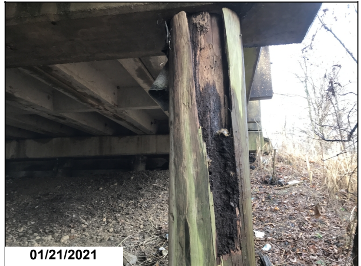
Bent #2 pile #1 is core decayed with 30% section loss.
