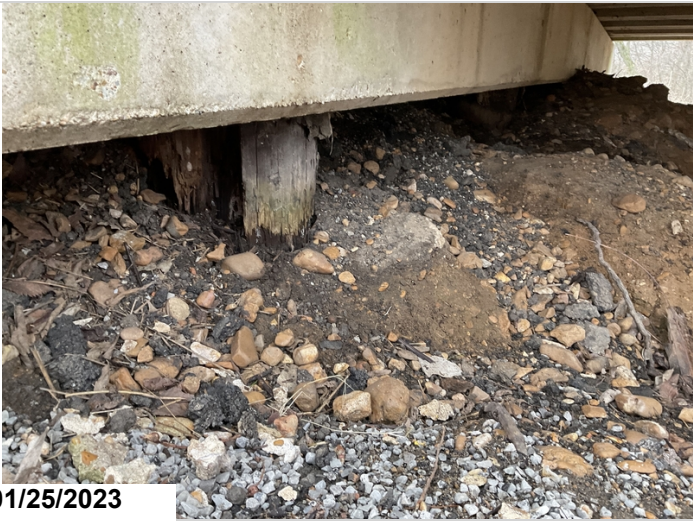
Bent #10 pile #1 sounds moderately hollow with hole in left side moderate section loss.
