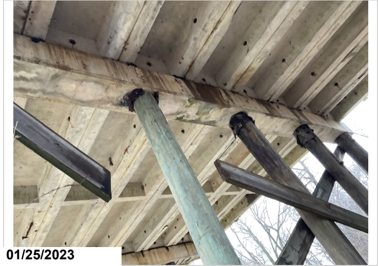
Bent#6 cap ahead face has several delaminations and two 6" spalls with rebar exposed with moderate section loss.
