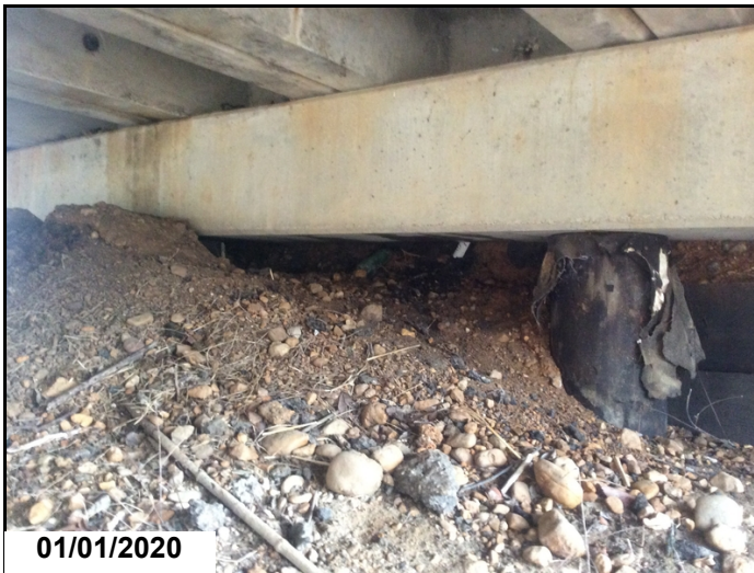
Settlement of abutment-#2 back wall
