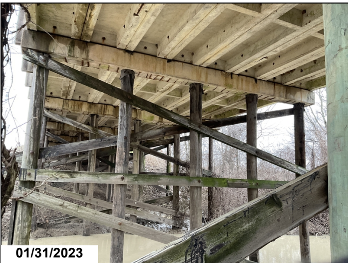
Bent #5 cap ahead face at top between piles #2,3 has a 1' spall with no rebar exposed.
