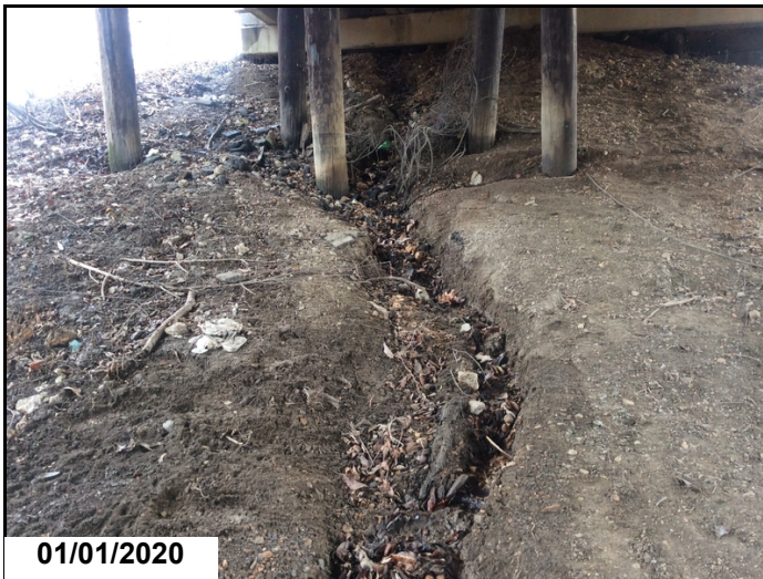
Minor erosion abutment #2 slope
