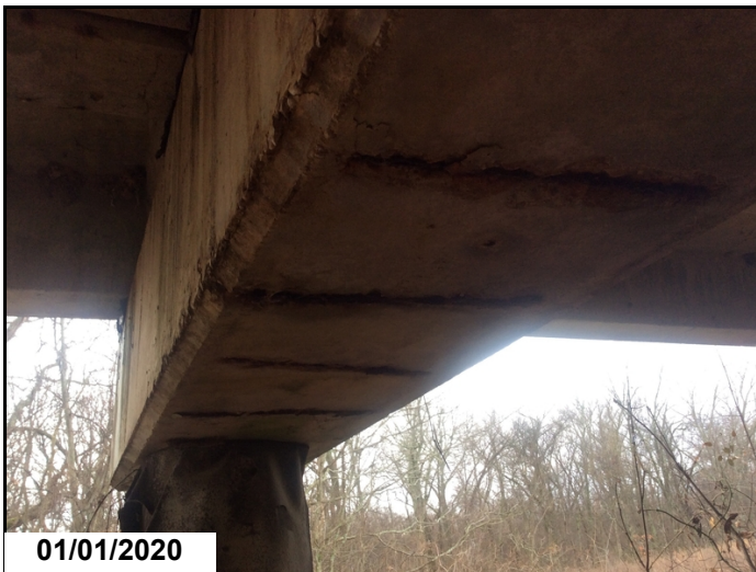
Typical spalls on bottom of caps
