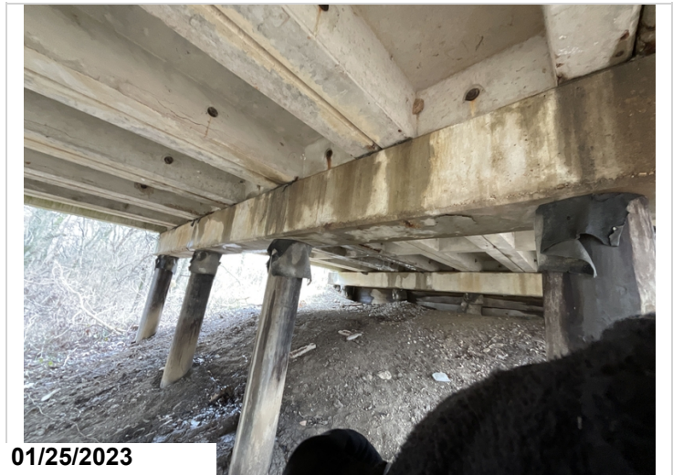
Bent #2 cap ahead face has three 1' delaminated areas.
