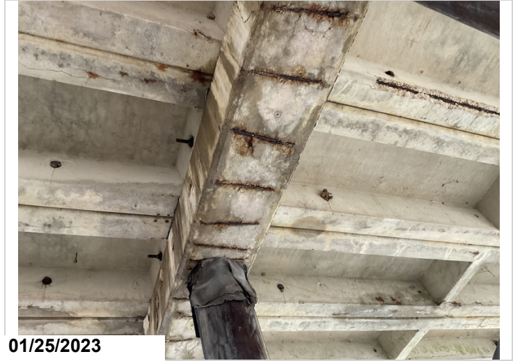
Typical rebar exposed on bottom of caps
