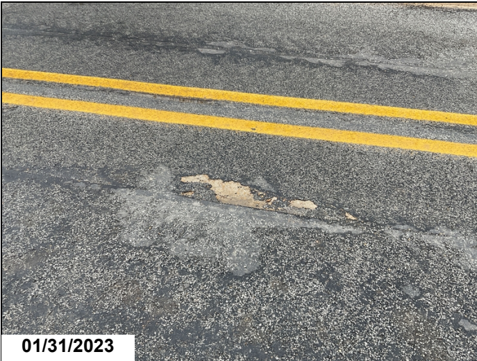
Span #3 unit #4 has 1' shallow spall center span no rebar exposed.
