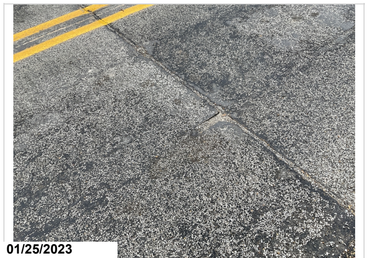
Grout joints in all spans between units are spalling up to one inch deep. Some have been filled with asphalt.
