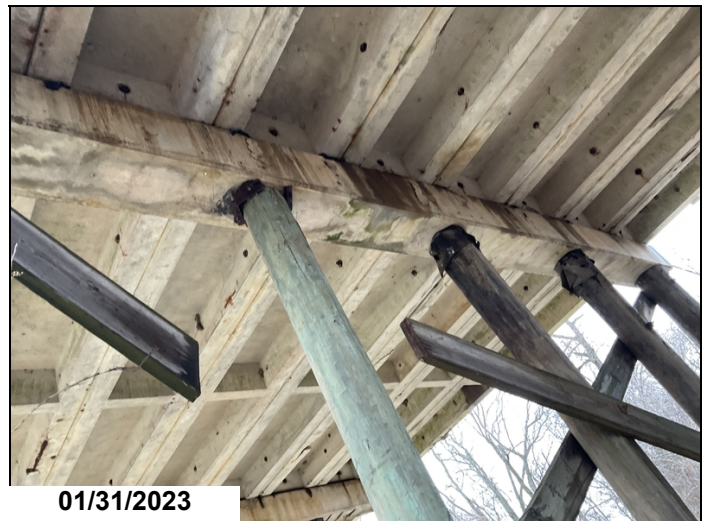
Bent#6 cap ahead face has several delaminations and two 6" spalls with rebar exposed with moderate section loss.
