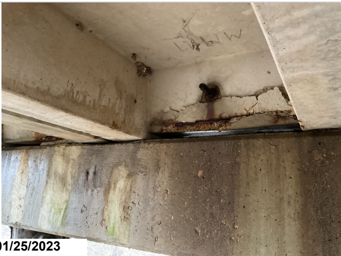
Typical spalling of diaphragms at bents.
