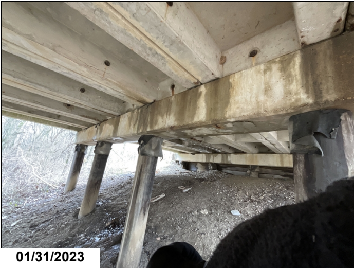
Bent #2 cap ahead face has three 1' delaminated areas.
