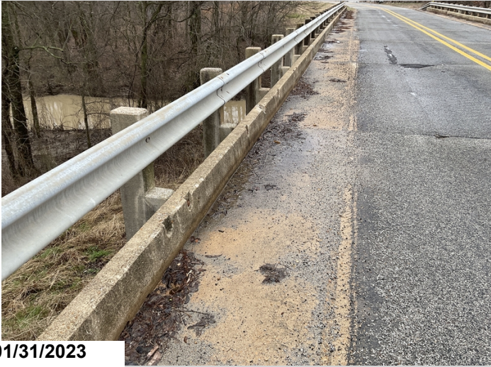
Typical debris in gutters
