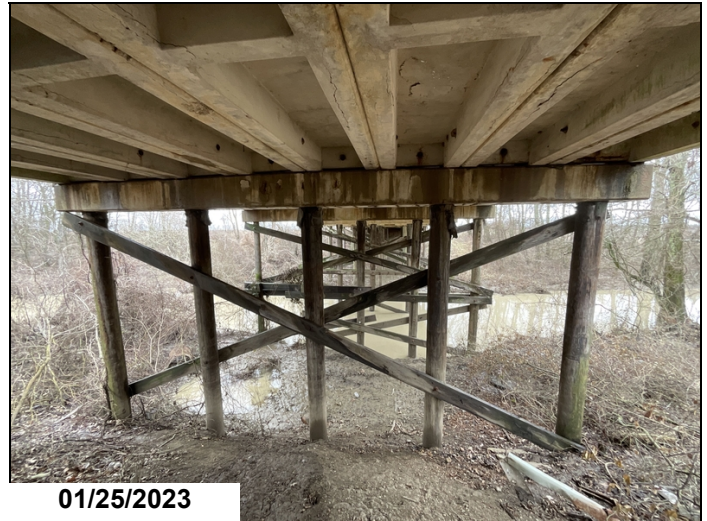
Bent #3 cap back face has three 6" spalls with exposed rebar with moderate section loss and several delaminations.
