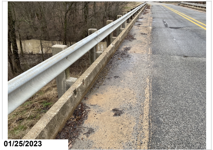
Typical debris in gutters
