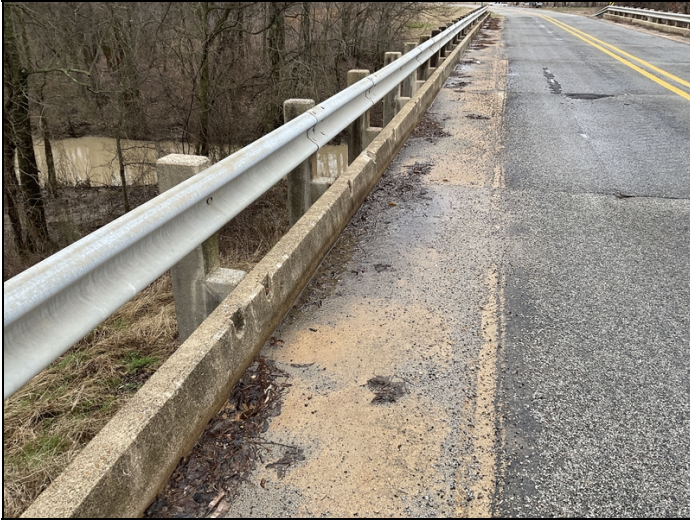
Typical debris in gutters
