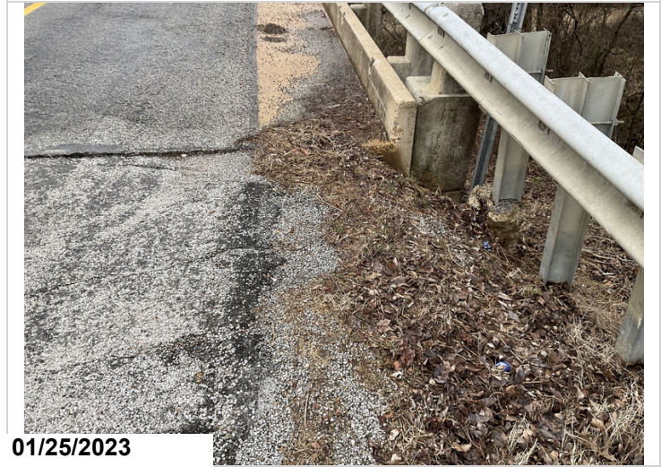
Abutment #2 left side erosion at bridge end
