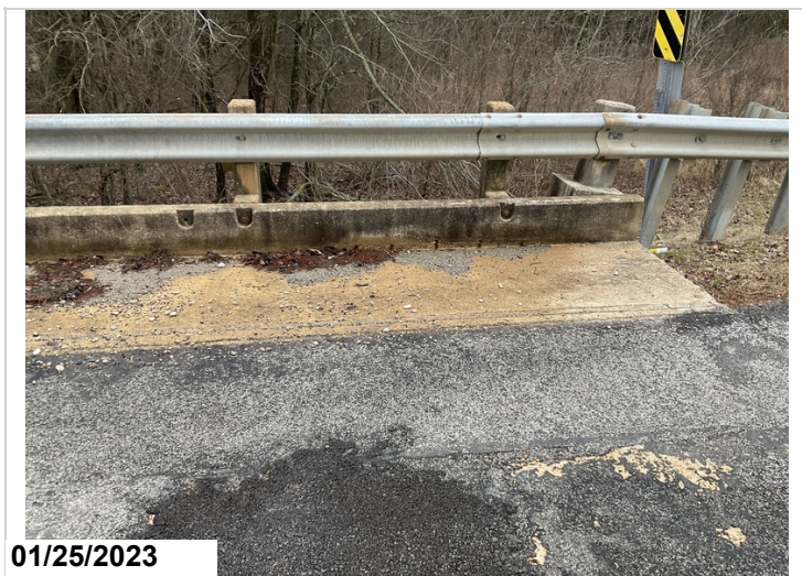
Curbs have areas of exposed rebar due to poor coverage.
