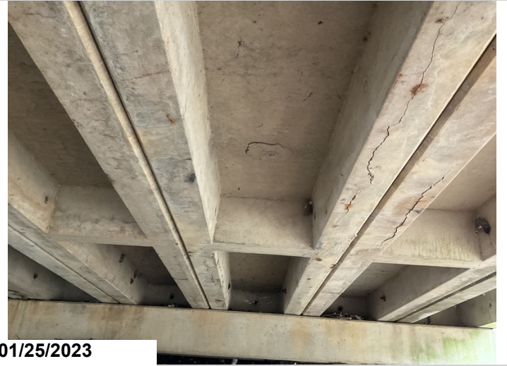
Soffit-under surface span #9 unit #6 has a 1' delaminated area at 1/4 span.
