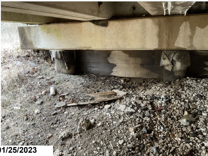
Abutment #1 cap has 1' long corner spalled off near pile #5.
