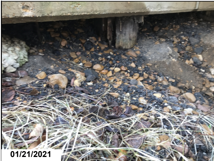
Bent #10 pile #1 is core decayed with 40% section loss.
