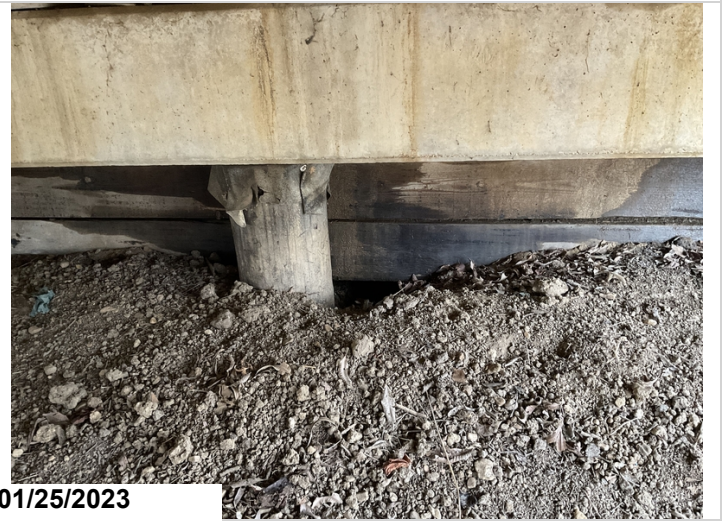
Abutment #1 beside pile #2 has a four foot void behind timber back wall.
