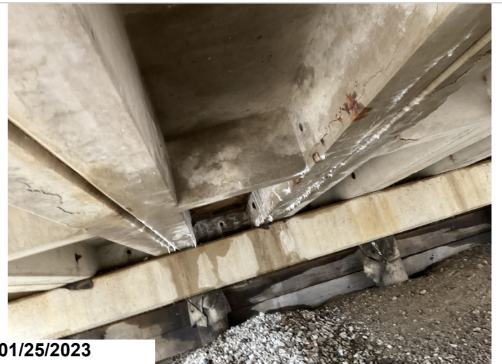
Span #1 unit #6 both legs have map cracking with moderate efflorescence first half of span.
