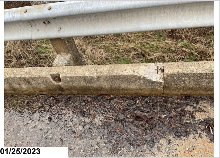
Deck span #9 right curb at bent #9 has one foot spall with exposed rebar no section loss.
