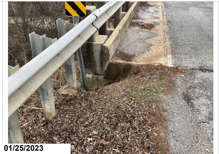
Abutment #1 left side erosion at bridge end.
