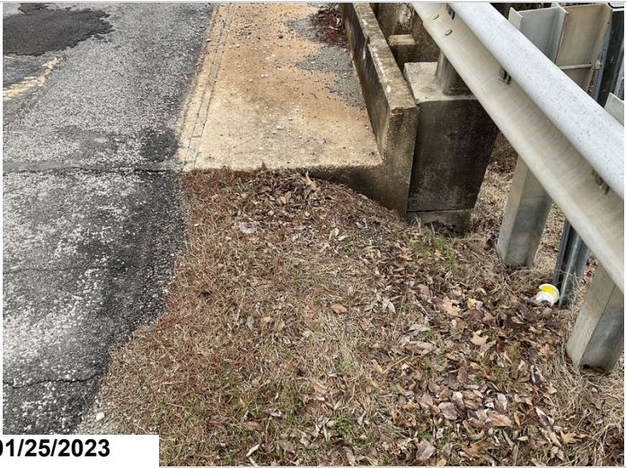
Abutment #1 right side erosion at bridge end.
