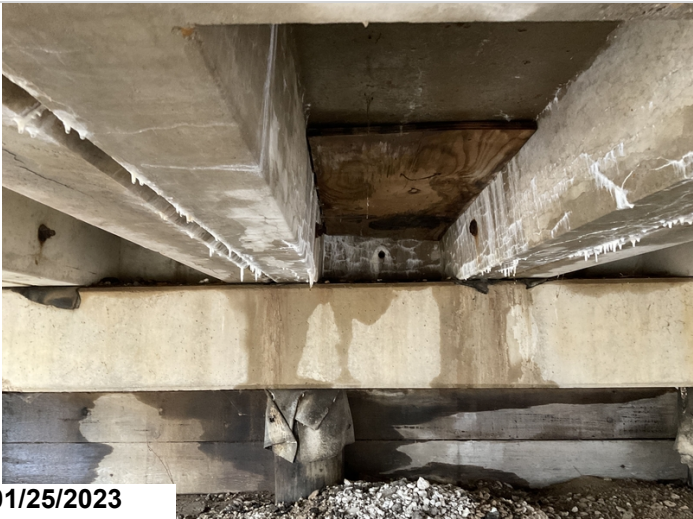
Soffit-Under surface span #1 unit #6 has a repair with form left in place.
