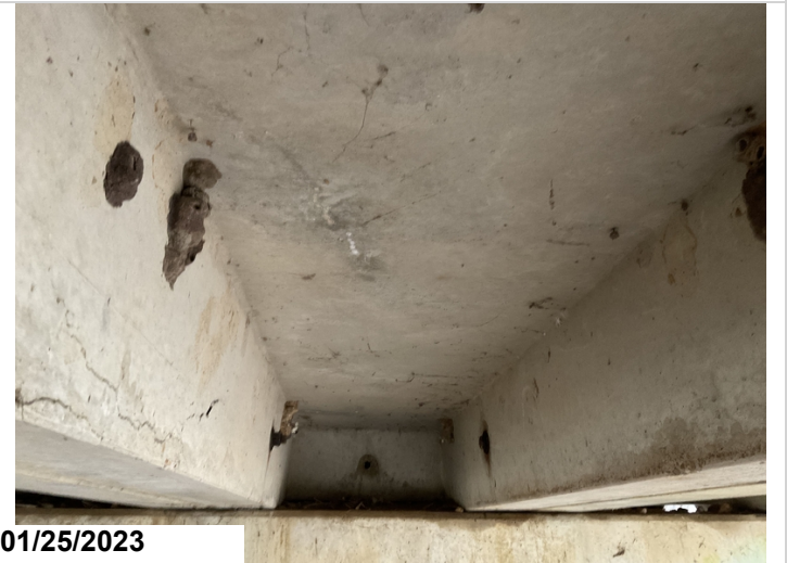
Soffit-Under surface span #1 unit #2 has cracks with light efflorescence.
