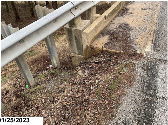
Abutment #2 right erosion at bridge end
