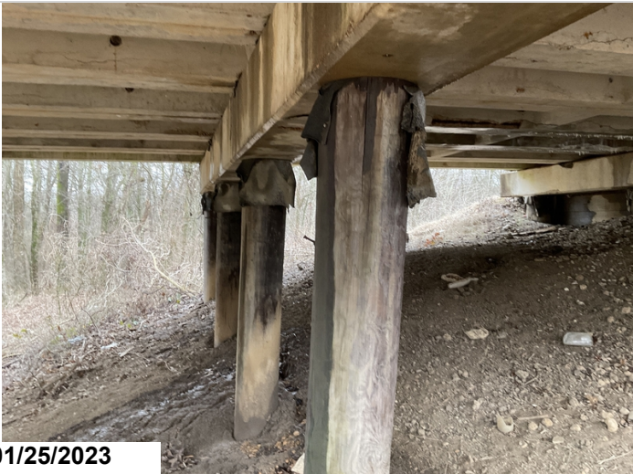
Typical cracks in piles
