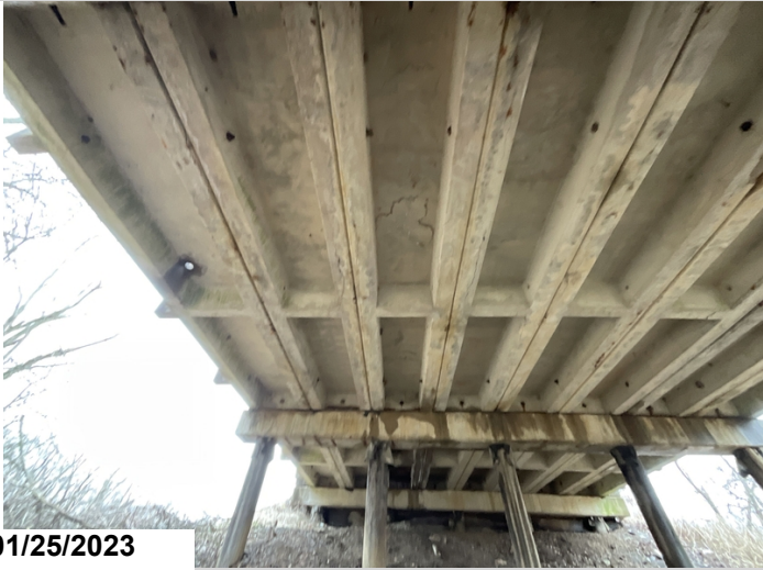
Soffit-Under surface span #2 unit #6 has six feet of cracks with light efflorescence, and 3 2' delaminated areas.
