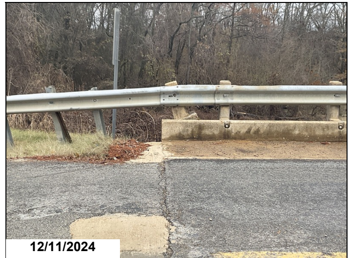
Abutment 1, left side, first rail post: leaning back. Typical of others.
