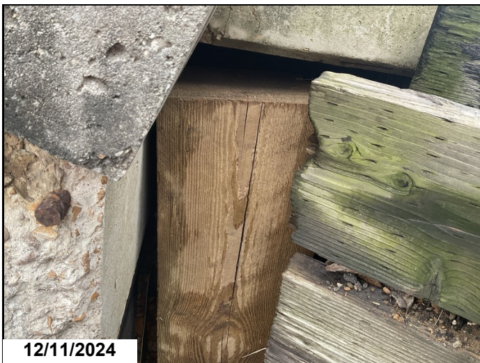
Abutment 2, right side void behind cap.
