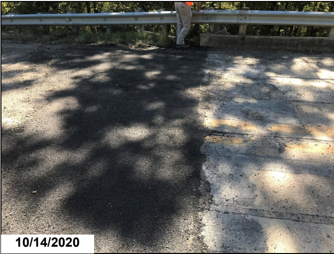
Abutment #2 approach roadway has been repaired with achm.
