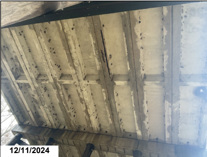
Span 4, unit 3, right leg: spalled 5' with exposed reinforcing steel with moderate section loss rest of leg is cracked.
