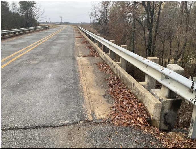
Dirt and debris in gutters
