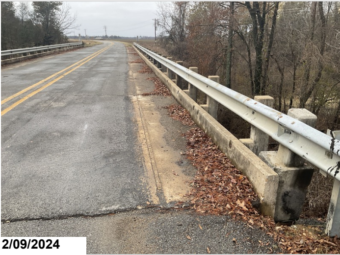
Dirt and debris in gutters
