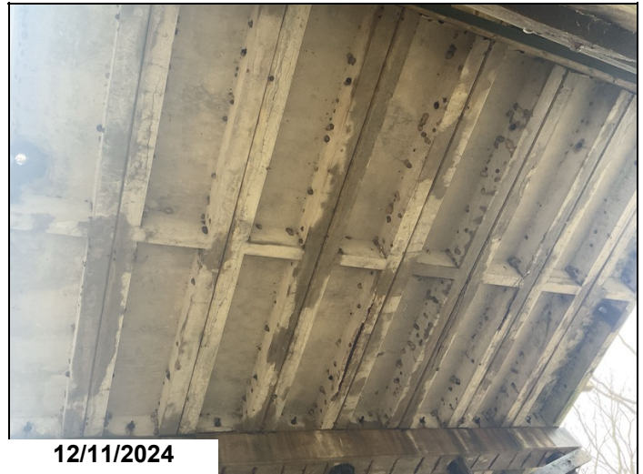
Span 5, unit 7, left leg: cracked for 10'.
