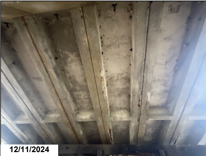
Span 1, unit 2, right leg: cracked and delaminated for 4' with 3' spall with exposed reinforcing steel with moderate section loss first 1/2 span.
