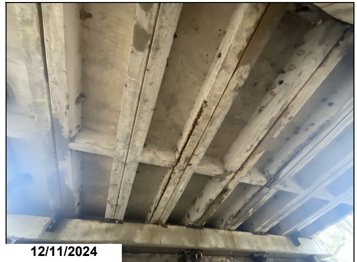
Span 9, unit 3, right leg: cracked and delaminated 2' with 14' spall with exposed reinforcing steel with moderate section loss.
