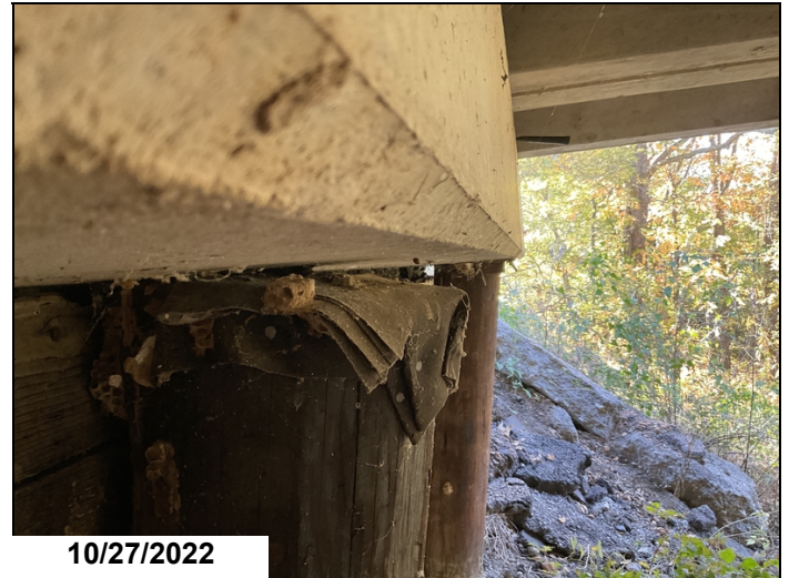
Typical bearing of piles at abutment #2 cap due to rotation
