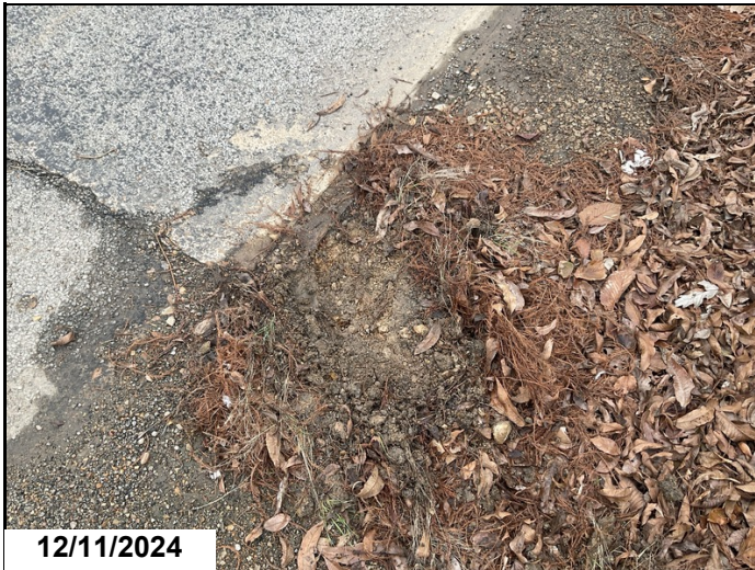
Span 1, unit 8, at bent 2, right side white line: 1' spall no rebar exposed. Spall
