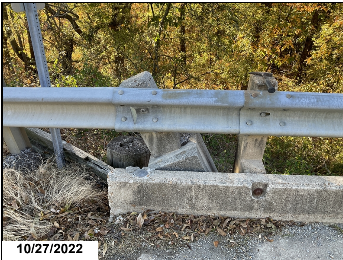
Abutment #2 right side last rail post leaning ahead
