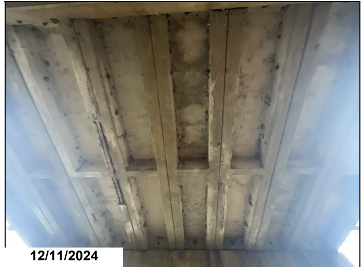
Span 2, unit 6, left leg, last 1/2 span: cracked for 8' with rust staining.
