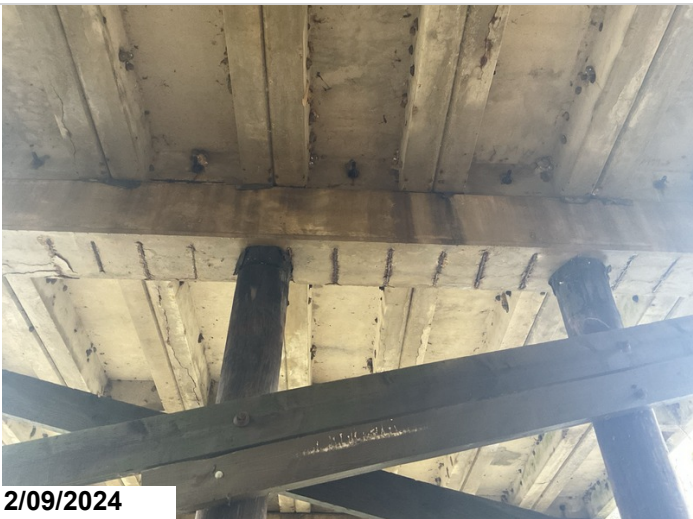
Typical exposed reinforcing steel on bottom of pile caps.
