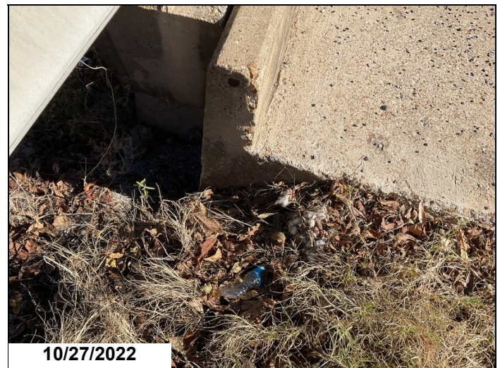
Erosion at abutment #1 right shoulder
