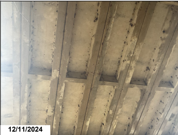
Span 3, unit 4, left leg: cracked 9' first half of span with rust stains, with 2' of cracking at 3/4 span.
