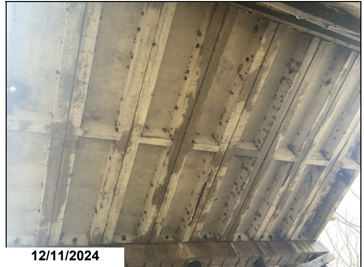
Span 5, unit 4, right leg: 5' spall with exposed rebar at 3/4 span with moderate section loss and 5' of cracking with rust staining.
