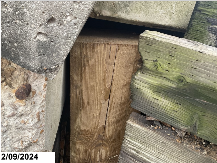
Abutment 2, right side void behind cap.
