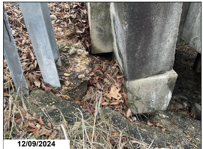
Abutment 2, left side: void behind cap
