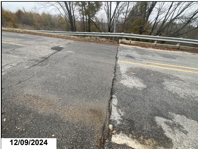
Abutment 2, approach roadway settlement
