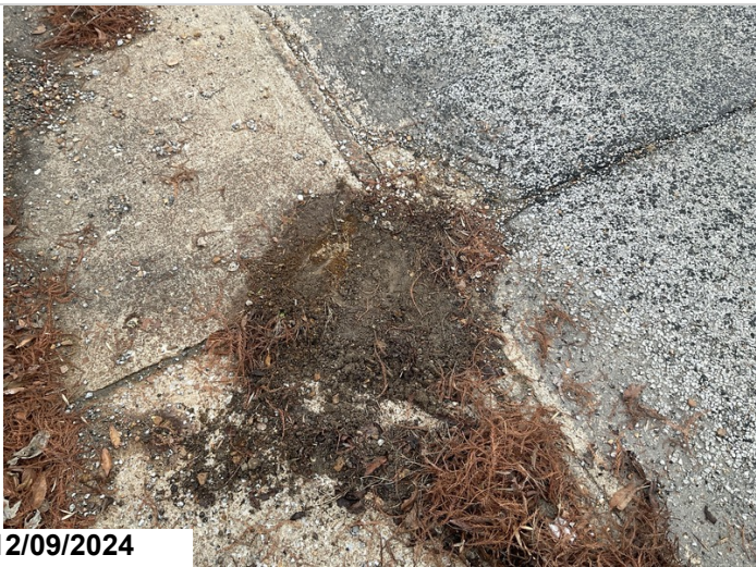
Span 1, unit 1, at bent 2: 1' heavy scaling 1" deep with loose aggregate. Span 2, unit 1, at bent 2: 1' heavy scaling 1", deep with loose aggregate
