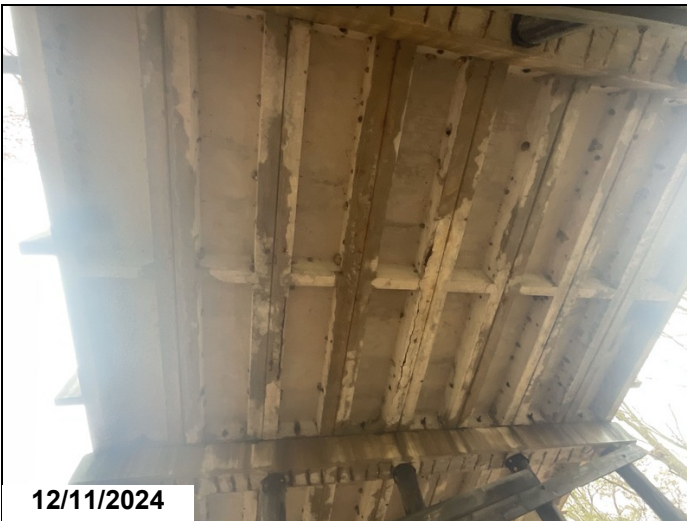
Span 7, unit 3, left leg, starting at 1/4 span: cracked with rust stains for 6' with 4' spall with exposed reinforcing steel with moderate section loss.
