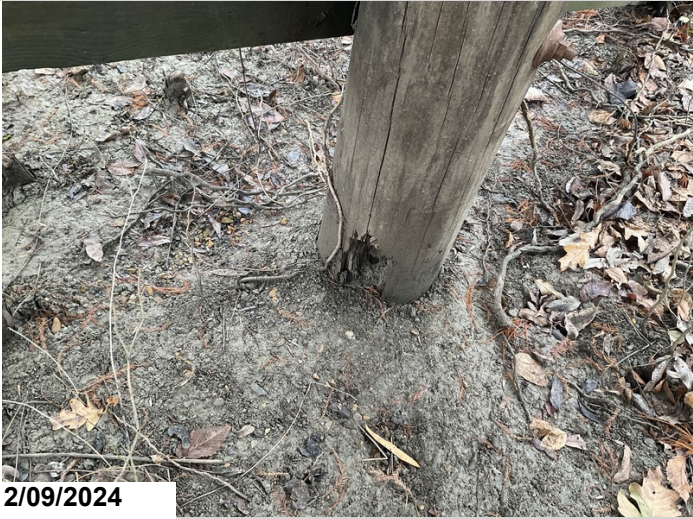
Bent 7 pile 2: 4" wide by 3" deep hole in outer shell at ground line.
