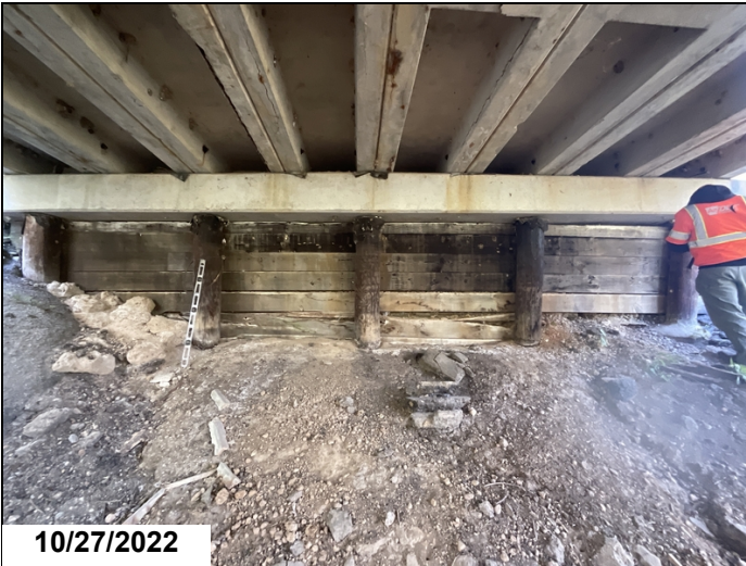
Abutment #2 timber back wall is decayed full width with areas of 100% section loss allowing for erosion.
