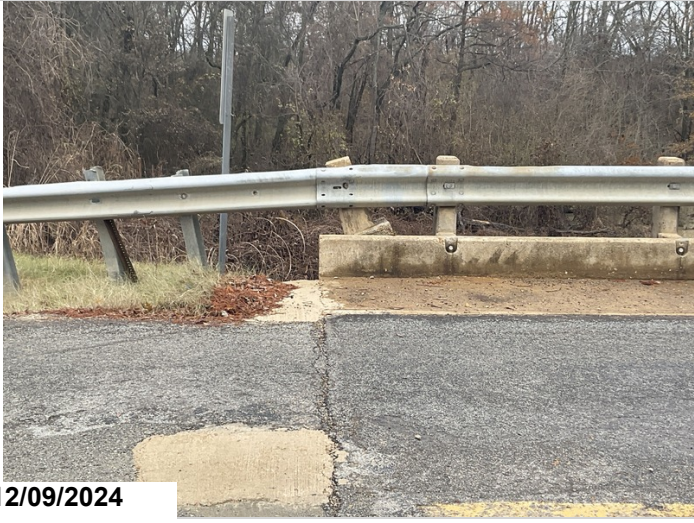
Abutment 1, left side, first rail post: leaning back.
