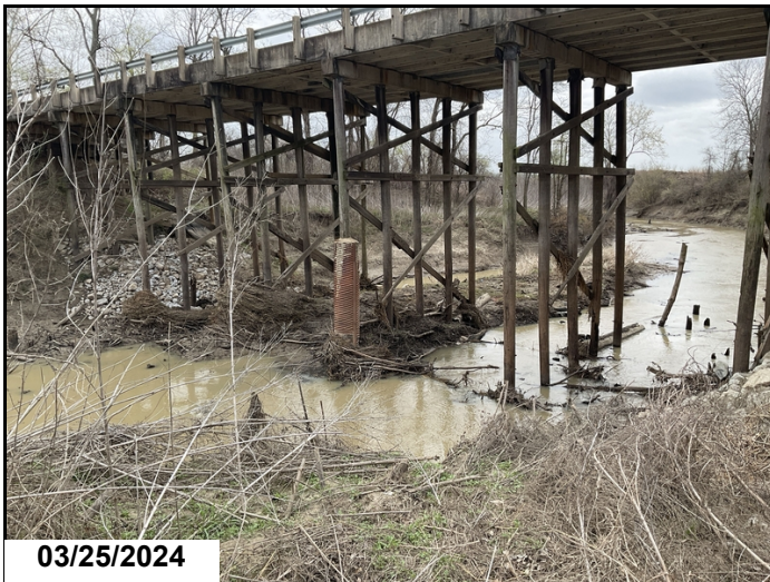
Silt and debris in channel
