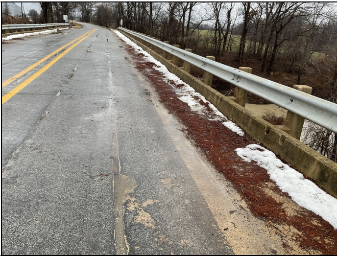
Dirt and debris in gutters
