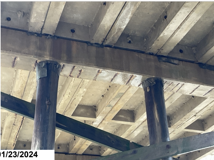
Typical exposed rebar on bottom of cap
