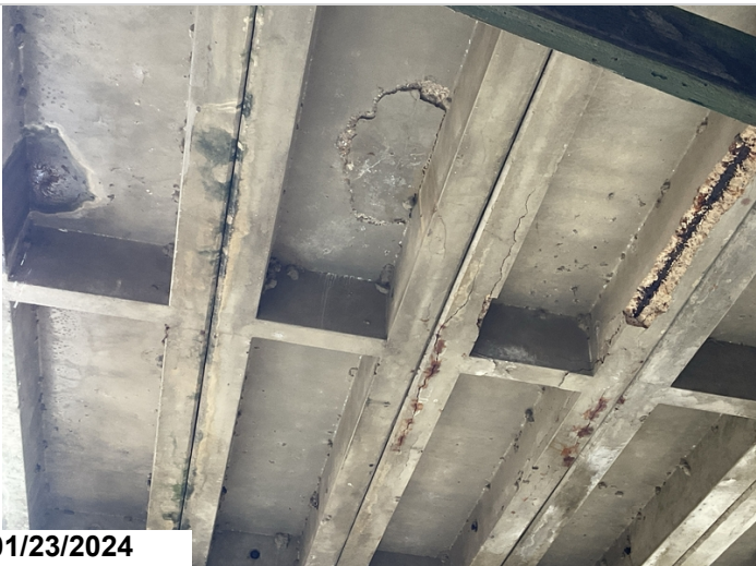
Span #3 girder #2 has two foot delaminated area in soffit near mid span.
