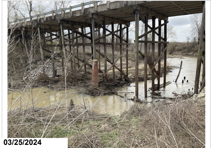
Silt and debris in channel
