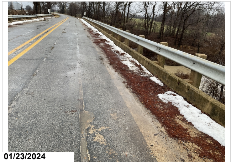
Dirt and debris in gutters
