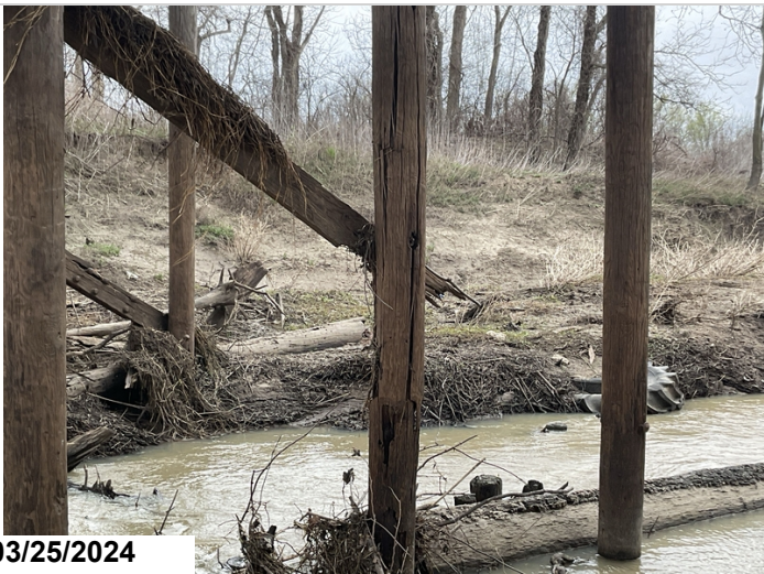
Bent #5 pile #4 is core decayed with large section loss and mushrooming.
