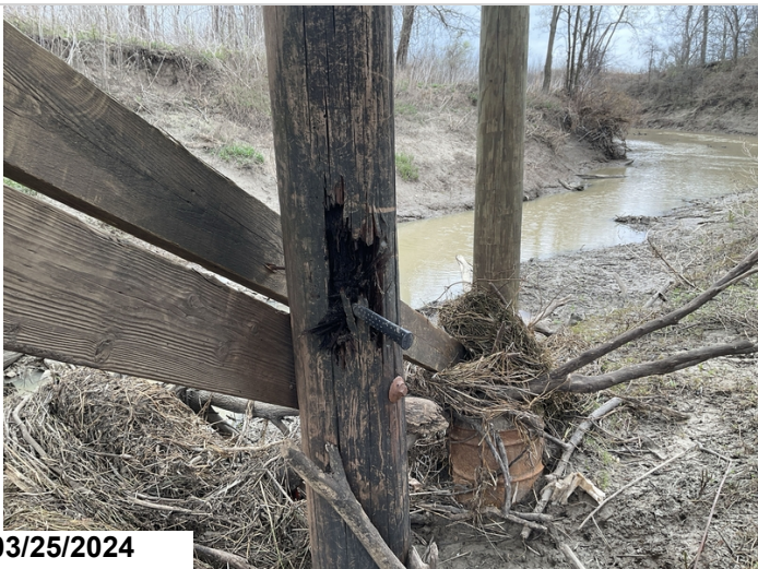
Bent #7 pile #4 sounds very hollow with hole in left face.
