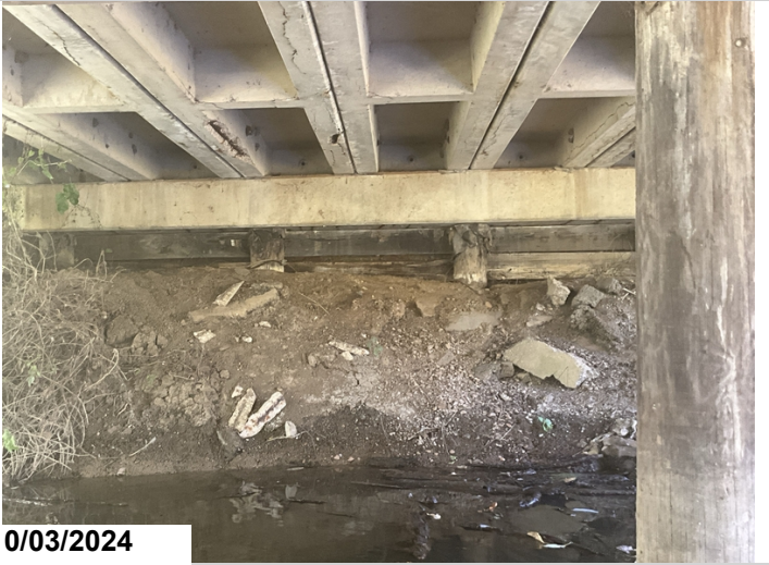
Bent 7: Decay in timber back wall full length.
