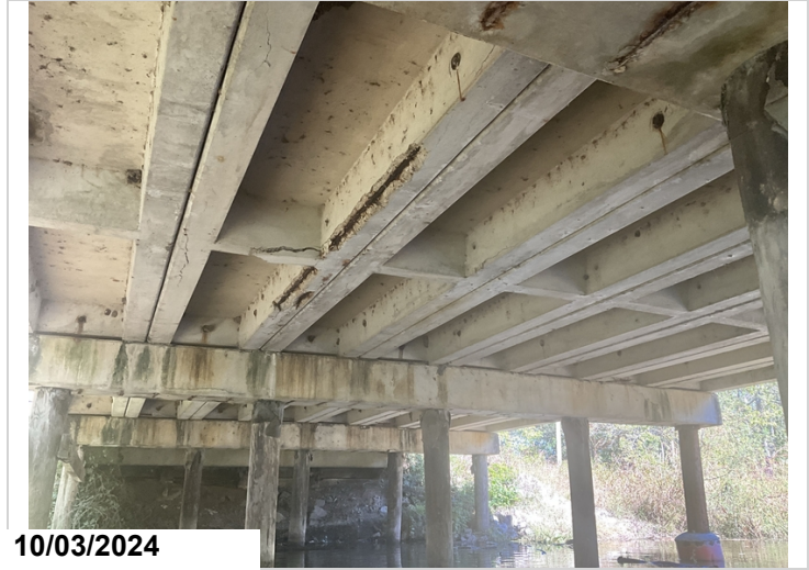
Span 4, Unit 2: Spalling with exposed reinforcing steel. CS3.
