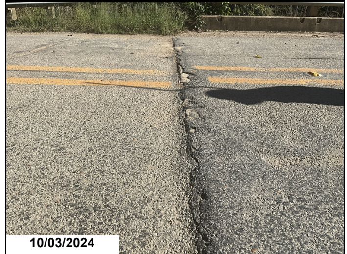
Bent 7: Approach roadway settlement.
