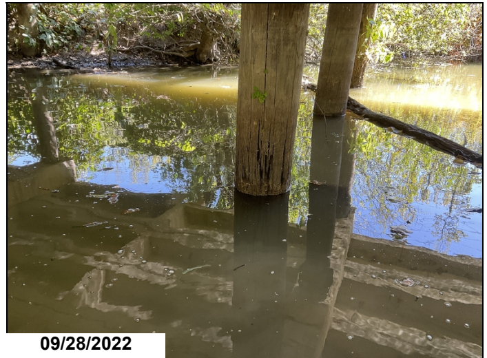
Bent #5 pile #3 has outer shell decay with minor section loss.
