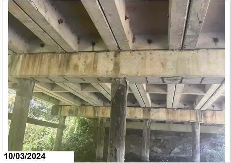
Bent 5, Bottom: Spalling with 20' cs3 rebar.
