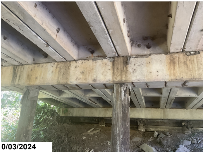
Bent 6: Spalling with 21' of exposed reinforcing steel. CS3.
