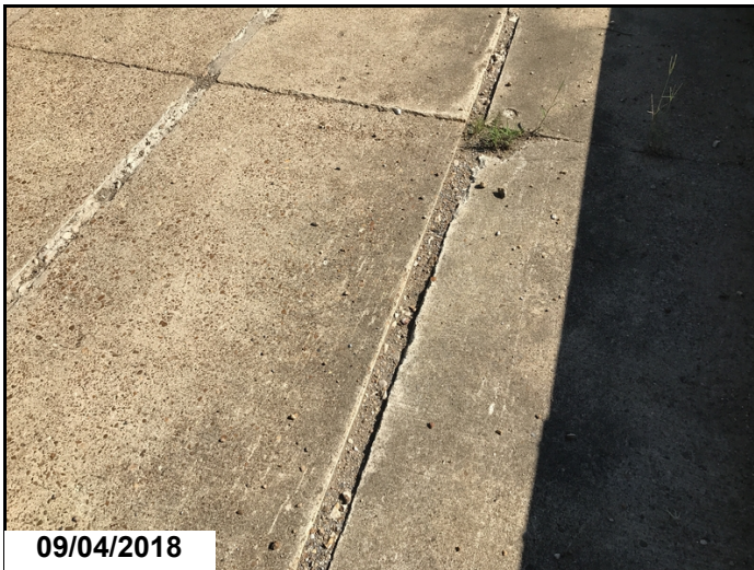
Typical spalled deck joint.
