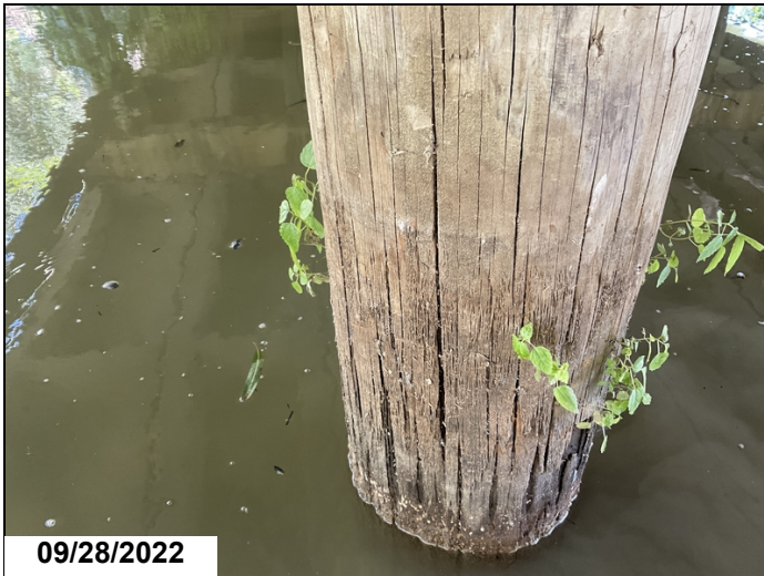
Bent #5 pile #2 has outer shell decay with minor section loss.
