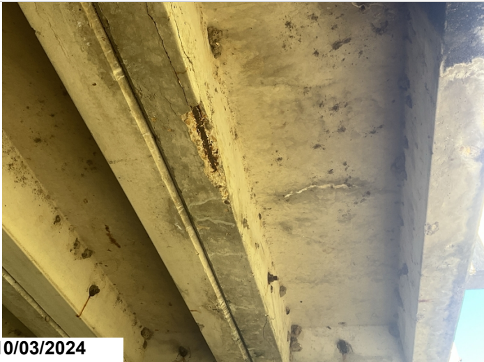
Span 4, unit 7: Rust staining & unit 8 efflorescence. CS2 & cs3.
