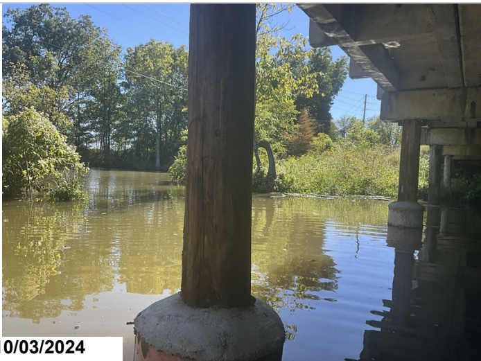
Bent 5, Pile 5: Minor cracking. CS2.
