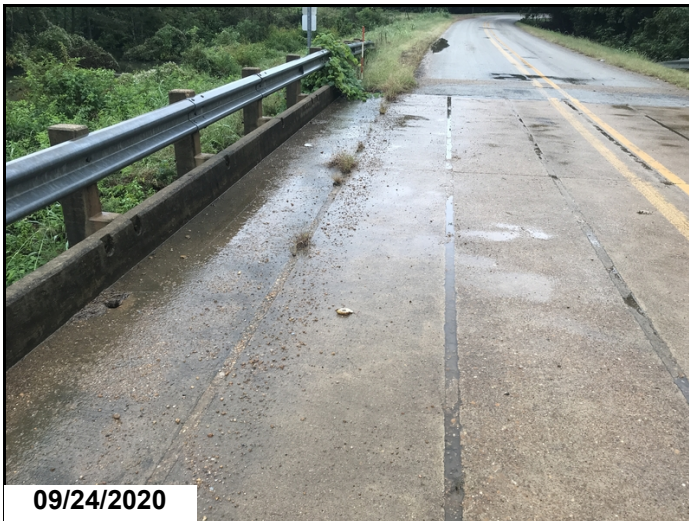
Vegetation growing in grout joint.
