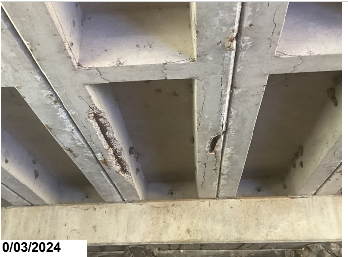
Span 6, Channel Unit 3: Spalling with 5' of exposed reinforcing steel. CS3.
