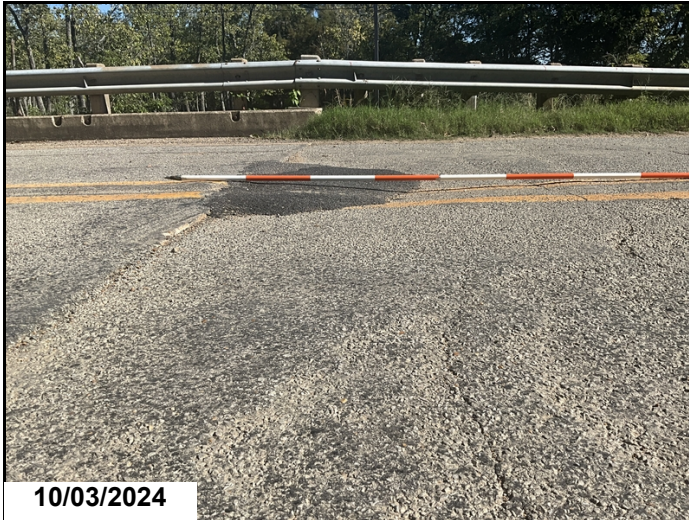
Bent 1, Approach: roadway settlement.
