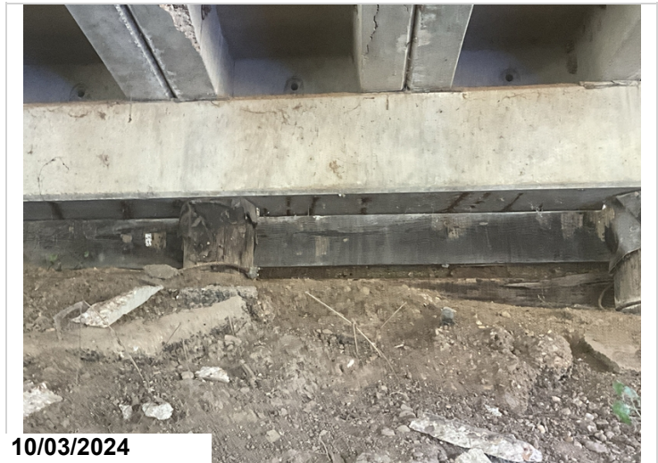
Bent 7, Bottom of cap: Spalling with 20' of exposed reinforcing steel. CS3.
