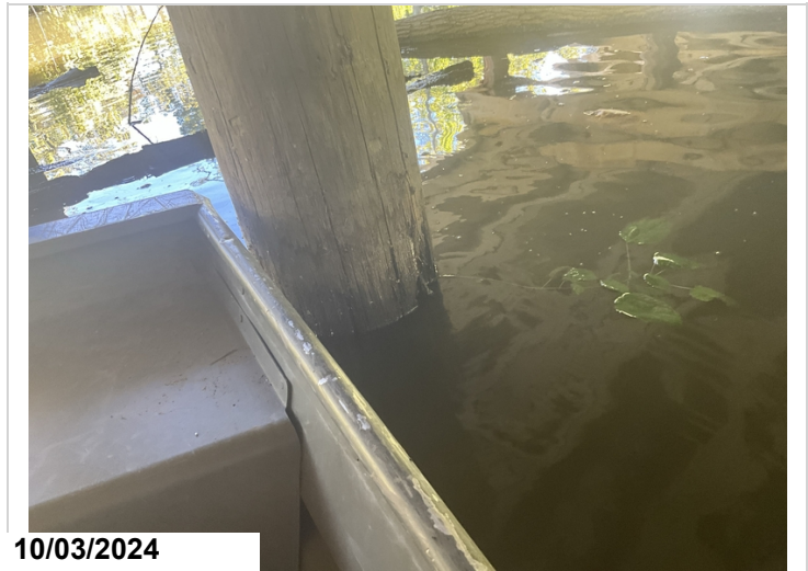
Bent 5, Piles 1 & 2: Minor to moderate decay to outer shell.
