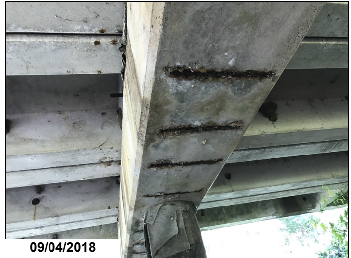
Typical spalls on bottom of caps.
