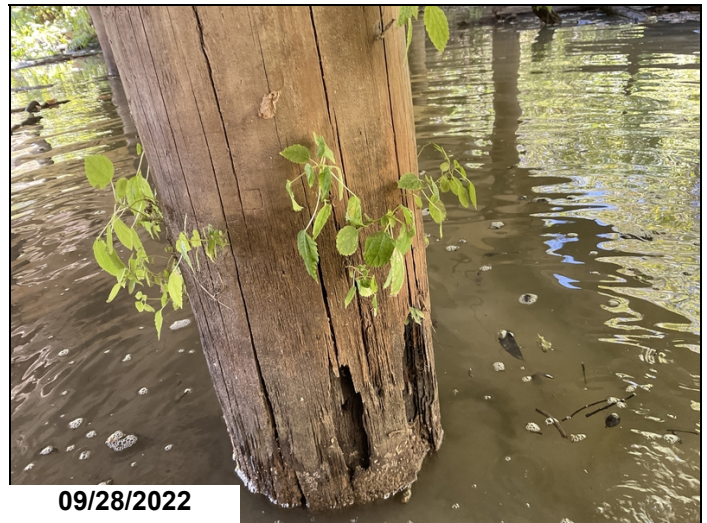
Bent #4 pile #2 has outer shell decay with moderate section loss.
