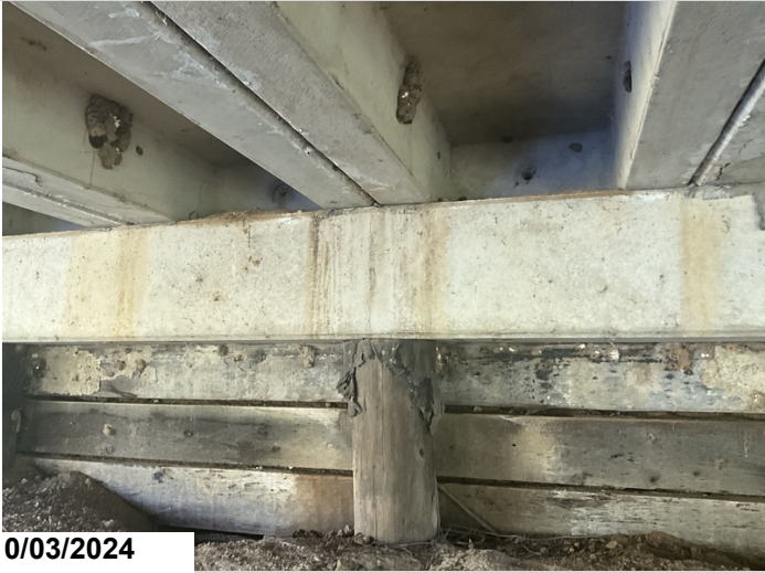
Bent 1: minor vertical crack above pile 3.
