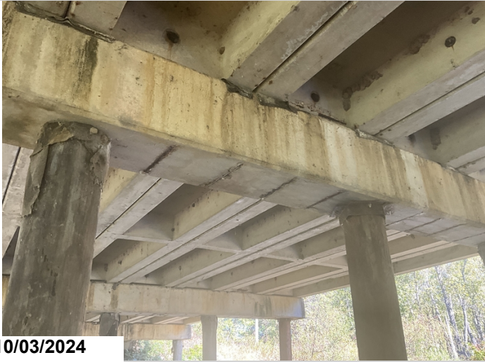
Bent 4, Bottom: Spalling with 20' of exposed reinforcing steel. CS3.
