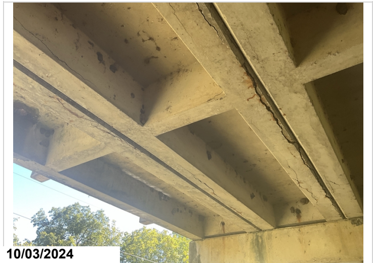
Span 5, Channel Unit7: large cracking.
