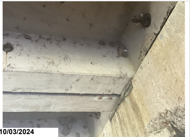
Span 2, Channel Unit 4: Minor shear type cracking.
