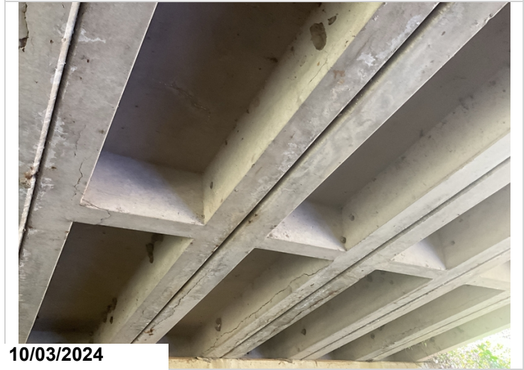
Span 6, Channel units: Longitudinal cracking.
