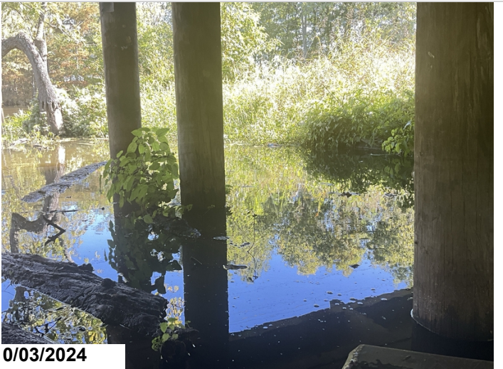
Bent 3, pile 4: Decay along the water line.
