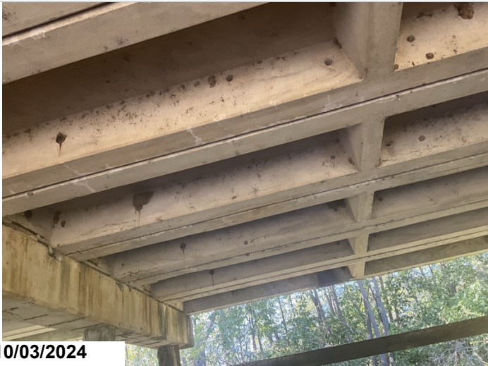
Span 5: Channel Units.
