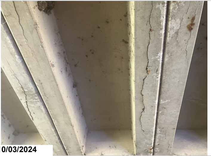
Span 6, Channel units: Longitudinal cracking.
