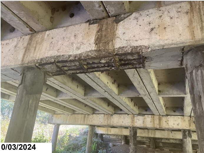
Bent 3, bottom: spalling with 19' exposed reinforcing steel. Cs3.
