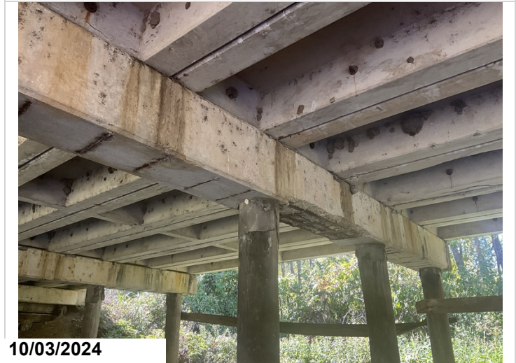
Bent 3, bottom: spalling with 19' exposed reinforcing steel. Cs3. Bent 2: 20.
