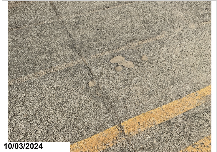
Span 5, Unit 4, wearing surface: 2' cs3 spalling.
