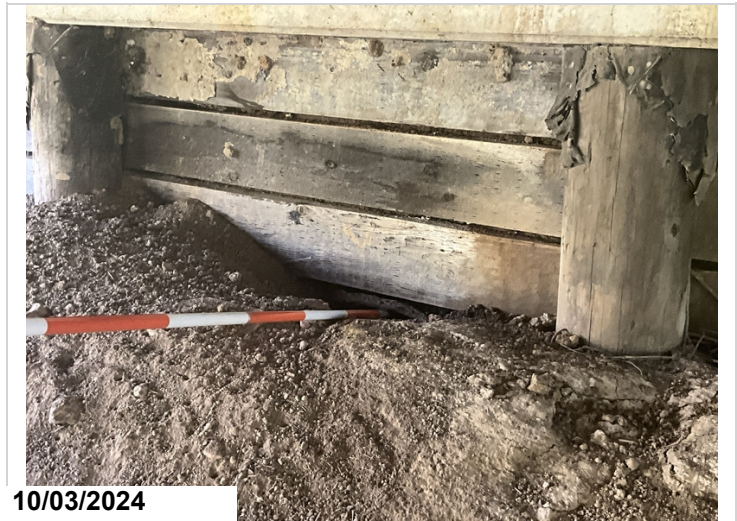
Bent 1, Between Piles 3 & 4: 2' erosion/void.
