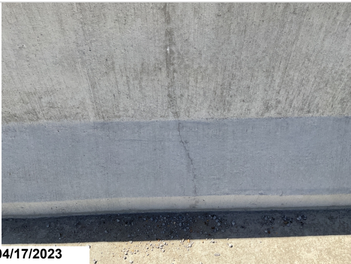
Typical hairline vertical crack in concrete bridge rail
