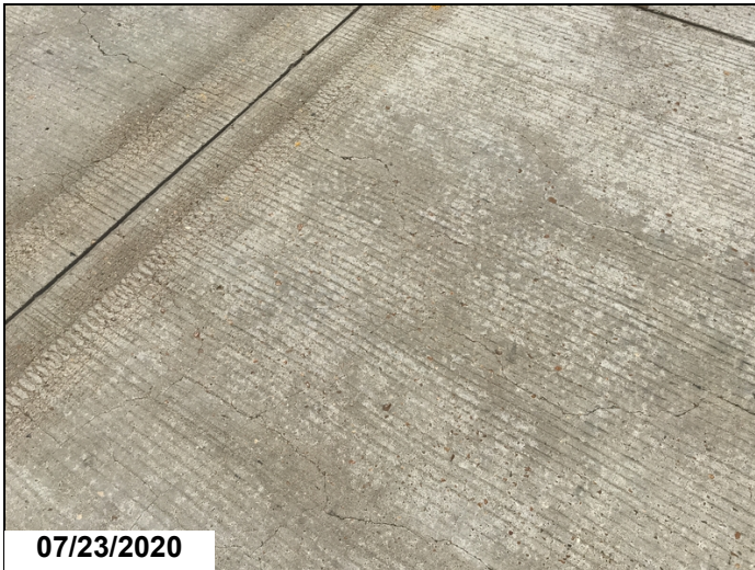
Abutment #1 approach slab map cracking.
