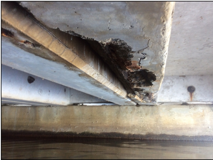
Span #3 unit #1 right leg spalled.
