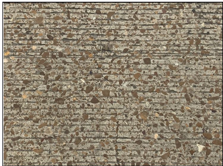
Typical longitudinal deck crack.
