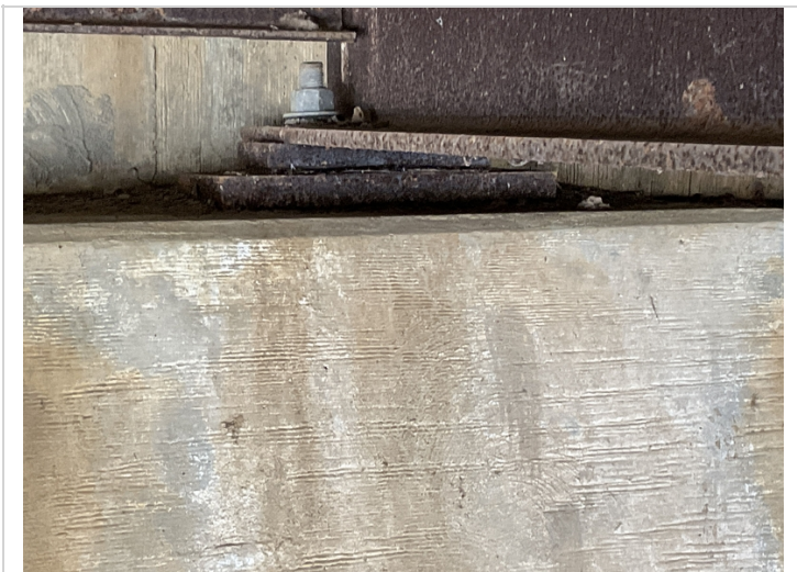
Typical abutment bearing
