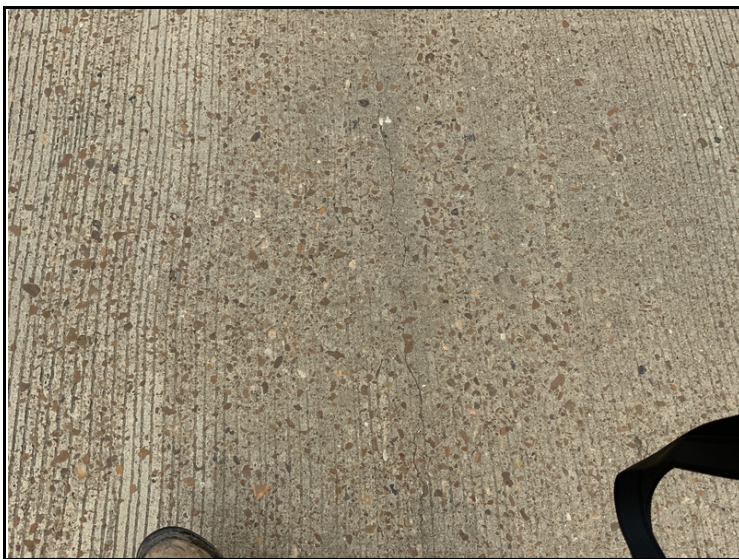
Typical transverse deck crack.
