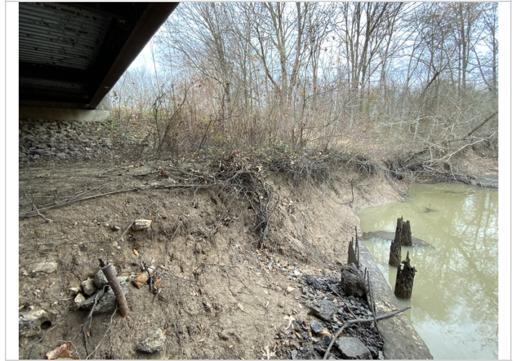
Abutment #1 left side channel eroded within 30' of bridge.
