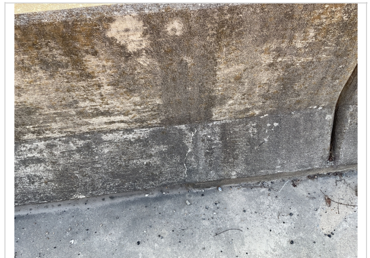
Typical bridge rail crack
