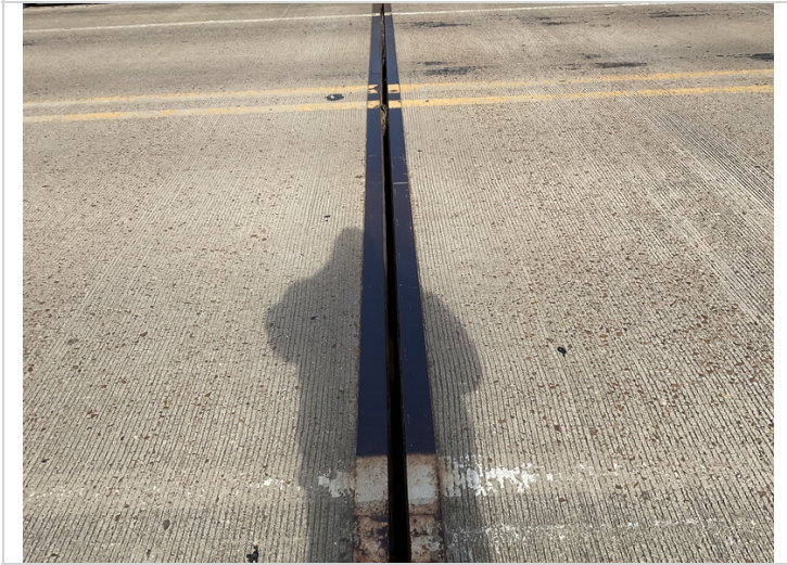
Bent #3 joint seal has failed.
