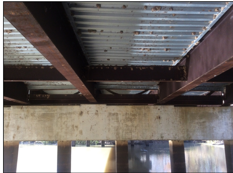
Bent #3 joint seal sagging onto cap
