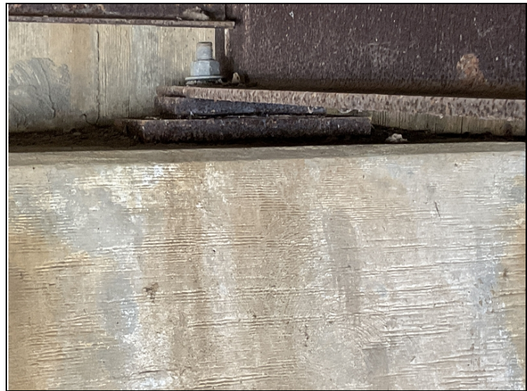
Typical abutment bearing
