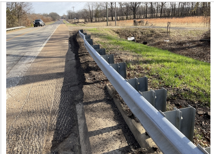
Abutment #2 right approach rail has minor collision damage.
