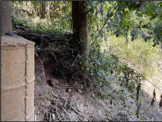
Bent #4 pile #5 has minor outer shell decay.
