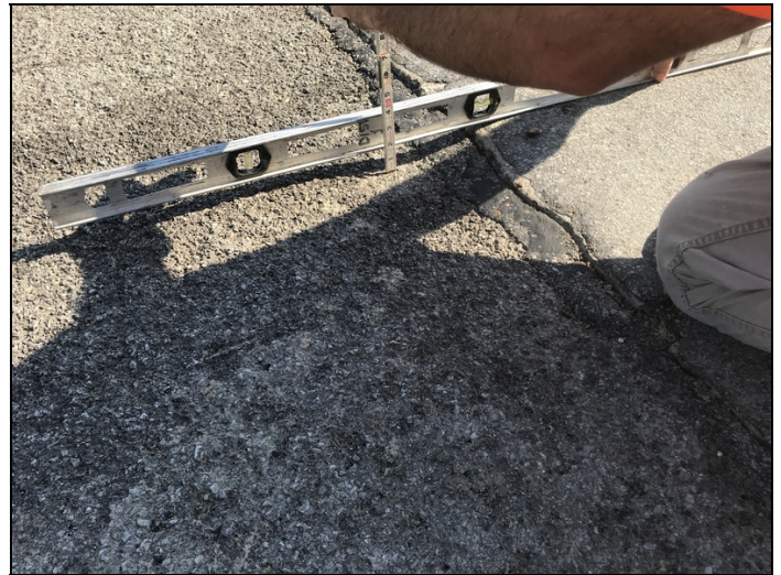
Abutment #2 approach roadway settlement.
