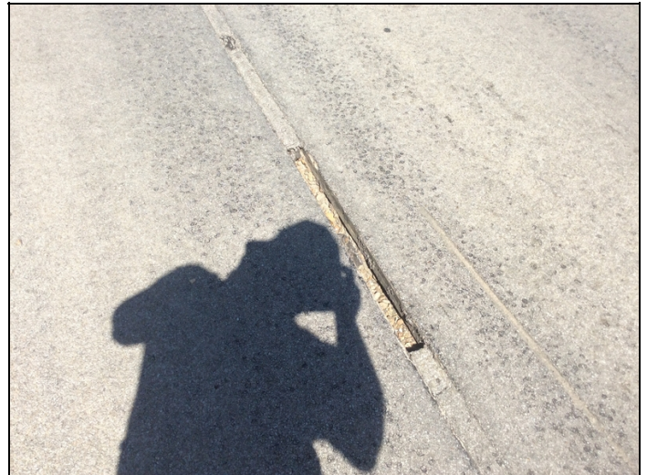
Span #3 deck joint between units #2,3 spalled three inches deep.
