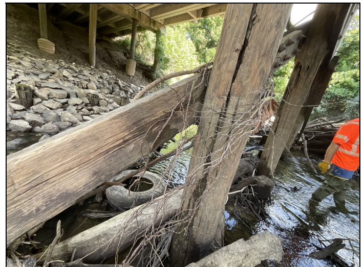
Bent #3 pile #2 has a split and outer shell decay with moderate section loss.
