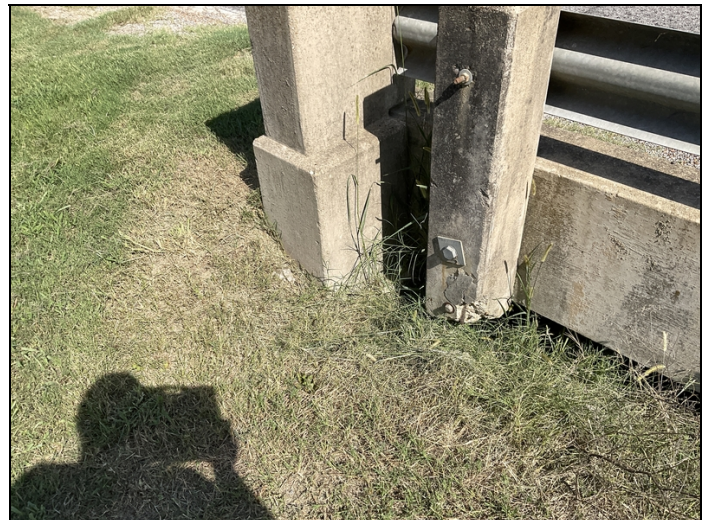
Span #4 left bridge rail last post is spalled at bottom with exposed rebar no section loss.
