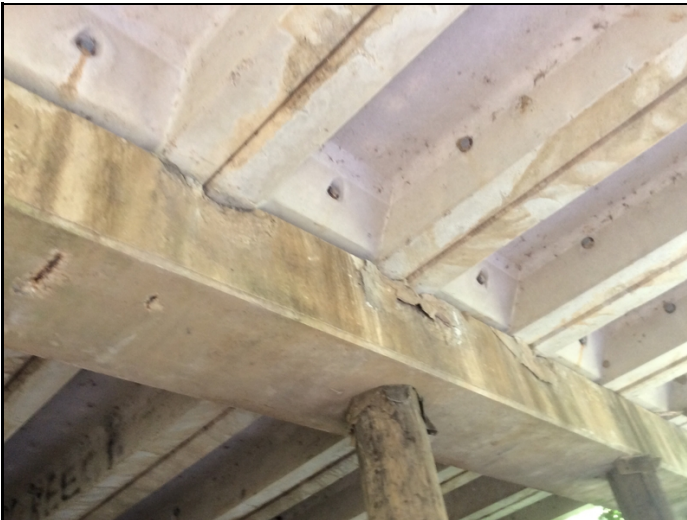
Bent #4 cap back face 6 sq ft spalls no rebar.
