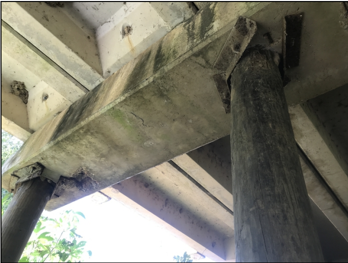
Bent #3 cap bottom face has 1' spall with exposed rebar with 5% section loss above pile #1.
