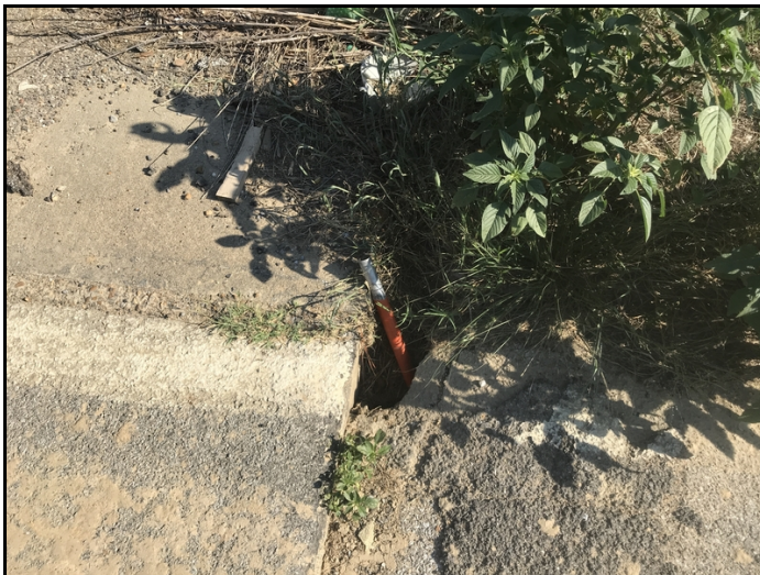
Hole in abutment #1 approach roadway, right side.
