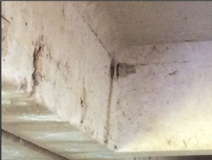
Loose bolt between units #4&5 span #1 typical other locations.
