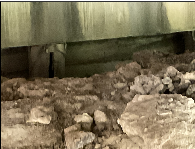
Bent #1 pile #3 is split 2" wide and core decayed with moderate section loss.
