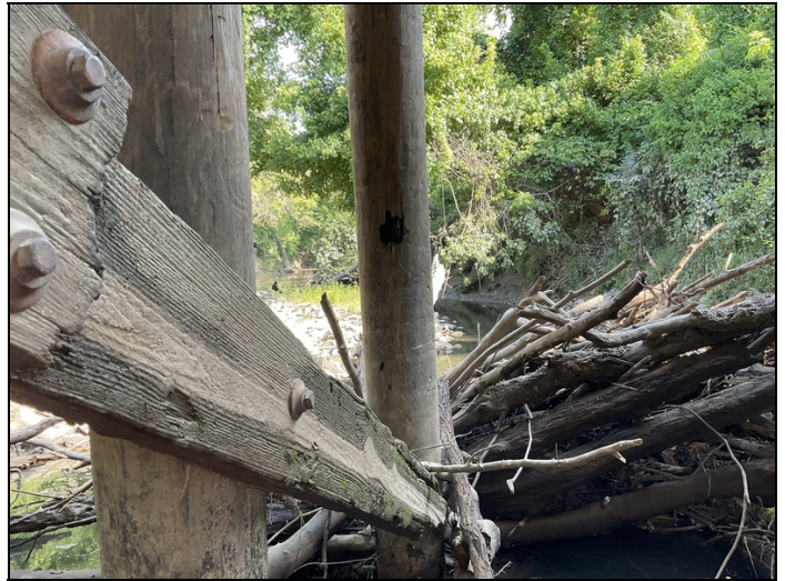
Bent #3 pile #5 each has outer shell decay with moderate section loss.
