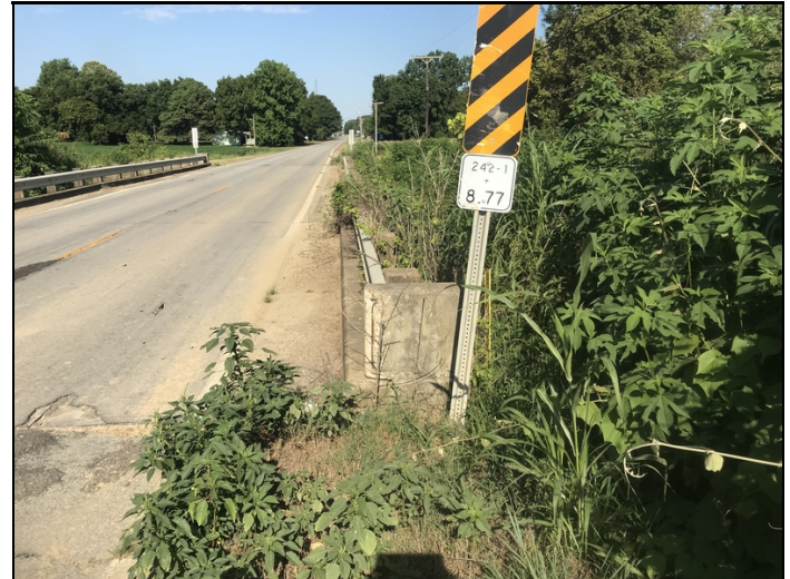
Vegetation growing beside, under and onto bridge.
