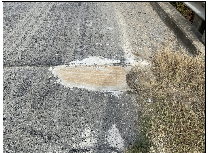
Abutment #1 hole in approach roadway repaired.
