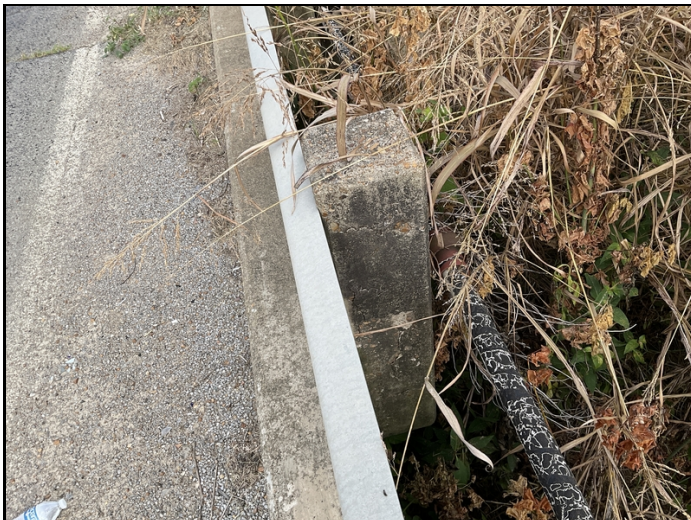
Span #4 right bridge rail span #4 post #4 has cs3 cracks and delaminated areas.
