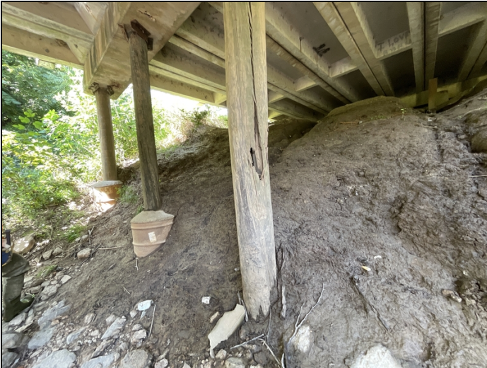
Bent #4 pile #3 has outer shell decay with moderate section loss and is split.
