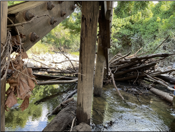
Bent #3 pile #3 has outer shell decay with moderate section loss.
