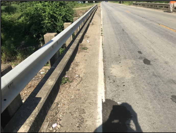
Dirt and debris in gutters.
