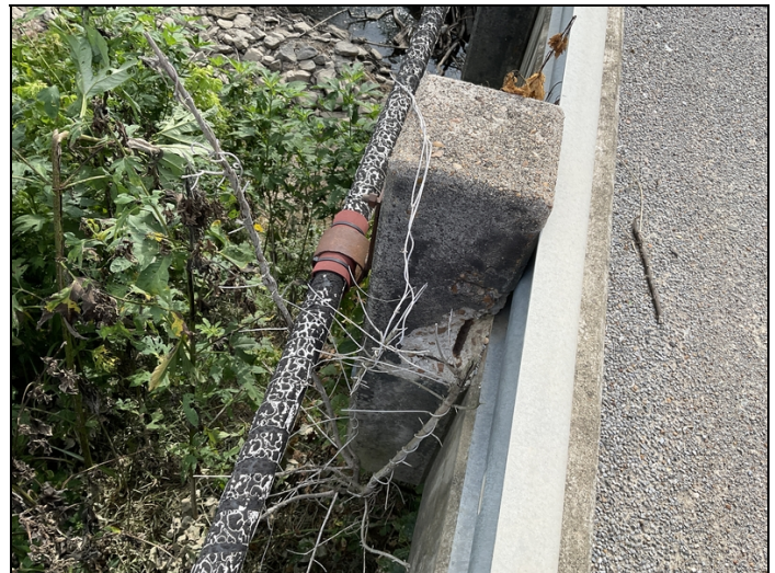
Span #4 right bridge rail span #4 post #2 is spalled with exposed rebar minor section loss.
