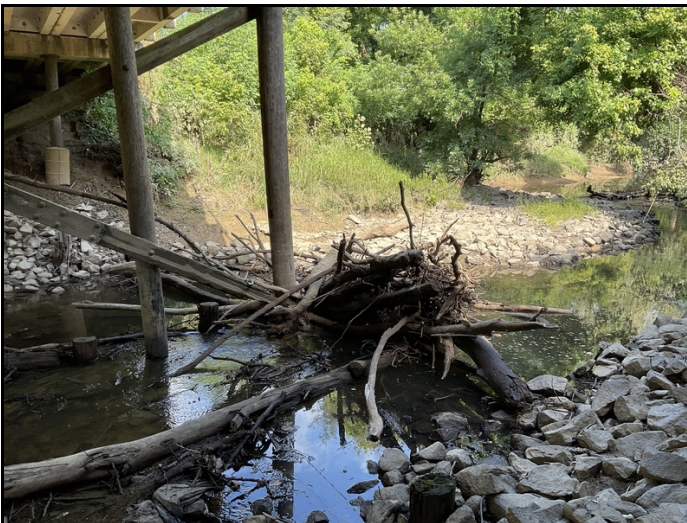
Drift in channel right side at bent #3
