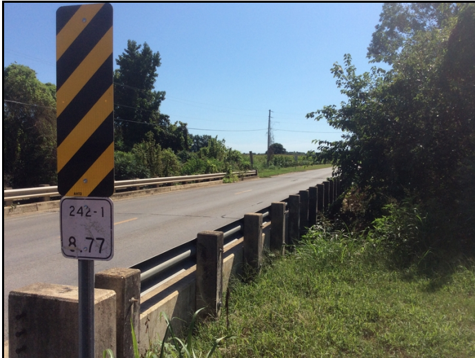
Trees and vegetation are growing beside and under bridge and onto roadway.
