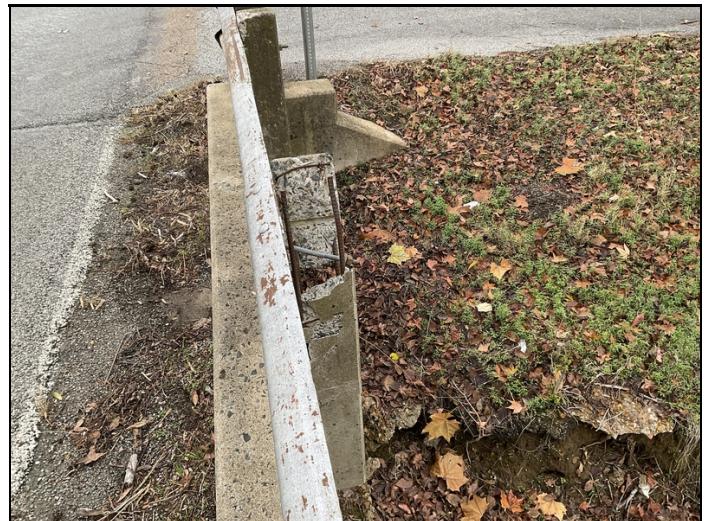
Fifth rail post right side broken, spalled with exposed rebar not connected to rail
