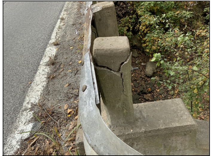
Abutment #1 right side first rail post broken.
