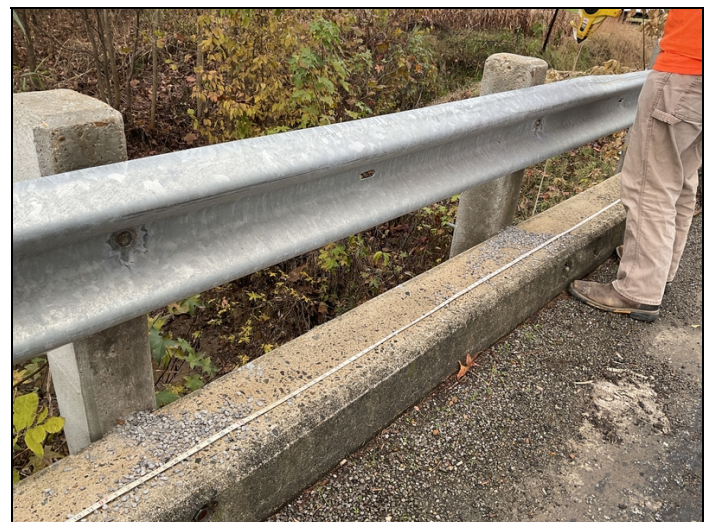
Left side, third and fourth rail posts not connected
