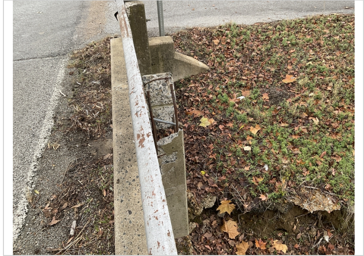
Fifth rail post right side broken, spalled with exposed rebar not connected to rail
