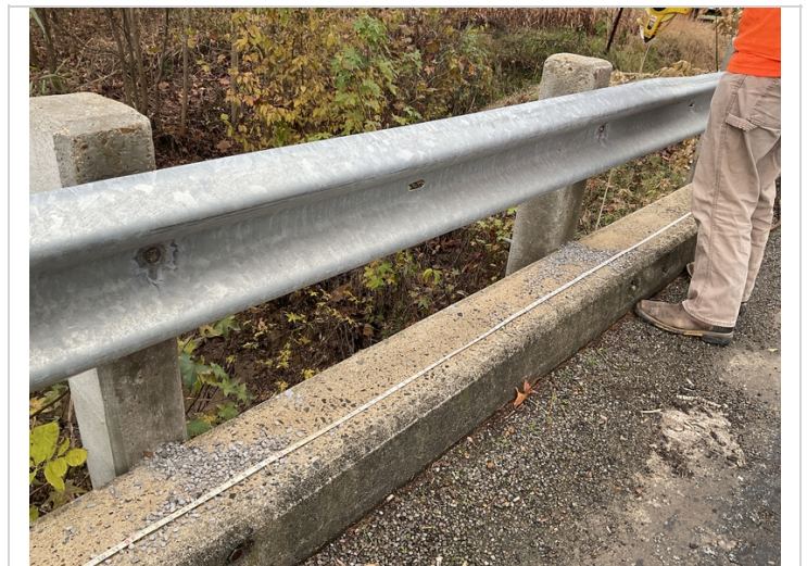
Left side, third and fourth rail posts not connected
