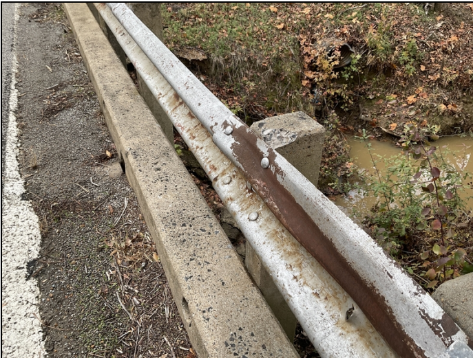
Second rail post right side has small spall with no exposed on top
