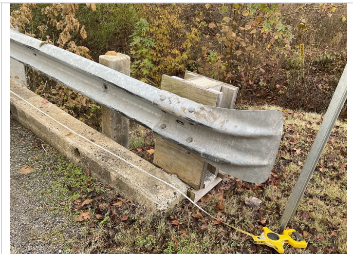
Left side rail posts #6 and 7 not connected, form left in place on rail post #7.
