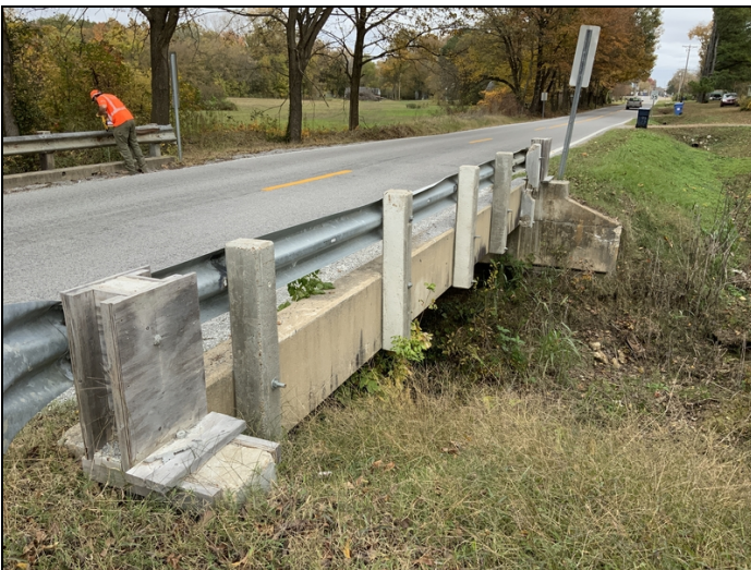
Second rail post on left side broken with exposed rebar. Fifth rail post on right side broken with exposed rebar. Abutment #1 and 2 left side first and last posts have been repaired, forms left in place.
