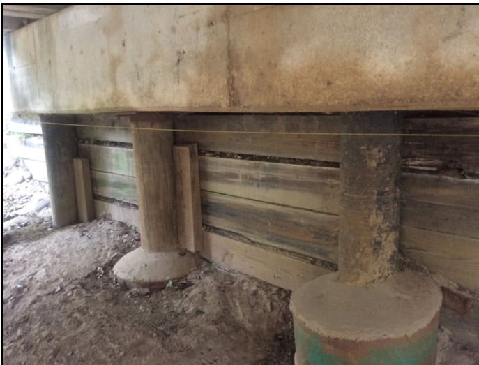
Abutment #2 back wall behind piles #4&5
