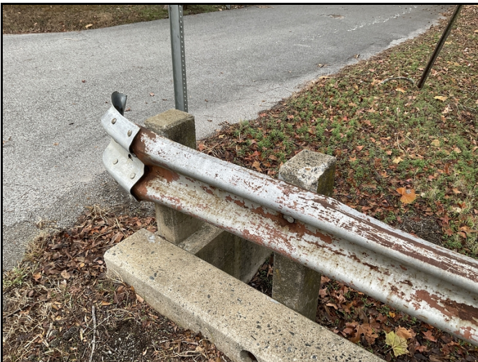
Sixth rail post right side has small spall on top with no exposed rebar end of rail has minor collision damage
