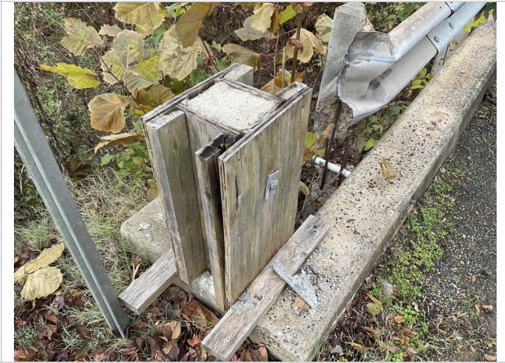
Abutment #1 left rail post has been repaired with form left in place. Second rail post broken, spalled with exposed rebar, first four feet of rail missing.
