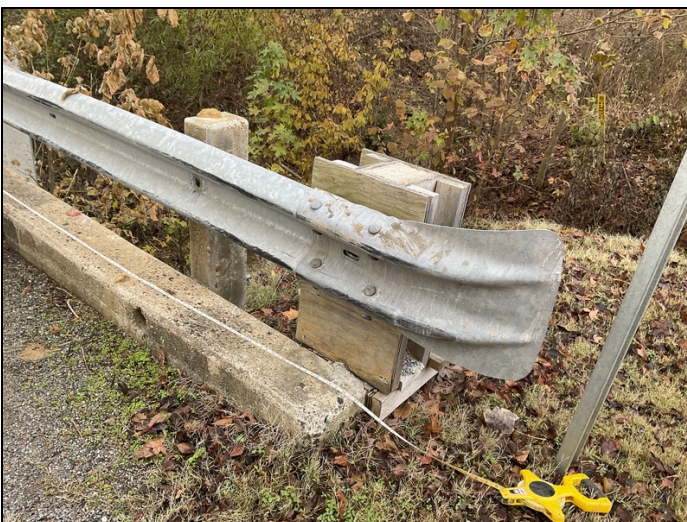
Left side rail posts #6 and 7 not connected, form left in place on rail post #7.
