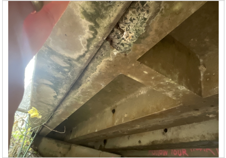
Unit #1 left leg spalled at half and three quarter span with no exposed rebar.
