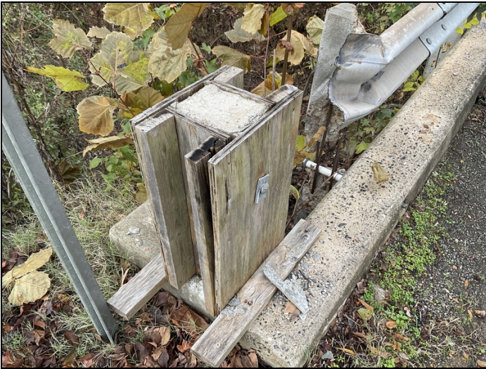
Abutment #1 left rail post has been repaired with form left in place. Second rail post broken, spalled with exposed rebar, first four feet of rail missing.
