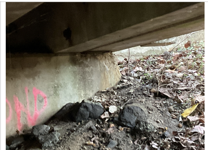
Abutment #2 cap back face right side has six inch shallow spall with no exposed rebar.
