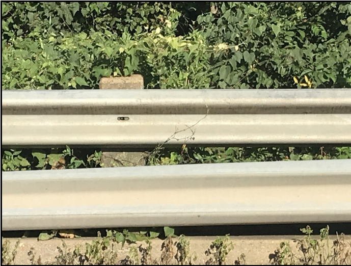
Span #3 left side fourth rail post missing bolt.
