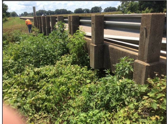
Vegetation growing beside and under bridge both side of both abutments
