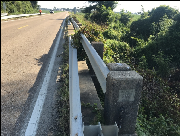
Vegetation growing in gutters and beside, under and onto bridge.
