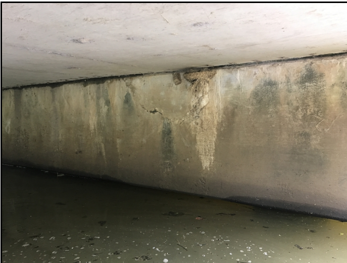
Delamination on bent #3 ahead face left side.
