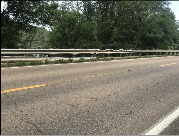
Left rail damage spans #1 and 2.
