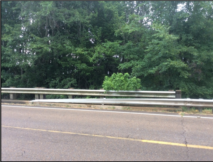
Trees and vegetation are growing beside and under bridge bridge and onto roadway.
