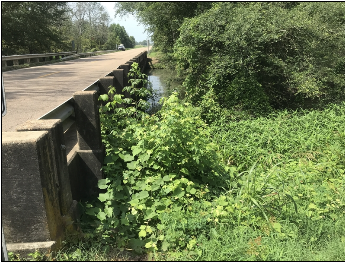
Trees and vegetation growing beside and under bridge left side.
