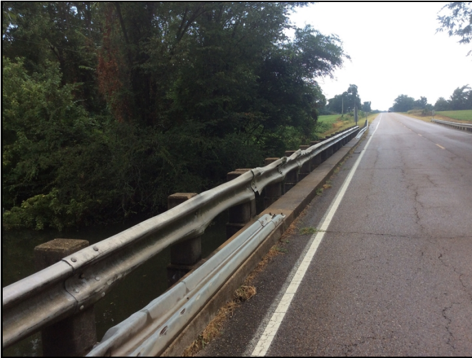
Span #1,2 bridge rail has collision damage full length.
