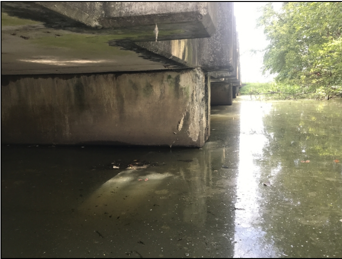
Bent #2 cap right end cracked with efflorescence last 1'.
