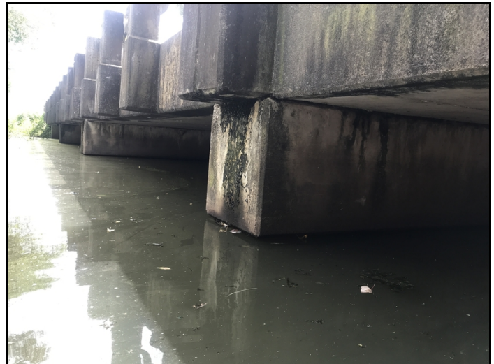
Bent #2 cap left end spalled with no exposed rebar.
