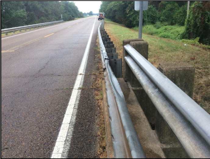
Abutment #1 left approach rail has multiple areas of collision damage.
