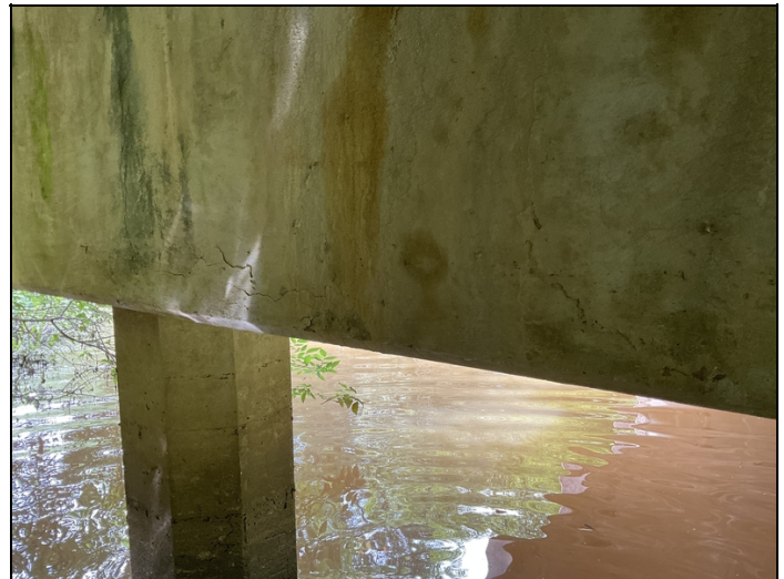
Bent #4 cap right side ahead face 3' from end has a 1' delaminated area and a 6" delaminated area.
