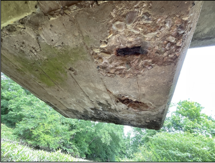
Bent #4 cap on bottom left end has 1' spall exposed rebar moderate section loss.
