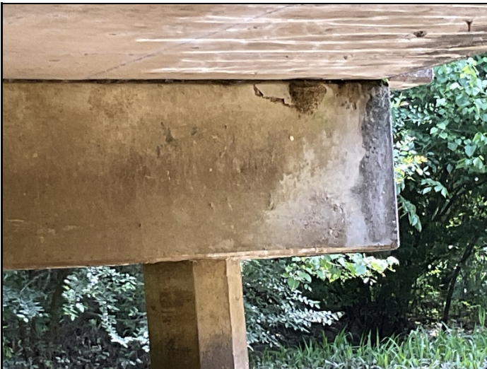
Bent #2 cap back face 1' from right side has a 1' delaminated area at top.
