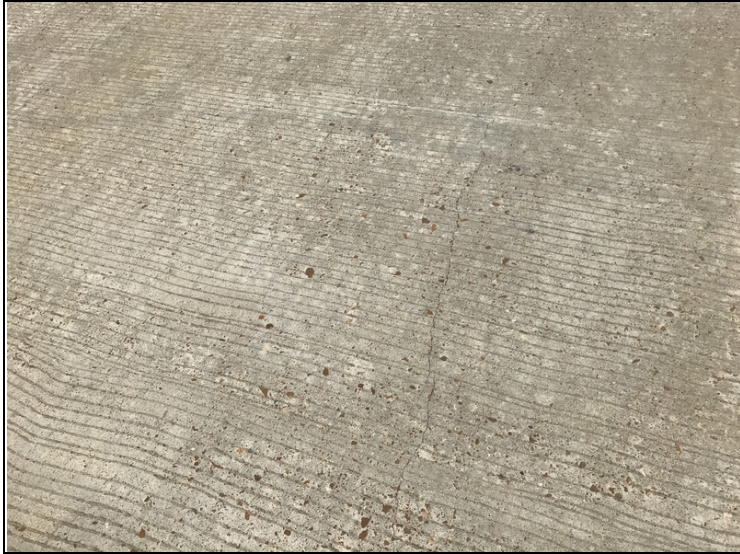
Typical longitudinal deck crack.
