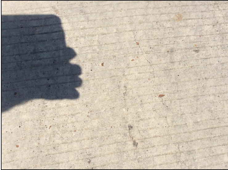
Typical longitudinal deck crack
