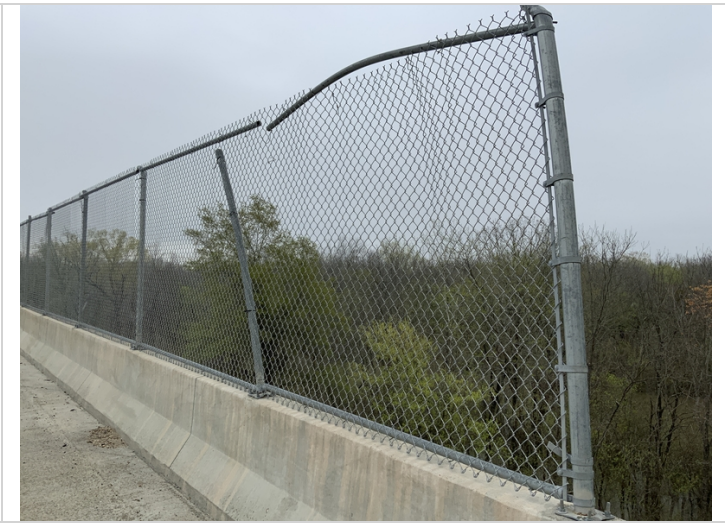
Damage chain link fence
