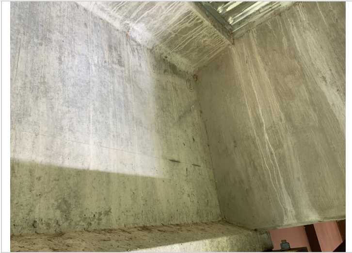
Bent 81 - span 80 - girder 3 has a diagonal crack with efflorescence
