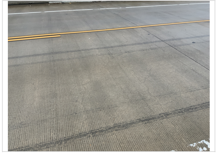
Map cracking
