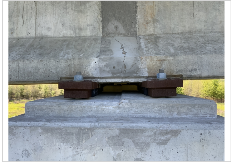
Typical bearings along the North prestressed girder unit on 04/12/2021 @ 9:45am with temps at 68 degrees
