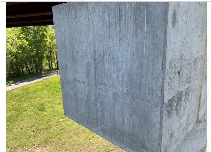
Typical cracking along the face of the pier caps
