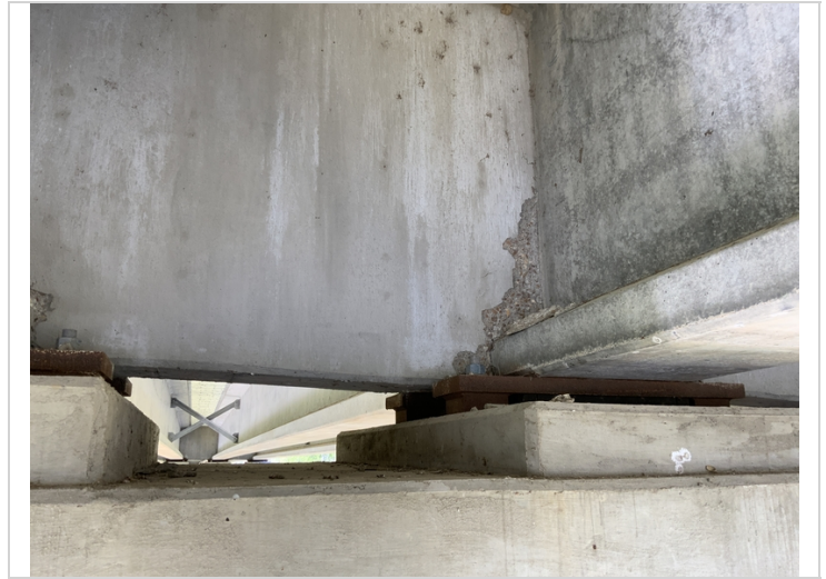
Typical spalling along the diaphragms
