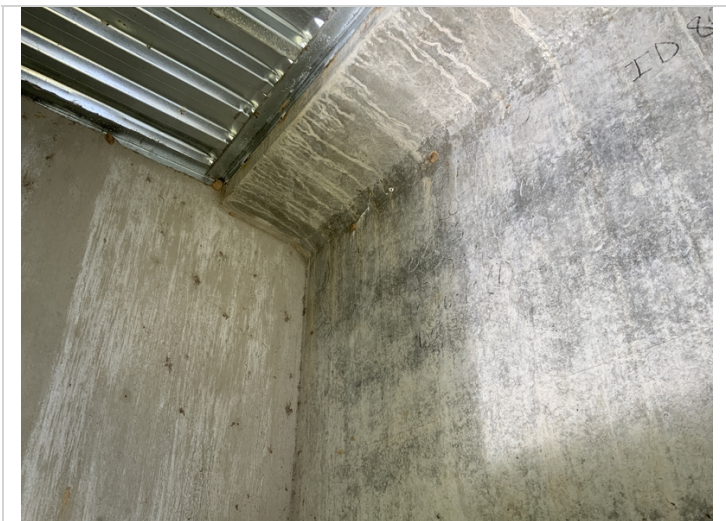
Bent 80 span 80 girder 1 has cracking with efflorescence along the top flange web juncture
