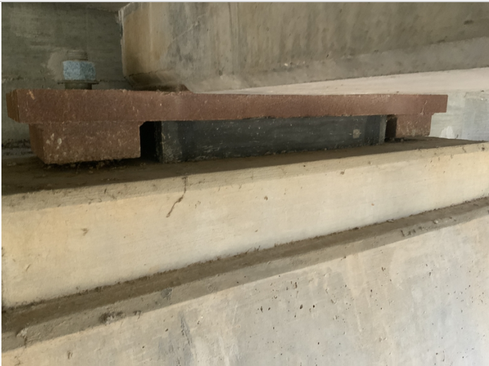
Typical bearings at bent 97
