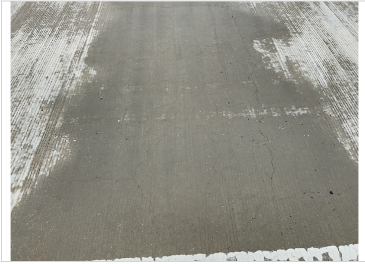
Map cracking
