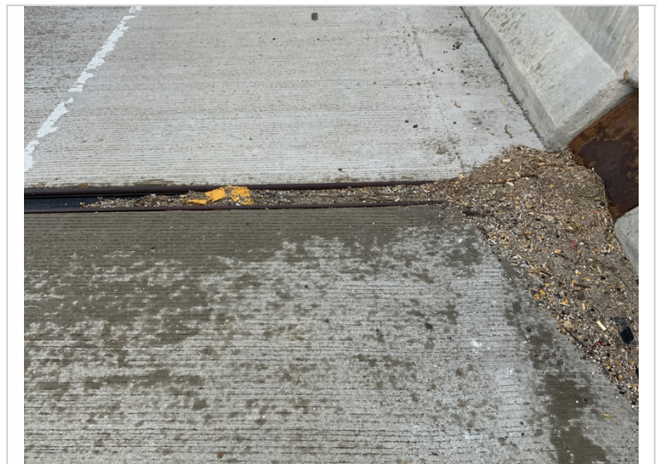
Typical debris accumulation along the gutters
