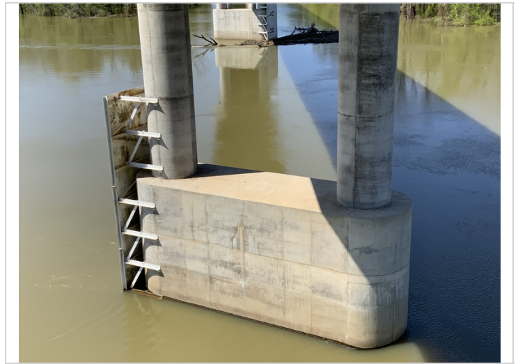
Pier walls 1 and 2 have vertical cracking with efflorescence
