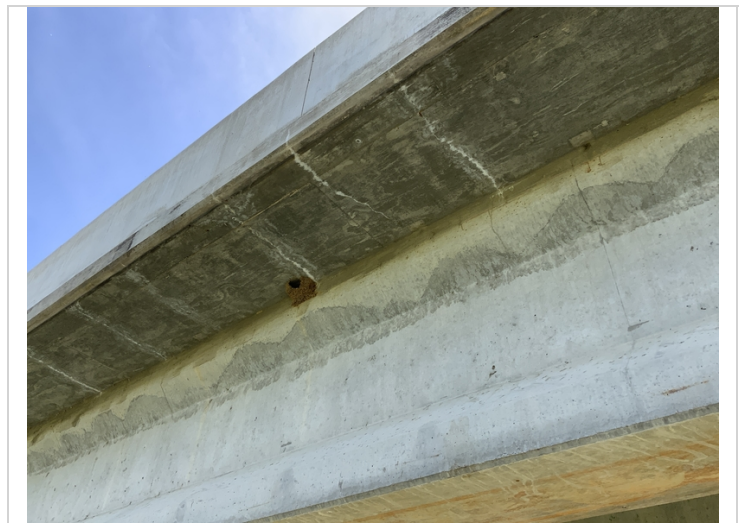
Typical cracking with efflorescence along the overhangs
