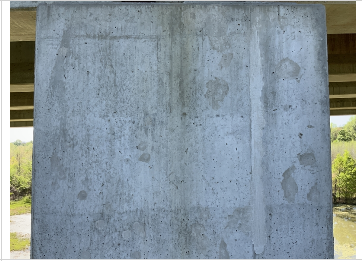
Bent 90 (upstream) has vertical and horizontal cracking along the face of the cap in the North prestressed girder unit
