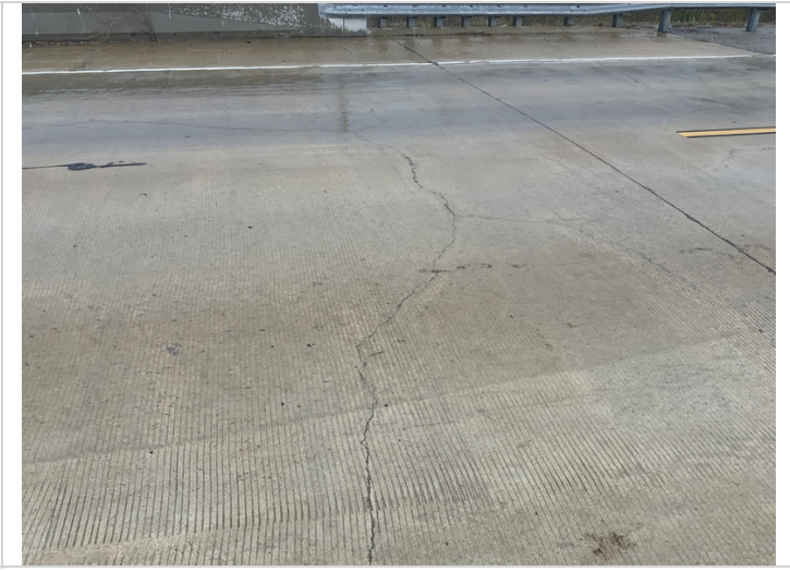
Typical cracking along bent 97 south approach
