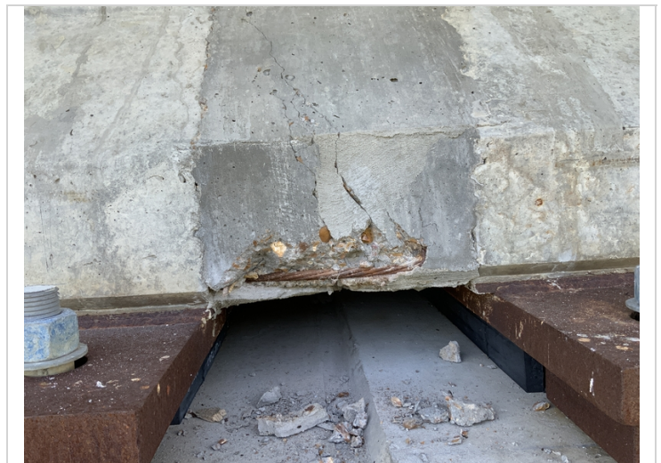
Bent 91 - Girder 1 (Upstream) has spalling with exposed prestressed strands where the girder is made continuous along the North prestressed girder unit
