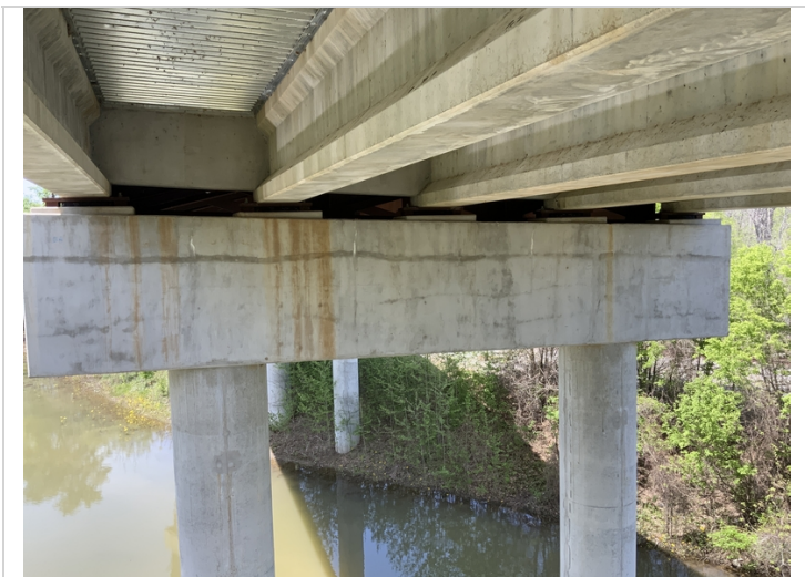
Bent 64 has 4 vertical cracks with efflorescence
