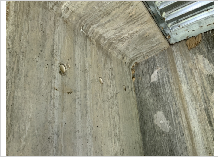
Span 85 - Girders 4 & 5 has cracking along the top flange web juncture with efflorescence and diagonal cracking center of the web adjacent to bent 86
