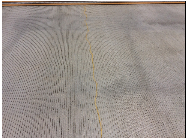
Sealable Transverse cracks.
