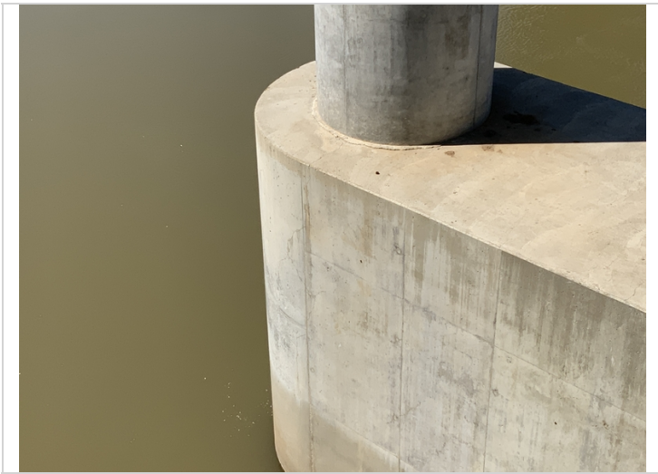
Pier 3 has map cracking along both ends of the pier wall
