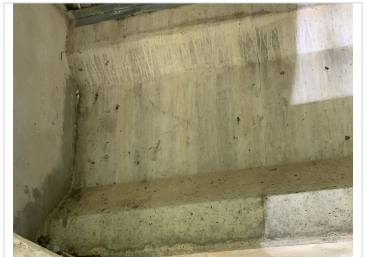
Typical diagonal cracking
