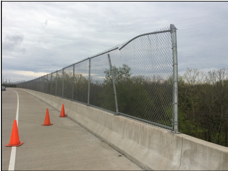
Steel Girder Spans, Chain Link Fence: Approximately 30' of damaged fencing.
