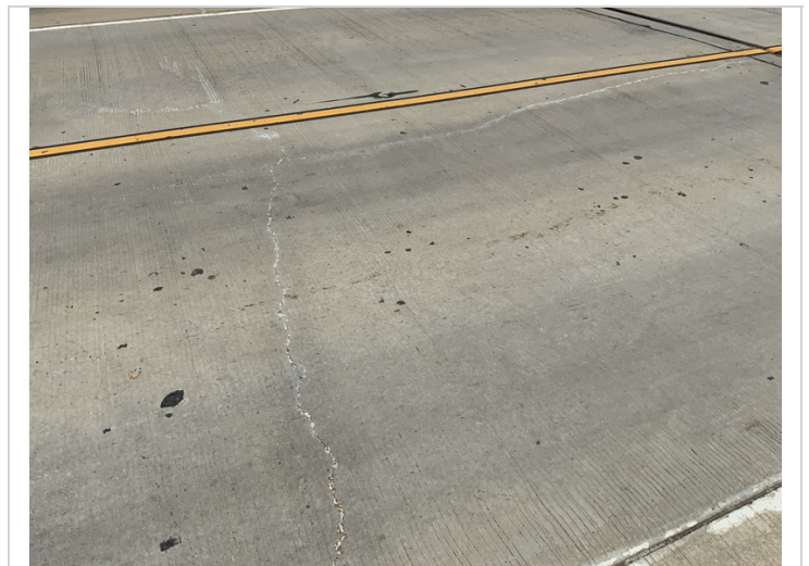
Typical transverse and longitudinal cracking along bent 1 South Approach
