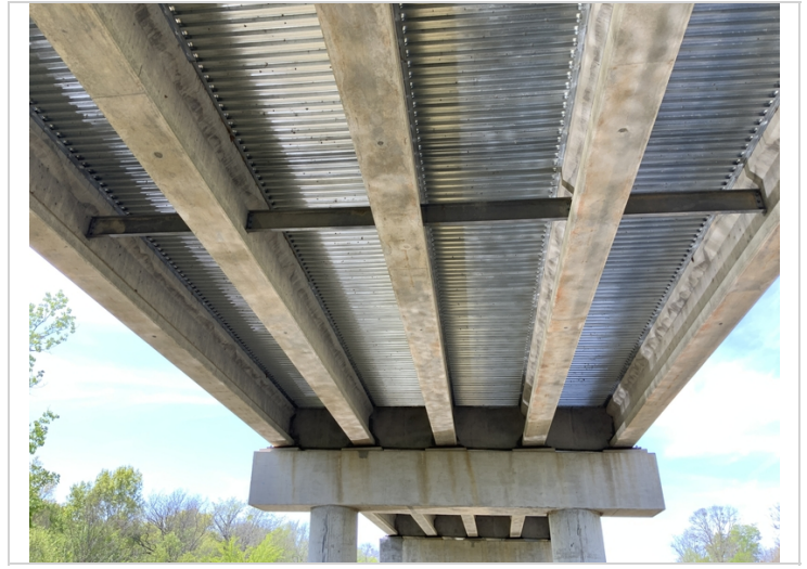
Typical under surface of prestressed girder units
