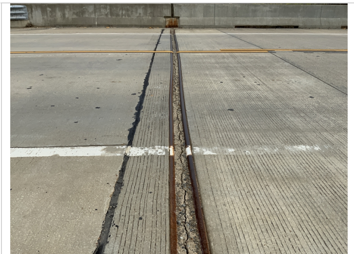
Bent 1 joint has debris impactation
