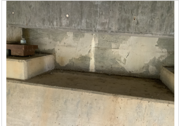
Bent 97 North Abutment typical vertical cracking with efflorescence
