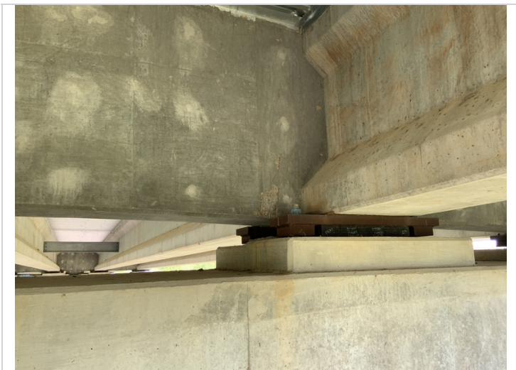
Typical spalling along the diaphragms in various locations throughout the north prestressed girder unit
