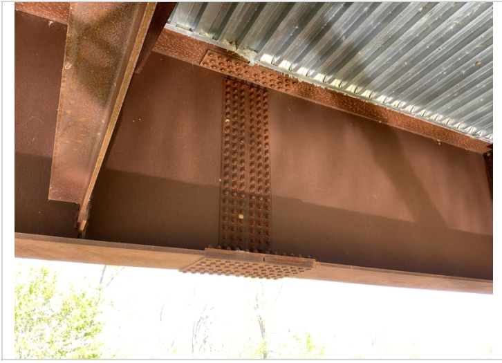
Typical splice plate connections
