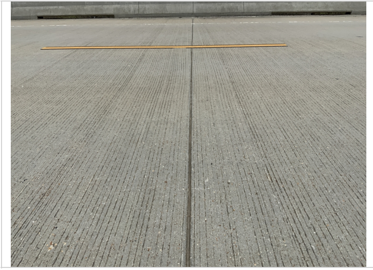
Typical saw joints
