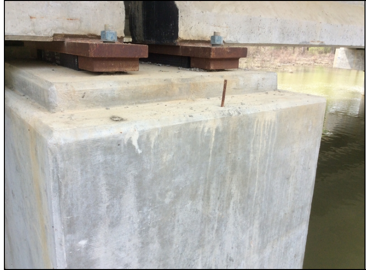
Left side bent 5 piece of all thread sticking up out of cap.
