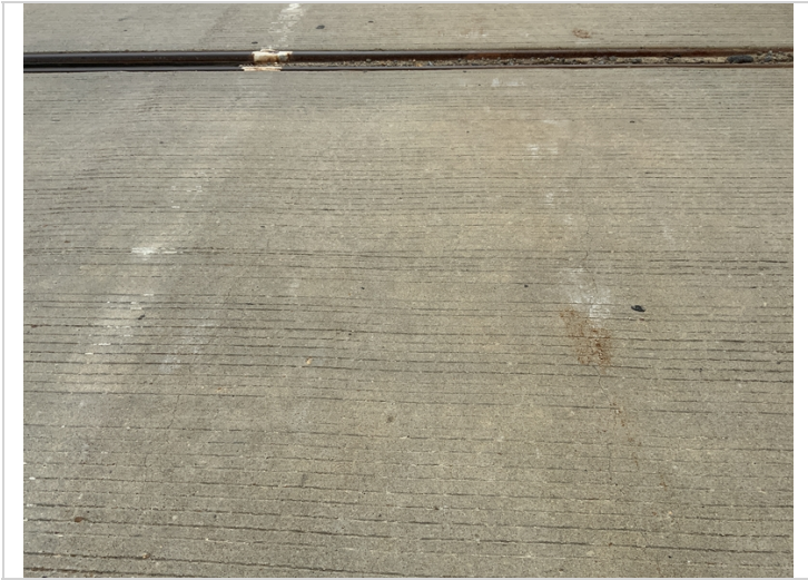
Typical longitudinal cracking adjacent to the joint seals
