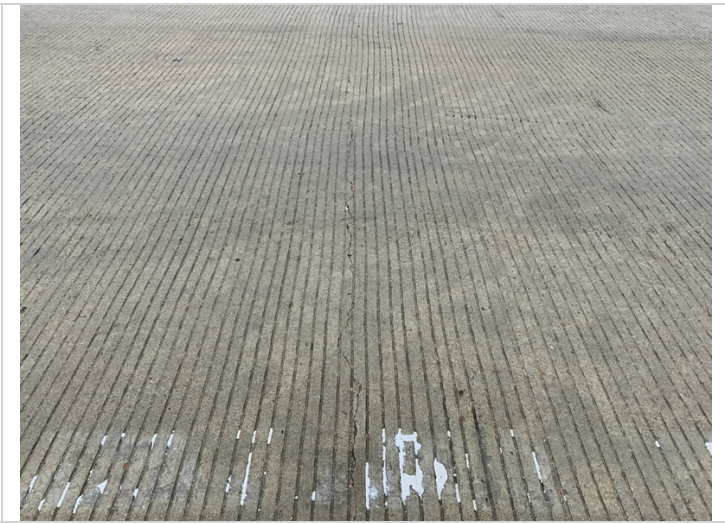
Typical transverse cracking
