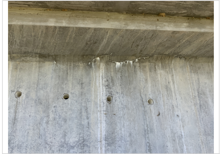
Bent 88 - Girder 1 (upstream) has diagonal cracking with efflorescence along the top flange web juncture
