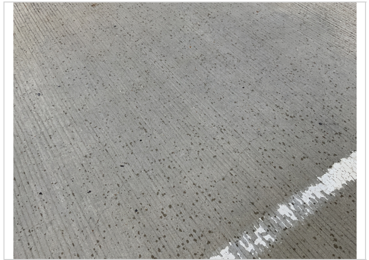
Minor map cracking
