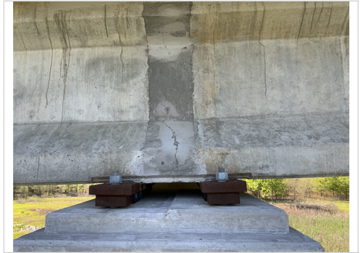
Typical cracking along the exterior girders where the girders were made continuous
