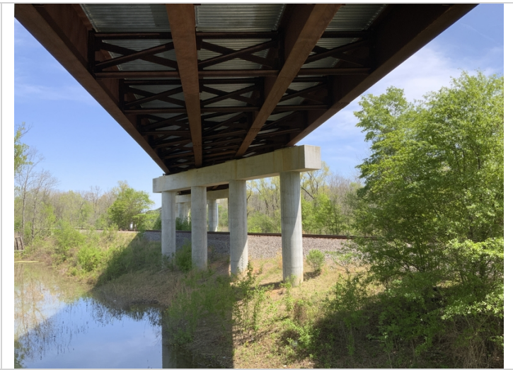
Typical under surface of multi steel girder units
