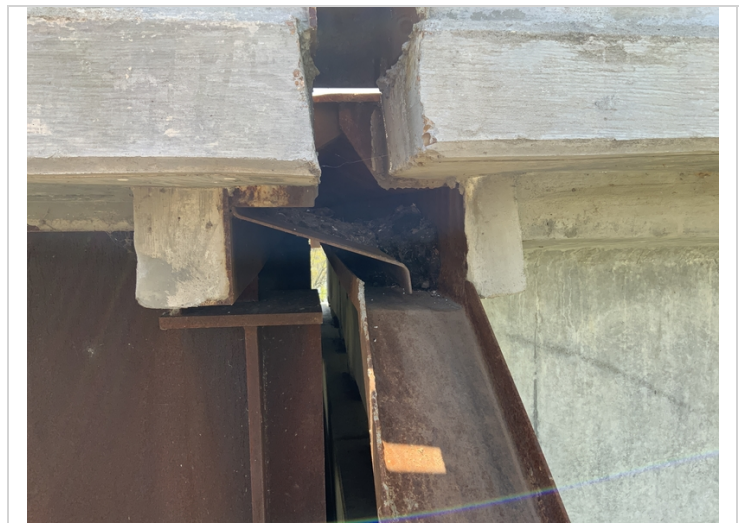
Joints have a accumulation of debris
