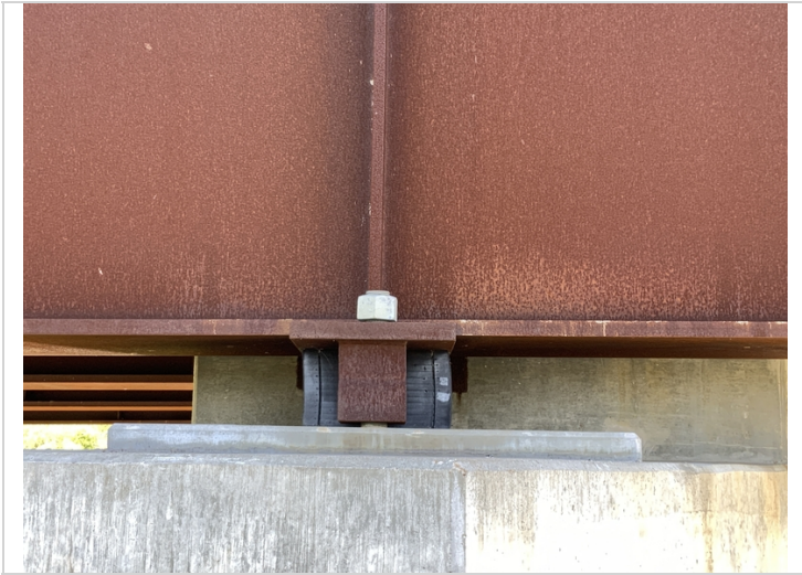
Typical bearings on 04/12/2021 @ 11:28am with temperature at 81 degrees
