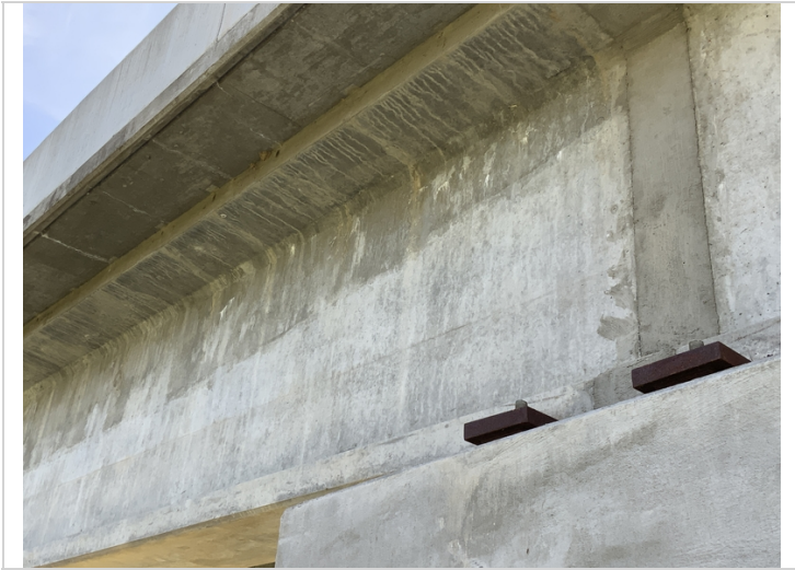
Bent 77 - Girder 1 has hairline cracking with efflorescence along the web
