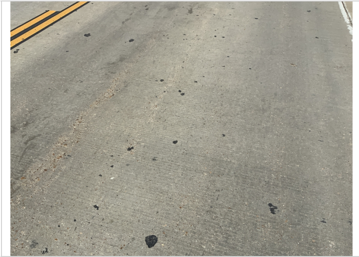
Bent 1 South approach has minor abrasion
