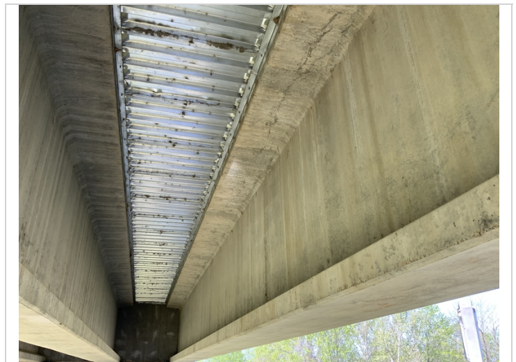
Span 87 - Girder 1 (upstream) has map cracking along the to flange and the top web juncture
