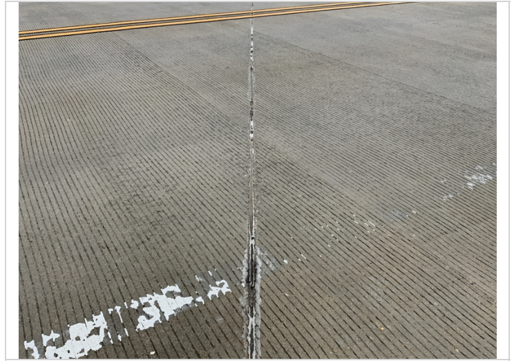
Typical deteriorated saw joints
