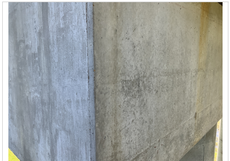
Bent 91 has horizontal cracking along the face of the cap on the upstream side and extends around on the back side of the cap in the North prestressed girder unit
