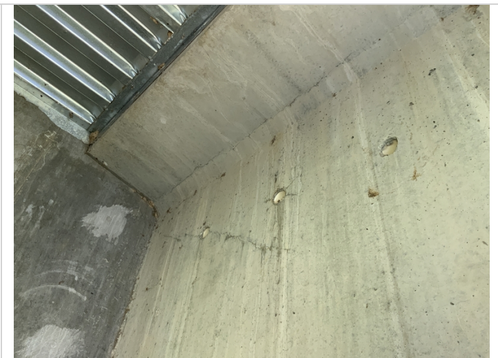
Bent 85 - Girder 2 (span 84) in bay 1 and 2 has a 45 degree crack that starts at the top web juncture and extends down approximately 3' and a longitudinal crack that follows along the top flange web juncture
