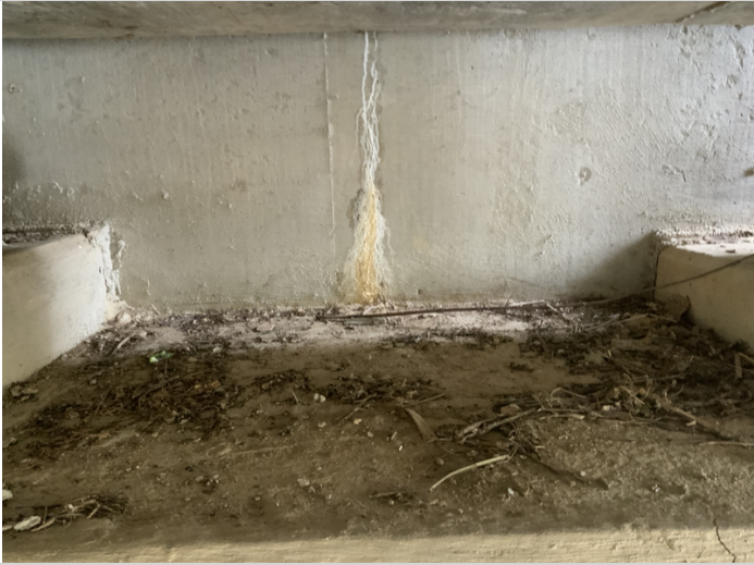
Typical vertical cracking with efflorescence along bent 1 South abutment
