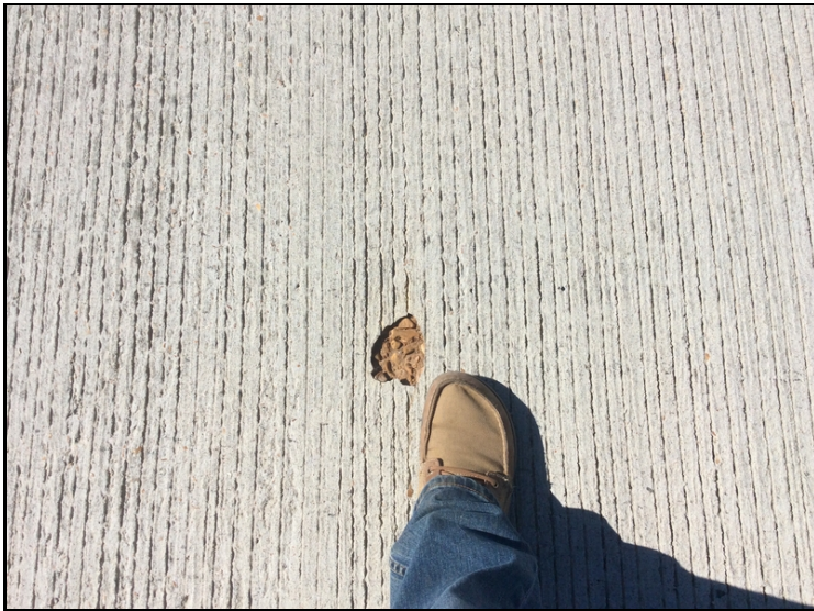
Spall in Deck located at Pier 1 north bound right lane.
