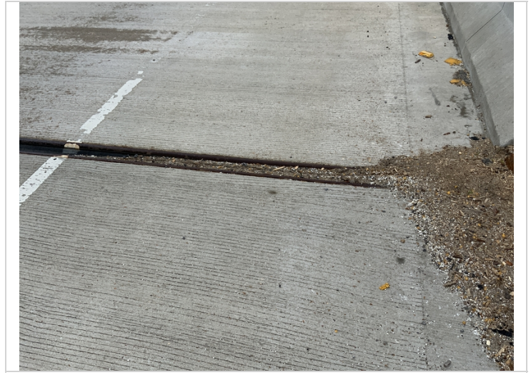
Typical debris accumulation
