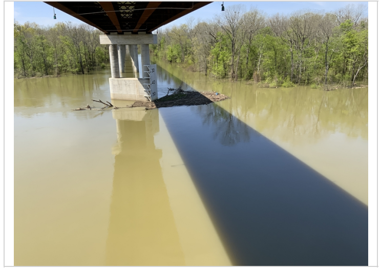
Pier 1 drift accumulation
