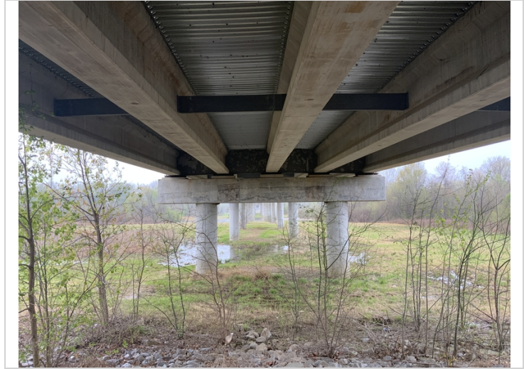
Typical under surface of the prestressed girder units
