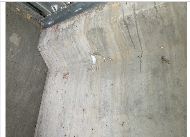
Bent 90 - Girder 1 (upstream) has minor cracking with efflorescence leaching through along the North prestressed girder unit
