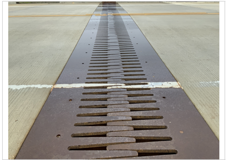
Typical finger joints
