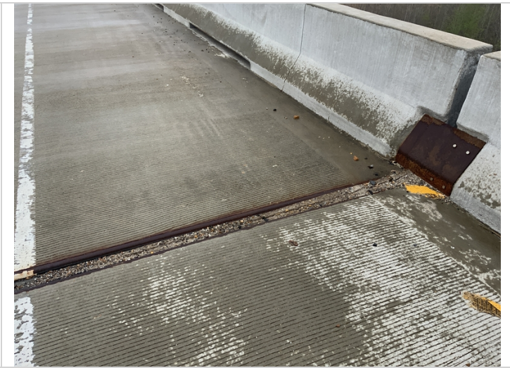
Typical debris accumulation
