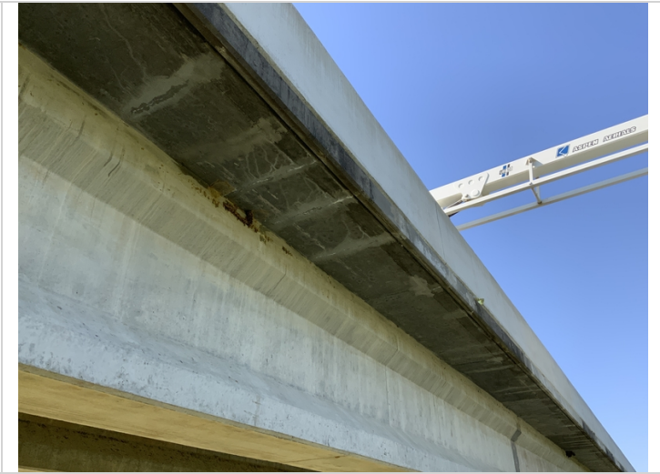
Typical transverse cracking with efflorescence along the overhangs of the North prestressed girder unit
