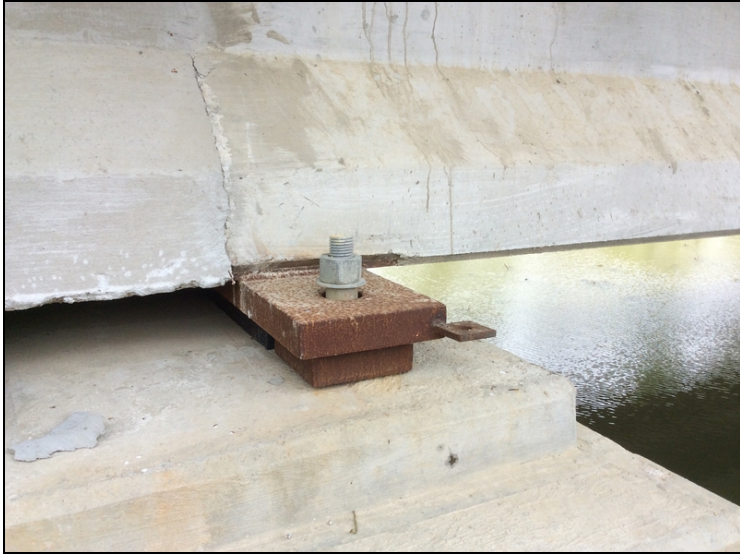
Bent 4 girder 1 bearing has a piece of metal welded to bearing plate.
