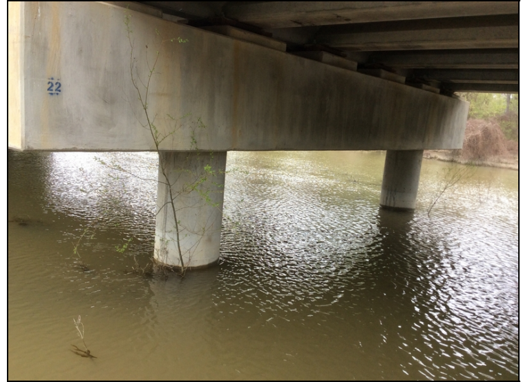
Looking back at bent 22, trees growing against columns.
