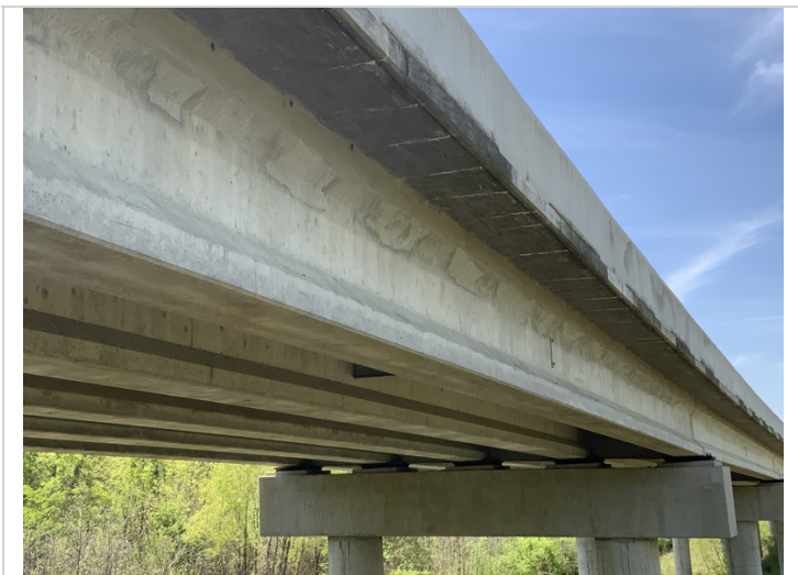
Typical cracking with efflorescence along the overhangs
