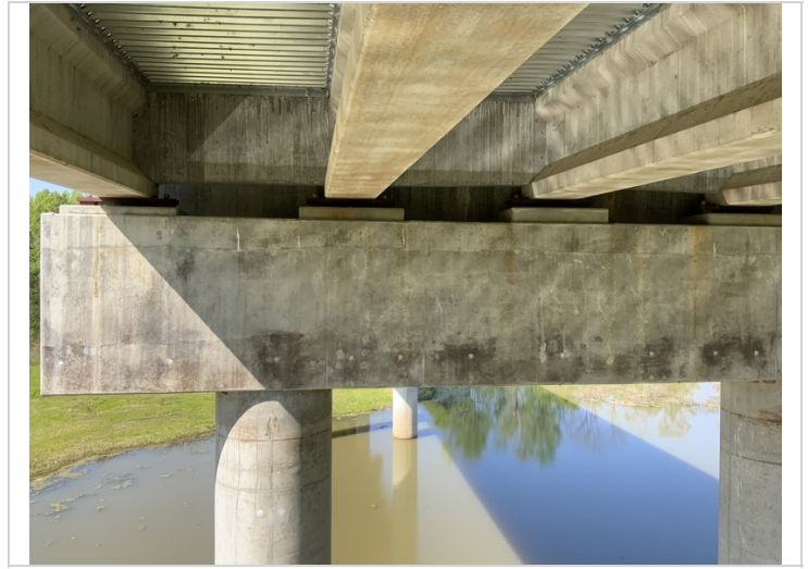
Bent 89 (AHD) has 6 vertical cracks with efflorescence along the North prestressed girder unit
