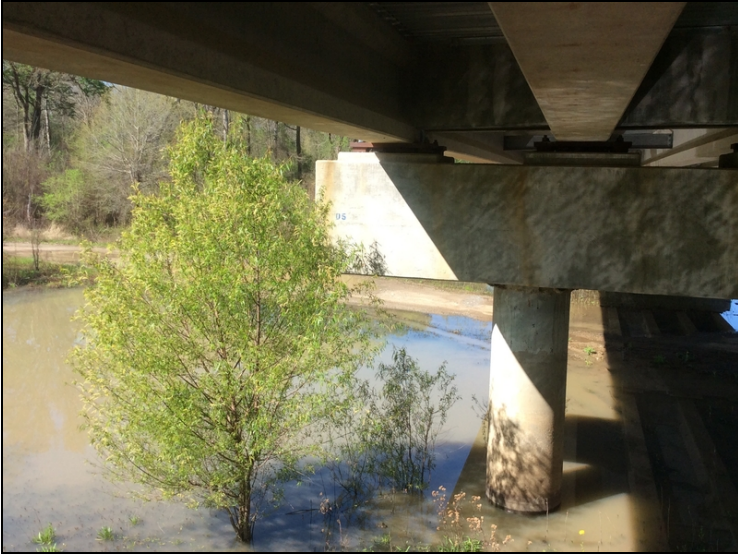
Bent 5 tree needs to be removed. Bent 14 similar.
