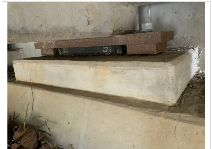
Typical bearings at bent 1
