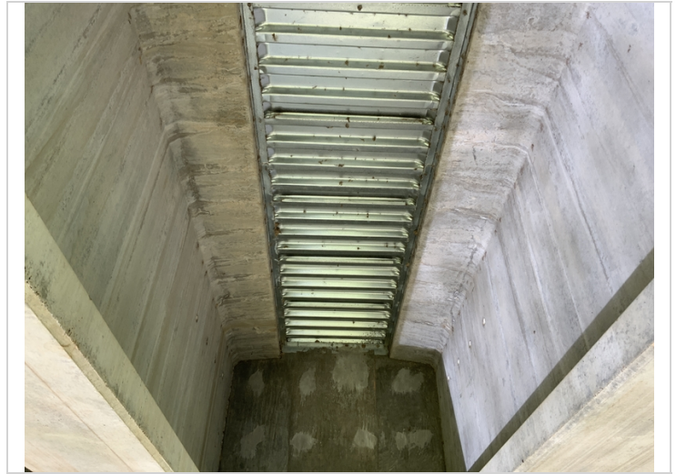
Span 85 - Girders 1 thru 6 (adjacent to bent 85) has cracking with efflorescence along the top flange and web juncture
