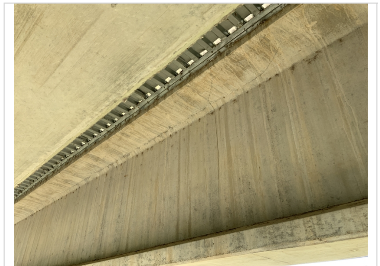
Span 84 - Girder 1 has 2 diagonal cracks along the top flange and a longitudinal crack along the top flange web juncture that starts approximately 20' from bent 85 and extends 30' towards bent 84
