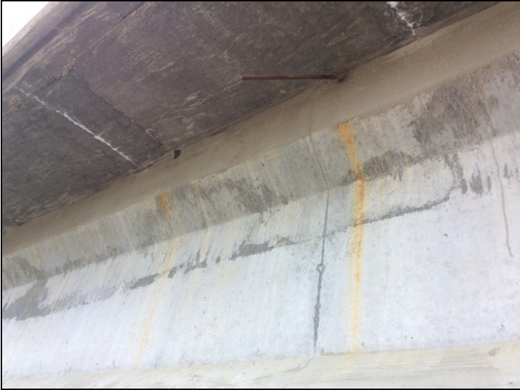
Span 52 girder 1 a piece of all thread was left.
