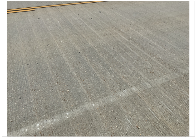
Typical abrasion in various locations throughout the structure
