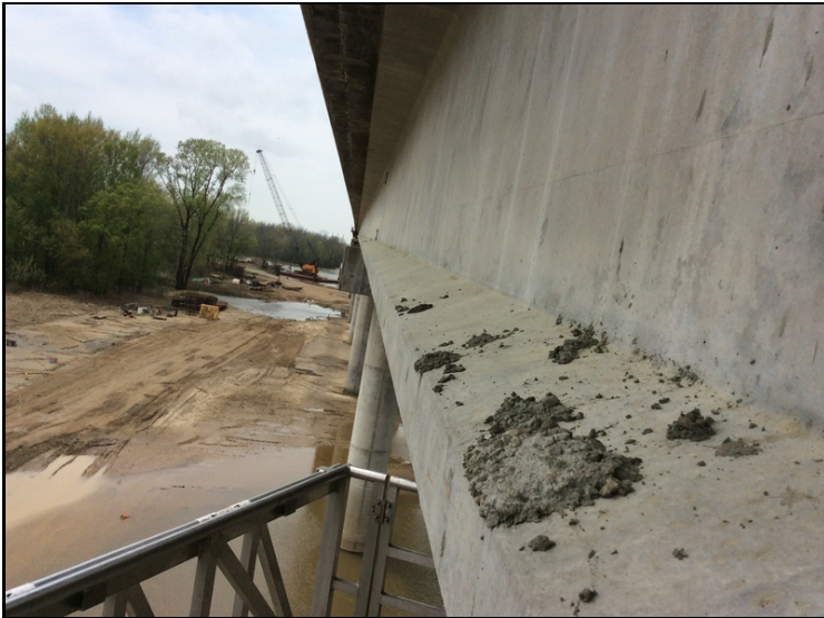
Span 88 girder 6 concrete debris on outside of Girder.
