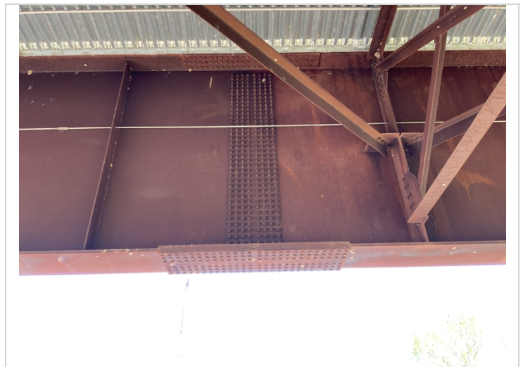
Typical splice plate connections
