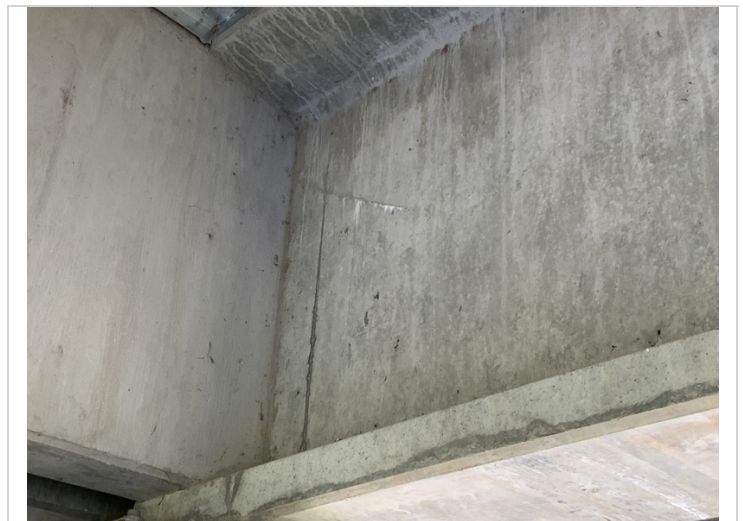
Typical diagonal cracking with efflorescence in various locations throughout the intermediate prestressed girder unit see notes for locations
