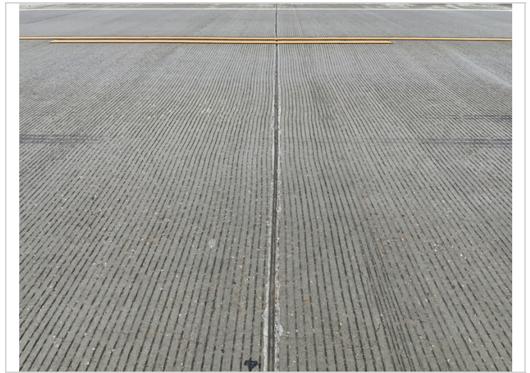
Typical saw joints
