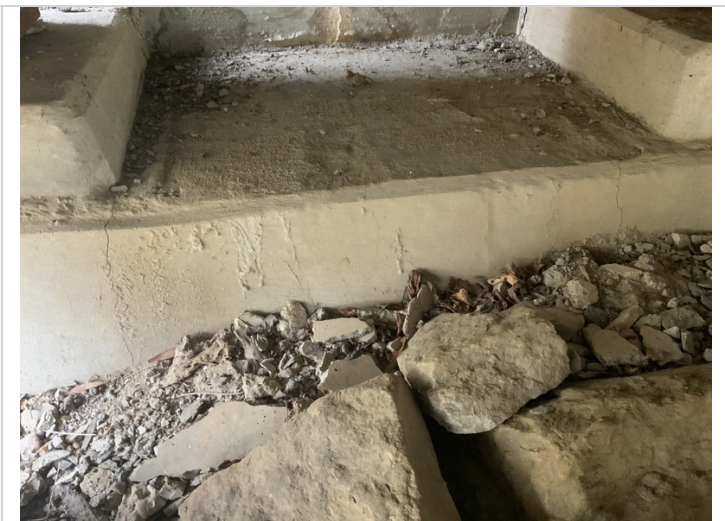
Typical cracking along the bridge seat at bent 1 South abutment
