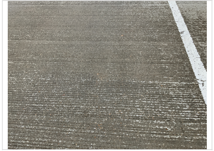
Typical map cracking
