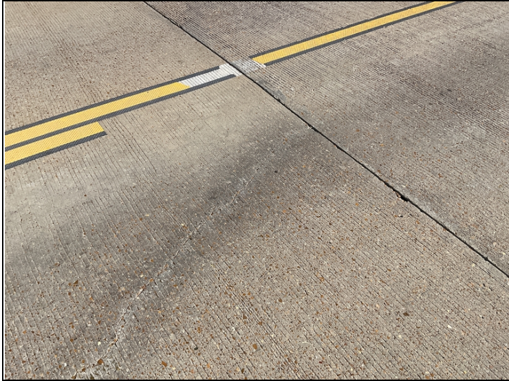
Typical approach slab crack
