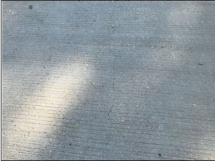
Typical longitudinal deck crack.
