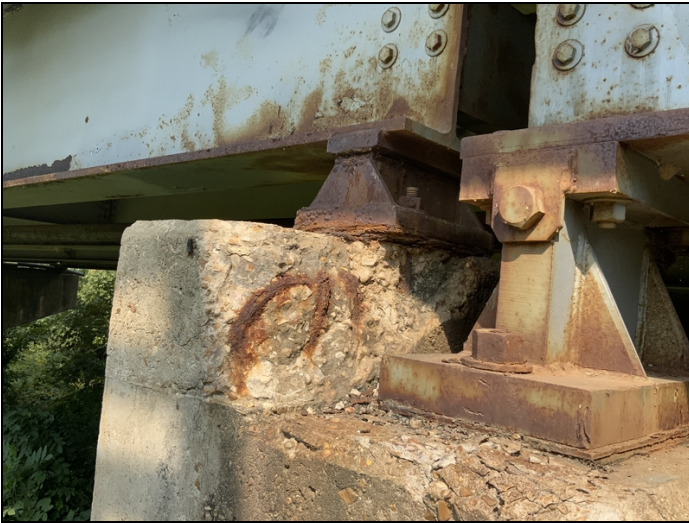
Span #5 bent #6 girder # 4 spalled under bearing with exposed rebar with 50% section loss.
