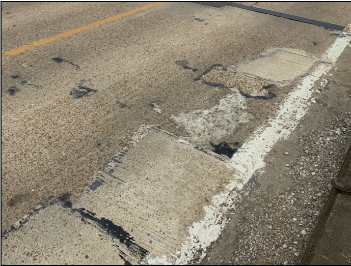
Span #13 2' x 3' shallow spall, right lane.
