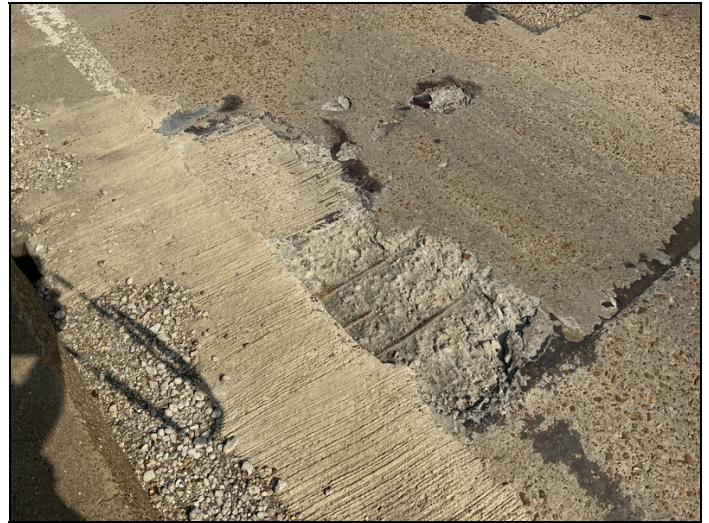
Span #9 left lane 2' x 3' spall with exposed rebar.
