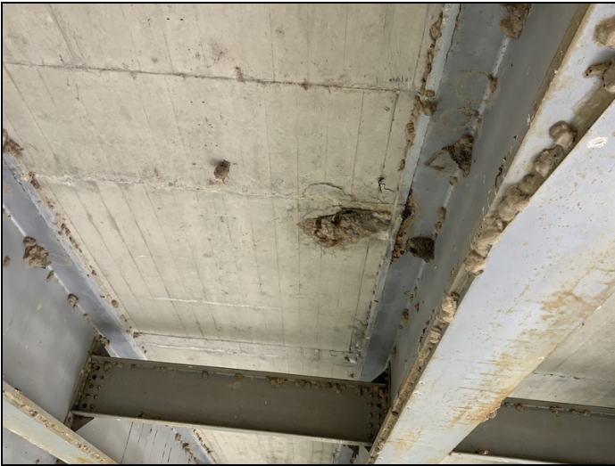
Span #8 soffit spall in bay #2.
