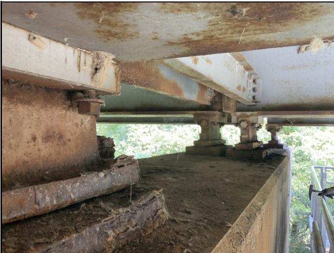
Bent #7 span #7 girders #2 and 3 each have loose bearing to girder bolt.
