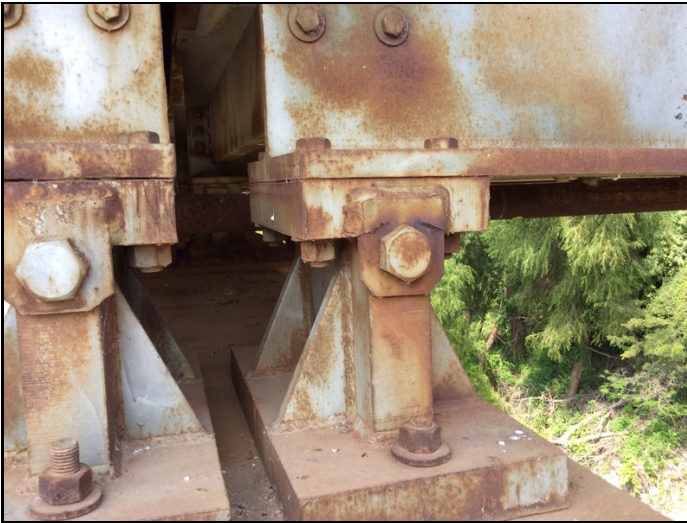
Bent 10 girder 4 right side tab for bolt from girder to bearing cracked.
