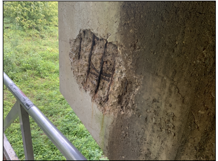
Bent #12 cap back face left side under girder #1 has two foot spall with exposed rebar with 25% section loss.
