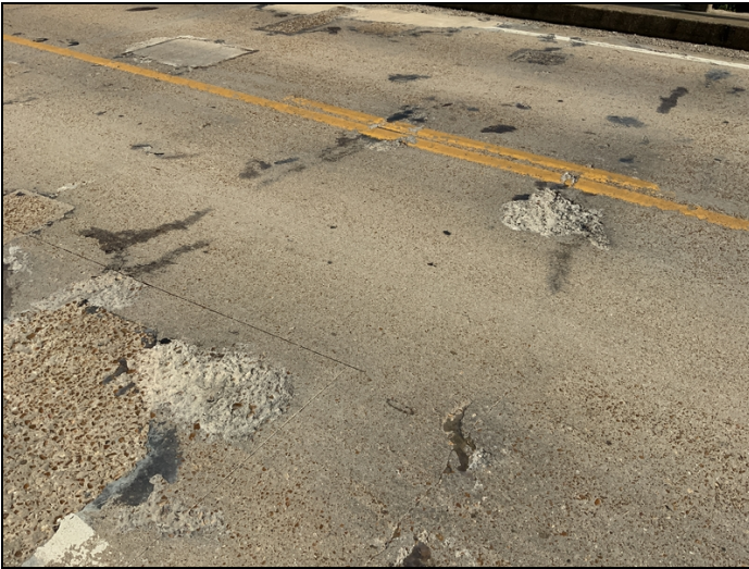
Span #6 left lane two 2 ' spalls one with exposed rebar.
