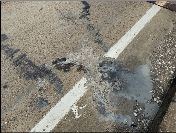
1' x 2' shallow spall right lane span #1.
