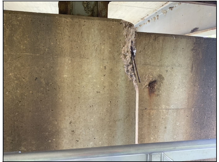
Bent #10 cap front face under girder #2 has a 1' spall with exposed rebar with 40% section loss.
