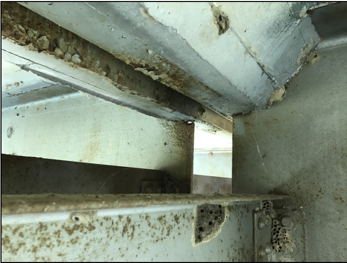
Span #12 girder #3 bent #12 one inch hole in web at haunch.
