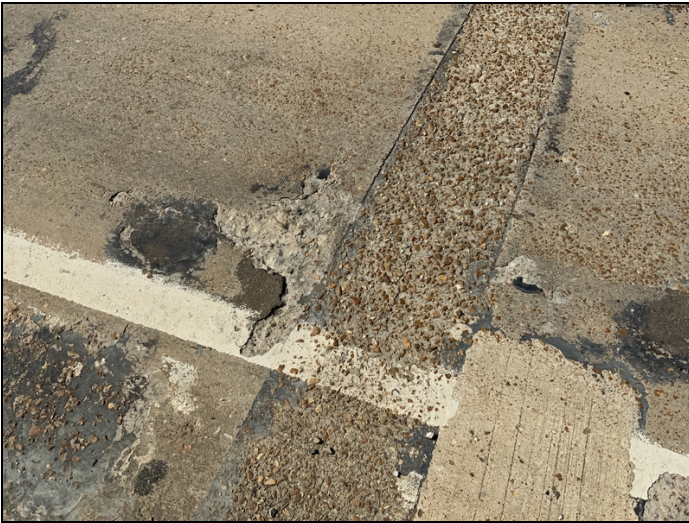
Span #3 2' spall right lane.
