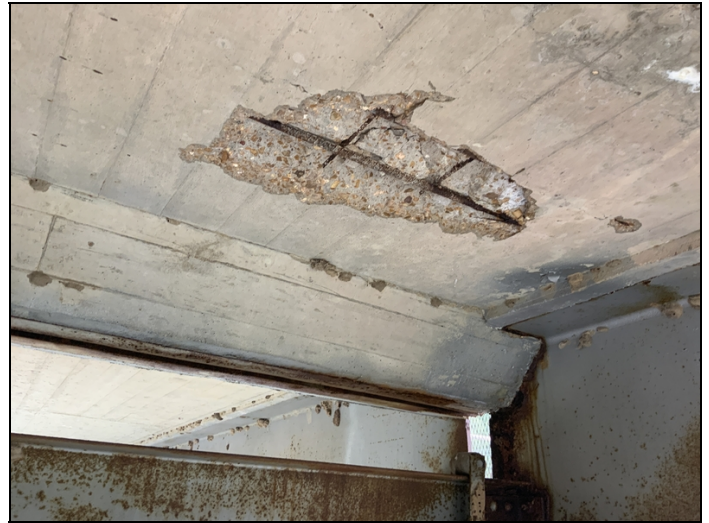
Span #8 soffit spall with exposed rebar near bent #9.
