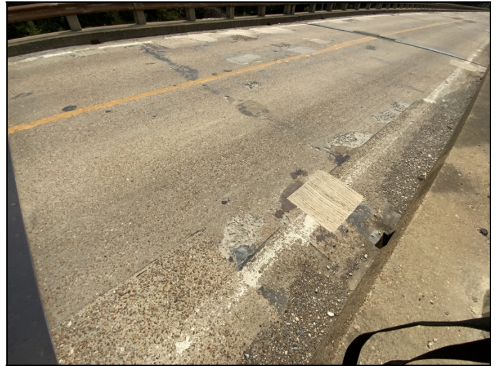
Shallow spalls in span #14 left lane.
