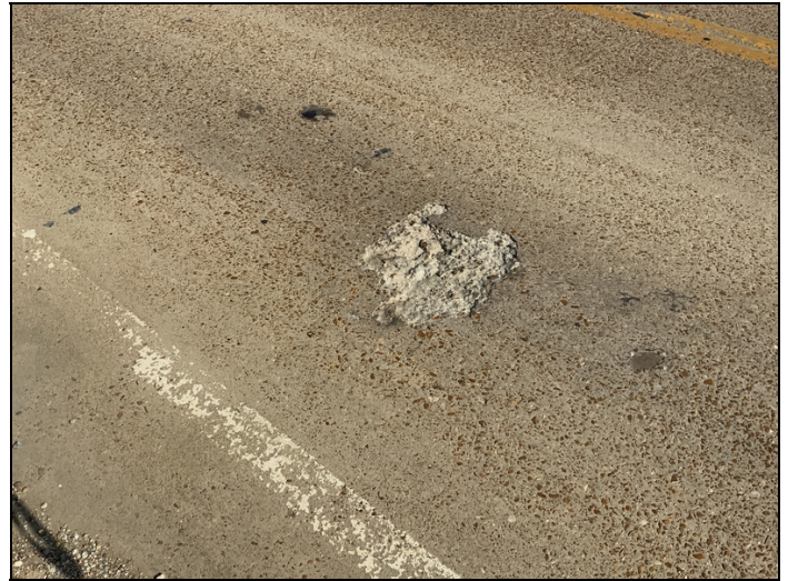
Span #10 left lane spall.
