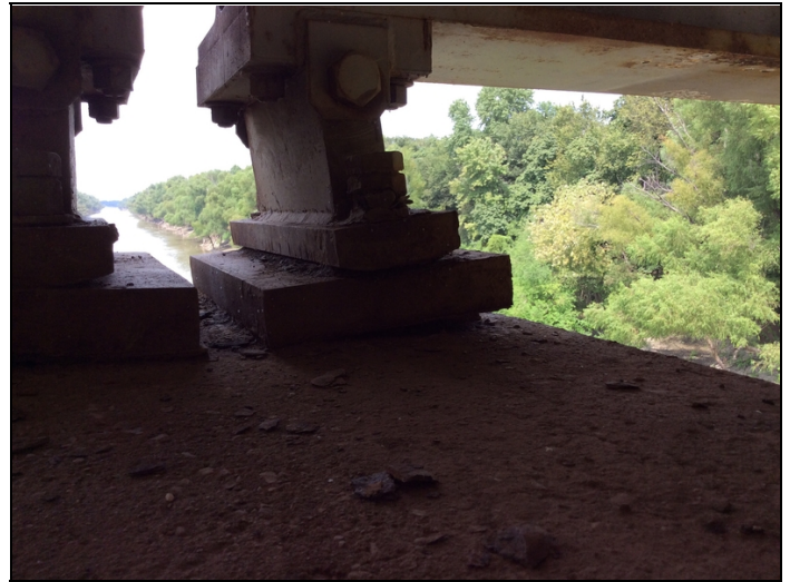
Bent 9 span 9 typical masonry plate shimmed up with pack rust.
