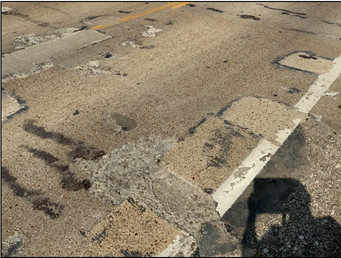
Span #5 right lane spalls
