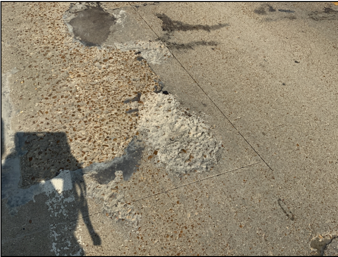
Span #6 left lane 1' x 3' spall.
