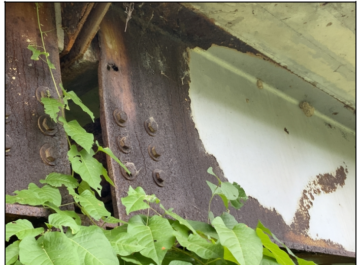
Span #16 bent #16 girder #4 has a two inch hole in web and web bowing outward at haunch.
