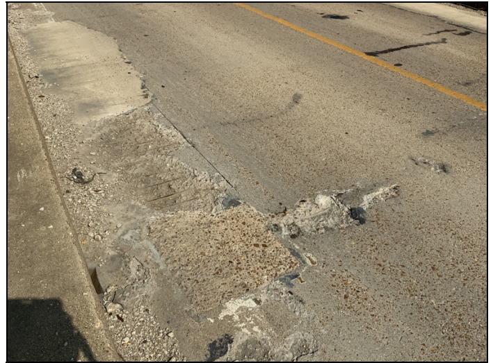
Span #6 left lane spalls with exposed rebar.
