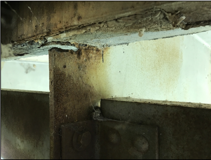
Span #13 bent #13 girder #3 at haunch has a two inch hole with a three inch crack.
