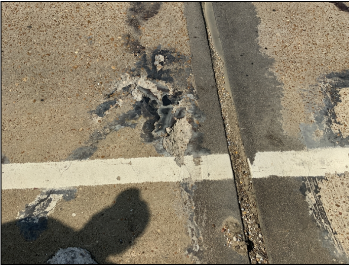
Span #4 right lane at bent #5 small spall
