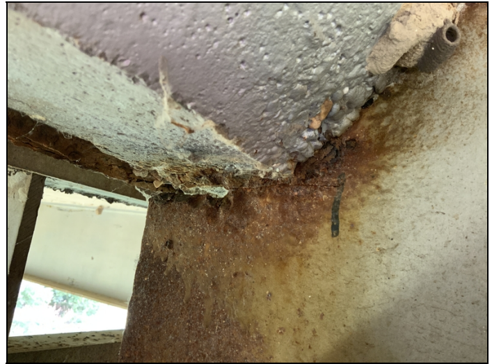
Span #13 bent #13 girder #3 at haunch has a two inch hole with a three inch crack extending out of it.
