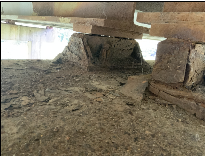
Span #14 bent #15 girder #3 floating, typical of girder #2.
