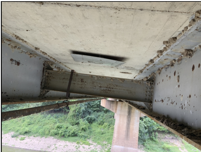
Span #8 bay #3 has form left in place near bent #9.
