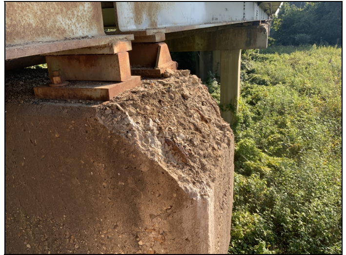
Bent #3 cap right end spalled at top with exposed rebar with 20% section loss.
