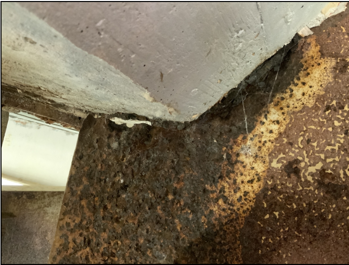
Span #15 bent #15 girder #3 has a three inch long hole with a one and a half inch crack extending out of it at haunch.
