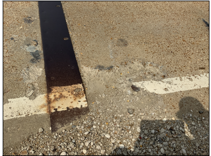
Span #13 bent #13 right lane has 2" x 2" shallow spall.
