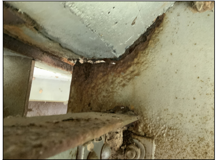
Span #3 girder #3 at bent #4 has a six inch long hole in web at haunch.
