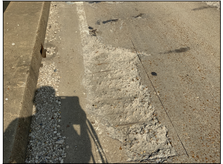
Span #6 left lane 2' x 5' spall with exposed rebar.
