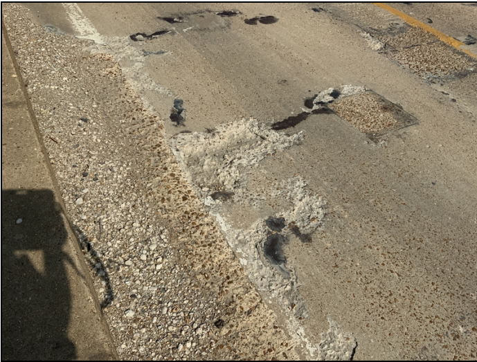
Span #9 left lane 3' x 2' spall with exposed rebar.
