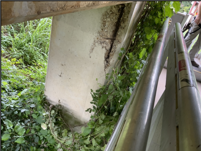
Bent #16 right column left side has 2' spall with exposed rebar with 20% section loss.
