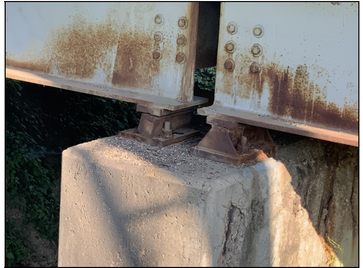
Bent #2 bearings.
