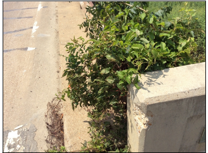
Abutment 2 left side vegetation growing onTo bridge.
