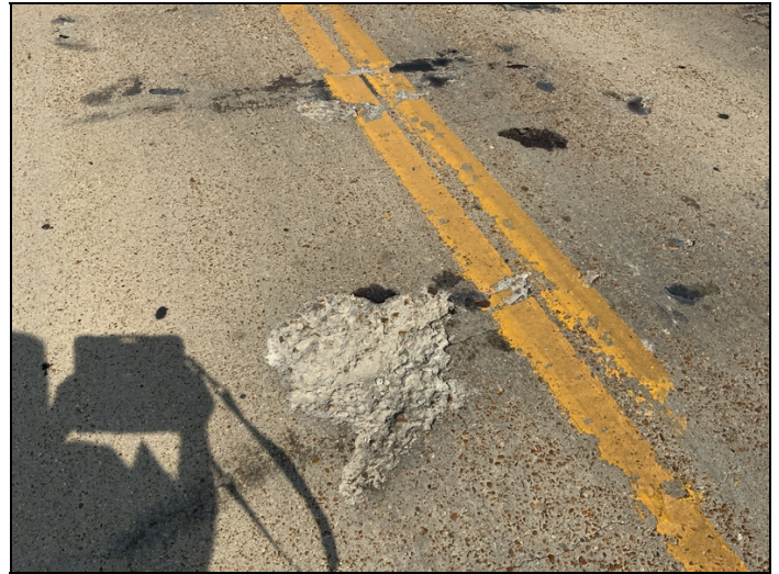
Span #6 left lane spalls at center line.
