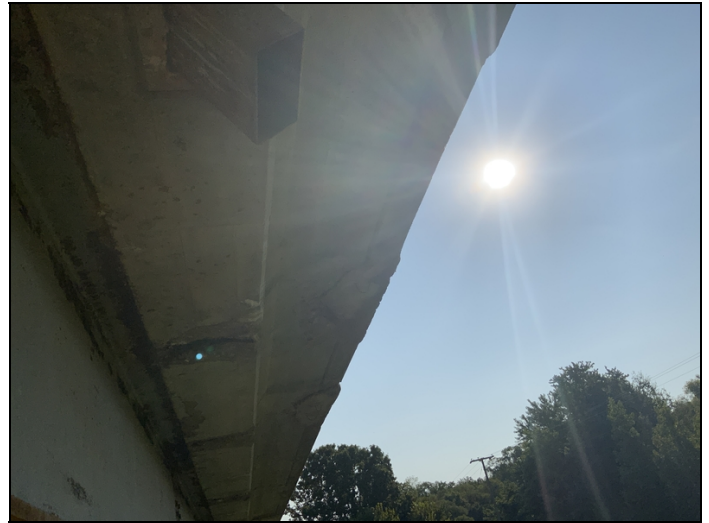
Span #1 right soffit overhang has four one foot spalls with exposed rebar with 20% section loss and four repaired areas at rail posts.
