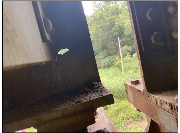
Span #12 bent #12 girder #4 has 2' hole in web at diaphragm connection.
