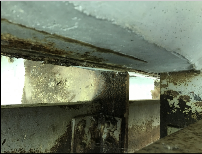
Span #15 bent #15 girder #2 has a one inch long hole at haunch.
