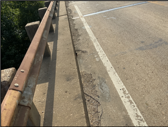
Dirt and debris in gutters.
