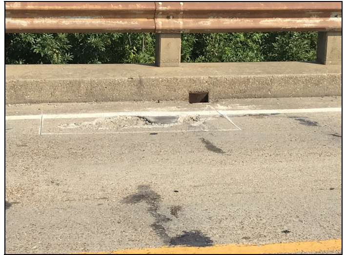
Deck span #6 left shoulder near bent #6 has a three foot spall with rebar exposed.
