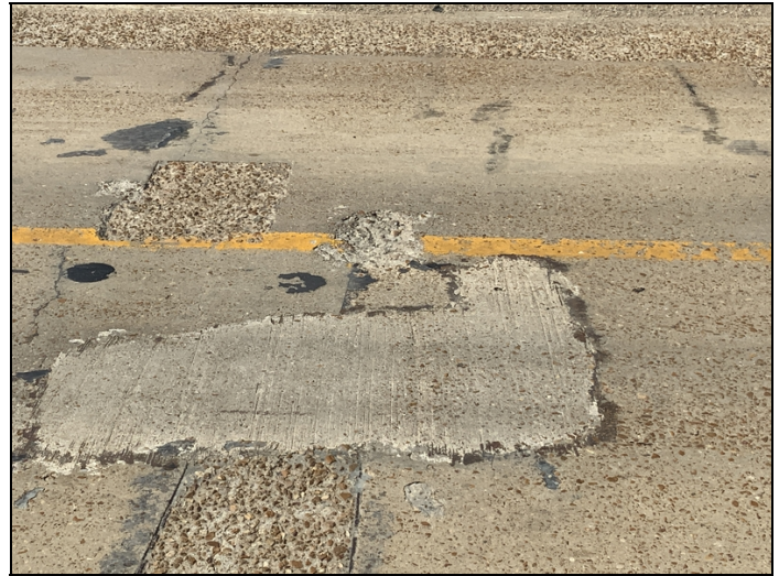
Span #3 1' x 2' spall at center line.
