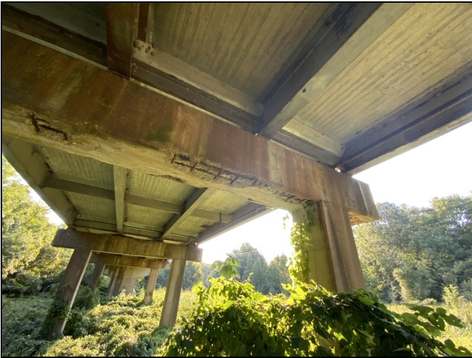
Bent #2 cap bottom face has 3' of delaminations one 2' spall, a 1' x 4' spall, a 1' x 2' spall, a 1', a 3' long spall and a 2' x 2' spall with exposed rebar with 20% section loss.
