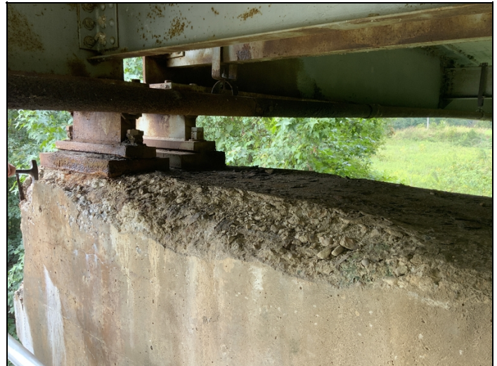
Bent #7 cap ahead face spalled at top for six feet under girder #4, with two foot delamination under girder #4.
