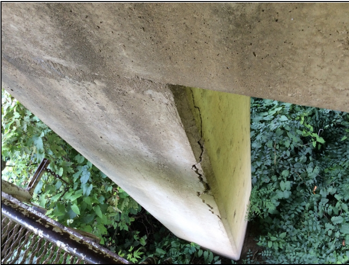
Bent 14 left column cracked.
