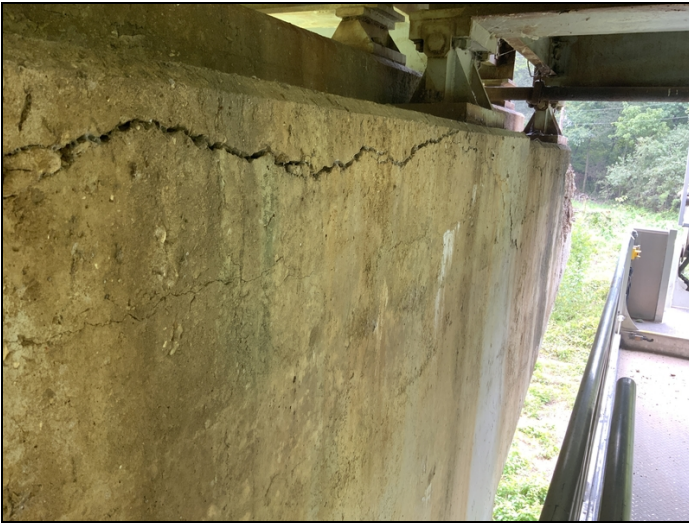
Cracking bent #12 cap back face.
