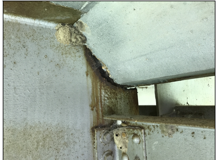
Span #2 girder #3 at bent #3 has a 2" hole corroded in web at haunch.
