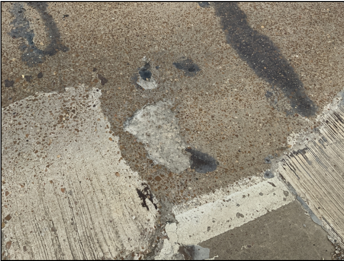
Span #16 right lane has 1' shallow spall with no exposed rebar.
