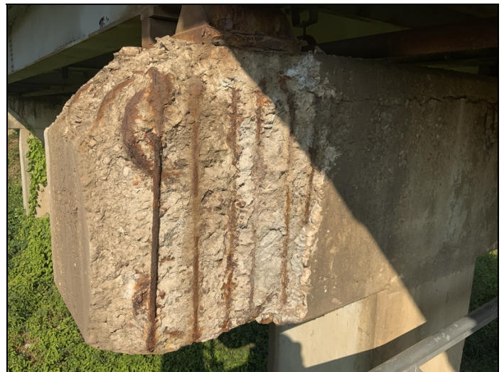
Bent #3 cap front face right corner has 2'long full height spall with exposed rebar with 20% section loss extending to the edge of span #3 girder #4 bearing.
