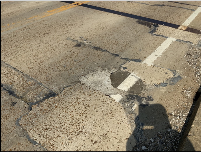
Span #3 deck 2' spall right lane.
