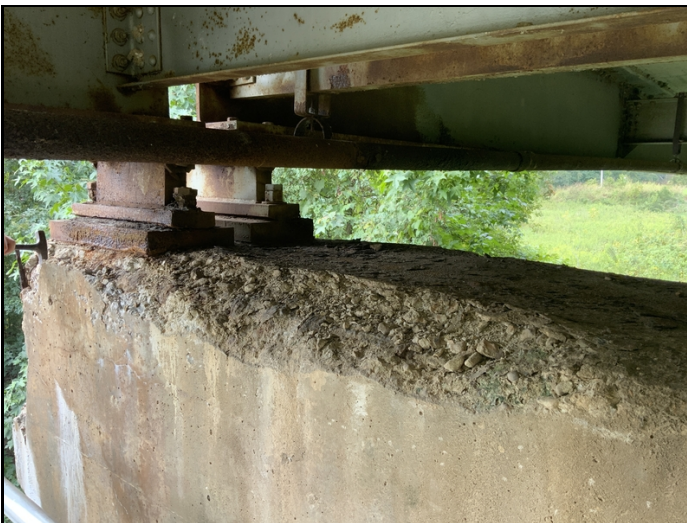
Bent #7 cap ahead face spalled at top for six feet under girder #4, with two foot delamination under girder #4.
