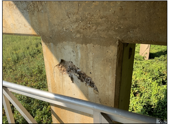
Bent #4 right column left and right sides have vertical cracks, ahead face has two foot delamination and spall with no exposed rebar.
