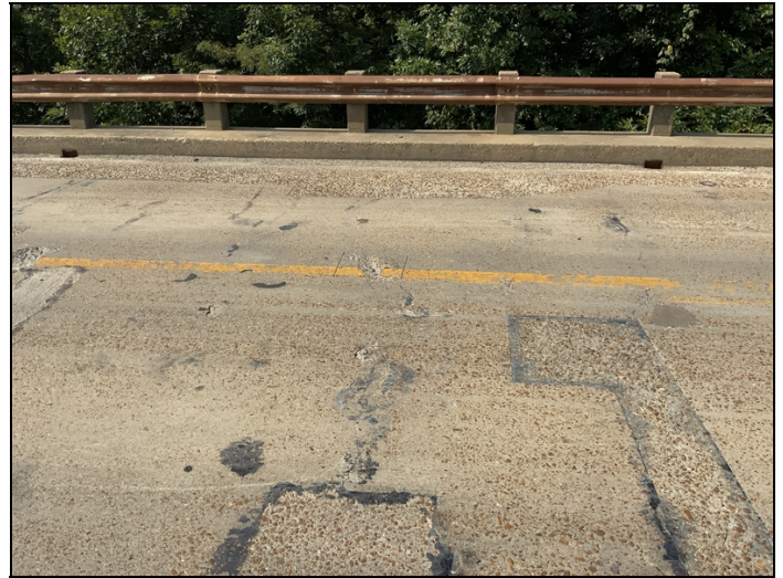
Span #3 center line 1' spall.
