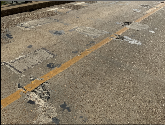
Span #10 spalls at center line.
