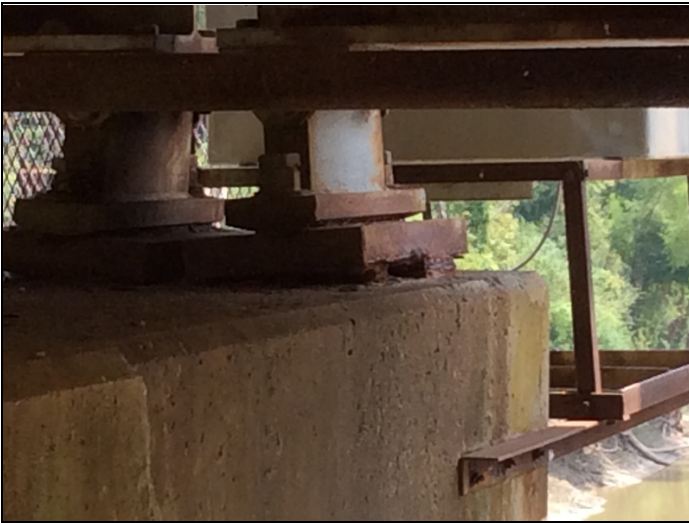
Bent 9 span 8 masonry plate shimmed by pack rust
