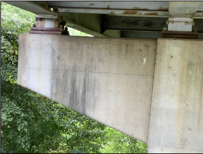
Bent #11 cap back face left side cracked horizontally.
