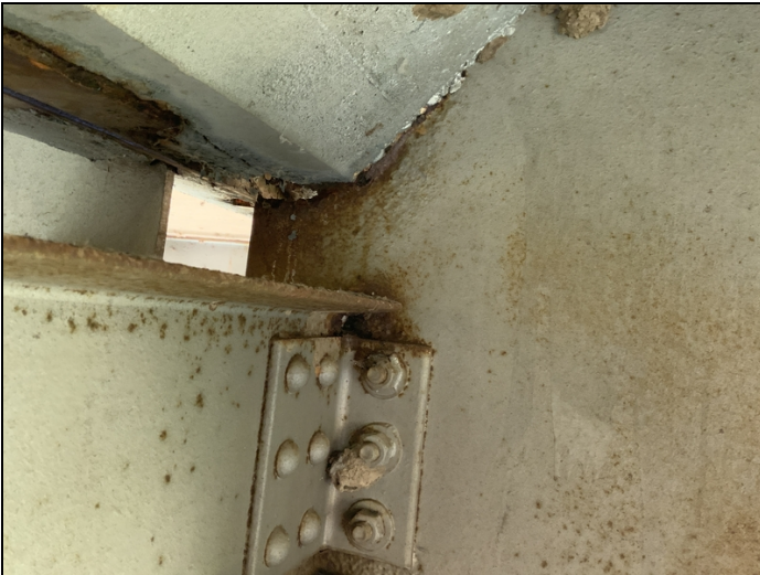
Span #2 girder #3 at bent #3 has a 2" long hole corroded in web at haunch.
