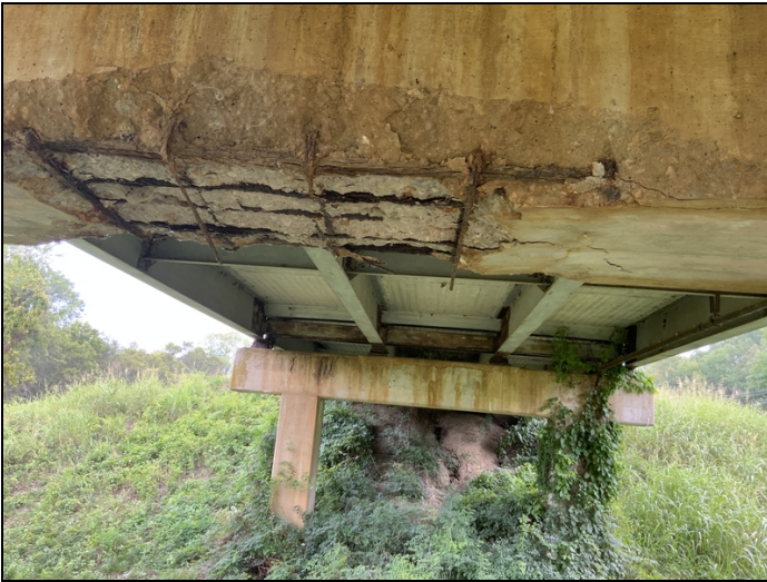
Bent #15 cap bottom face.
