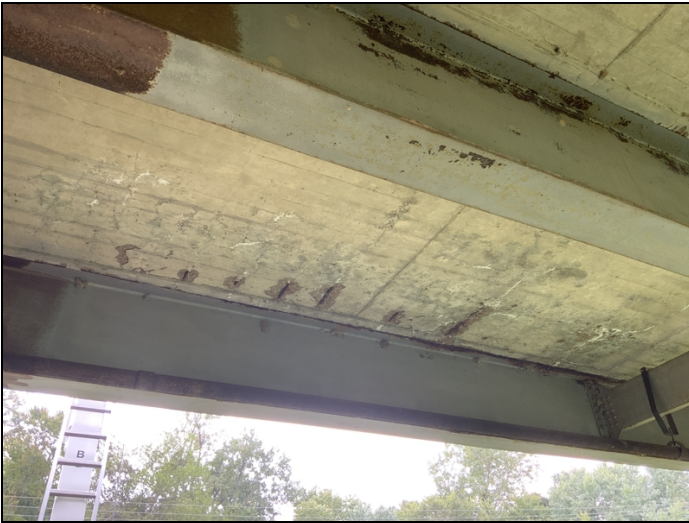
Span #13 soffit bay #3 has five 1' spalls with exposed rebar with 5% section loss.
