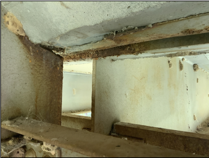
Span #12 girder #2 bent #12 one inch hole in web at haunch.
