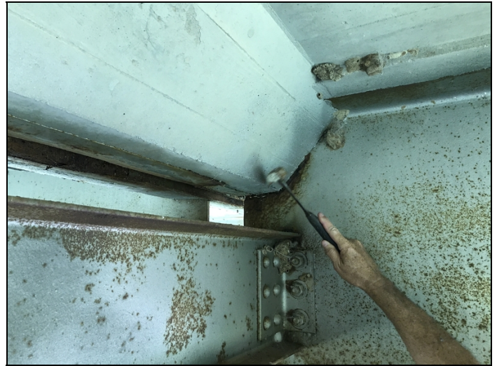
Span #3 girder #3 at bent #4 has a six inch long hole at haunch.
