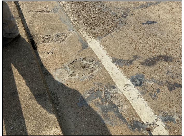
Spalls in span #2 right gutter.
