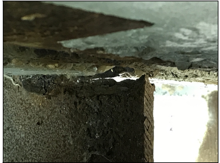
Span #16 bent #16 girder #3 has one inch hole with a one inch crack extending out of it at haunch.
