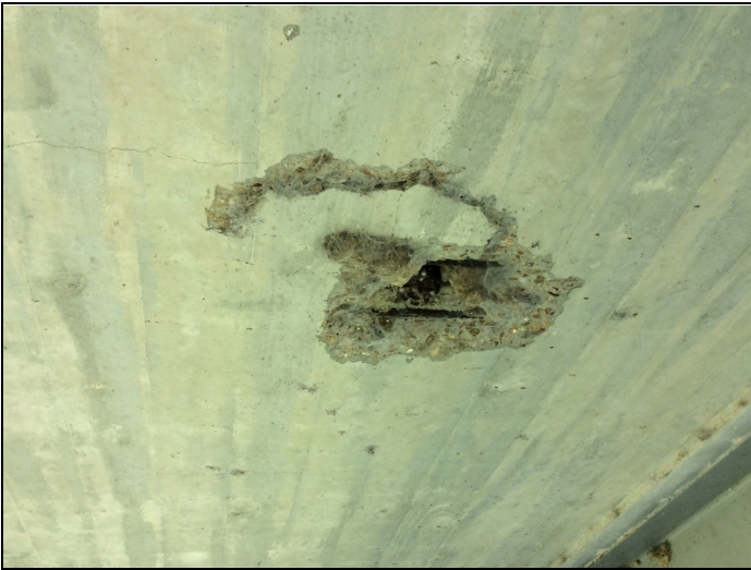
Span 3 bay 1 spall in soffit.
