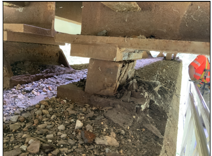
Span #14 girder #3 bearing is twisted under girder.
