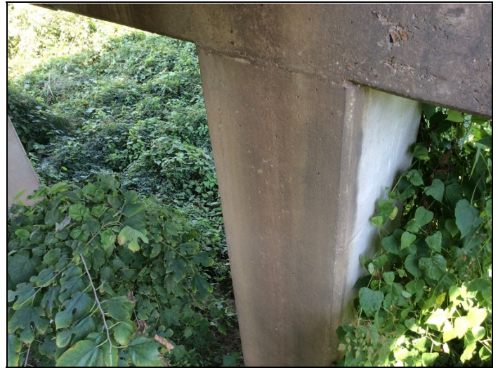
Bent 2 back face right column cracked.
