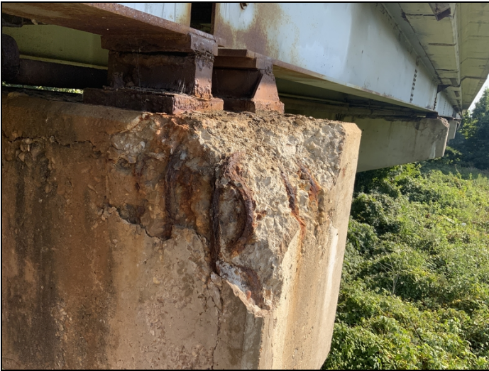
Bent #4 cap right end top right corner, back face spalled with exposed rebar with 25% section loss.
