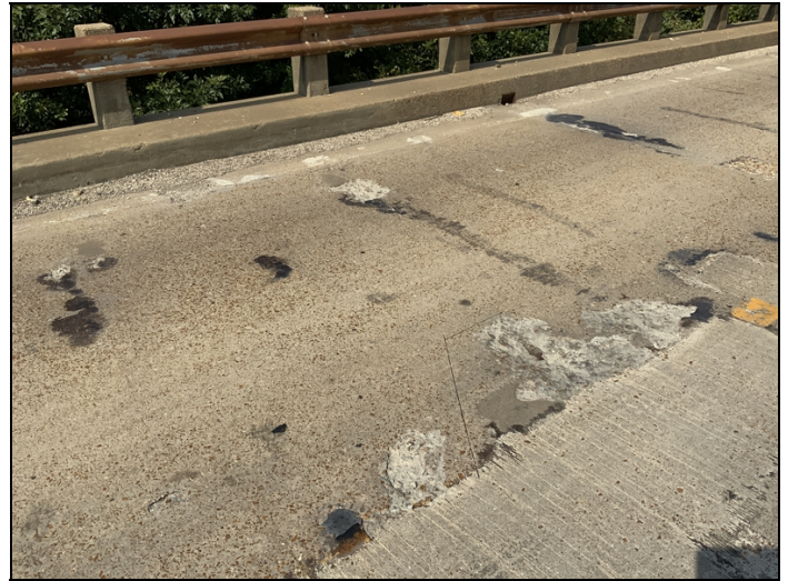
Span #5 left lane spalls.
