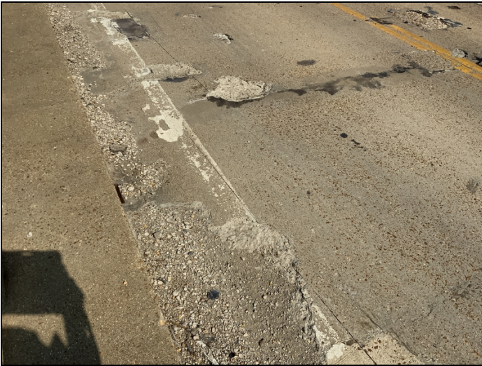
Span #6 left lane spalls with exposed rebar.
