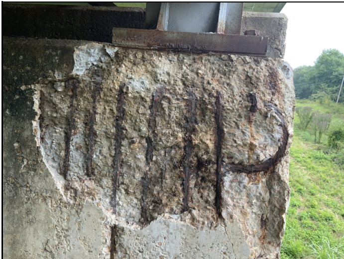
Bent #12 cap back face right side under girder #4 bearing has three foot spall with exposed rebar with 25% section loss.
