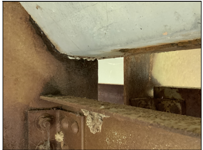
Span #14 bent #14 girder #3 has a four inch long hole at haunch.
