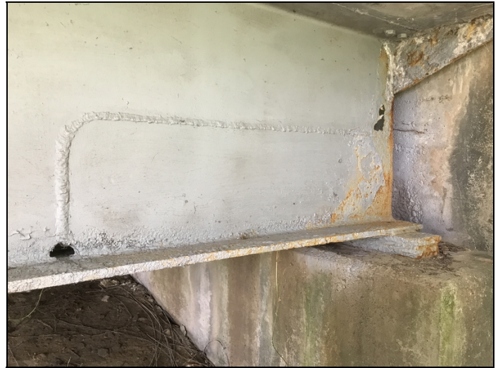
Span #1 girder #1 at bent #1 has a one and a half foot tall by three foot long t-splice at girder end. With area in web above the T-splice has a three inch hole.
