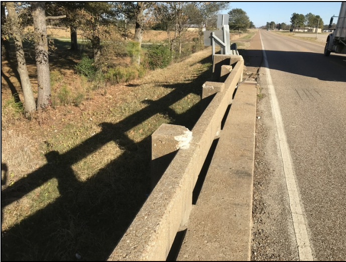
Span #3 left rail posts #2,3,4 all have collision damage on top with spalls posts #4 with rebar exposed.
