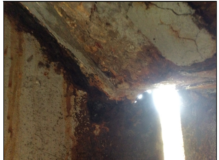
Bent 2 span 2 girder 4 has a 2" long hole at haunch.
