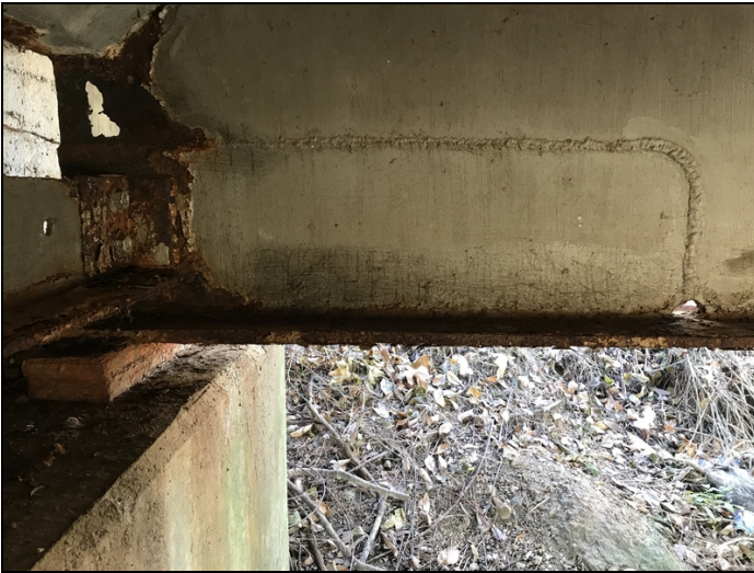
Span #1 girder #1 at bent #1 has a one and a half foot tall by three foot long t-splice at girder end. Area above T-splice has 3" hole in web.
