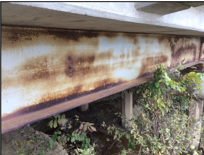
Typical paint condition
