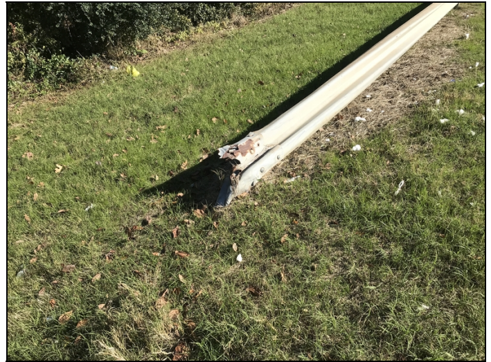
Abutment #1 left approach rail end
