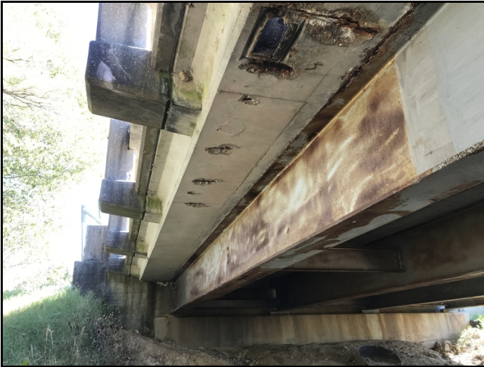
Spalls in soffit overhang with exposed rebar
