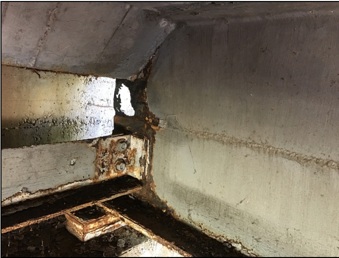
Abutment #1 girder #1, 3" x 6" hole in web at haunch
