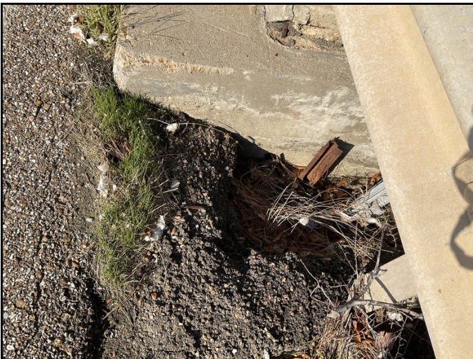
Abutment #2 left approach shoulder eroded
