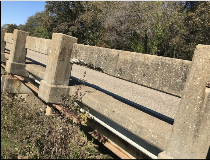
Span #2 right rail spalled
