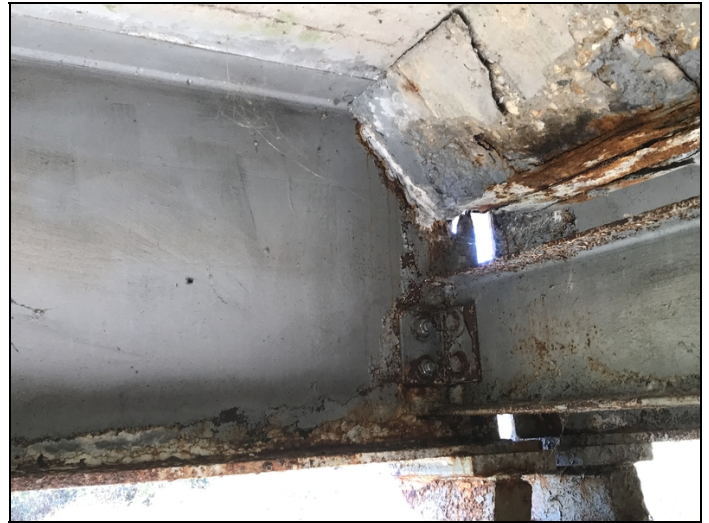
Span #2 bent #2 girder #4 hole in web at haunch
