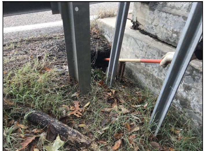
Erosion under approach roadway abutment #2 left side
