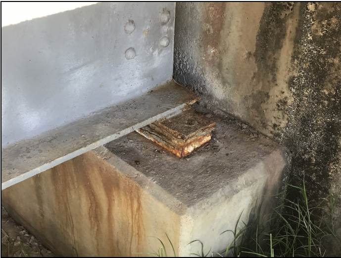
Typical fixed abutment bearing with broken anchor bolt
