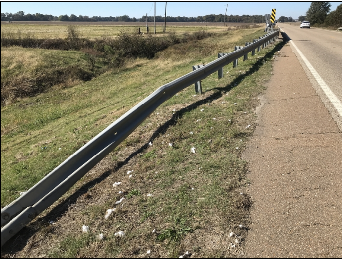
Abutment #2 right approach rail has collision damage fifteen feet from end
