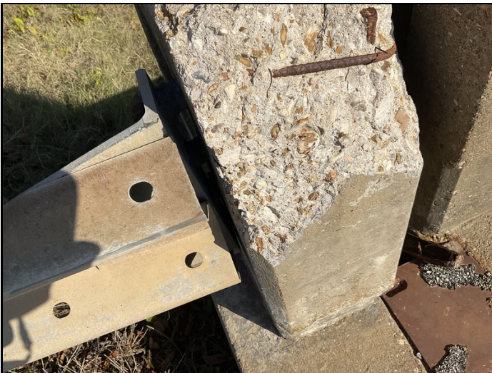
Abutment #1 left approach rail beginning to separate from monument post
