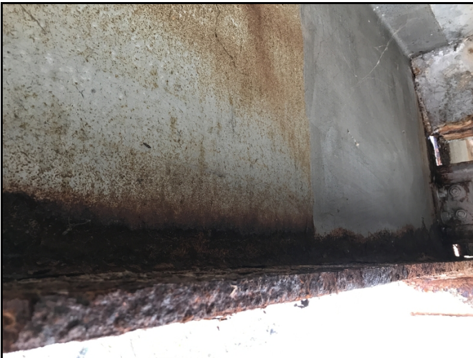
Span #2 bent #2 girder #4 has a 2" long hole at haunch, with up to 50% section loss around diaphragm area in web, and has 5' long area of corrosion with laminations and section loss up to 65% in web near bottom flange at end of girder.
