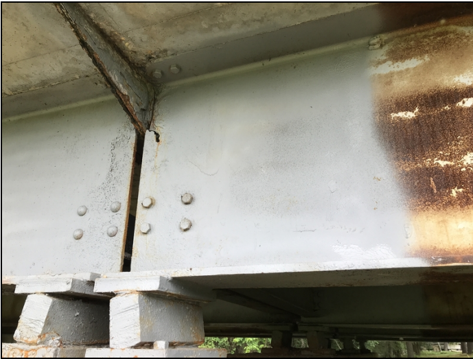
Span #2 bent #2 girder #4 has a two inch long hole at haunch, with up to 50% section loss around diaphragm area in web, and has a five foot long area of corrosion with laminations and section loss up to 65% in web near bottom flange at end of girder.
