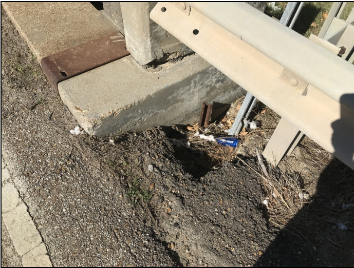
Erosion at abutment #2 left side
