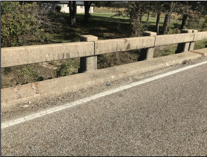
Dirt and debris in gutter
