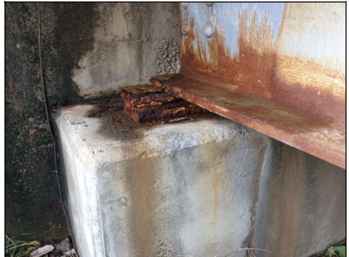
Typical fixed bearing.
