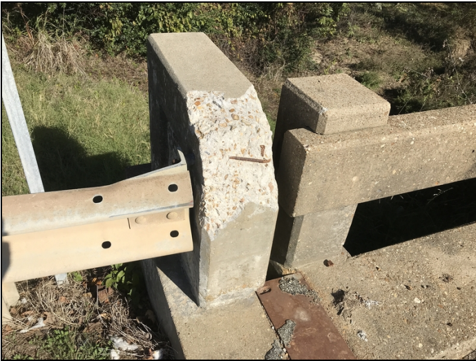
Abutment #1 left monument post spalled with exposed rebar no section loss
