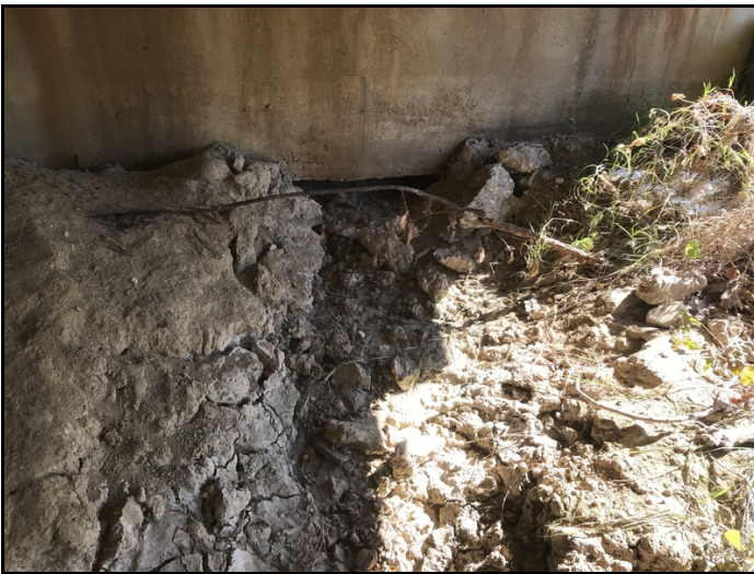
Abutment #2 erosion, right side
