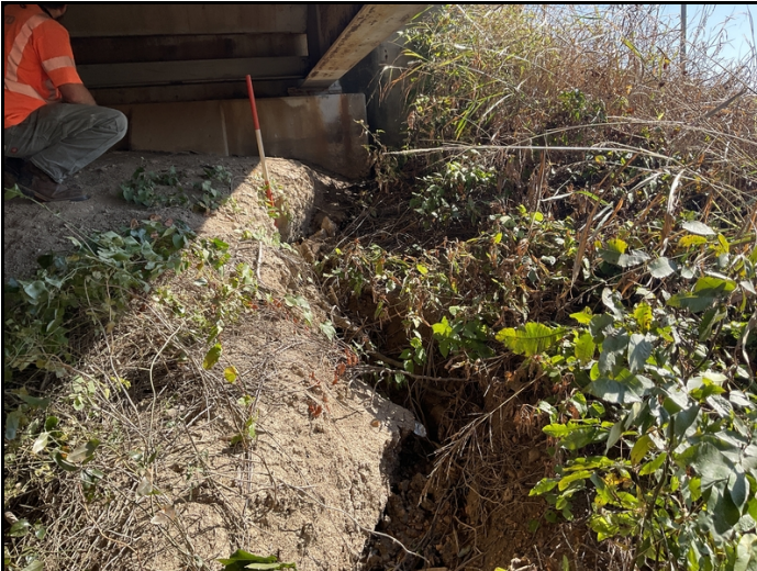
Abutment #2 slope right side has erosion vein up to two-foot deep running down slope.
