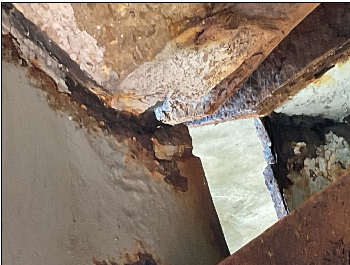
Span #3 bent #3 girder #4 has 1 1/2" hole at haunch.
