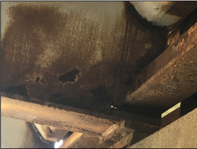
Span #2 bent #2 girder #3 has a three inch hole in web at diaphragm connection.
