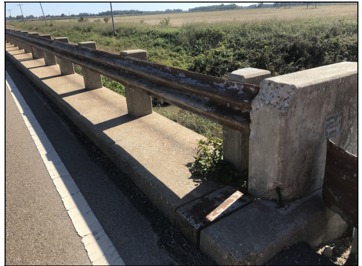
Abutment #1 right side post damage
