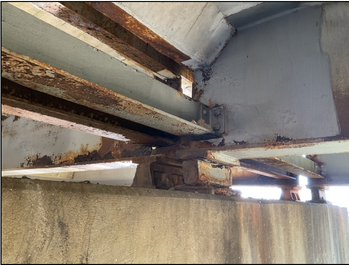
Span #2 bent #2 girder #3 has a four inch hole in web at diaphragm connection and a one inch hole in web at haunch, bottom flange and lower web corroded with laminations for first three feet.
