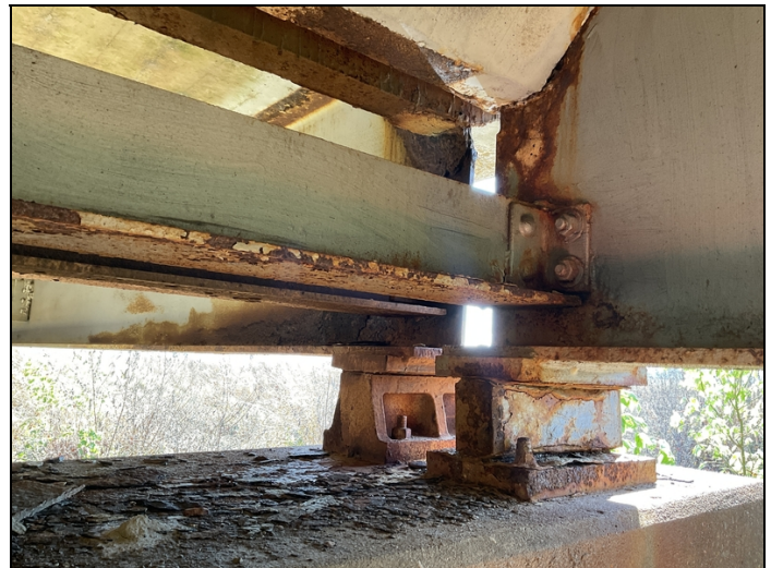
Span #2 bent #2 girder #4 corroded at haunch with up to 70% section loss, first two feet of bottom flange and lower web corroded with laminations.
