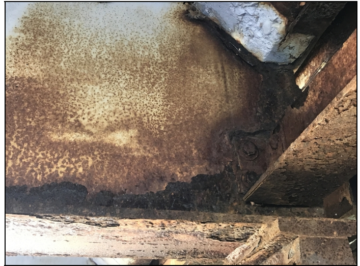
Span #2 bent #2 girder #2 has a two inch hole in web at diaphragm , and a five inch hole at haunch.
