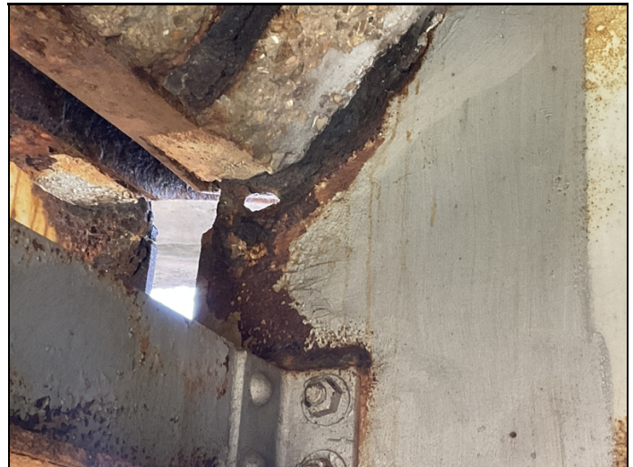
Span #3 bent #3 girder #1 has 1 1/2" hole rusted through at haunch
