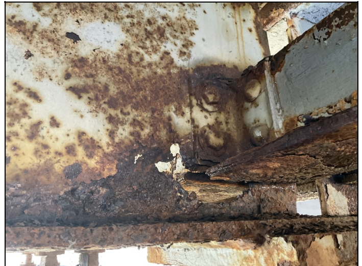
Span #3 bent #3 girder #2 web at diaphragm connection
