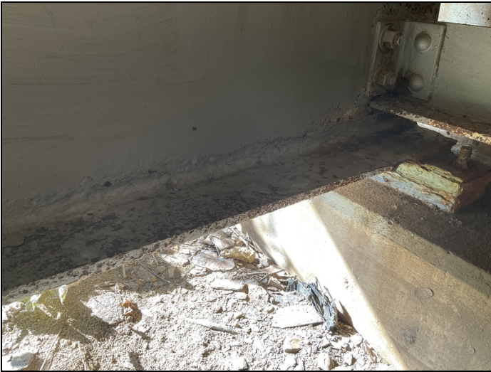
Span #1 abutment 1 girder #4 has section loss on lower flange and migrating into web first 2' 50% section loss.
