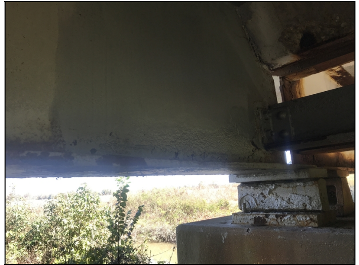
Span #1 , girder #1 at bent #2 bottom flange has 35% section loss for 2'.
