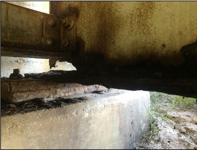
Span #1 abutment #1 girder #1 bottom flange section loss.
