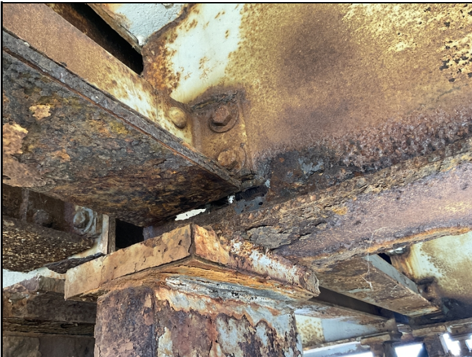
Span #3 bent #3 girder #3 web at diaphragm connection
