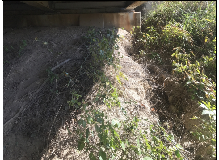
Abutment #2 slope right side has erosion vein up to one foot deep running down slope.
