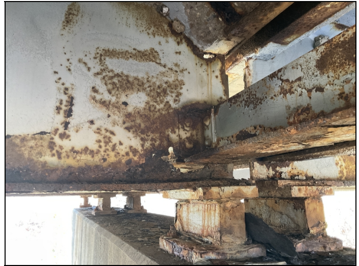
Span #3 bent #3 girder #2 has a eight inch hole in web at diaphragm and a one and a half inch hole at expansion dam haunch.
