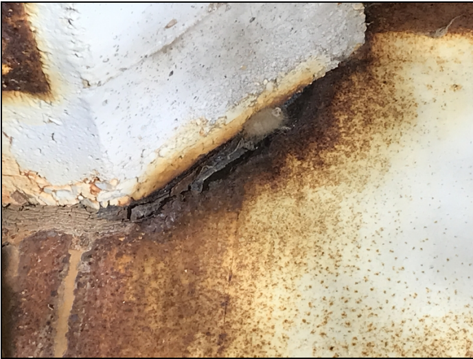
Span #2 bent #2 girder #2 hole at haunch
