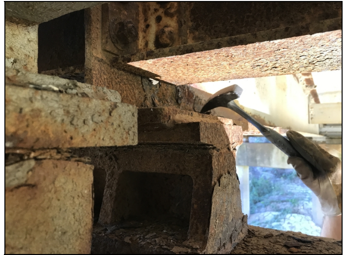
Span #2 bent #2 girder #2 hole at diaphragm connection
