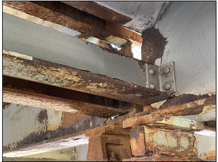
Span #2 bent #2 girder #2 has a three inch hole in web at diaphragm , and a five inch hole at haunch, bottom flange and lower web corroded with laminations for four feet.
