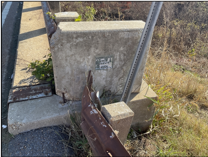
Abutment #1 right monument post spalled with exposed rebar
