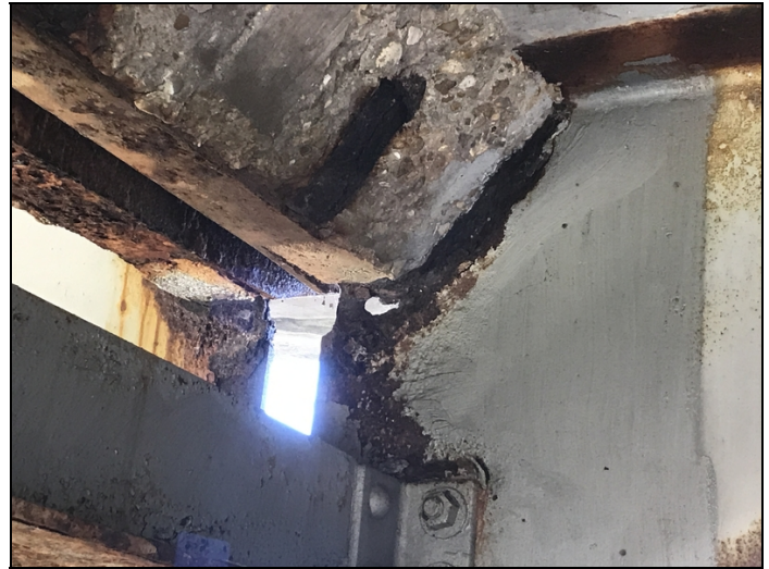
Span #3 bent #3 girder #4 has 1 1/2" hole at haunch.
