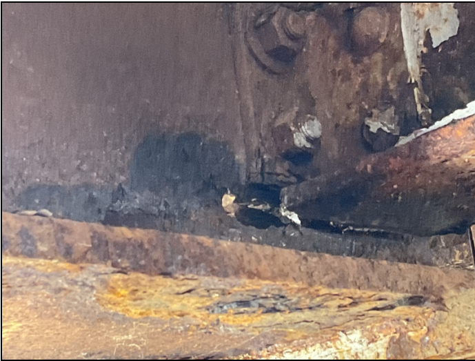
Span #3 bent #3 girder #3 has a eight inch hole in web at diaphragm connection.
