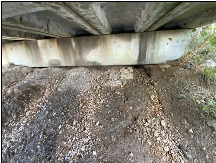
Erosion at abutment #1 cap.
