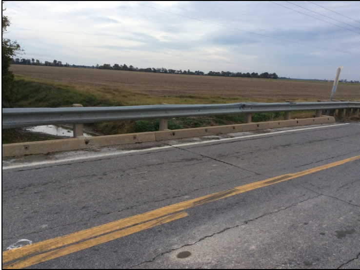
Bridge rail on left side has collision damage full length of bridge.
