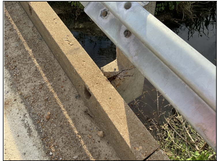
Span #2 right side first rail post spalled.
