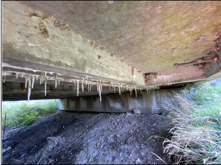
Span #3 unit #7 left leg has map cracking full length with moderate to heavy efflorescence.
