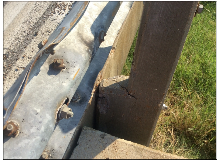
Broken rail post and rail.
