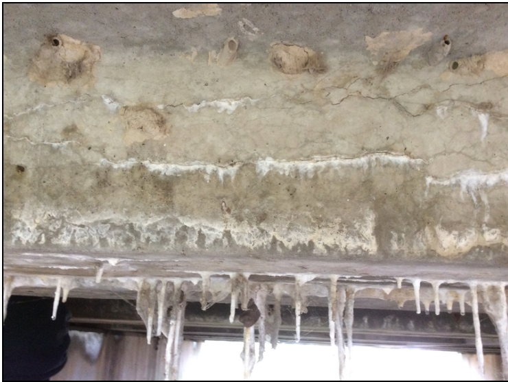
Span three girder seven right and left legs have longitudinal cracks
