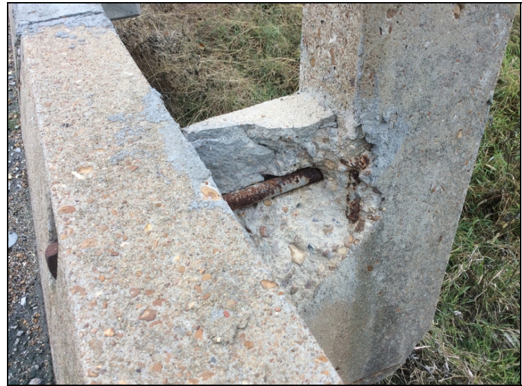
Typical spalled rail post .
