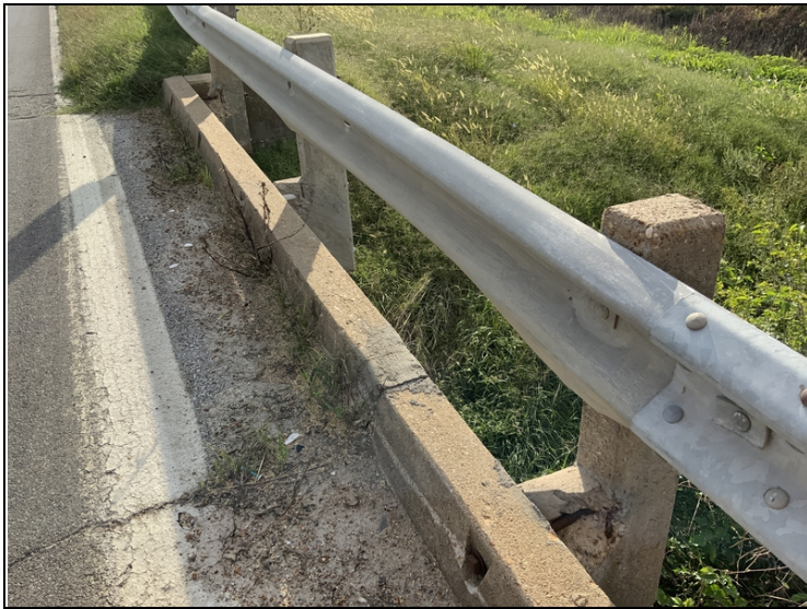
Span #2 right side second rail post spalled, span #3 right side, both rail posts spalled,
