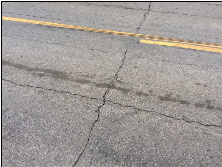
Typical cracks in asphalt on deck.
