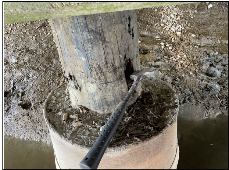
Bent #2 pile #3 has outer shell decay with up to 15% section loss above splice.
