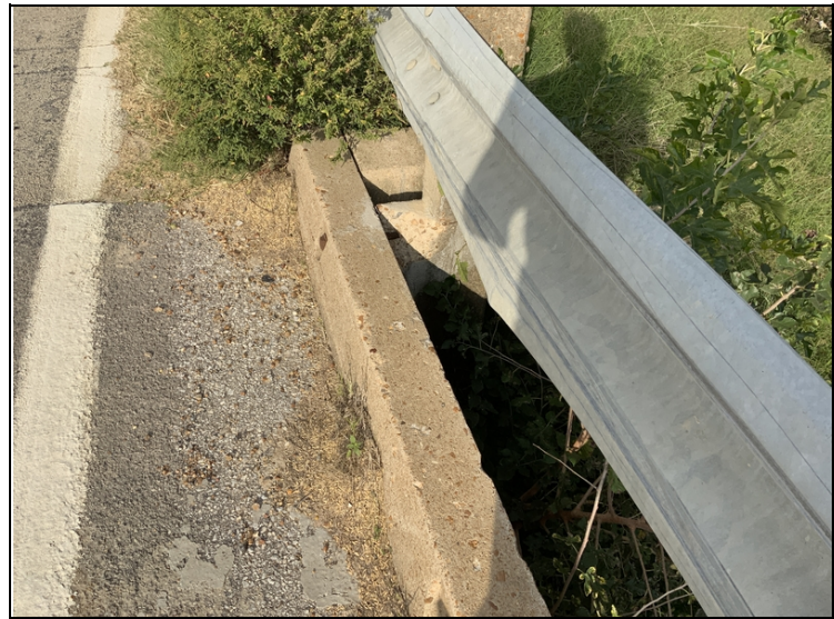
Span #1 left side first rail post spalled
