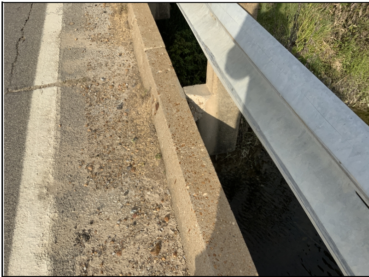
Span #2 left side first rail post spalled.
