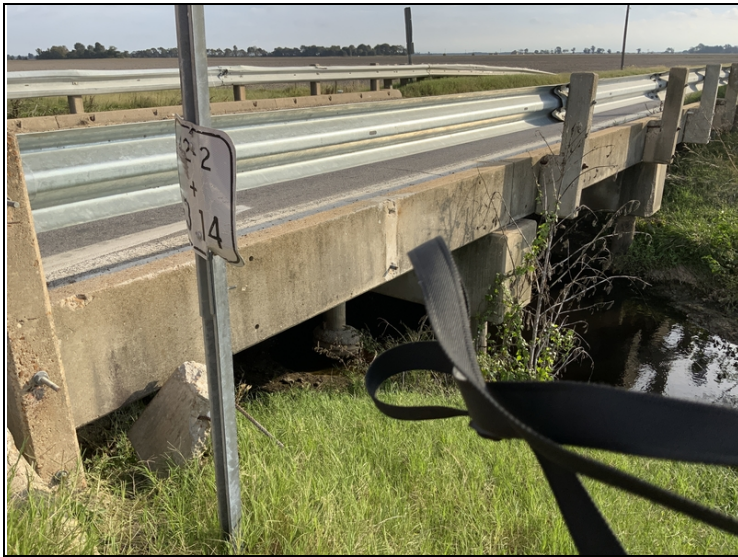
Second rail post, span #1 right side missing
