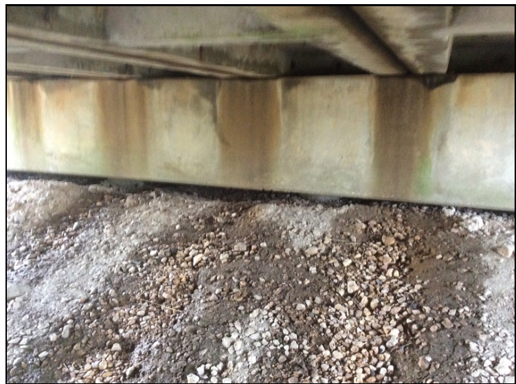
Abutment two cap is undermined.
