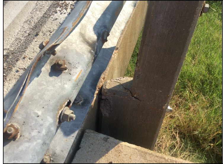
Broken rail post and rail.
