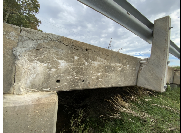
Span #3 unit #7 right leg has map cracking for 6' with moderate efflorescence.
