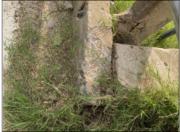
Span #1 right curb spalled at abutment #1 for one foot with exposed rebar.
