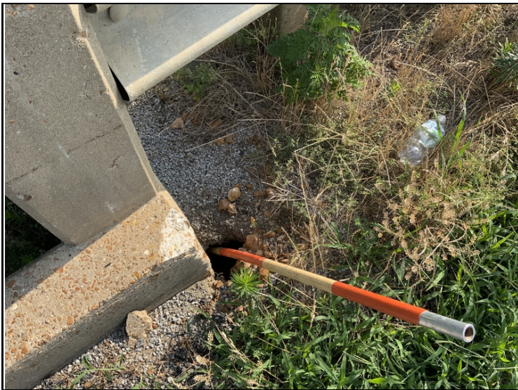
Hole in abutment #2 left approach shoulder at bridge end.
