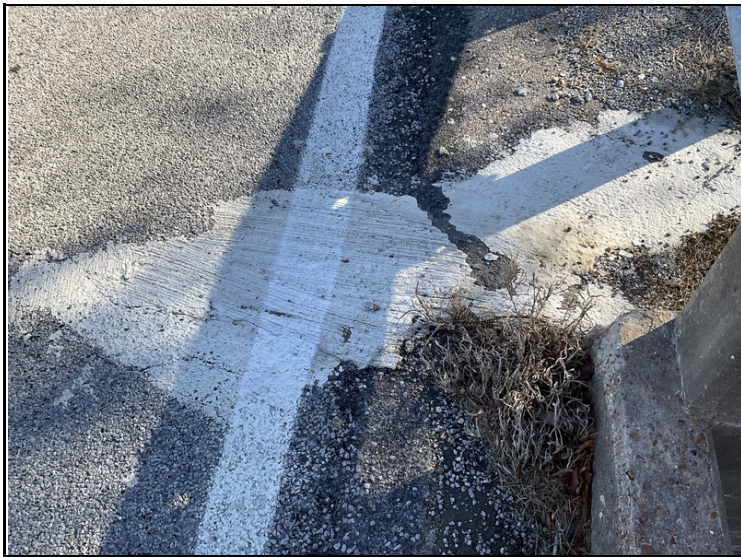
Abutment #2 hole in roadway repaired.
