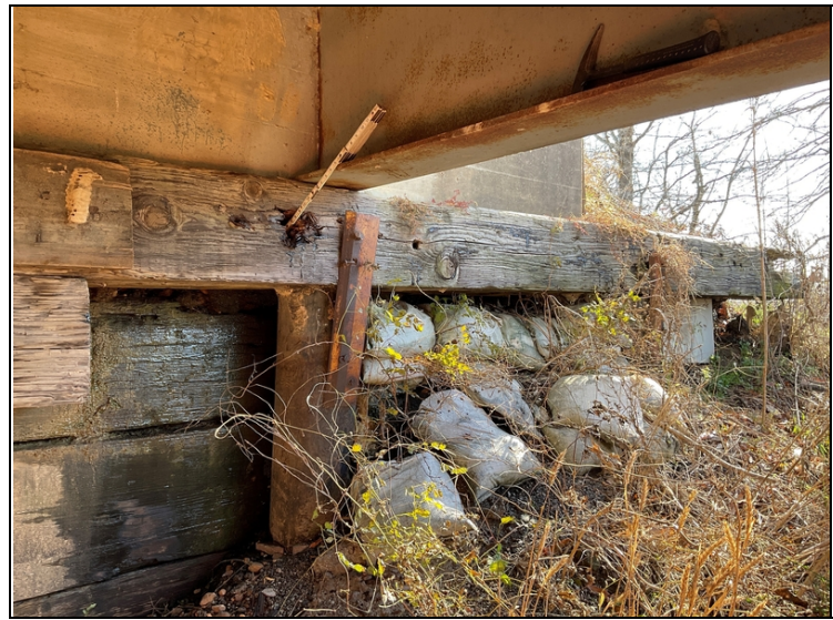
Abutment #2 pile #9 decayed non-functional
