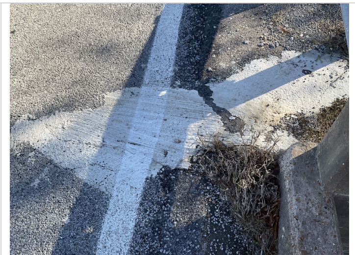
Abutment #2 hole in roadway repaired.
