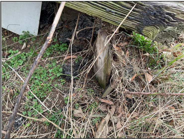
Abutment #2 pile #9 decayed non-functional
