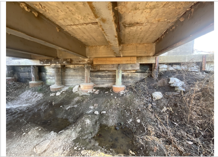
Abutment #2 cap repaired
