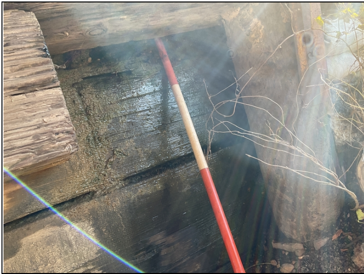
Small void behind abutment #2 back wall by pile #5 causing hole in abutment #2 approach roadway right side at bridge end.
