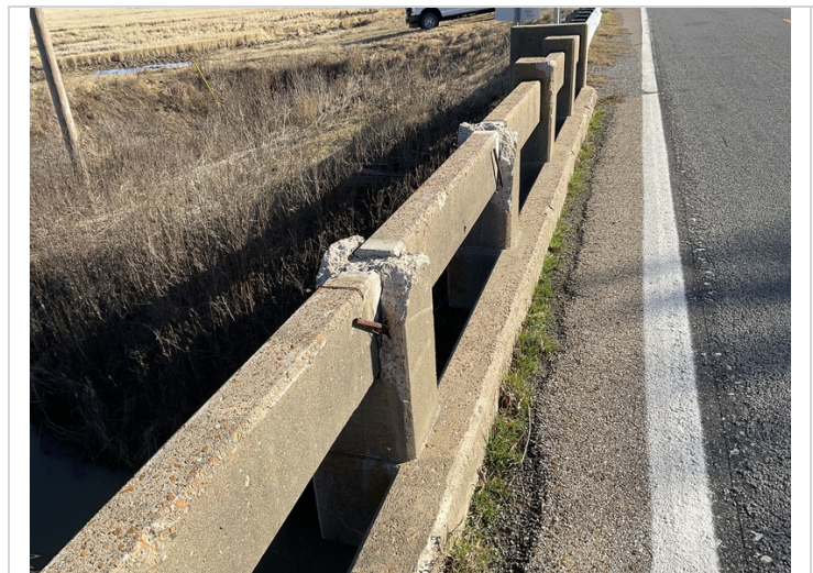
Left rail posts 1&2 are spalled with exposed rebar
