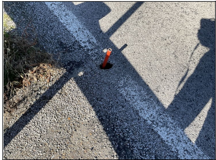
Small hole in abutment #2 right approach roadway at bridge end with small void behind backwall.
