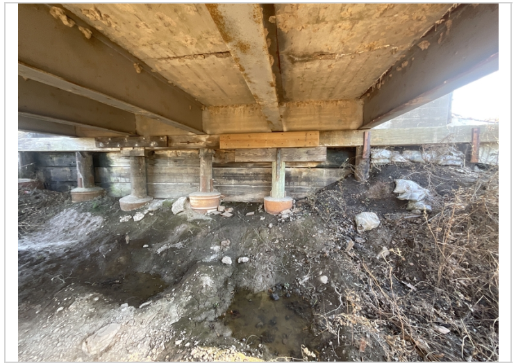
Abutment #2 cap repaired
