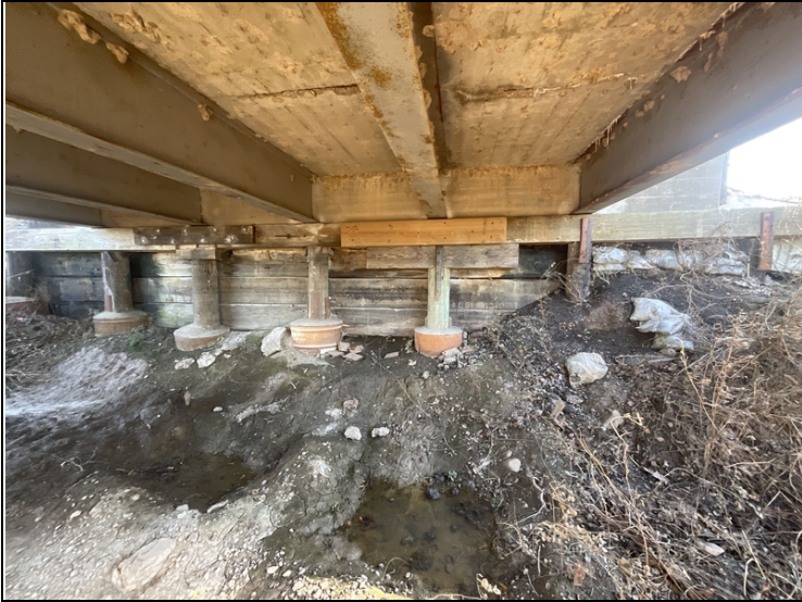
Abutment #2 cap repaired
