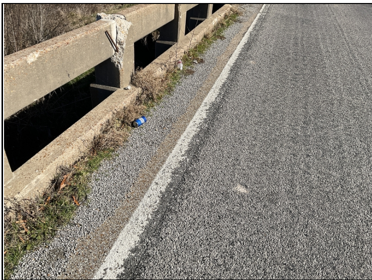
Debris and vegetation in gutters
