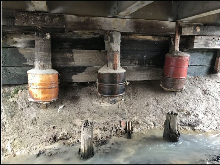
Voids starting under and behind abutment #1 back wall between piles #2,4.
