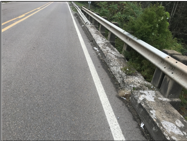
Typical heavily scaled curb.
