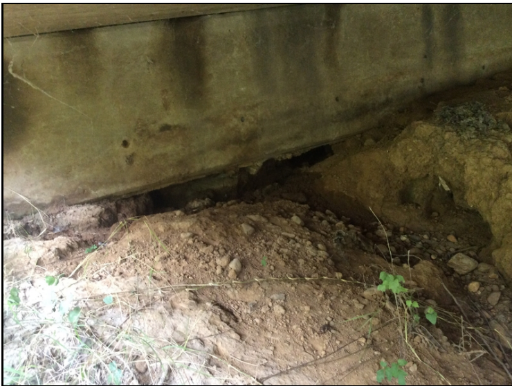
Abutment #2 left side erosion.
