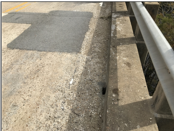
Right shoulder full length has moderate scaling with loose aggregate.
