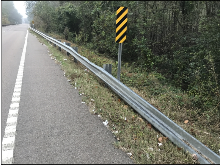
Abutment #2 left approach rail damage and 2 rail posts not connected.
