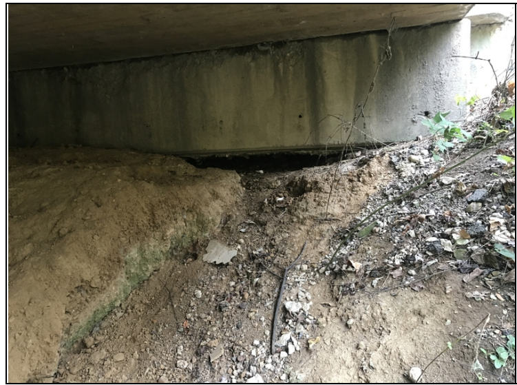
Abutment #1 cap left side undermined.
