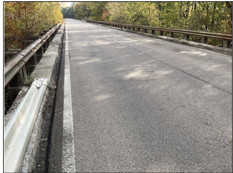
Typical deck asphalt overlay
