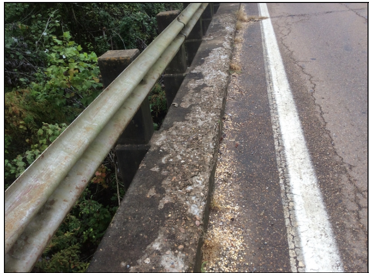
Typical curb condition spans #1-7 left and right sideline
