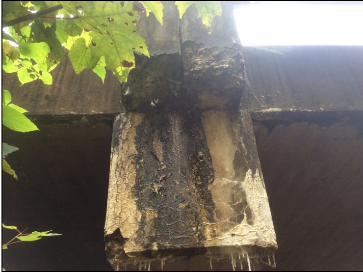
Typical cap end and bent #2 guard rail post bottoms
