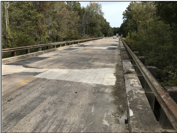
Gutters have moderate scaling full length.
