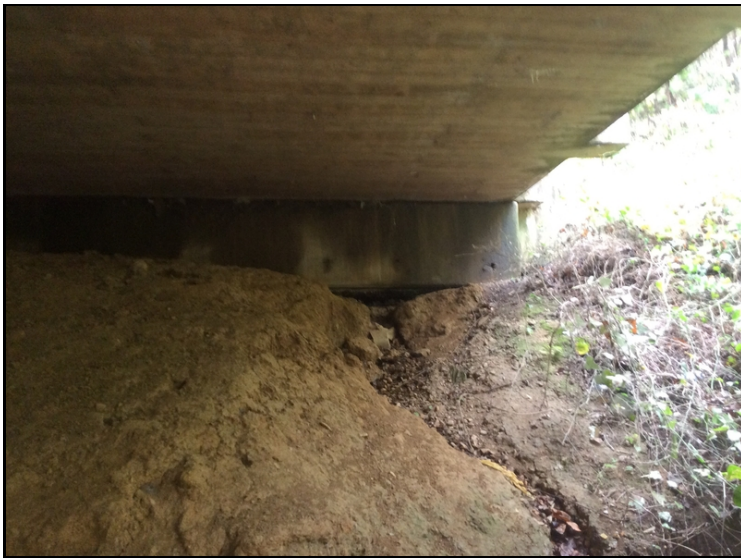
Abutment #1 left side erosion
