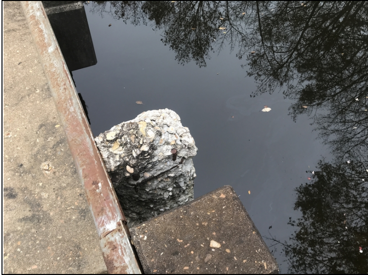
Span #9 at bent #10 left rail post spalled with exposed rebar.
