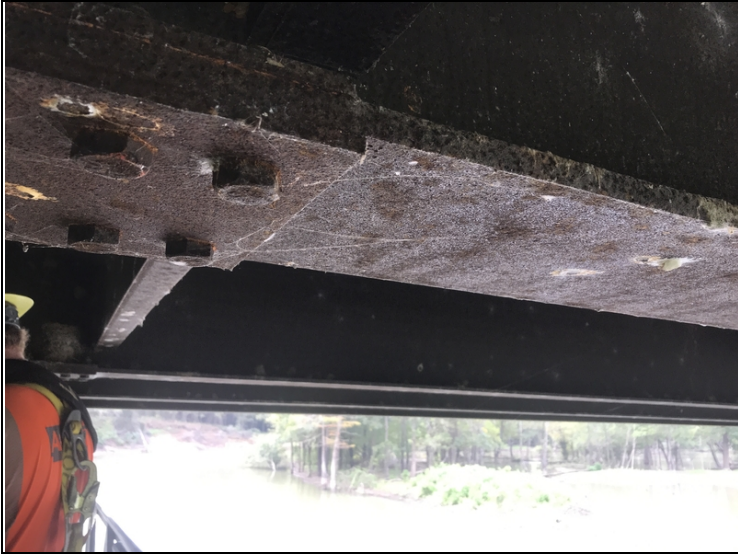
Span #6 girder #3 splice bolt has been tightened.
