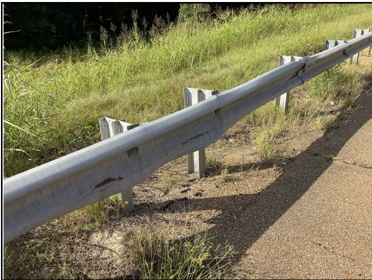
Abutment #1 right approach rail collision damage
