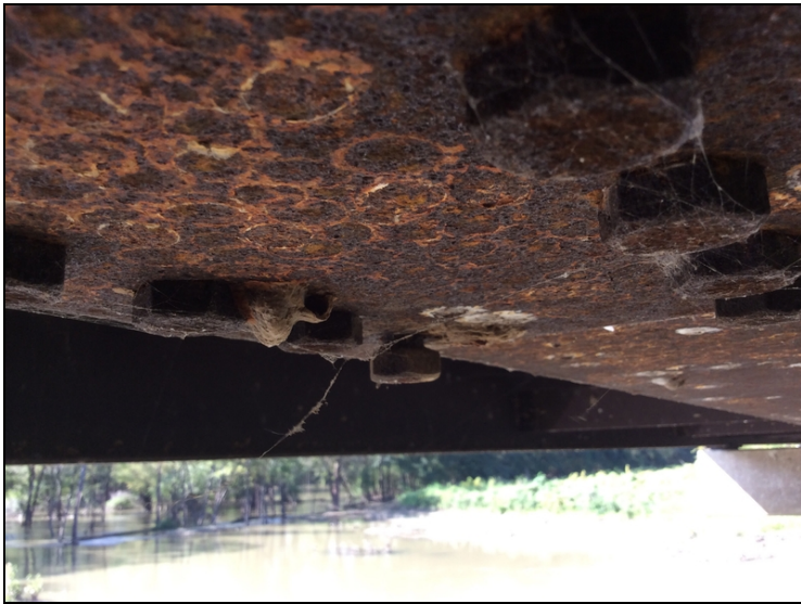
Span #5 girder #5 bottom splice bolt loose and backed out.
