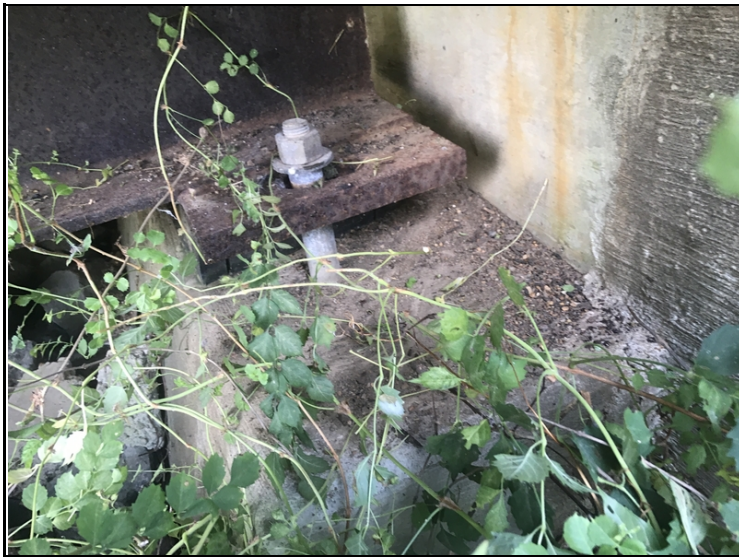
Abutment #1 girder #1 left anchor nut has been tightened.
