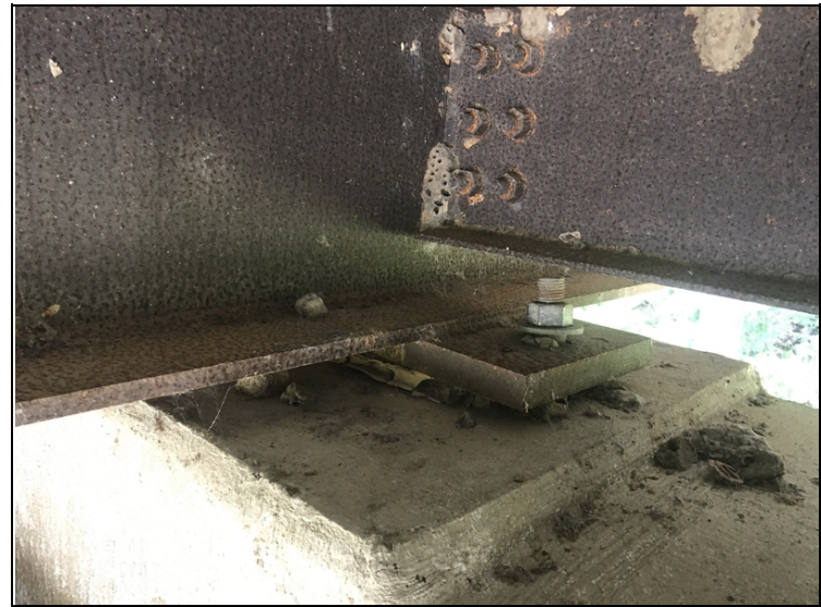
Span #6 girder #4 right anchor nut has been tightened.
