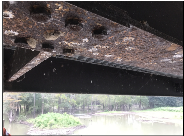
Span #5 girder #5 splice bolt has been tightened.
