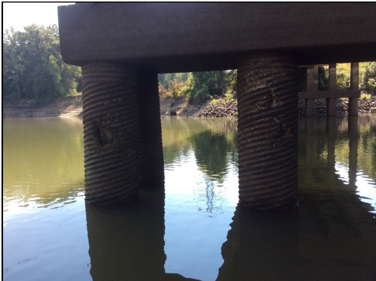
Typical voids in concrete surrounding piles.
