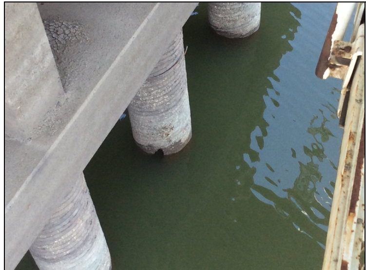
Void in concrete bent 6 pile encasement.
