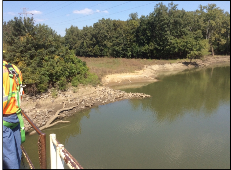
Abutment 2 right bank 60' from abutment 2 is eroding.
