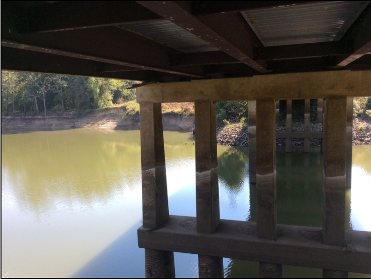
Abutment 1 right side bank is eroding within 50' of bridge.
