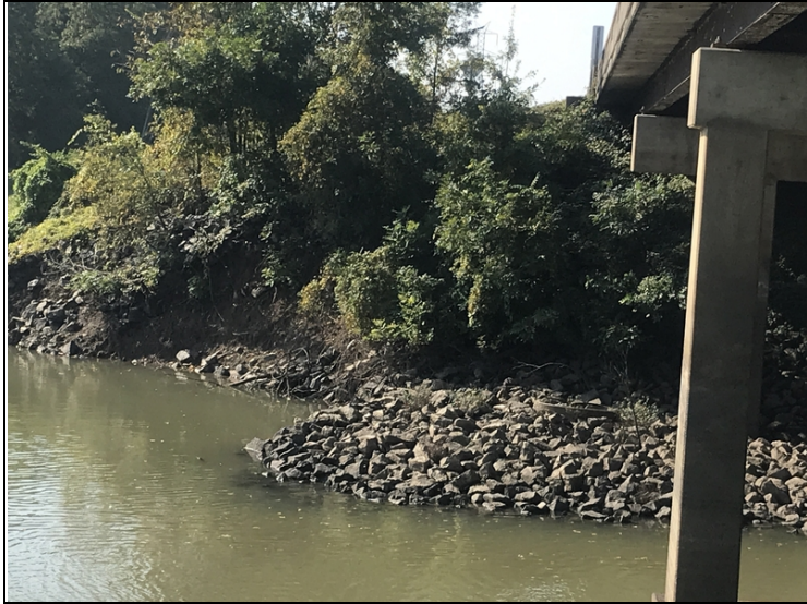
Slope erosion at abutment #1 right side.
