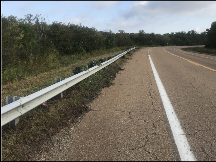
Abutment #2 left side approach rail has minor collision damage 70' from bridge end.
