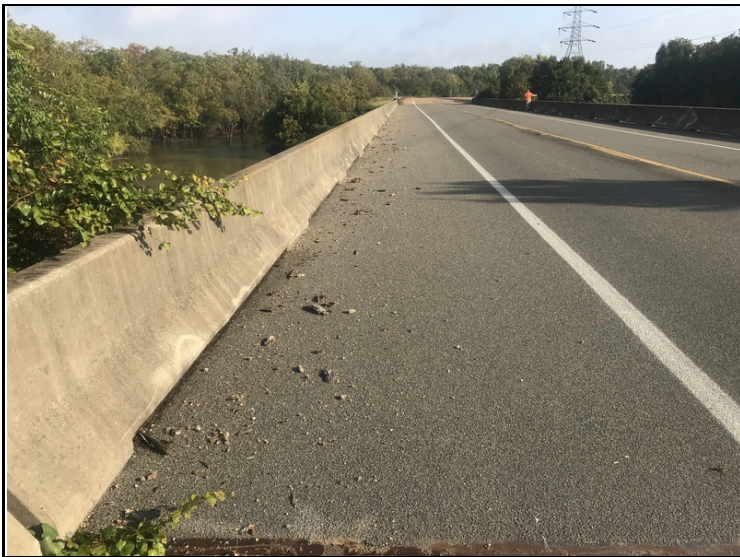
Debris in gutters.
