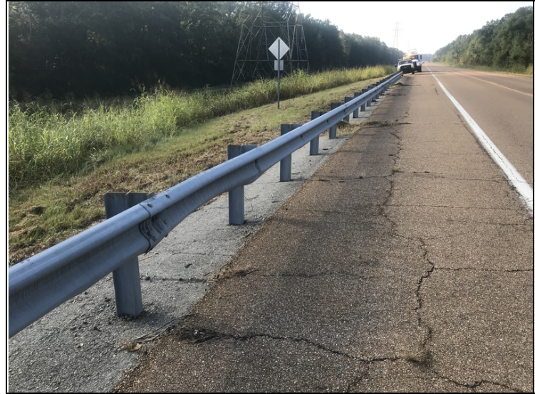
Abutment #1 right approach rail has several areas of minor collision damage.
