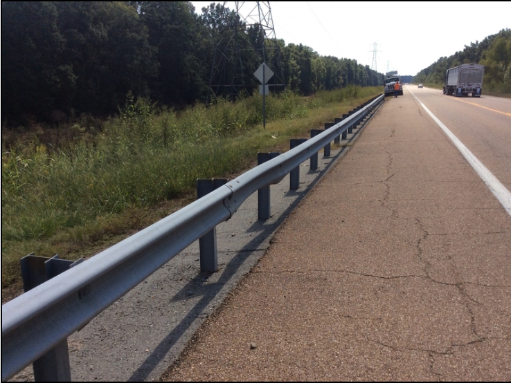
Abutment 1 right approach rail damage.
