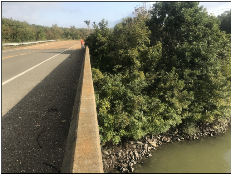
Trees and vegetation growing beside, under and onto bridge abutment #2 right side.
