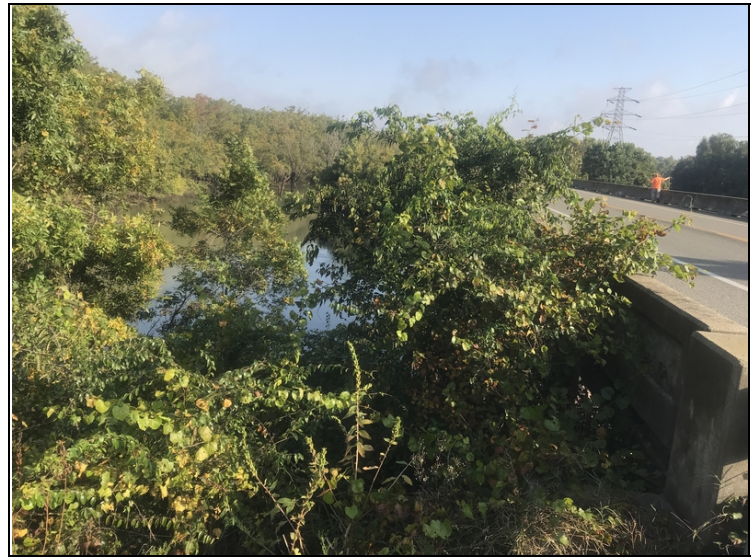
Trees and vegetation growing beside and under bridge abutment #1 left side.
