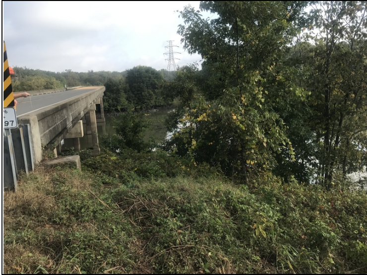
Trees and vegetation growing beside and under bridge abutment #1 right side.
