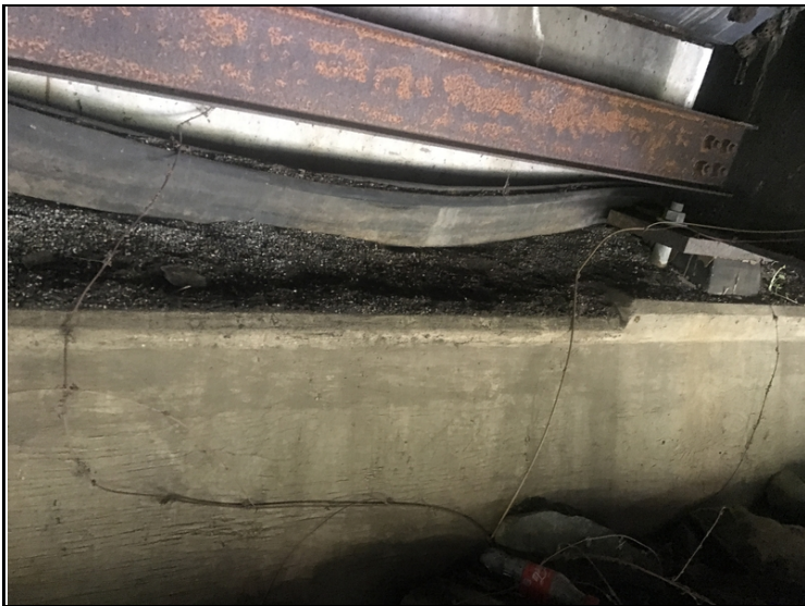
Dirt and debris on abutment #2 cap, typical of abutment #1.
