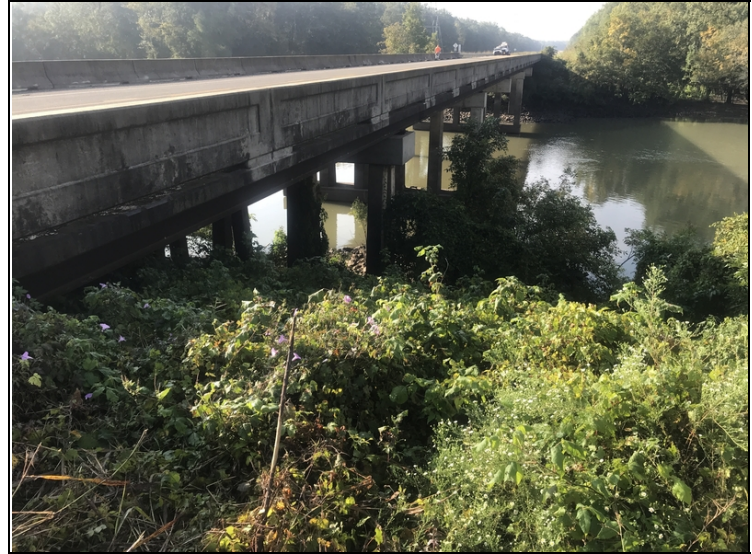
Trees and vegetation growing beside and under bridge abutment #2 left side.
