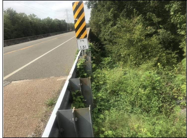
Trees and vegetation growing beside, under and onto bridge abutment #2 left side.
