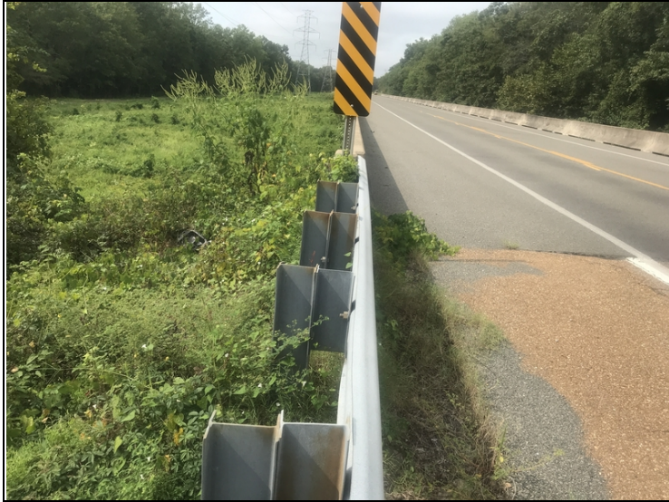
Vegetation growing beside and under and onto bridge abutment #2 right side.
