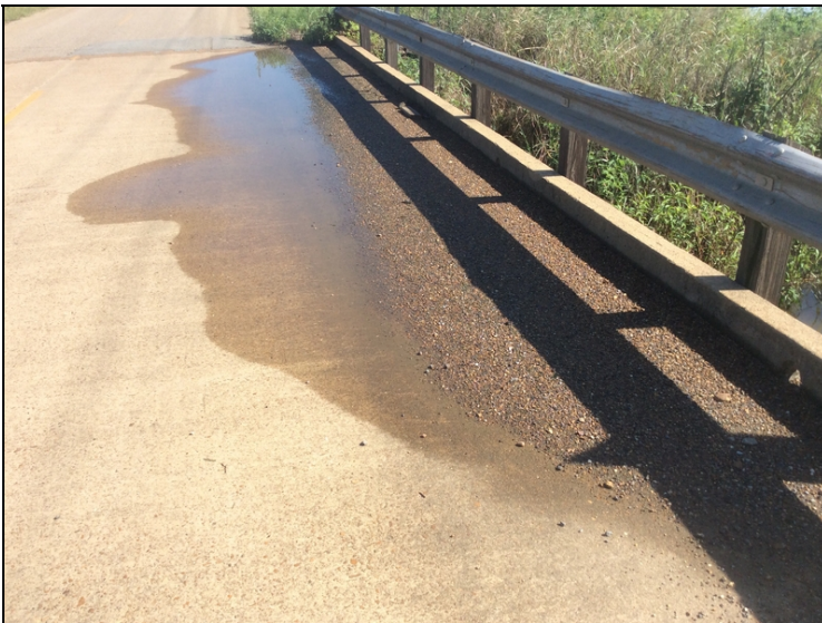
Gutters have dirt and debris.
