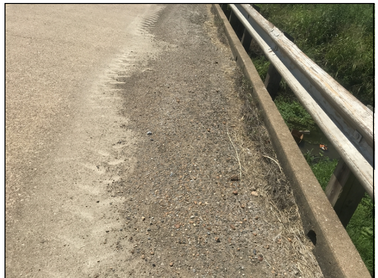
Dirt and gravel in gutters.
