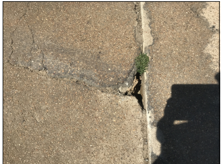
Abutment #1 approach roadway right lane has hole with void underneath.
