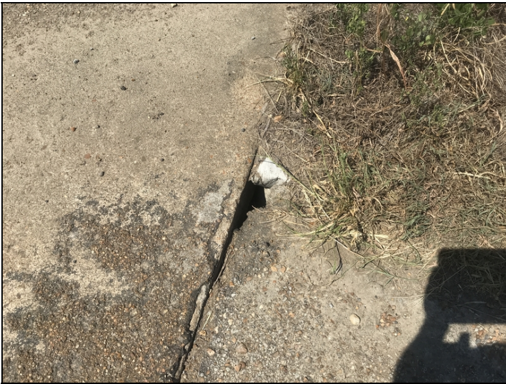
Hole in abutment #2 left shoulder with void.
