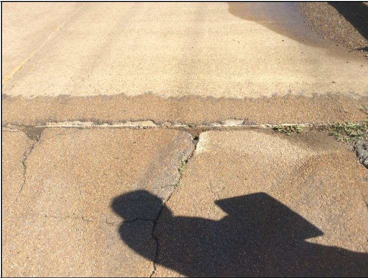
Abutment #1 approach roadway has settled with small void underneath increasing impact loading on bridge.
