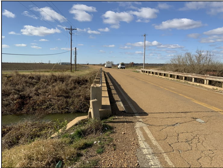
Abutment #2 right flair board missing.
