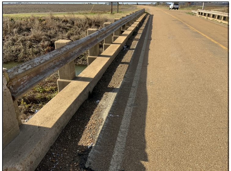
Dirt and debris in gutters.
