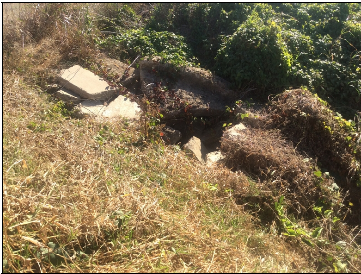
Abutment #2 right side erosion under rubble
