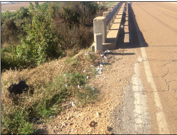
Abutment #2 right approach rail gone
