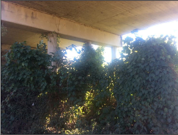
Vegetation growing under bridge and up piles bent #4
