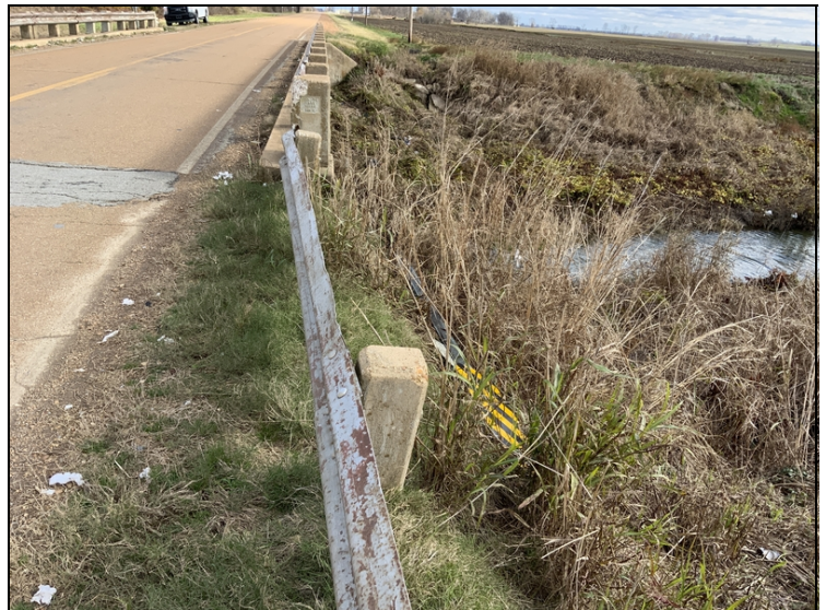
Abutment #1 right flair board and log mile sign knocked.
