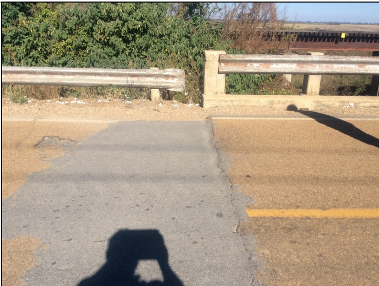
Abutment #1 approach roadway settled left lane
