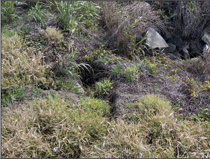
Slope erosion at abutment #2 right side 10' +/- from bridge end.
