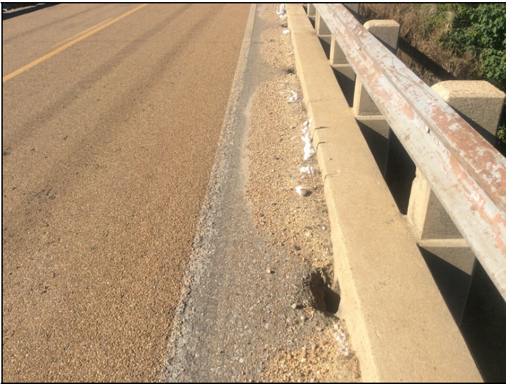
Gutters full of dirt and debris
