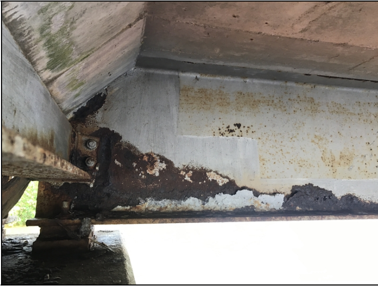
Bent #2 span#2 girder #1 first three feet of girder web has up to 75% section loss.
