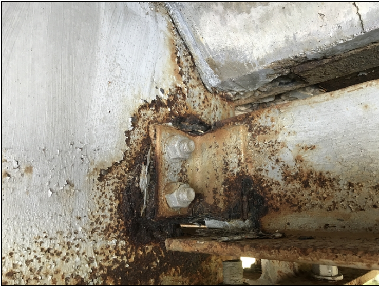
Bent #2 span #2 girder #3 has area around diaphragm condition with a three inch hole above and below diaphragm.
