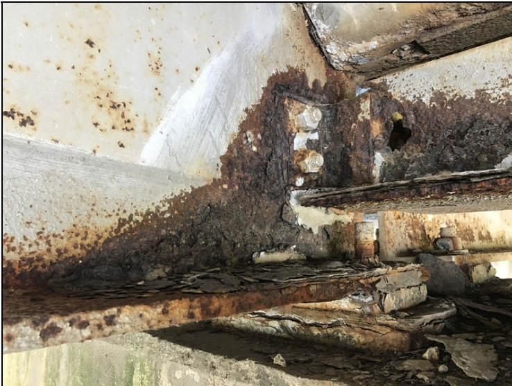
Span #4 bent #5 girder #3 web around diaphragm connection and lower flange first foot has section loss up to 75%.
