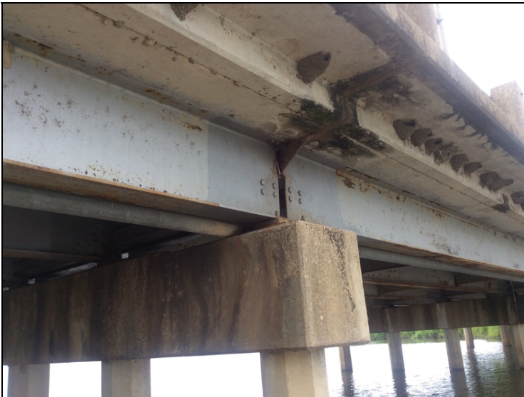
Bent #3 span #2 girder #5 anchor nut missing typical of other locations.
