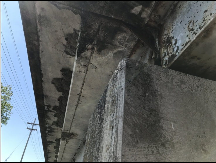
Bent #3 ahead face right top corner is cracked.
