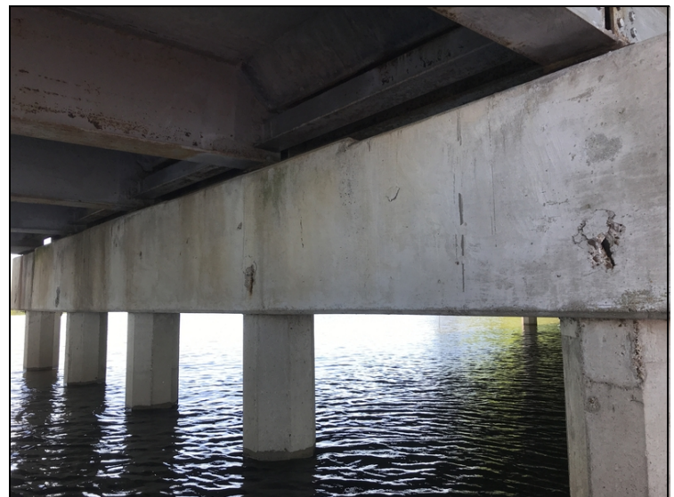
Bent #4 cap has four 1' spalls on ahead face with exposed rebar with 5% section loss.
