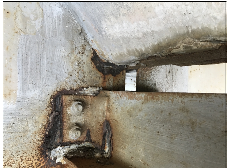
Span #3 bent #4 girder #3 has one inch hole in web at haunch and up to 75% section in web around diaphragm connection.
