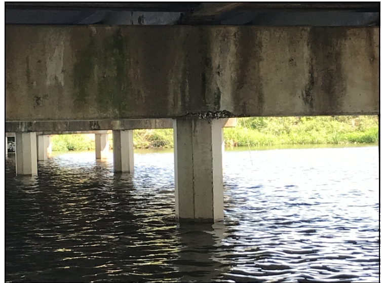
Bent #2 back face above pile #3 at bottom has 1' honey comb and 2' of delamination and cracking.
