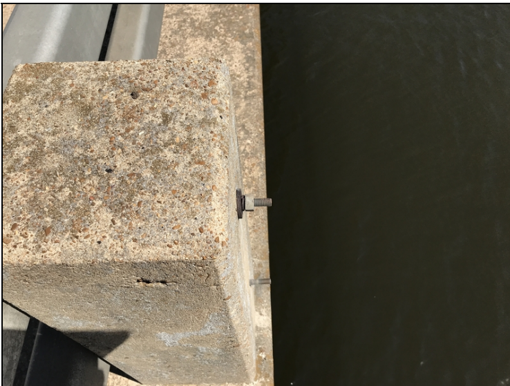
Typical rail nut missing
