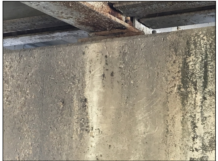
Bent #3 cap back face under girder #2 has vertical crack one foot long.
