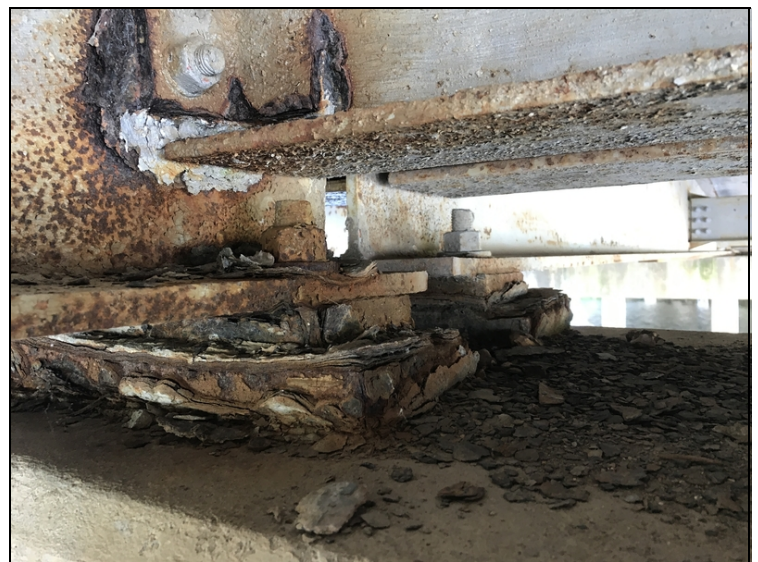
Typical bent bearings
