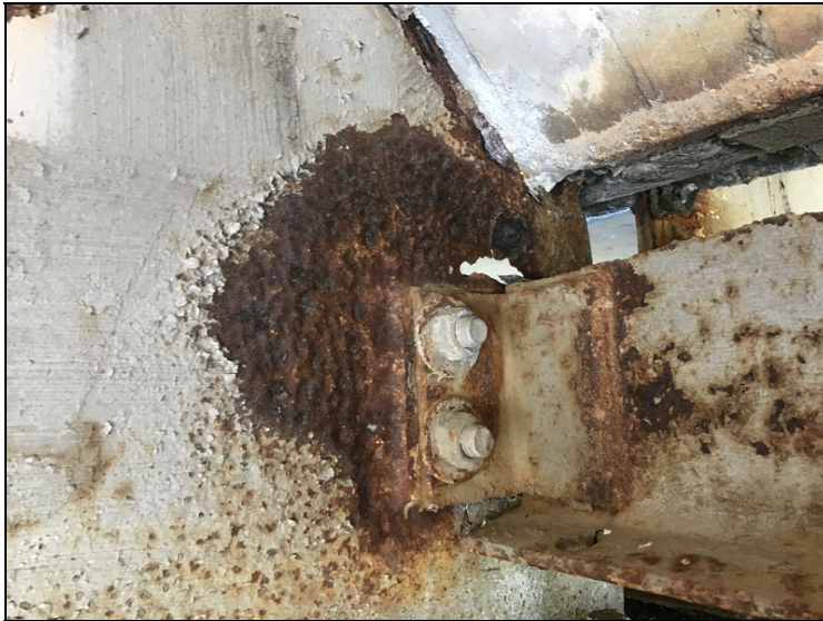
Span #4 bent #5 girder #4 web at diaphragm connection has large section loss with a three inch hole and a pin hole.
