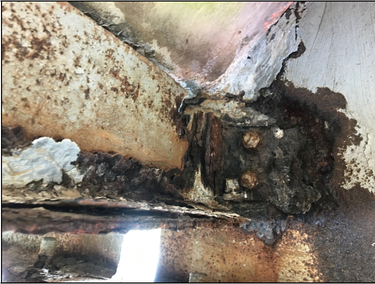
Span #3 bent #4 girder #5 web at diaphragm connection has up to 80% section loss.
