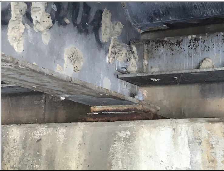
Typical abutment bearing.
