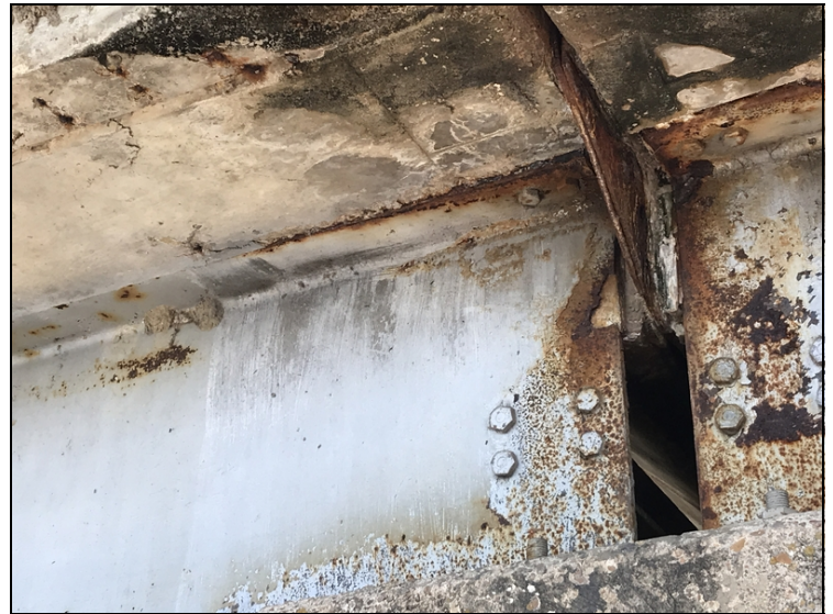
Span #2 bent #3 girder #5 web at top on end has a three inch area on outside that is rusted off.
