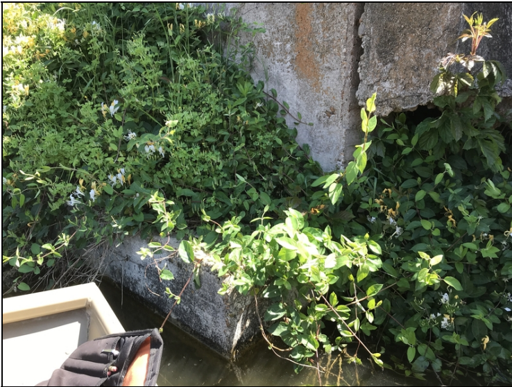
Abutment #2 left wing footing is exposed full length.
