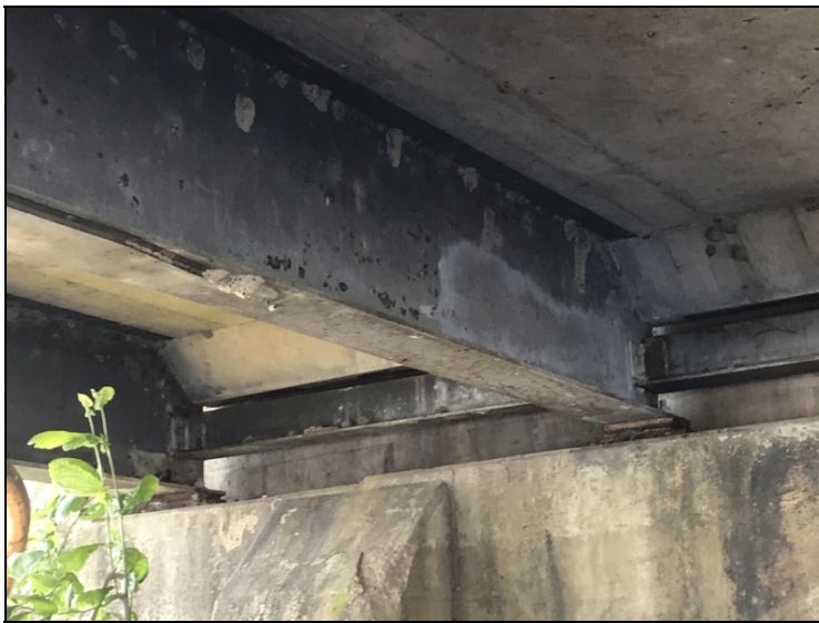
Typical girder ends that have been painted
