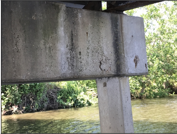
Bent #2 cap has 2 small pop outs on ahead face left end above pile #1 with exposed rebar no section loss.
