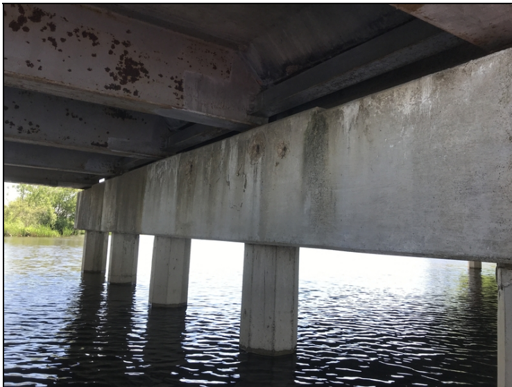
Bent #5 cap ahead face has 2' of delaminations and four 1' spalls with exposed rebar with no section loss.
