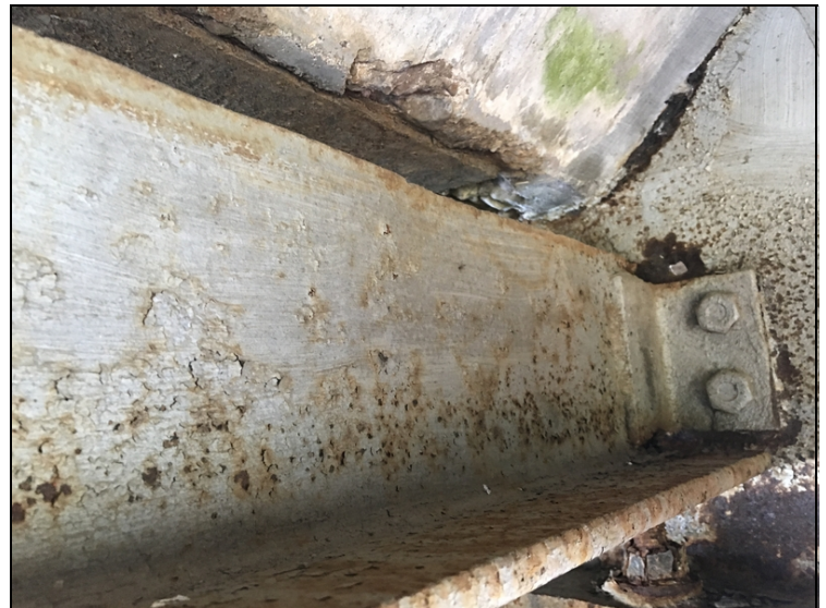
Span #2 bent #3 girder #3 has large section loss around diaphragm with a one inch hole in web.
